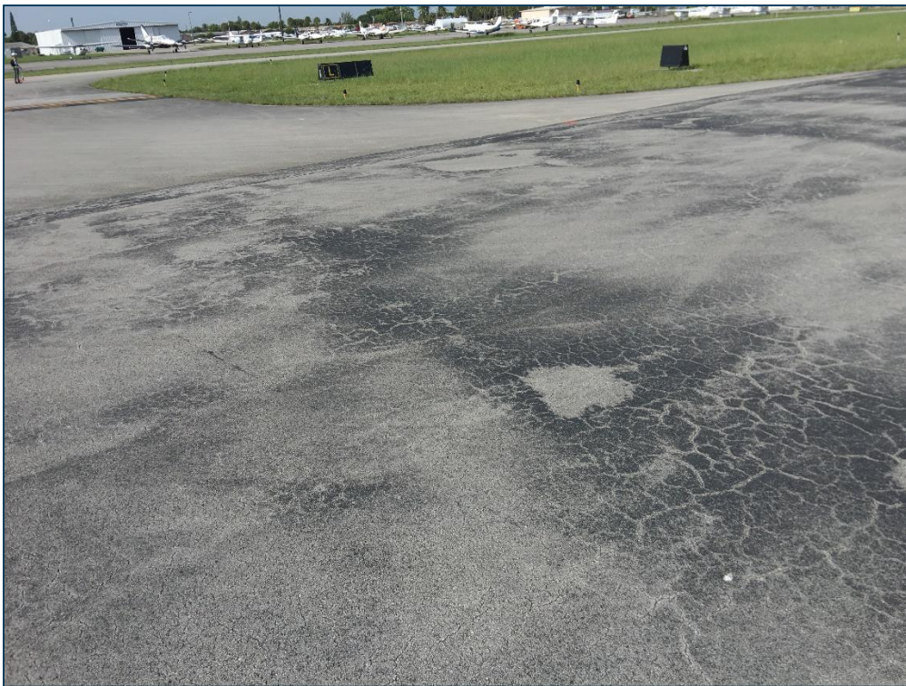
RW 10R-28L, Section 6405, Sample Unit 159 - Low Severity (43) Block Cracking, Low Severity (48) Longitudinal & Transverse Cracking, Low Severity (52) Raveling, and Low Severity (57) Weathering
