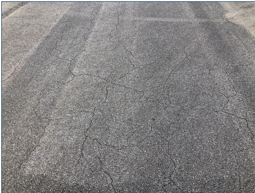
AP SOUTH, Section 4105, Sample Unit 309 - Low Severity (43) Block Cracking, Low Severity (50) Patching, and Low Severity (52) Raveling
