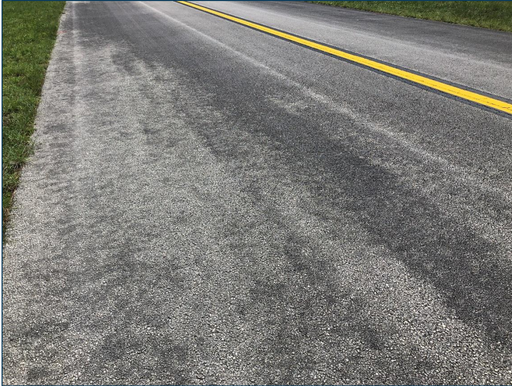
TW E, Section 565, Sample Unit 109 - Low Severity (52) Raveling and Low Severity (57) Weathering
