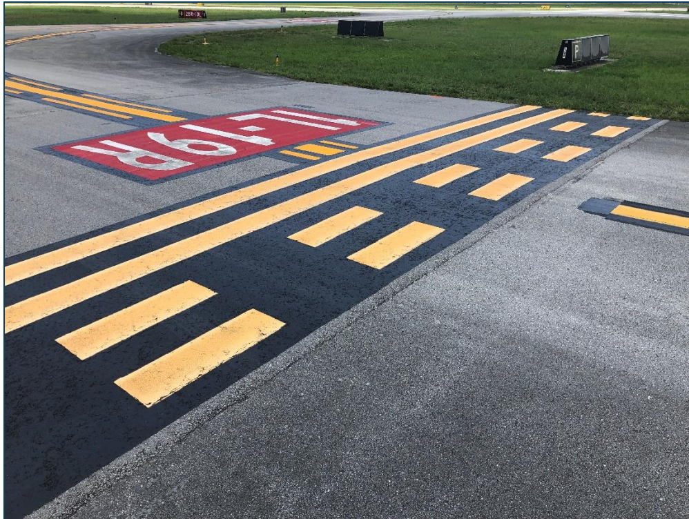
TW P, Section 1602, Sample Unit 99 - Low Severity (48) Longitudinal & Transverse Cracking, Low Severity (50) Patching, and Low Severity (57) Weathering
