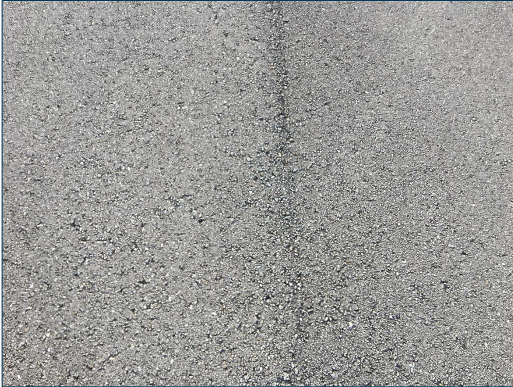
RW 10L-28R, Section 6205, Sample Unit 95 - Low Severity (57) Weathering
