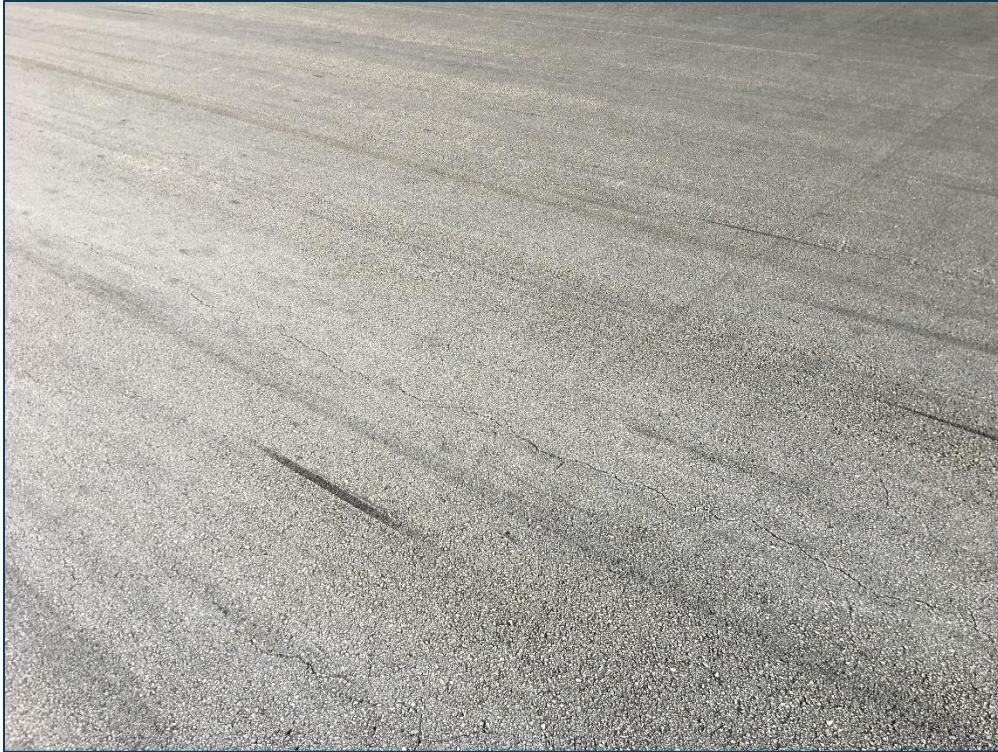
RW 10R-28L, Section 6405, Sample Unit 112 - Low Severity (48) Longitudinal & Transverse Cracking, Low Severity (52) Raveling, and Low Severity (57) Weathering
