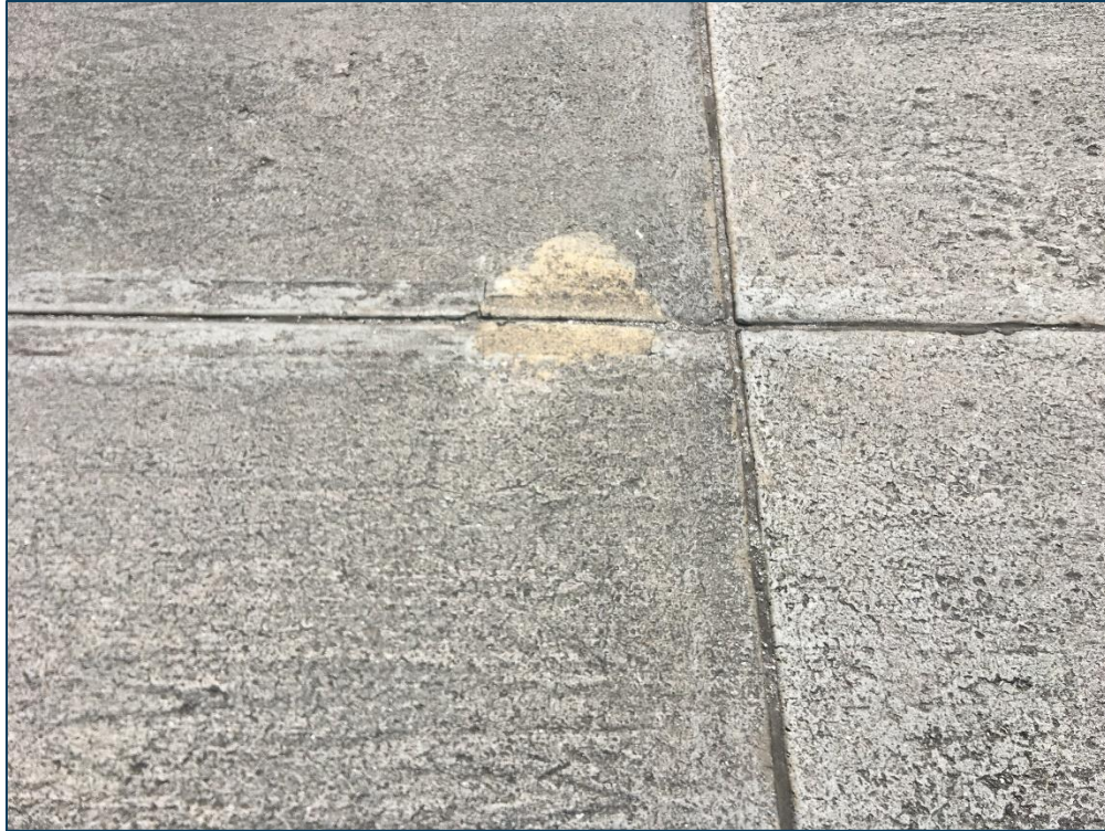
AP SOUTH, Section 4110, Sample Unit 207 - Low Severity (65) Joint Seal Damage and Low Severity (66) Small Patch
