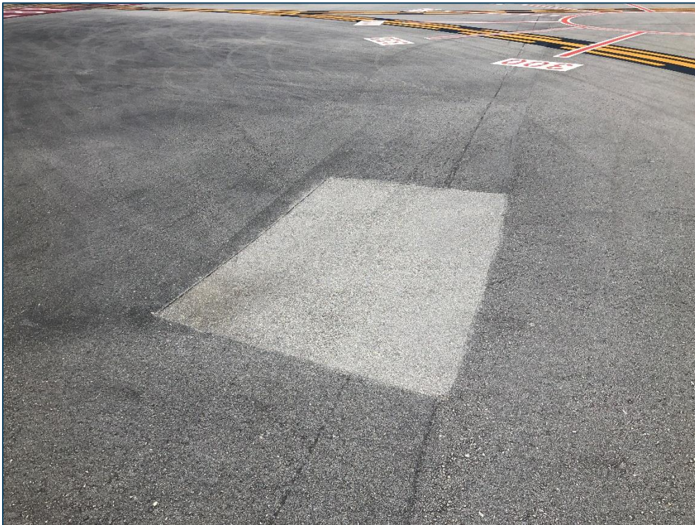
TW N, Section 1415, Sample Unit 102 - Low Severity (48) Longitudinal & Transverse Cracking, Low Severity (50) Patching, Low Severity (52) Raveling, and Low Severity (57) Weathering
