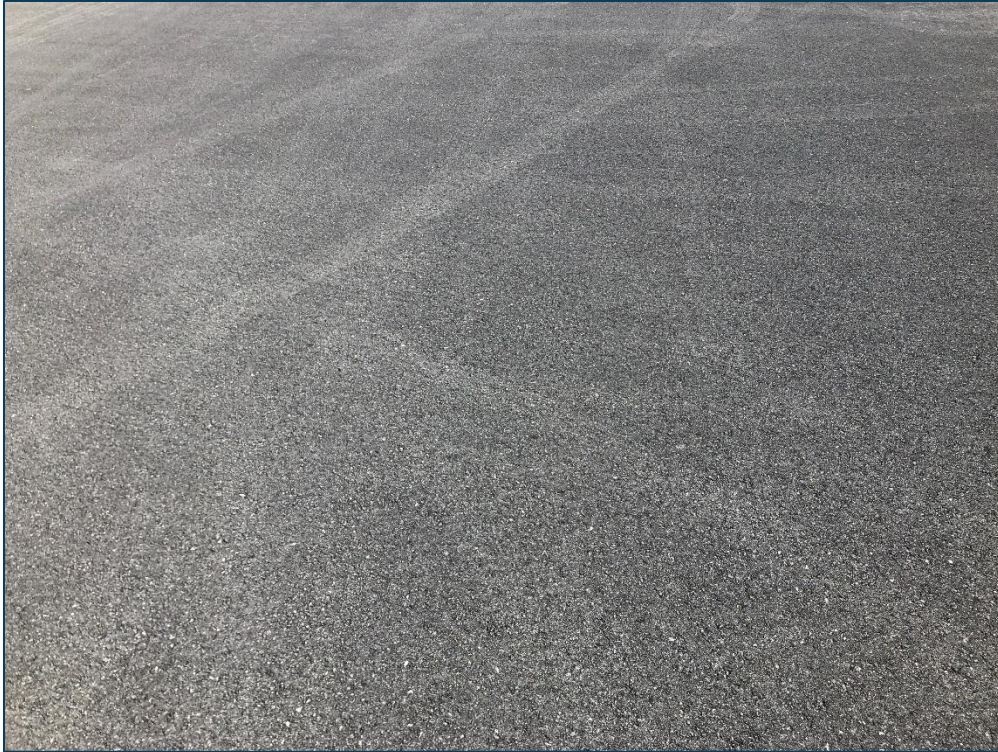
RW 01R-19L, Section 6305, Sample Unit 97 - Low Severity (57) Weathering
