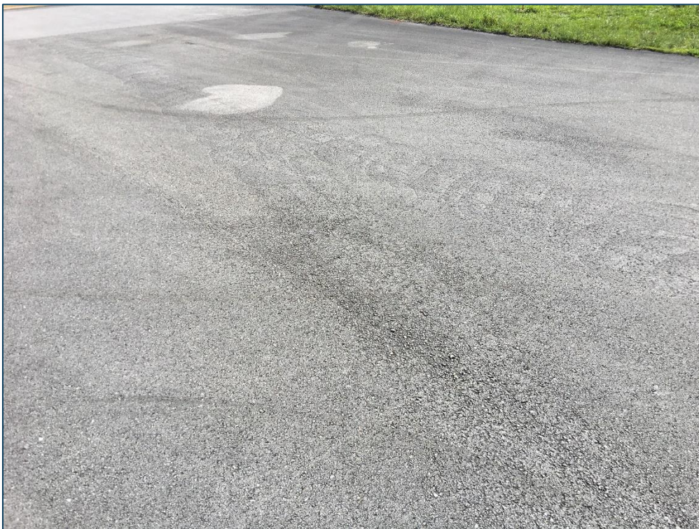
TW L, Section 1215, Sample Unit 102 - Low Severity (48) Longitudinal & Transverse Cracking, Low Severity (52) Raveling, and Low Severity (57) Weathering
