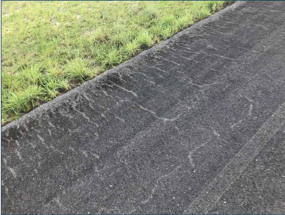
TW M, Section 2010, Sample Unit 102 - Low Severity (48) Longitudinal & Transverse Cracking and Low Severity (57) Weathering
