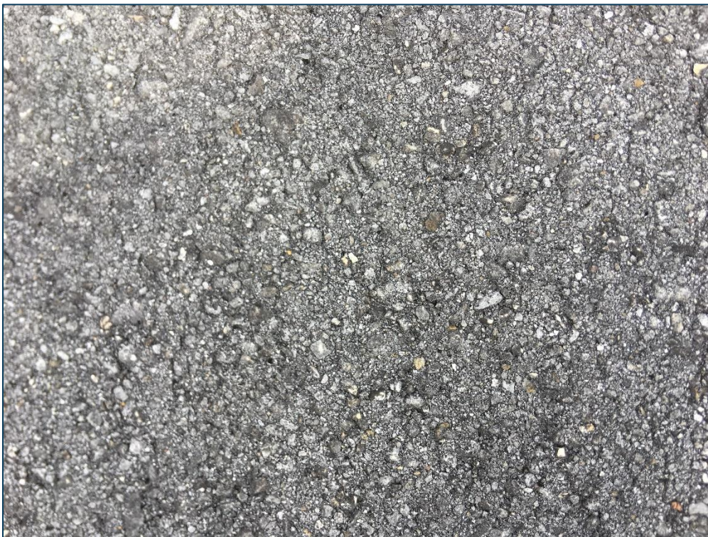
RW 01L-19R, Section 6105, Sample Unit 154 - Low Severity (57) Weathering
