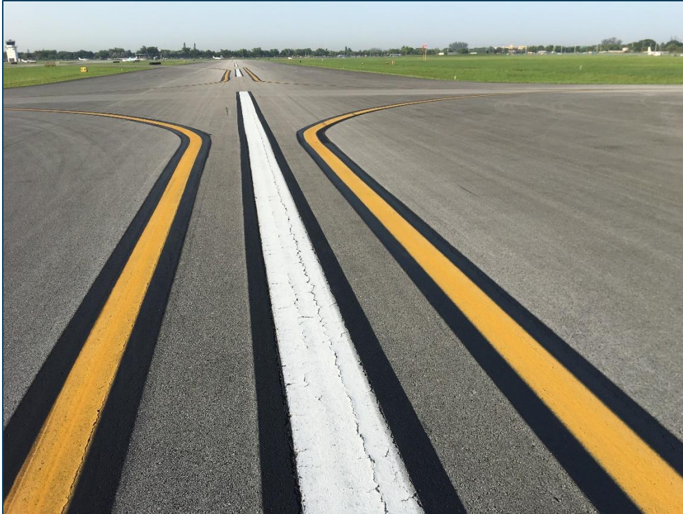
RW 01L-19R, Section 6105, Sample Unit 122 - Low Severity (57) Weathering
