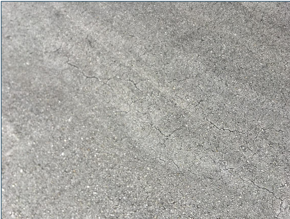
TW D, Section 403, Sample Unit 100 - Low Severity (48) Longitudinal & Transverse Cracking, Low Severity (52) Raveling, and Low Severity (57) Weathering
