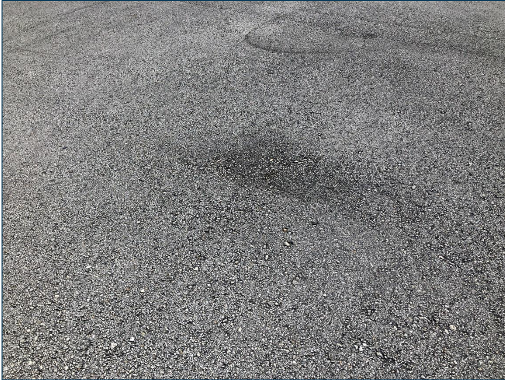
TW B, Section 202, Sample Unit 102 - Low Severity (52) Raveling
