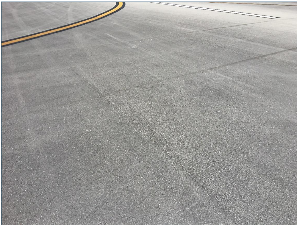
RW 01R-19L, Section 6305, Sample Unit 142 - Low Severity (57) Weathering and Medium Severity (57) Weathering
