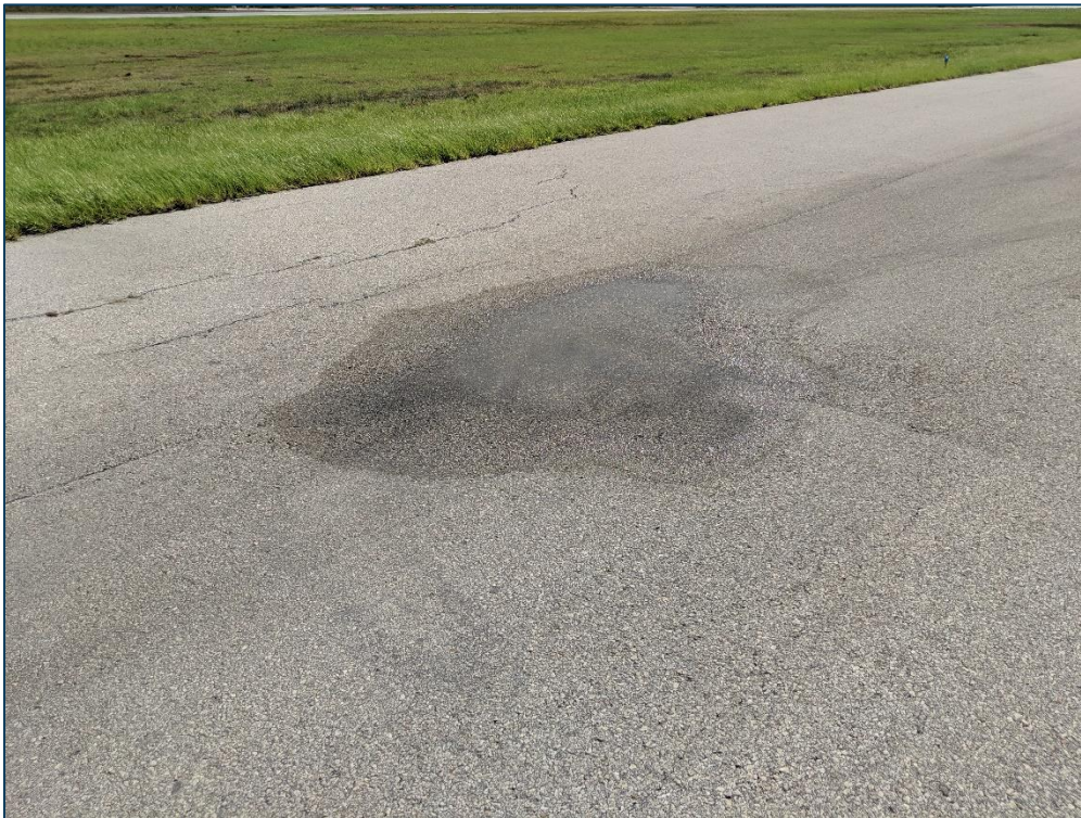
TW A, Section 110, Sample Unit 137 - Low Severity (48) Longitudinal & Transverse Cracking, Low Severity (52) Raveling, and Low Severity (57) Weathering
