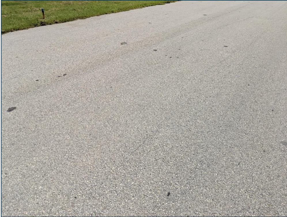
TW A, Section 105, Sample Unit 111 - Low Severity (48) Longitudinal & Transverse Cracking and Medium Severity (57) Weathering
