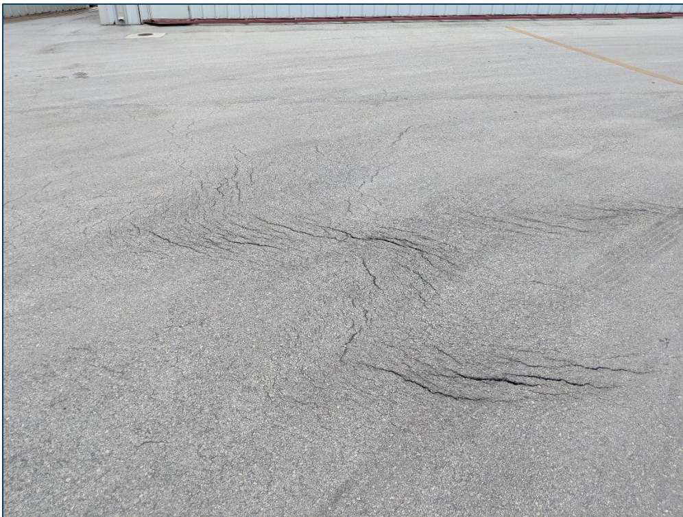
AP E, Section 4155, Sample Unit 816 - Low Severity (48) Longitudinal & Transverse Cracking, (55) Slippage Cracking, and Low Severity (57) Weathering
