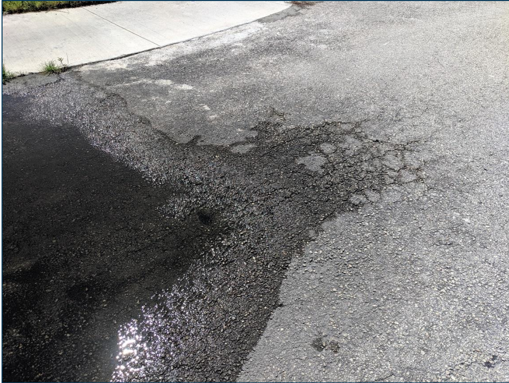
AP W, Section 4205, Sample Unit 102 - Low Severity (41) Alligator Cracking, Low Severity (45) Depression, and Low and Medium Severity (52) Raveling
