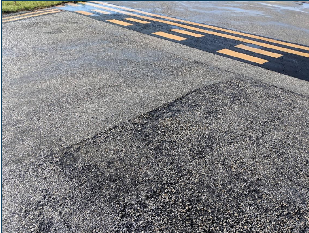
TW B, Section 210, Sample Unit 401 - Low Severity (48) Longitudinal & Transverse Cracking, Low Severity (52) Raveling, and Medium Severity (52) Raveling
