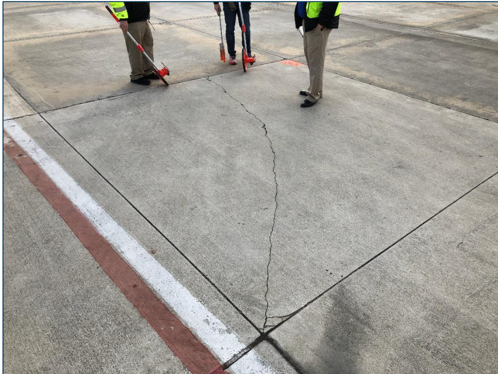
AP TERM, Section 4110, Sample Unit 153 - Medium Severity (63) Linear Cracking, Low Severity (65) Joint Seal Damage, Medium Severity (75) Corner Spall
