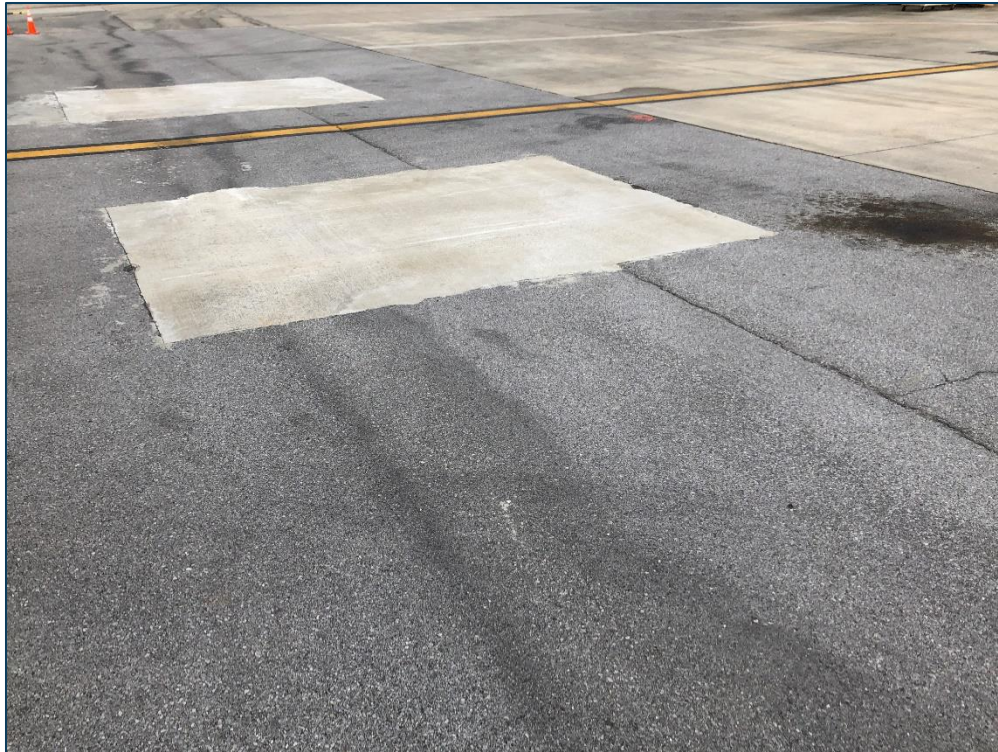
AP TERM, Section 4105, Sample Unit 301 - Low Severity (45) Depression, Low Severity (48) Longitudinal & Transverse Cracking, Medium Severity (48) Longitudinal & Transverse Cracking, Low Severity (50) Patching, Low Severity (52) Raveling, and Low Severity (57) Weathering
