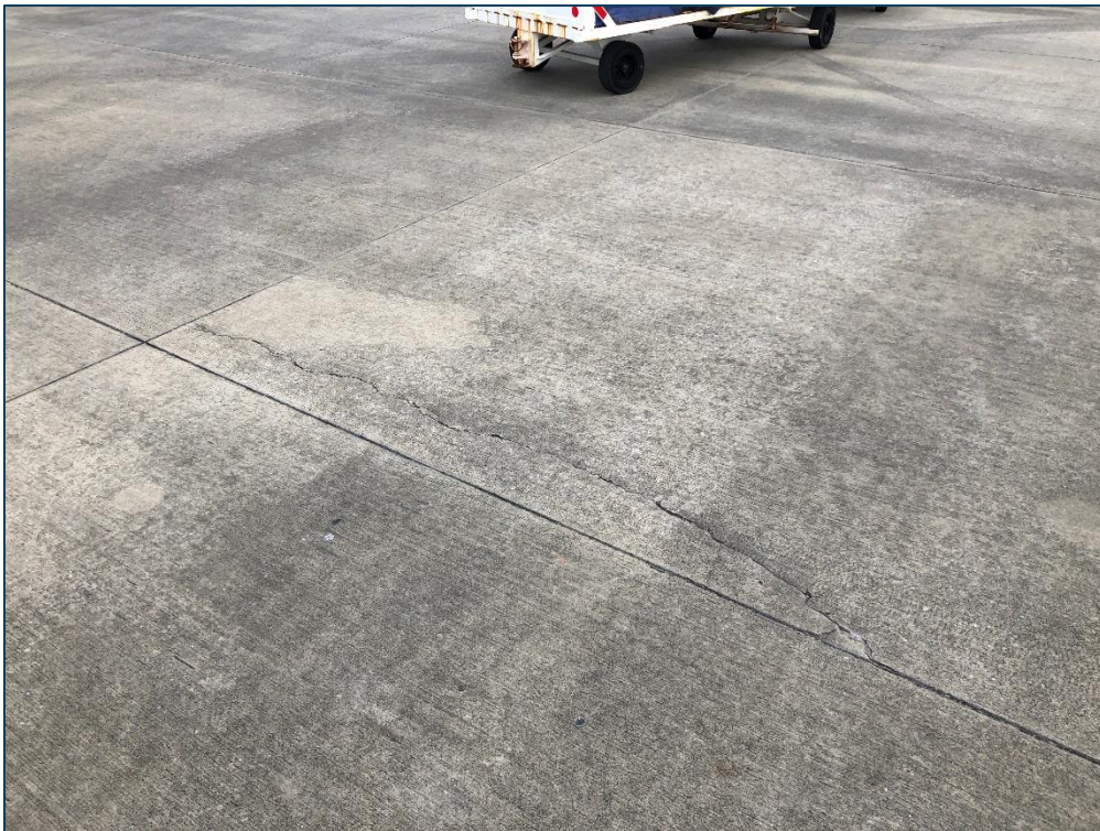
AP TERM, Section 4120, Sample Unit 304 - Low Severity (63) Linear Cracking
