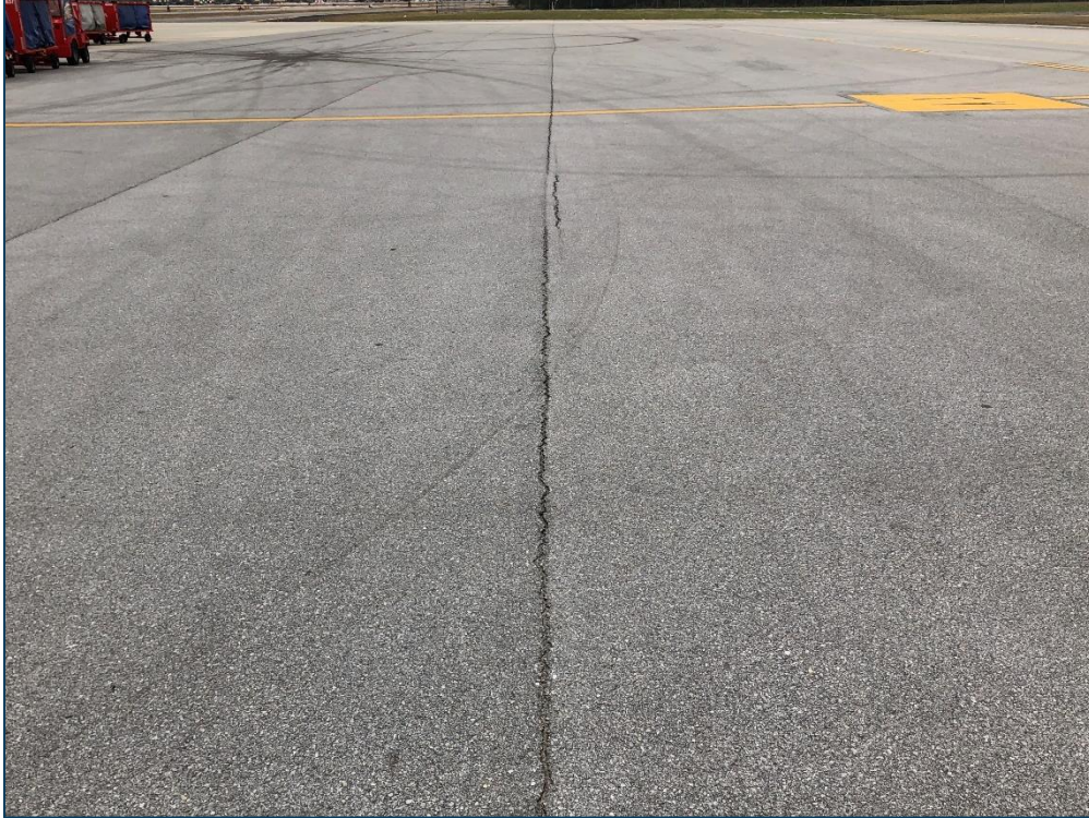
AP TERM, Section 4105, Sample Unit 203 - Medium Severity (48) Longitudinal & Transverse Cracking, Low Severity (52) Raveling, and Low Severity (57) Weathering
