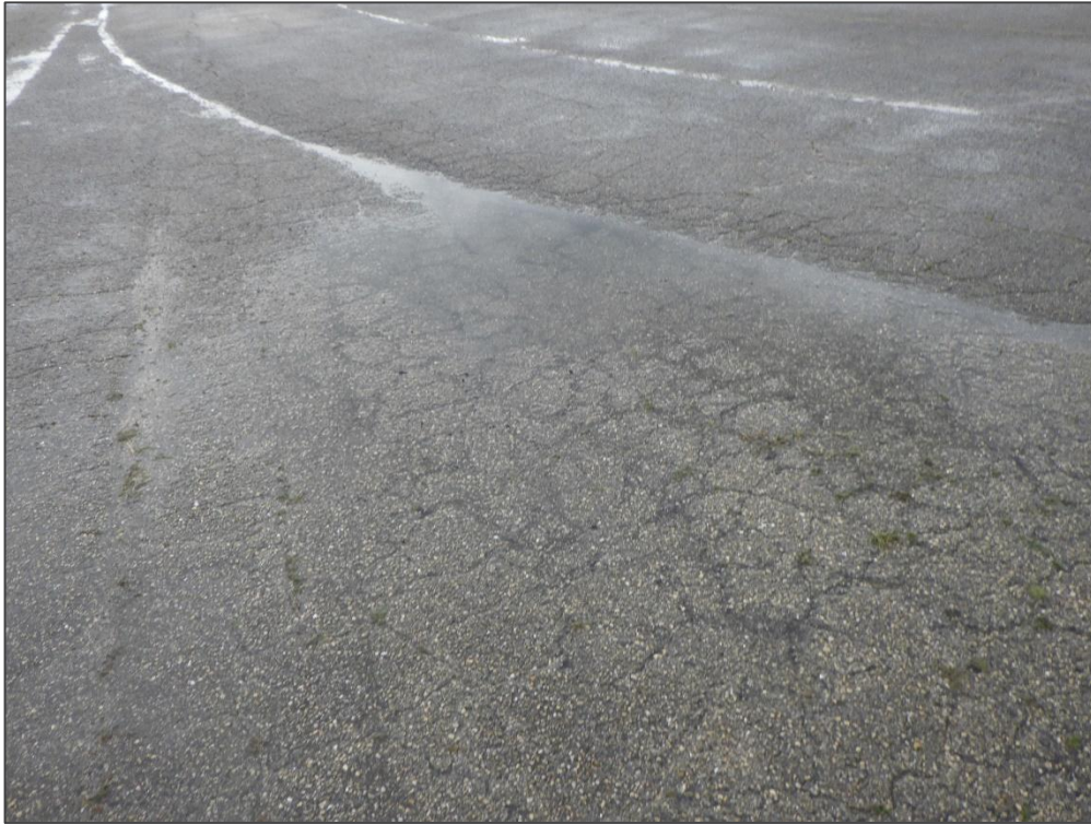
TW HANG, Section 405, Sample Unit 103 - Alligator Cracking and Depression
