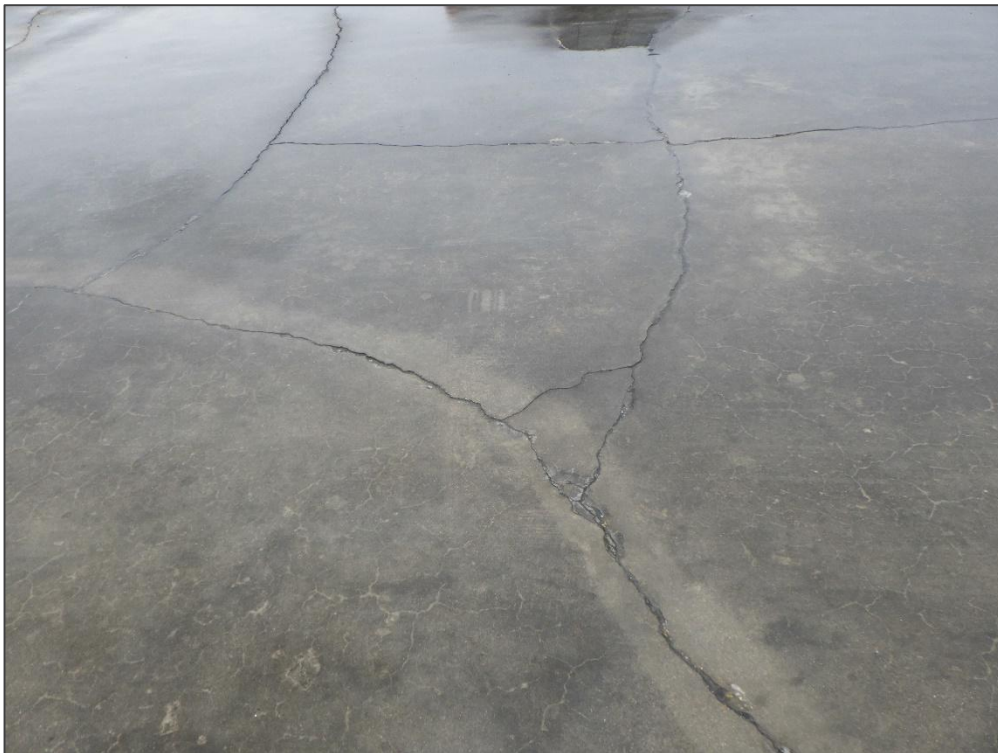
AP NW, Section 4410, Sample Unit 100 - Shattered Slab
