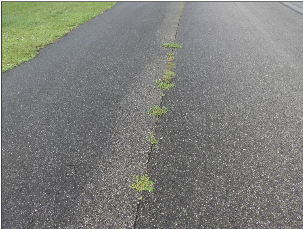
TW A, Section 105, Sample Unit 113 - Longitudinal & Transverse Cracking
