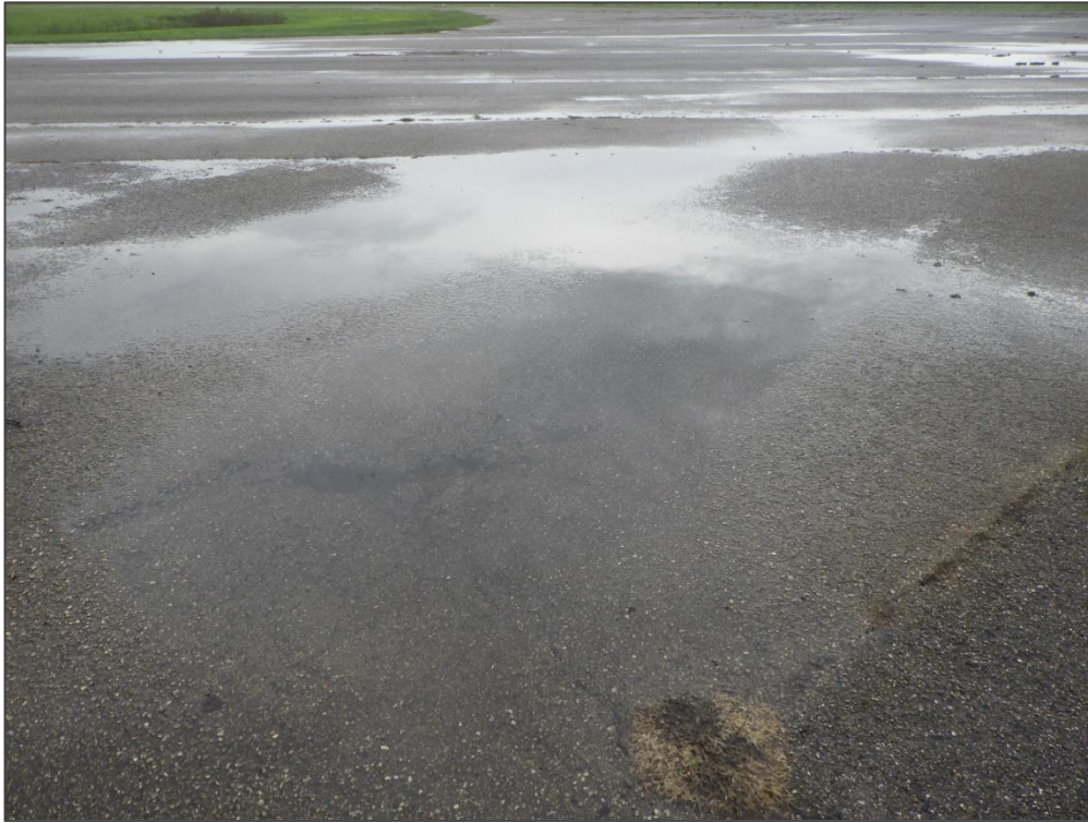
AP S, Section 4305, Sample Unit 201 - Depression
