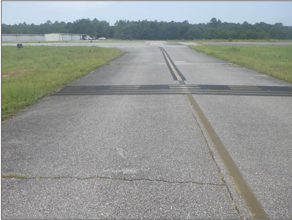
TW B, Section 290, Sample Unit 100 - Longitudinal & Transverse Cracking
