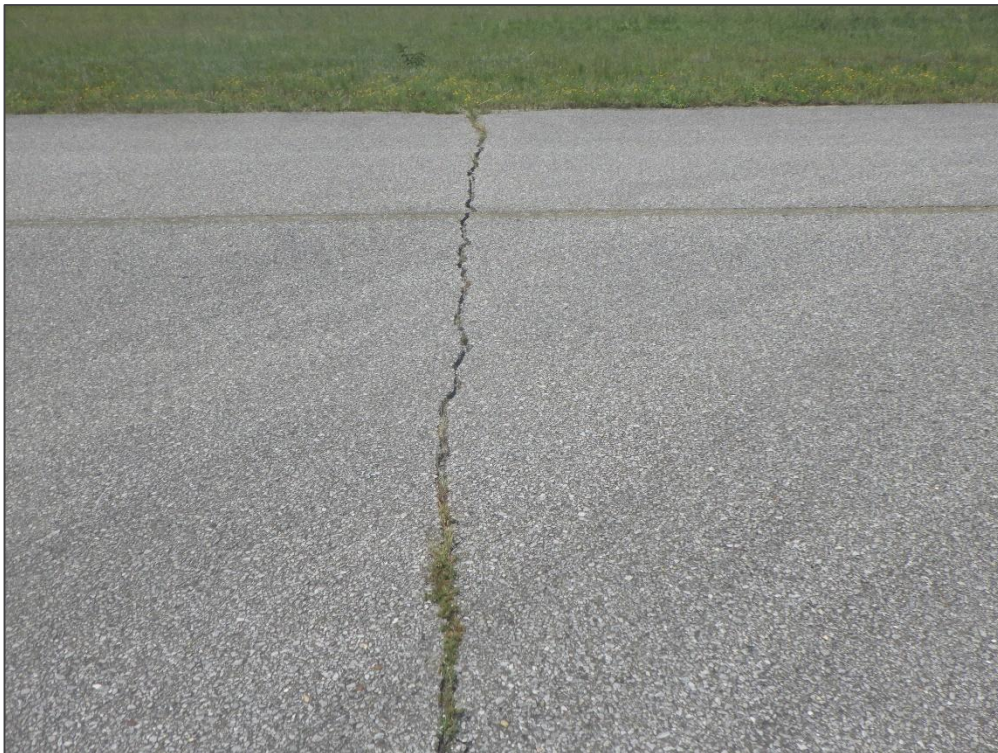
TW B, Section 205, Sample Unit 118 - Longitudinal & Transverse Cracking
