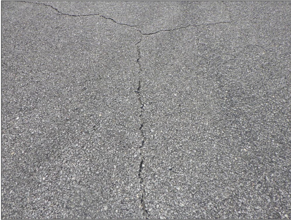
AP W, Section 4115, Sample Unit 502 - Longitudinal & Transverse Cracking
