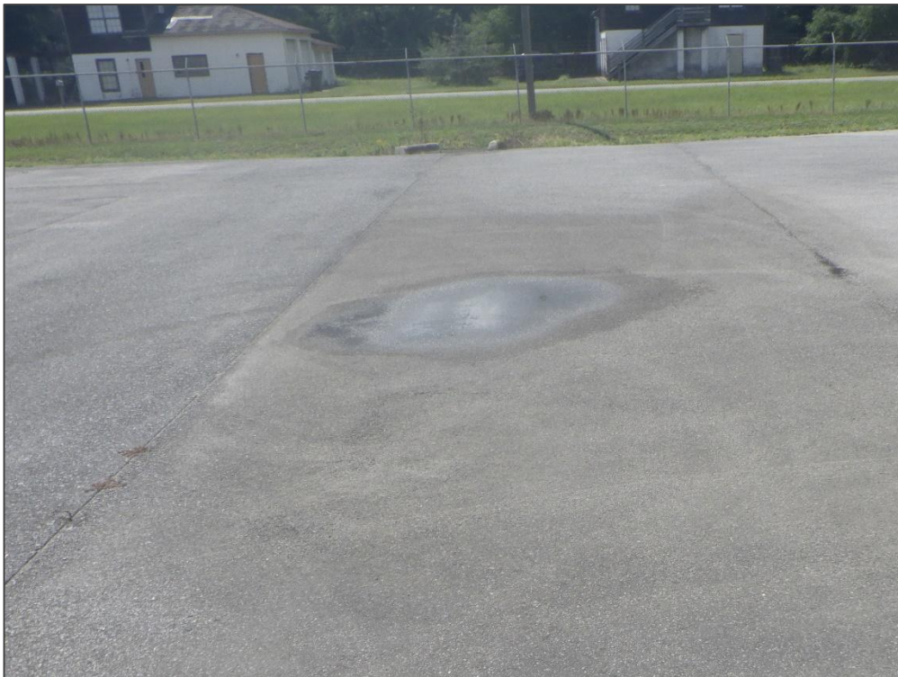
AP W, Section 4130, Sample Unit 700 – Depression
