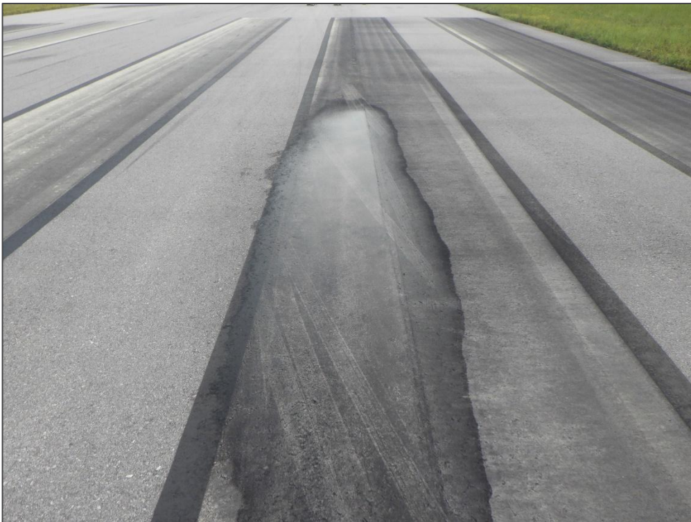
RW 18-36, Section 6105, Sample Unit 171 - Depression
