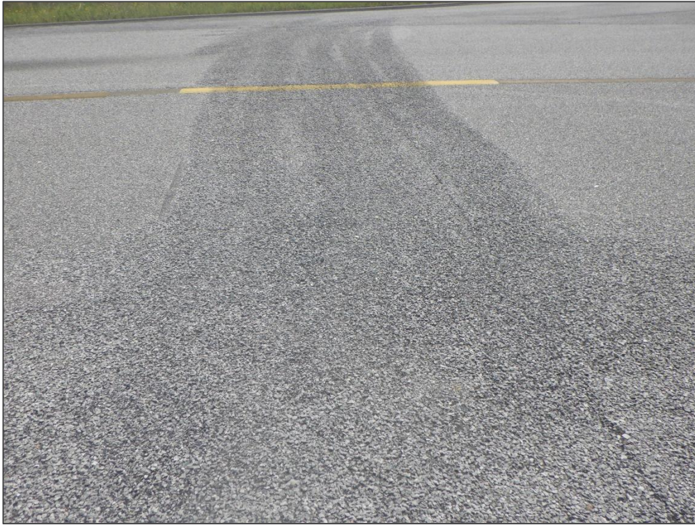
TW A, Section 150, Sample Unit 107 – Raveling
