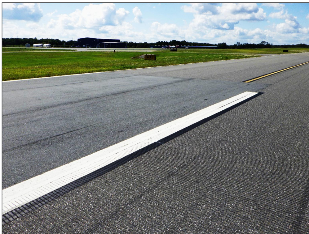
RW 1-19, Section 6105, Sample Unit 130 - Patching
