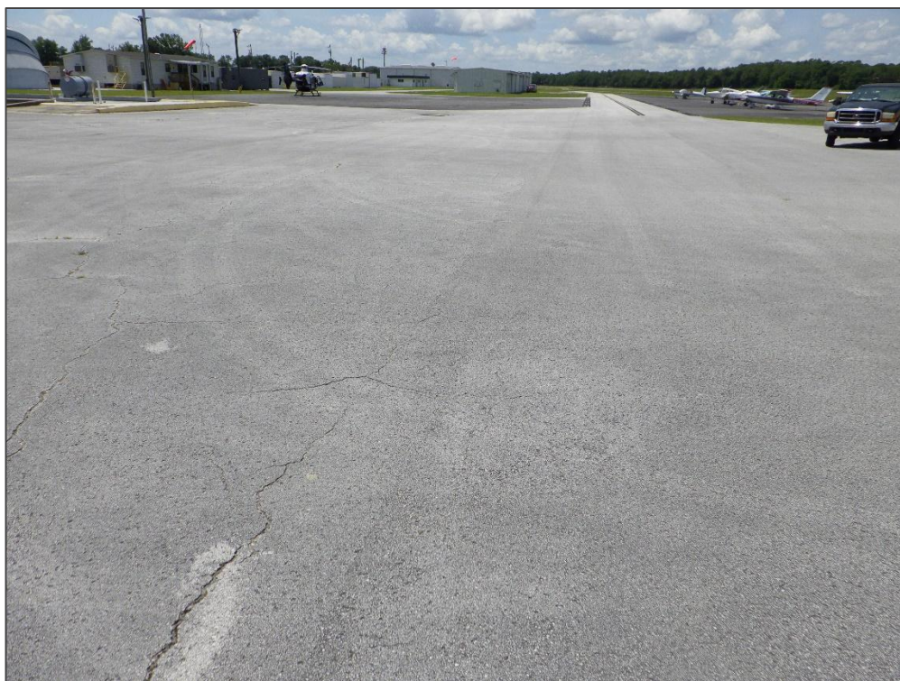
AP GA, Section 4005, Sample Unit 604 - Longitudinal & Transverse Cracking
