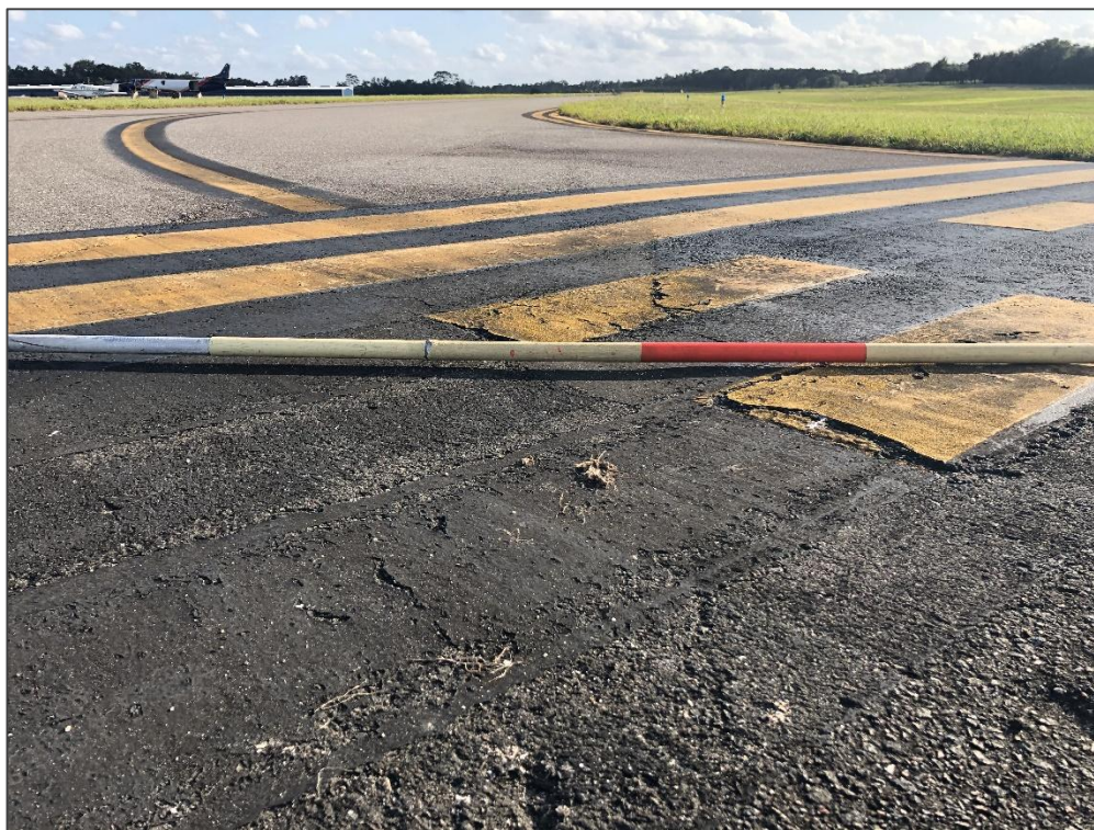
TW A1, Section 115, Sample Unit 201 - Depression
