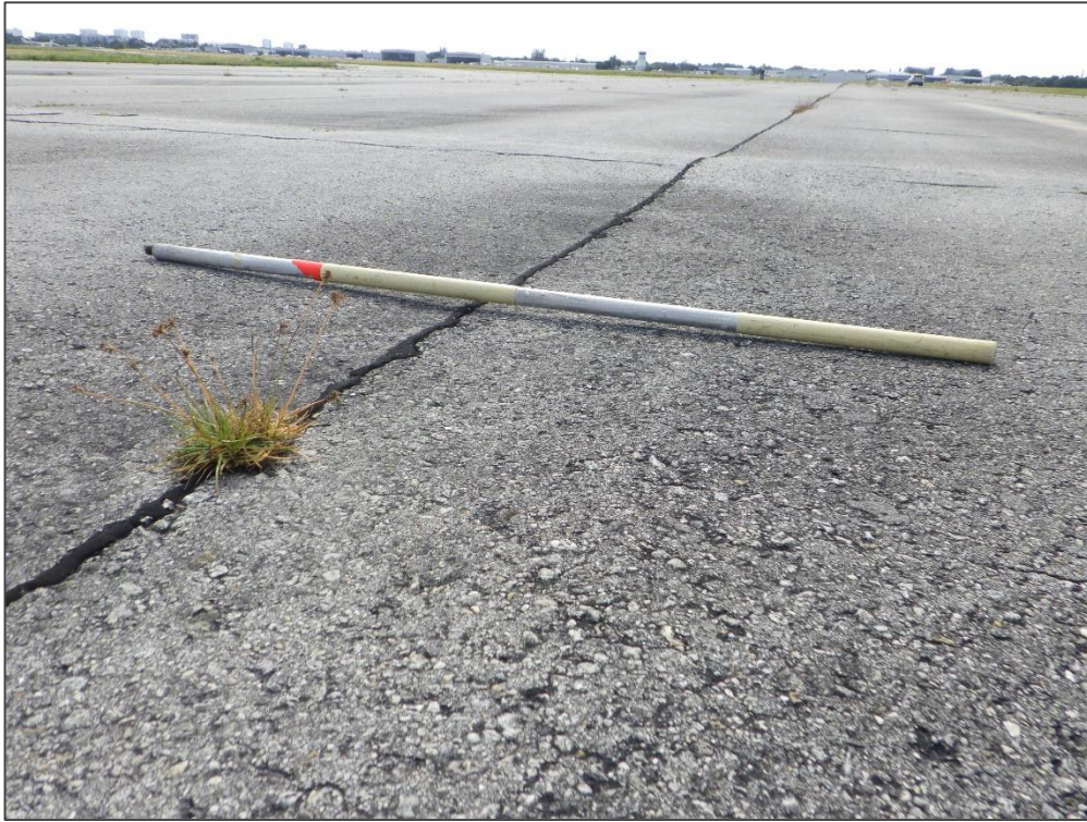
AP N, Section 4205, Sample Unit 109 - Depression and Longitudinal & Transverse Cracking
