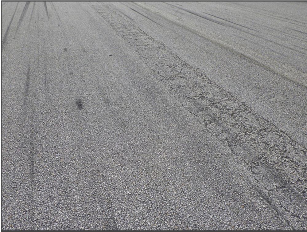
RW 10-28, Section 6105, Sample Unit 117 - Raveling
