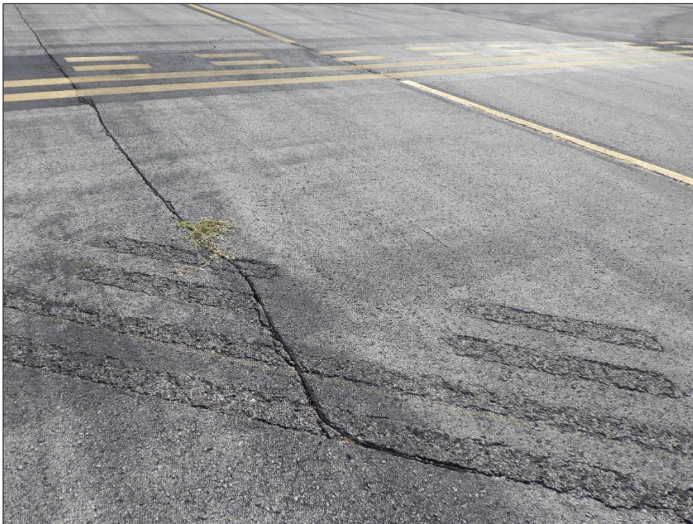
TW F, Section 610, Sample Unit 601 - Longitudinal & Transverse Cracking and Raveling
