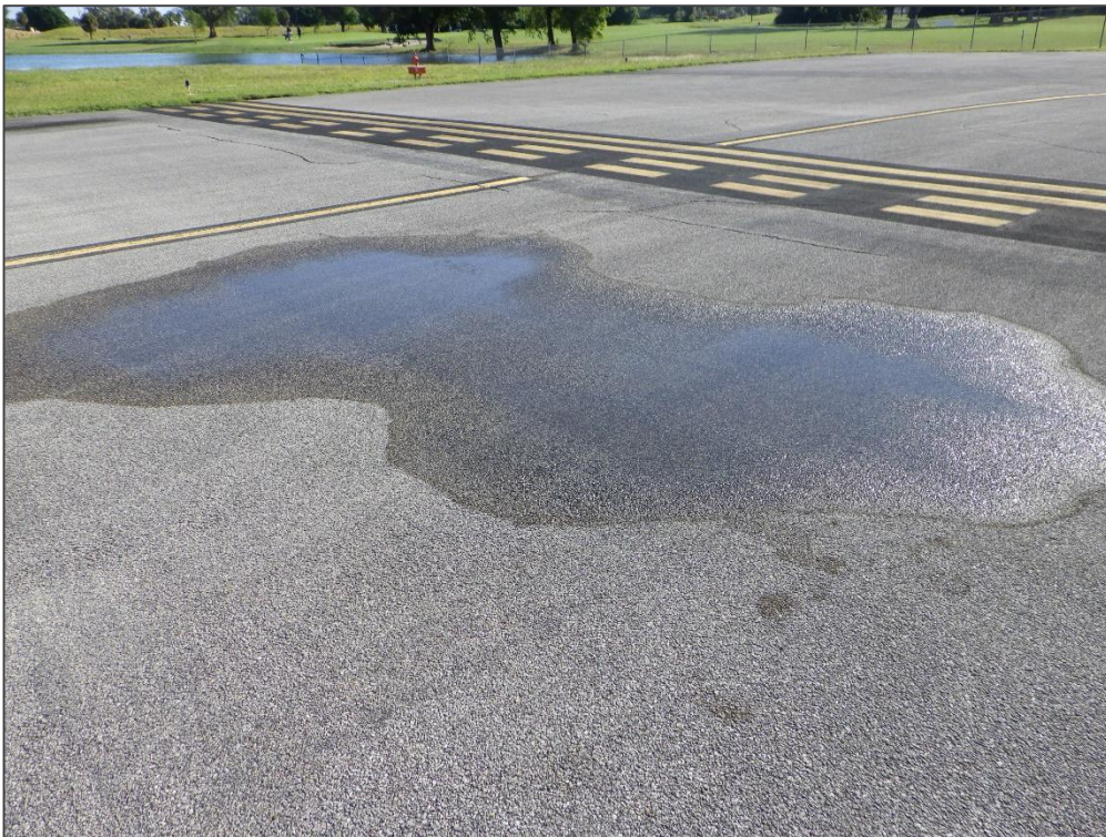
TW M, Section 1320, Sample Unit 198 - Depression
