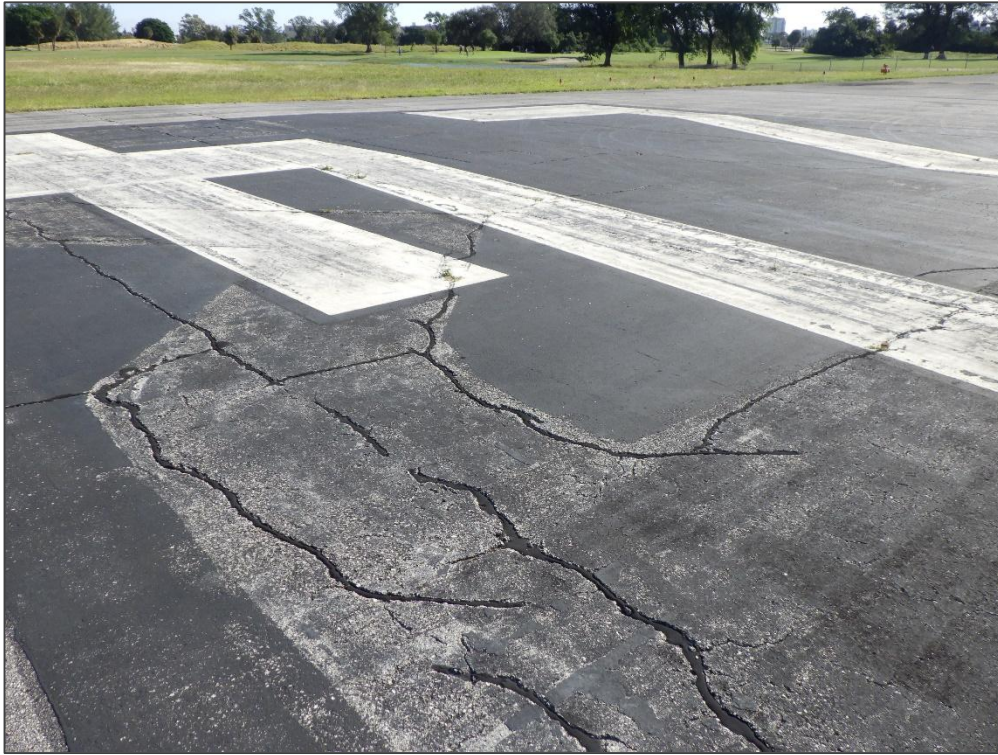
RW 6-24, Section 6205, Sample Unit 378 – Longitudinal and Transverse Cracking
