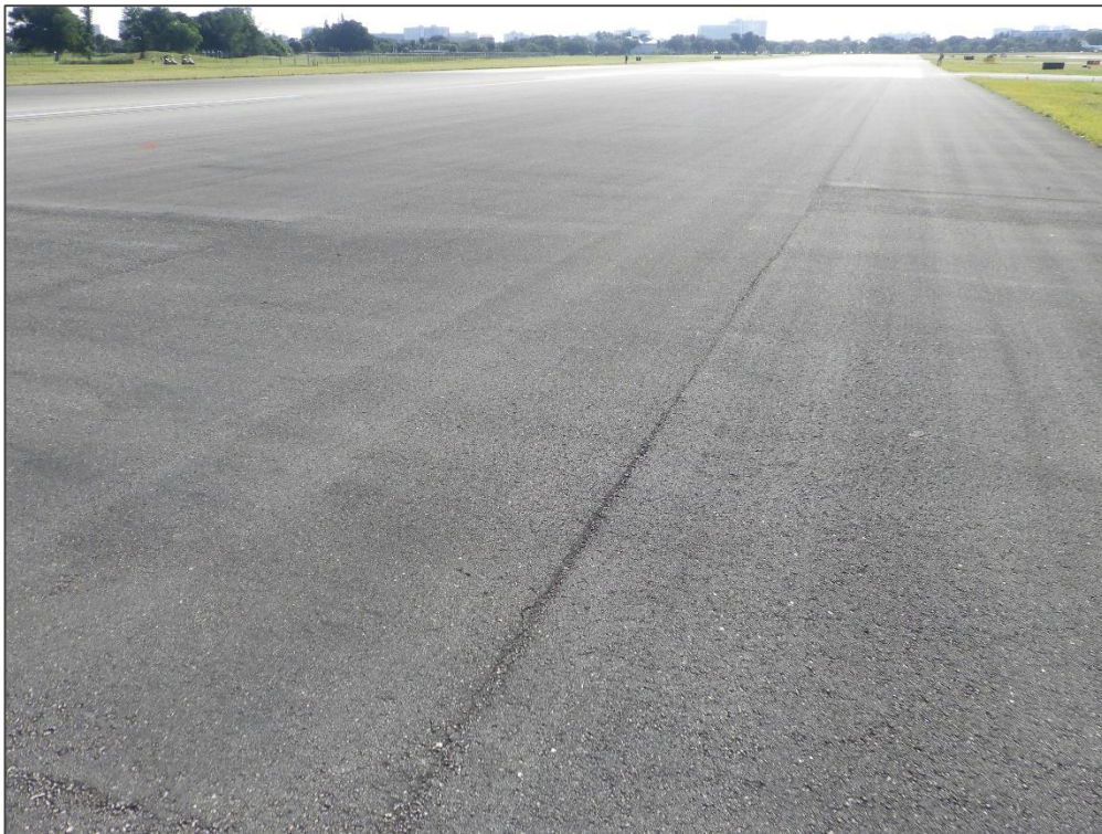
RW 15-33, Section 6310, Sample Unit 117 - Longitudinal & Transverse Cracking
