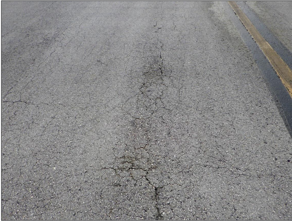
TW D, Section 420, Sample Unit 410 - Alligator Cracking
