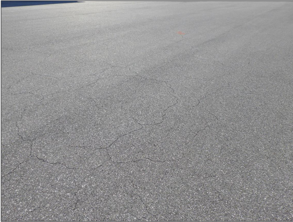
AP S, Section 4130, Sample Unit 305 - Block Cracking
