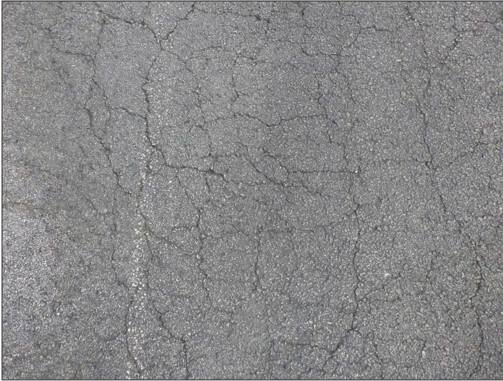
AP W, Section 4115, Sample Unit 503 - Alligator Cracking
