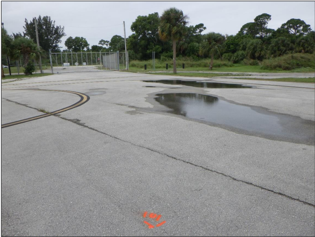
AP RU 16, Section 5105, Sample Unit 101 – Longitudinal & Transverse Cracking and Depression
