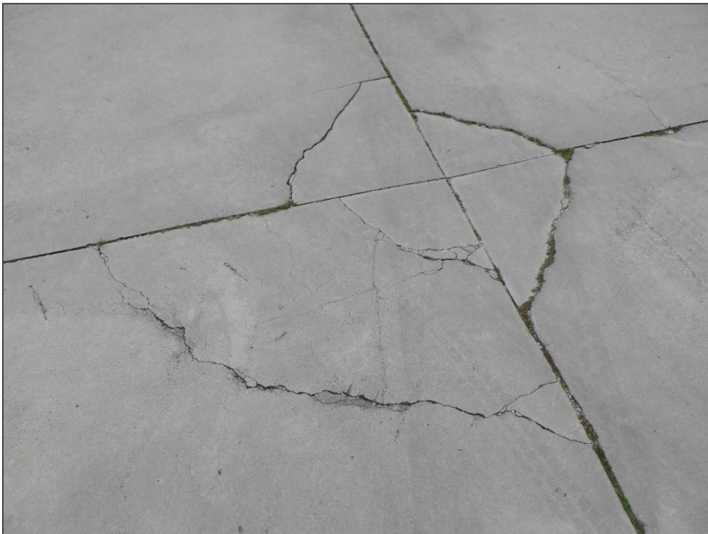
AP W, Section 4125, Sample Unit 710 - Corner Break
