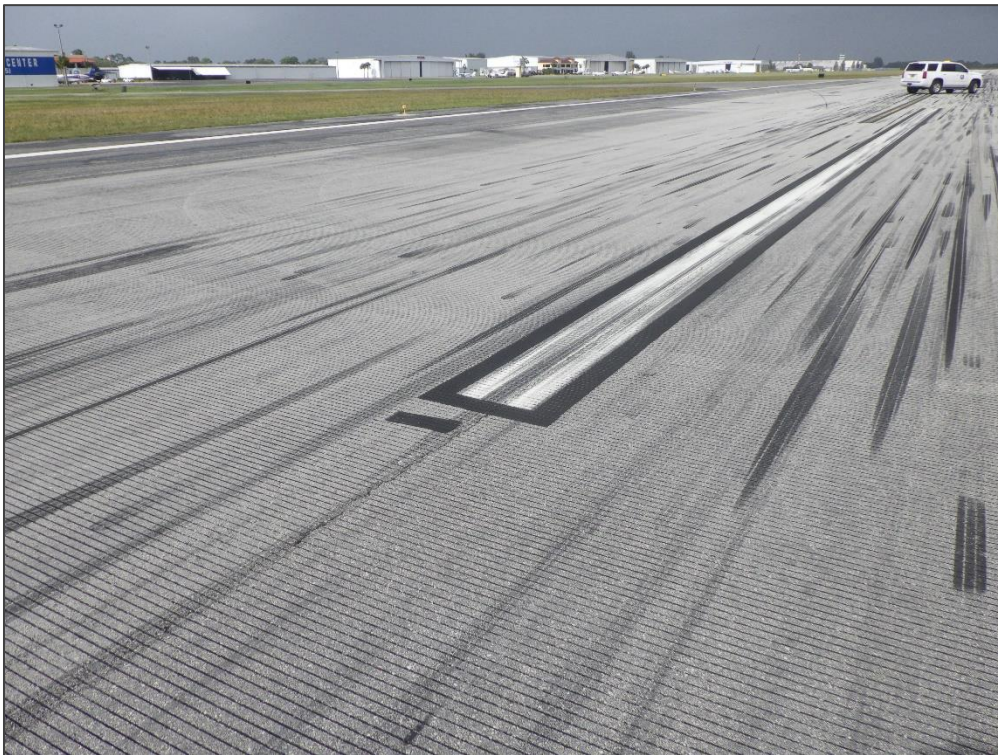
RW 12-30, Section 6105, Sample Unit 392 - Longitudinal & Transverse Cracking
