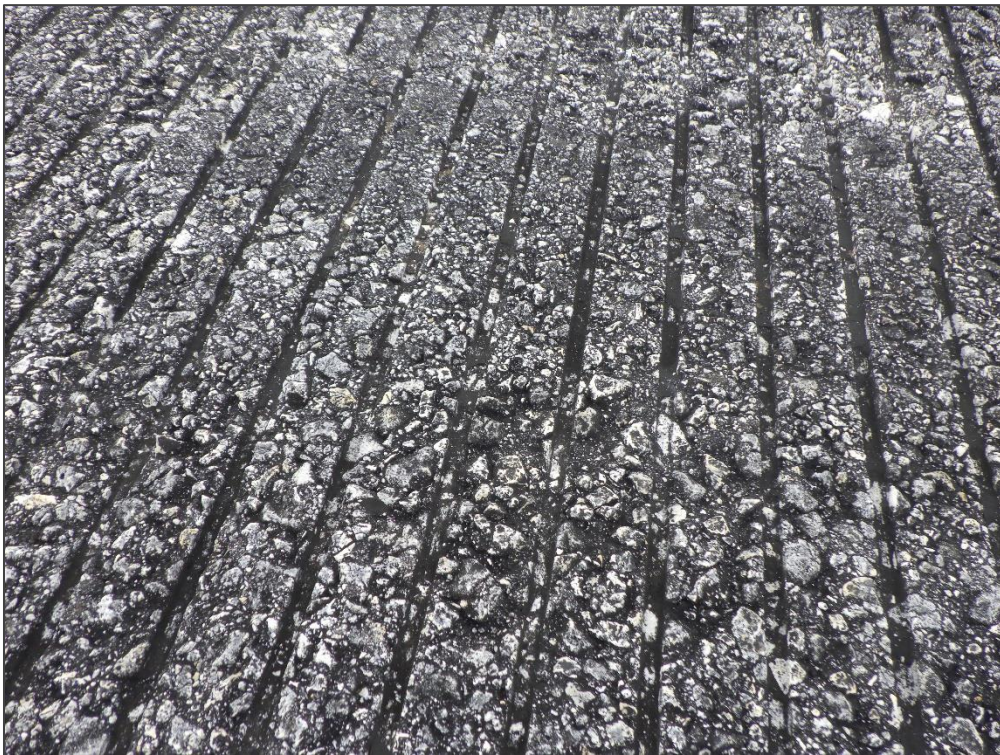
RW 16-34, Section 6305, Sample Unit 369 - Weathering
