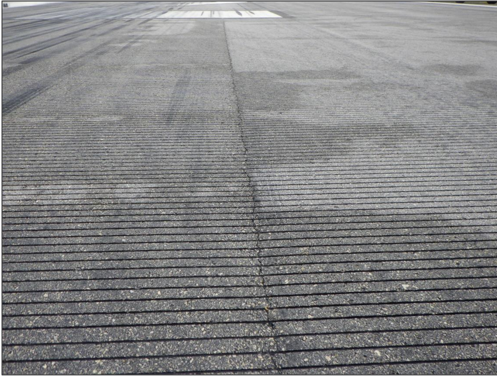
RW 7-25, Section 6205, Sample Unit 395 - Longitudinal & Transverse Cracking
