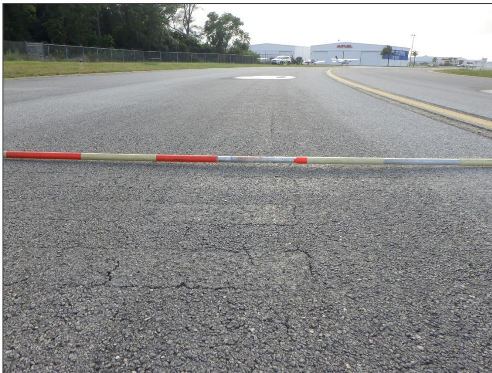
TW A, Section 110, Sample Unit 202 - Rutting
