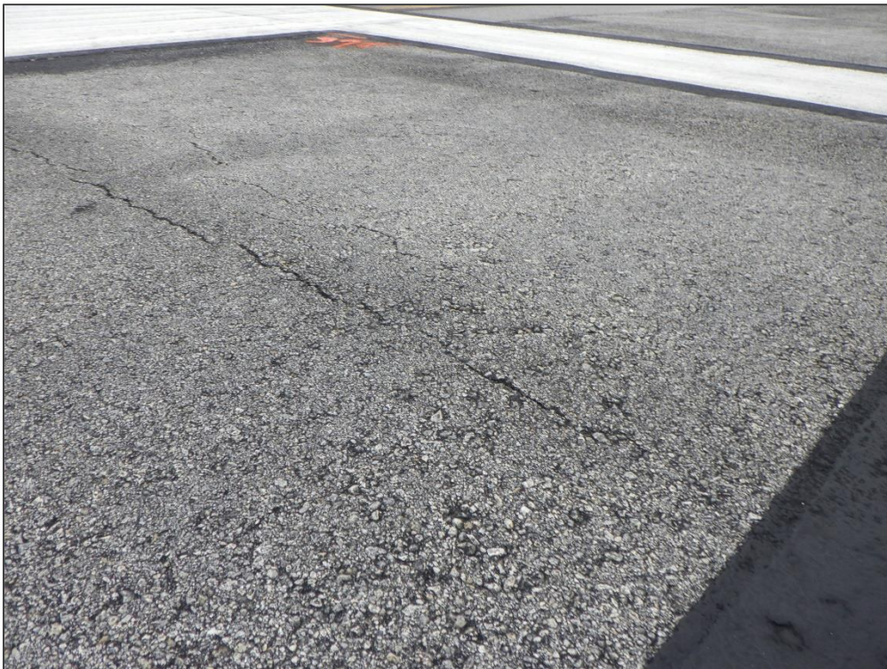
RW 7-25, Section 6205, Sample Unit 395 – Longitudinal and Transverse Cracking and Swelling
