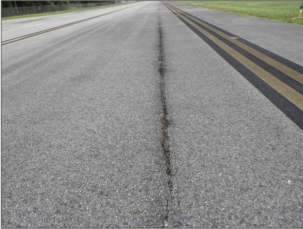
TW C, Section 305, Sample Unit 406 - Longitudinal & Transverse Cracking
