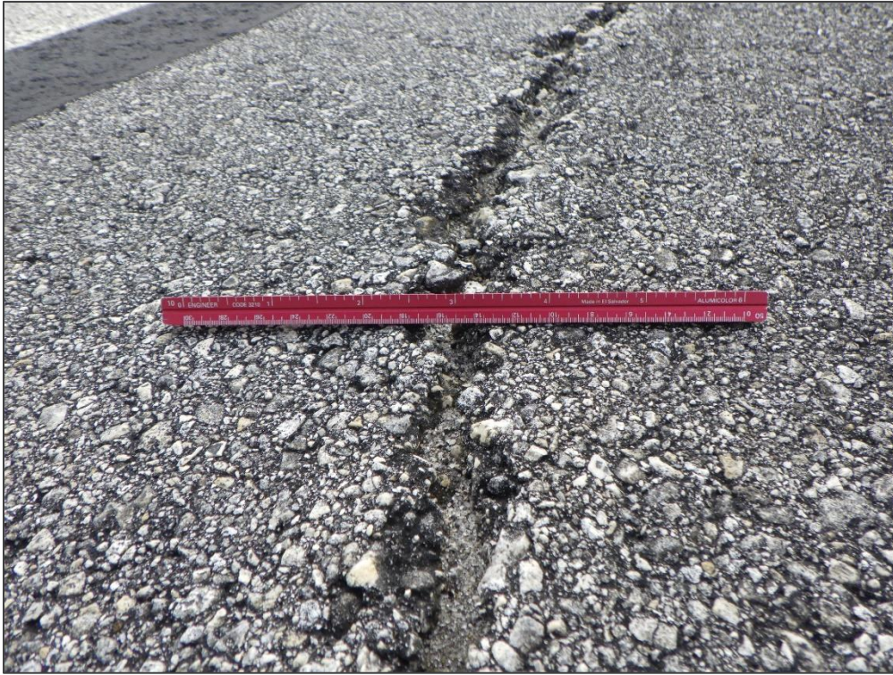
RW 7-25, Section 6205, Sample Unit 334 - Longitudinal & Transverse Cracking
