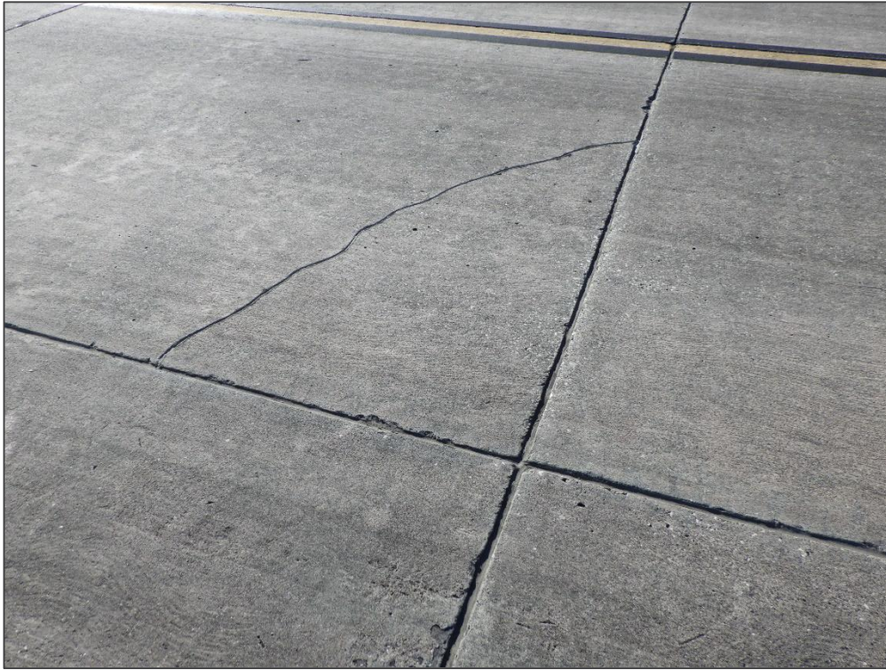
TW A, Section 110, Sample Unit 289 - Corner Break
