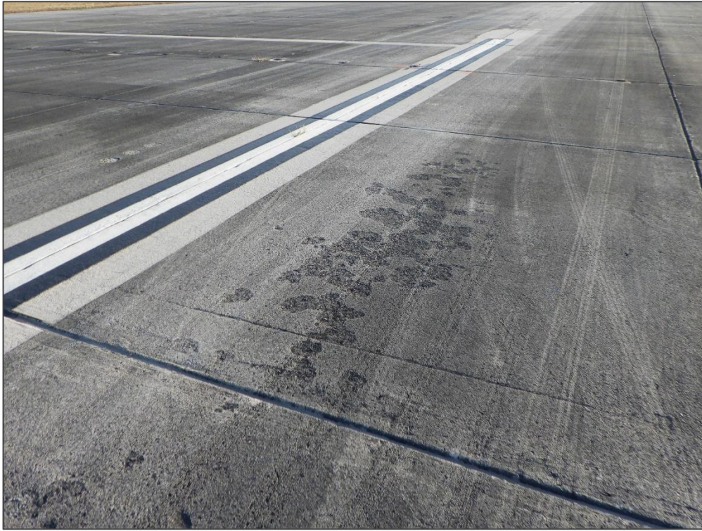
RW 9L-27R, Section 6405, Sample Unit 503 - Scaling
