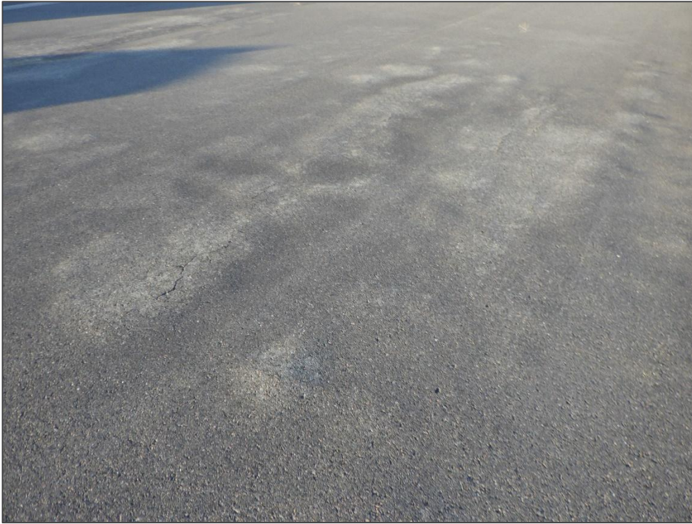
RW 9R-27L, Section 6320, Sample Unit 752 – Swelling
