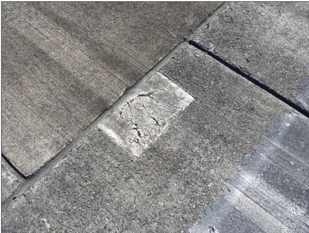
RW 18R-36L, Section 6110, Sample Unit 101 – Small Patch
