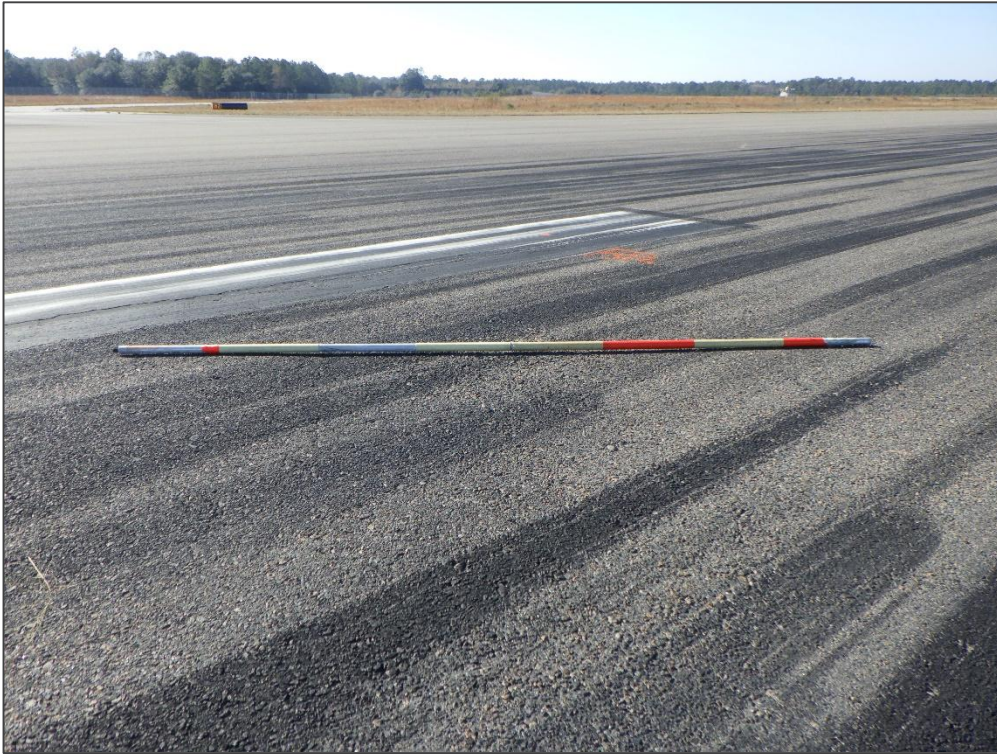
RW 9R-27L, Section 6315, Sample Unit 322 – Depression
