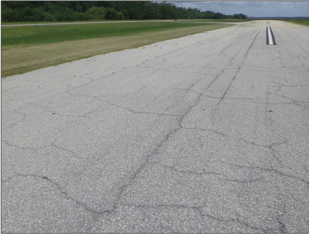
RW 15-33, Section 6110, Sample Unit 117 - Block Cracking
