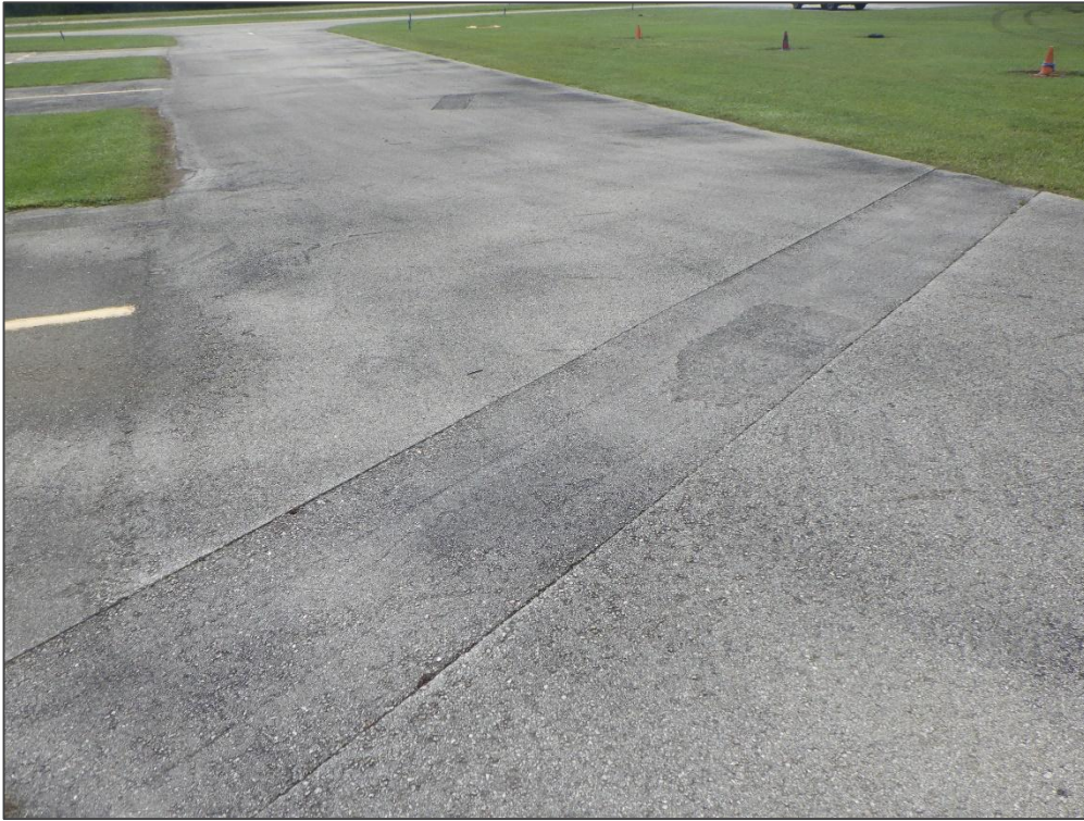
AP, Section 4110, Sample Unit 100 - Patching
