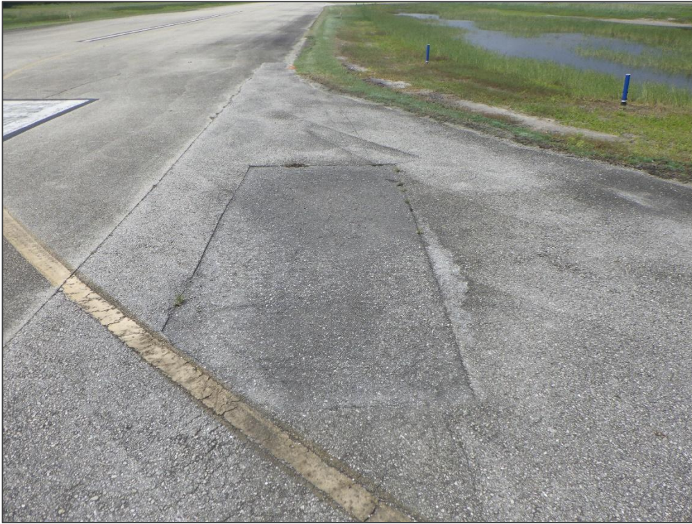
TW A, Section 125, Sample Unit 106 - Patching
