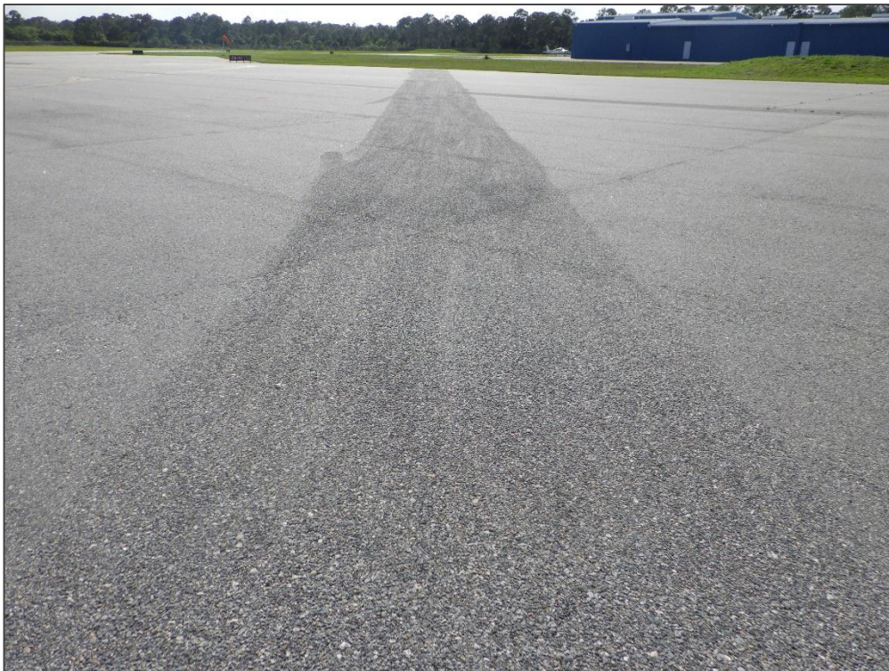
AP, Section 4105, Sample Unit 300 - Raveling
