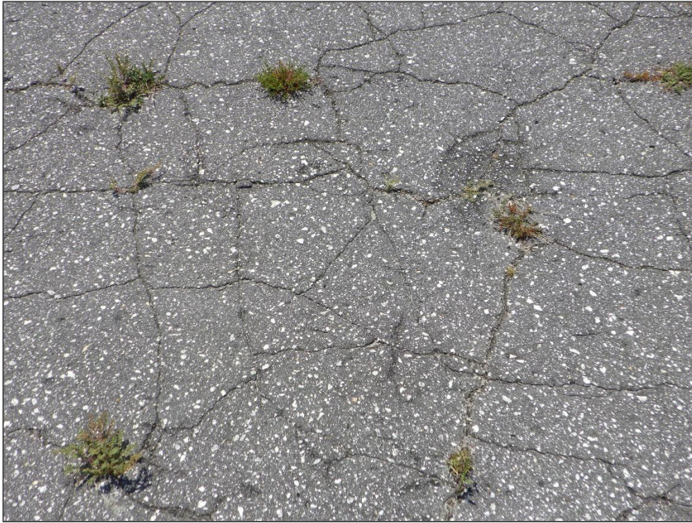
AP, Section 4130, Sample Unit 104 - Alligator Cracking
