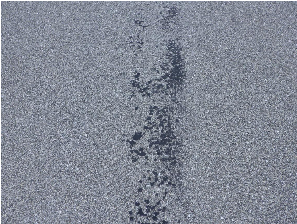
TW B, Section 260, Sample Unit 101 – Bleeding
