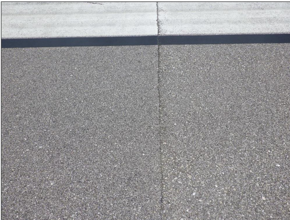
RW 14-32, Section 6225, Sample Unit 359 – Longitudinal & Transverse Cracking and Weathering
