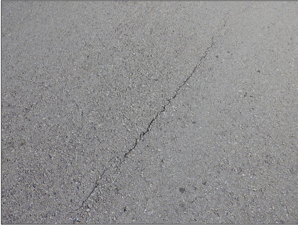
TW A, Section 115, Sample Unit 148 – Longitudinal & Transverse Cracking
