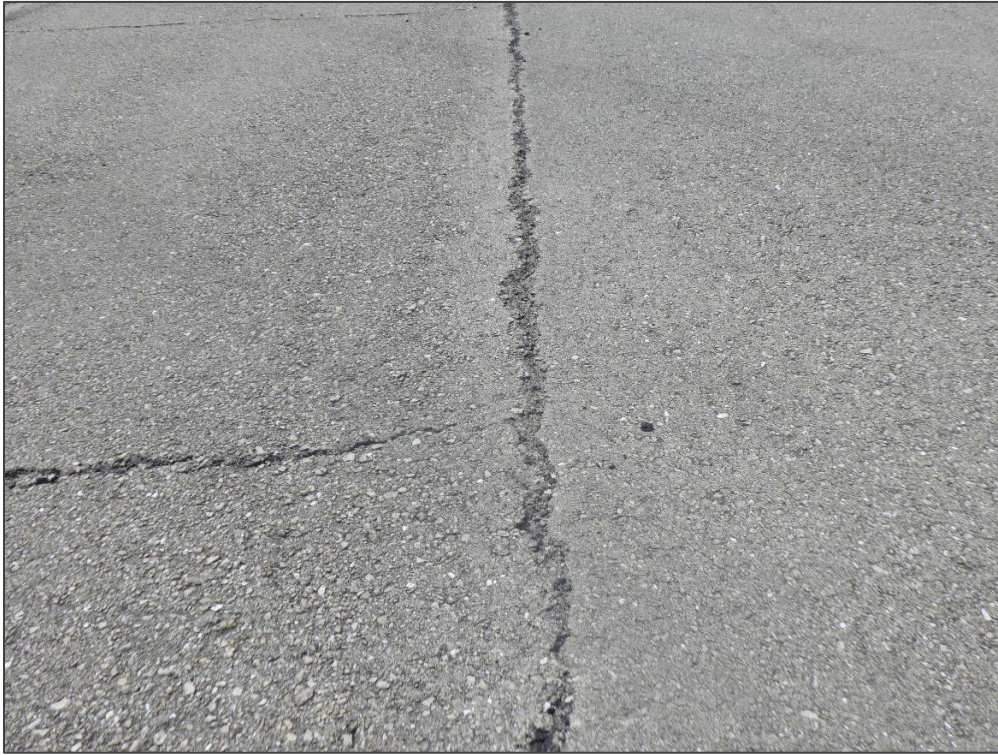
TW C, Section 330, Sample Unit 105 – Longitudinal & Transverse Cracking and Weathering
