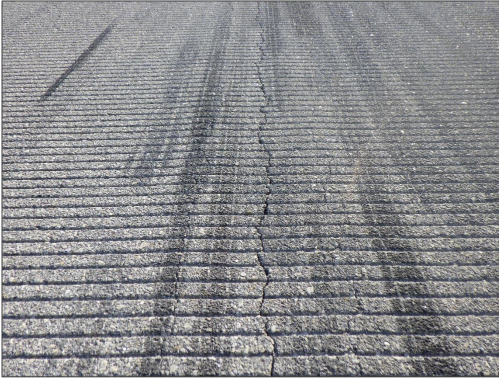
RW 5-23, Section 6105, Sample Unit 335 – Longitudinal & Transverse Cracking
