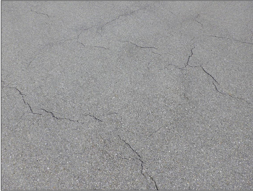
AP GA, Section 4255, Sample Unit 209 – Block Cracking
