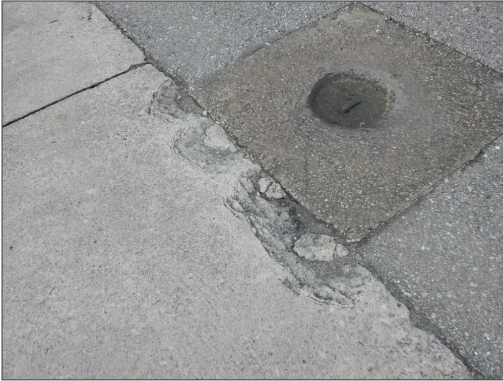
AP GA, Section 4287, Sample Unit 100 - Joint Spall
