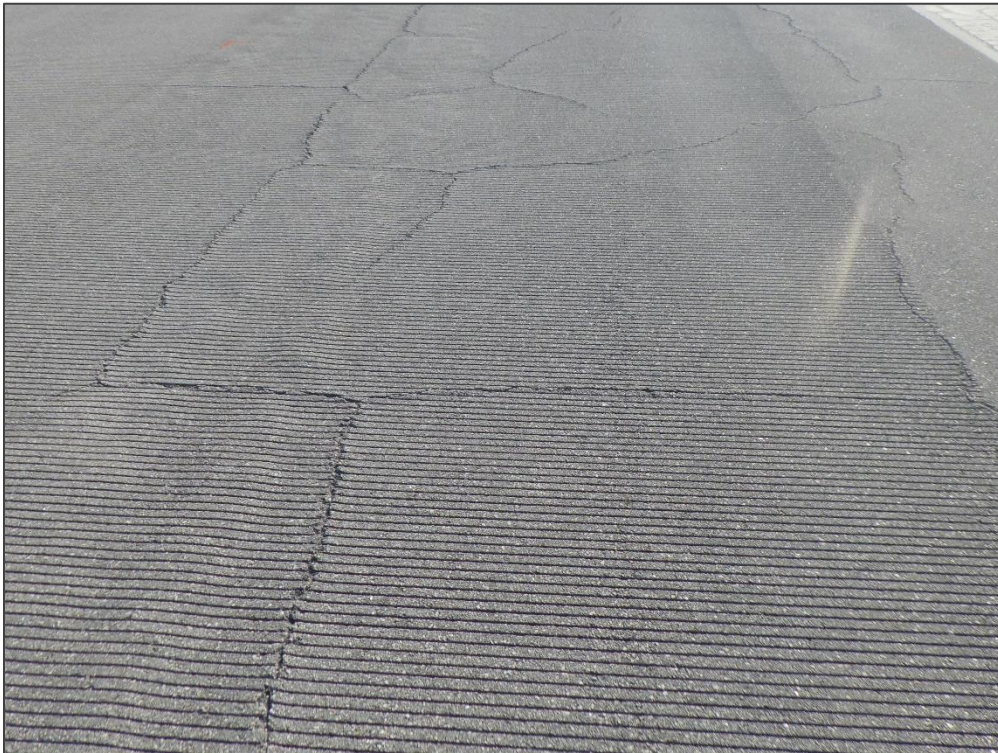
RW 5-23, Section 6110, Sample Unit 544 – Block Cracking
