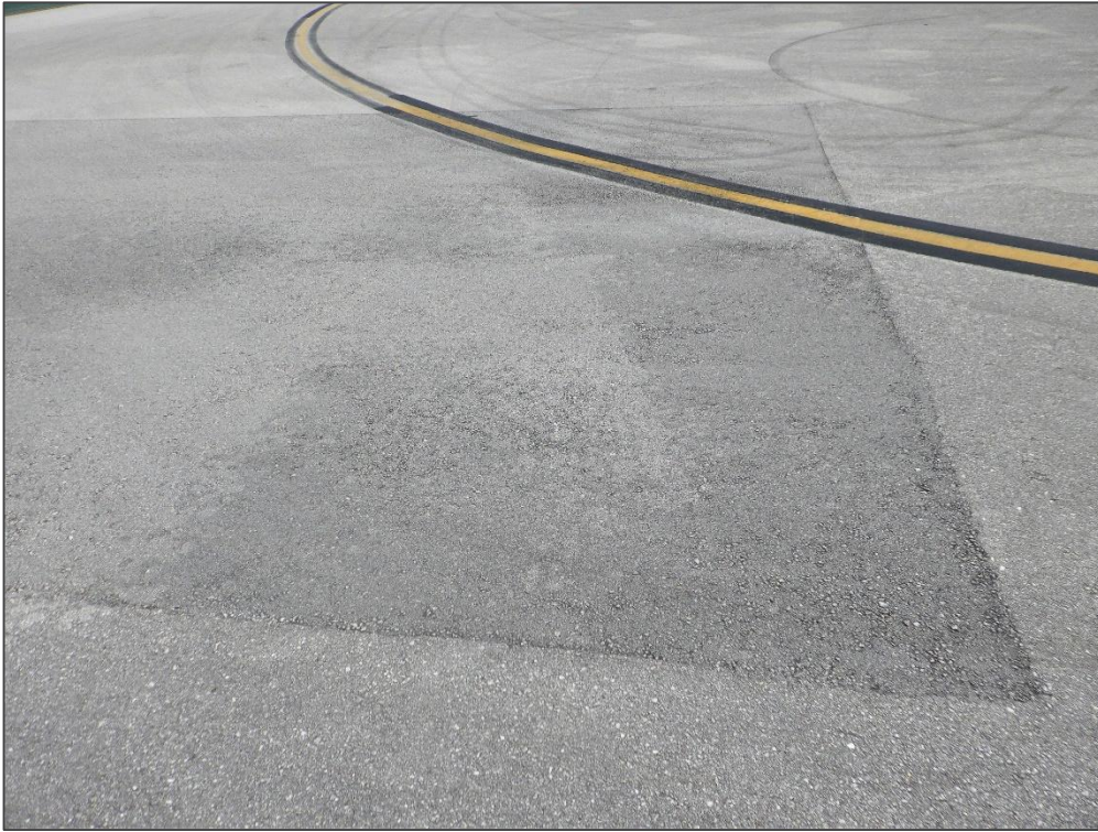
AP RU 5, Section 5115, Sample Unit 201 – Patching
