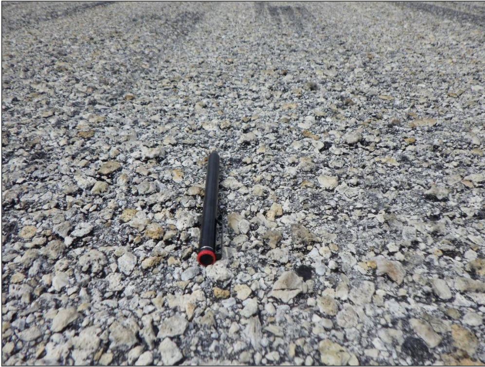
RW 5-23, Section 6105, Sample Unit 304 –Raveling
