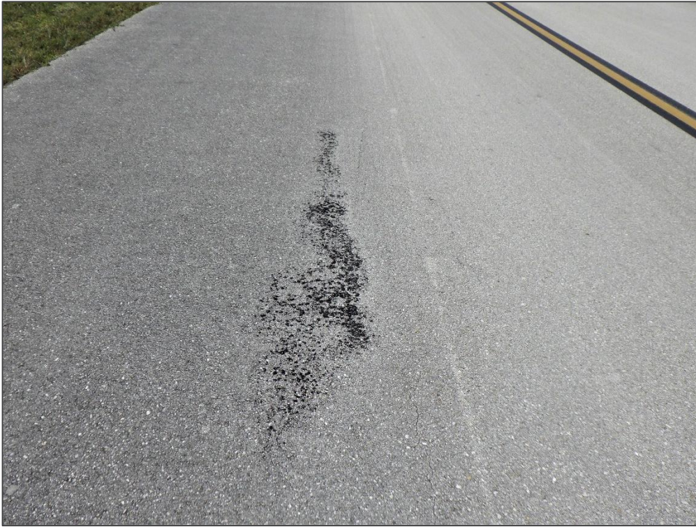
TW P, Section 105, Sample Unit 105 – Bleeding
