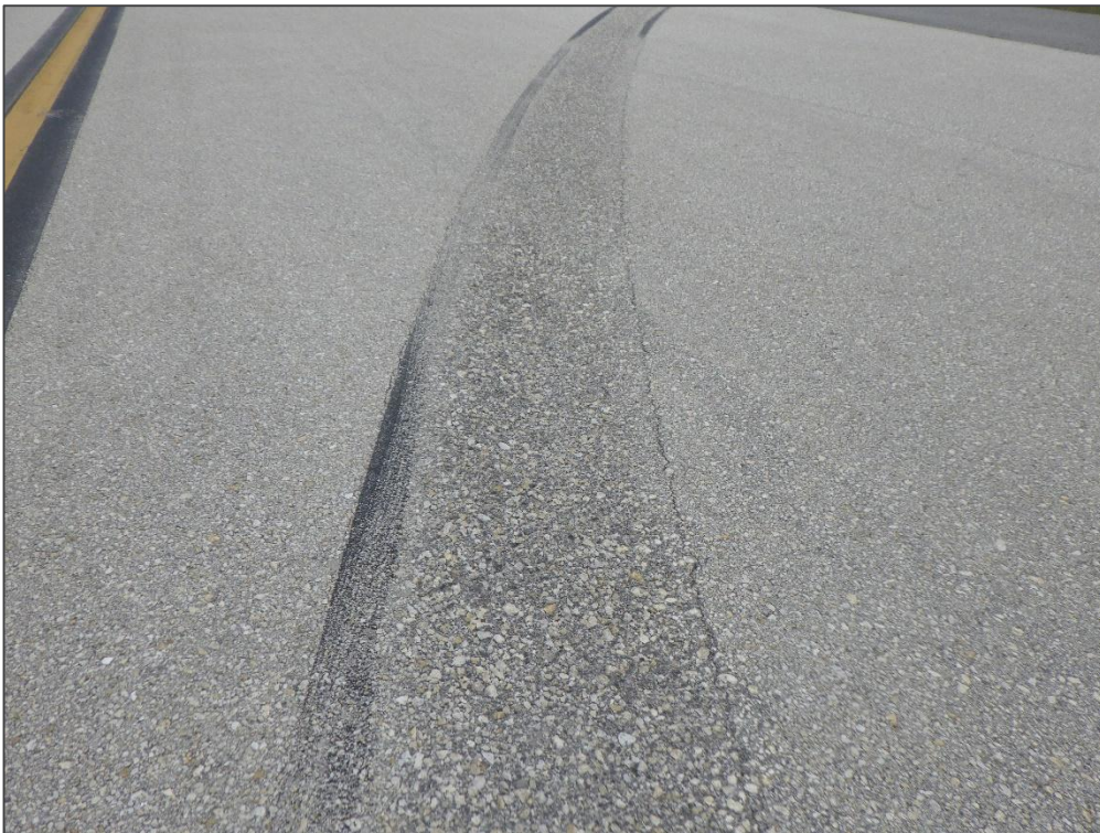
TW P, Section 105, Sample Unit 145 – Raveling
