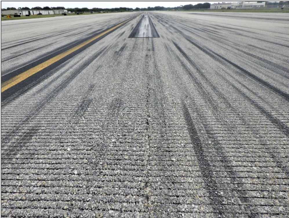
RW 5-23, Section 6105, Sample Unit 382 – Longitudinal & Transverse Cracking and Raveling
