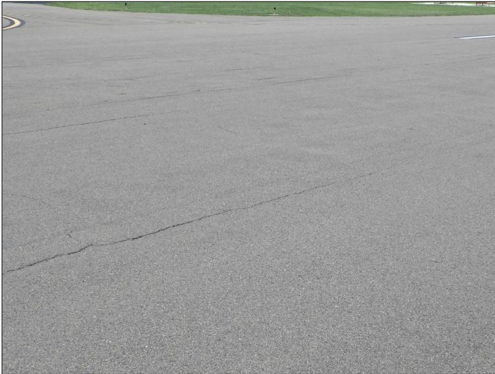
RW 16-34, Section 6110, Sample Unit 130 – Longitudinal & Transverse Cracking and Swelling
