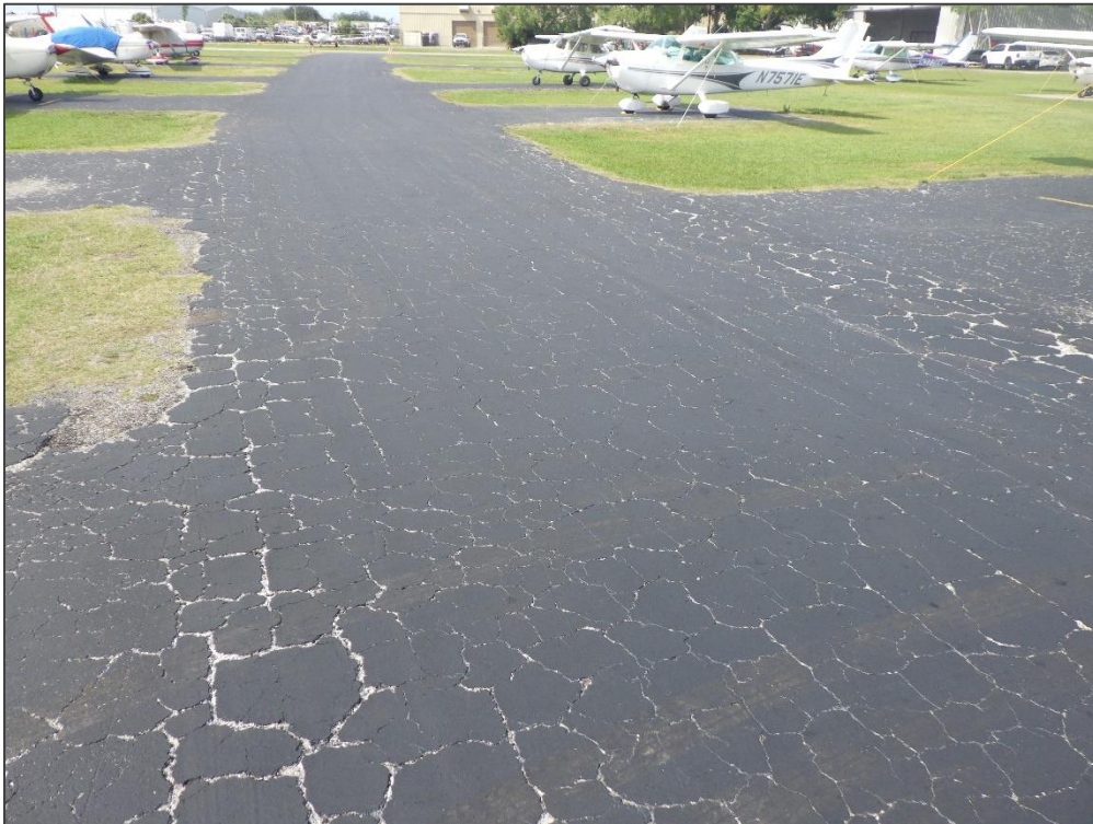
TL CENTER, Section 3410, Sample Unit 301 – Raveling
