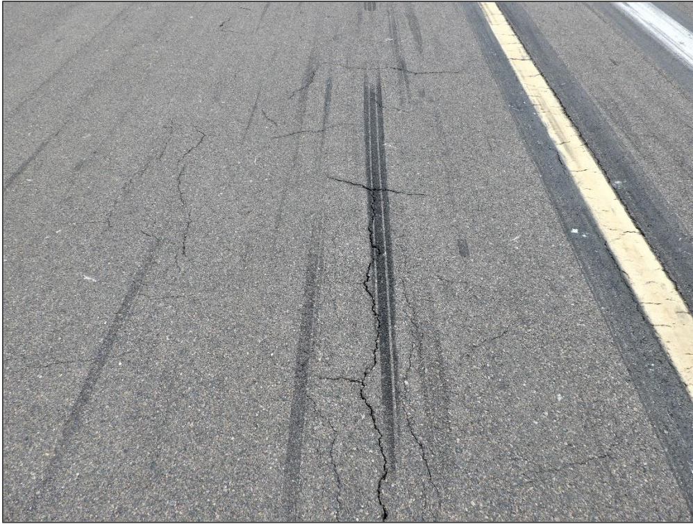
RW 16-34, Section 6110, Sample Unit 155 – Longitudinal & Transverse Cracking
