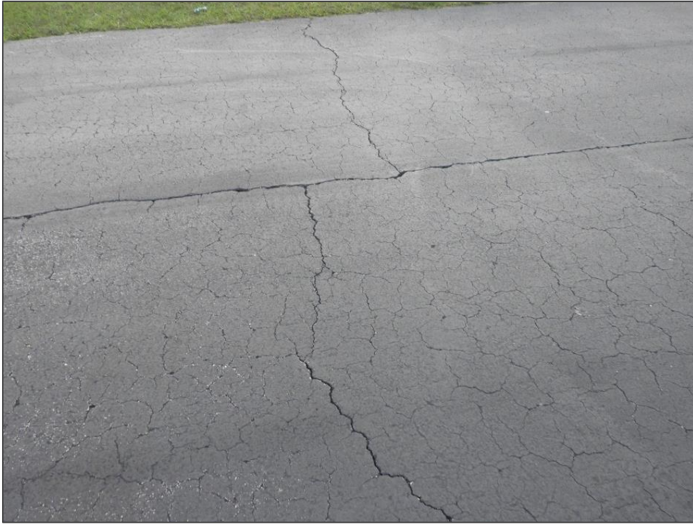
TL T-HANG, Section 3605, Sample Unit 105 – Longitudinal & Transverse Cracking and Raveling
