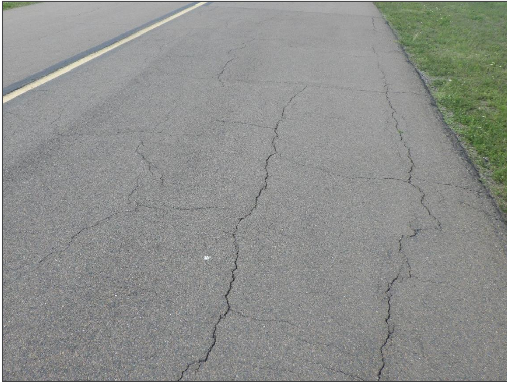
TW A, Section 135, Sample Unit 128 – Block Cracking
