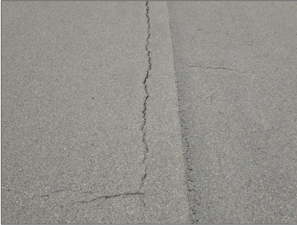
RW 16-34, Section 6110, Sample Unit 110 – Longitudinal & Transverse Cracking
