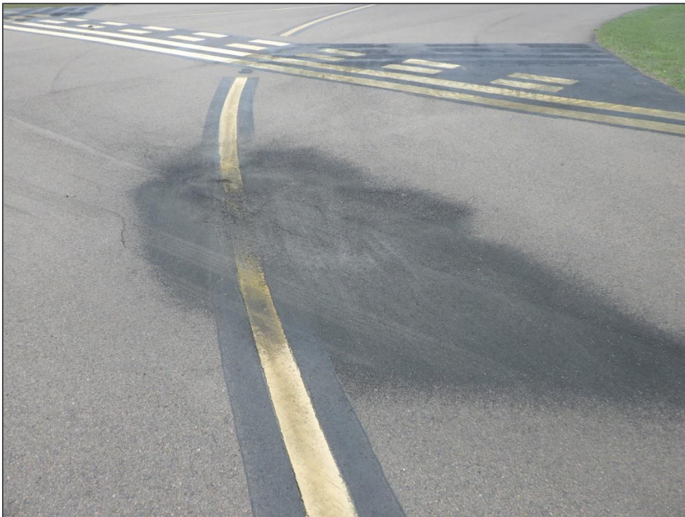
TW A, Section 105, Sample Unit 102 – Depression
