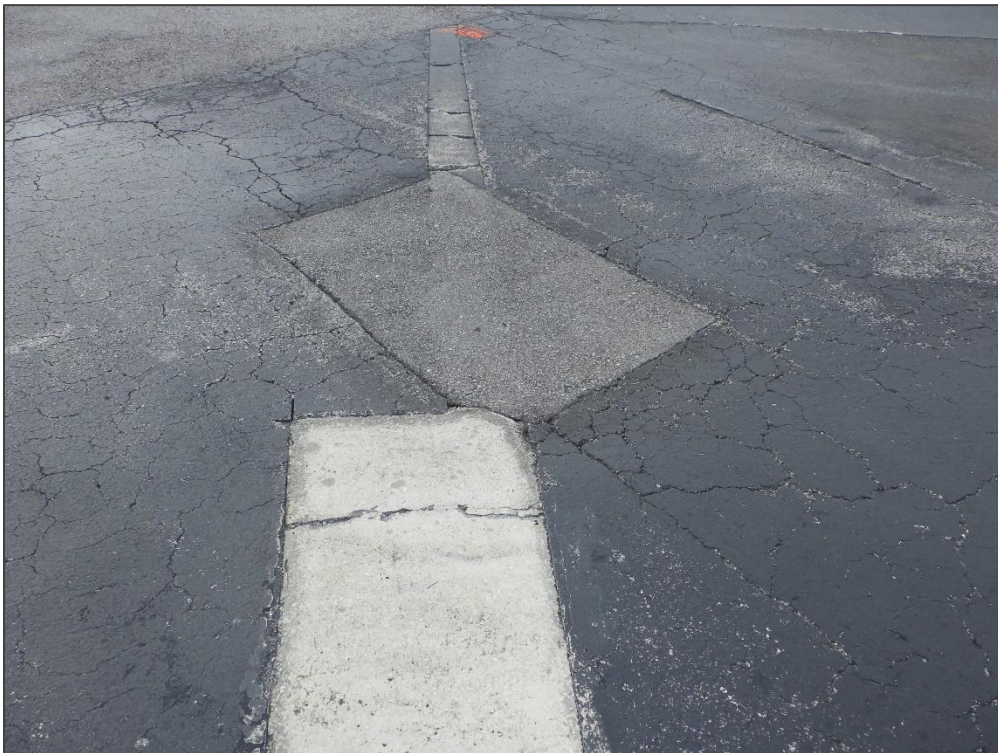
AP T-HANG, Section 4305, Sample Unit 650 – Patching and Raveling
