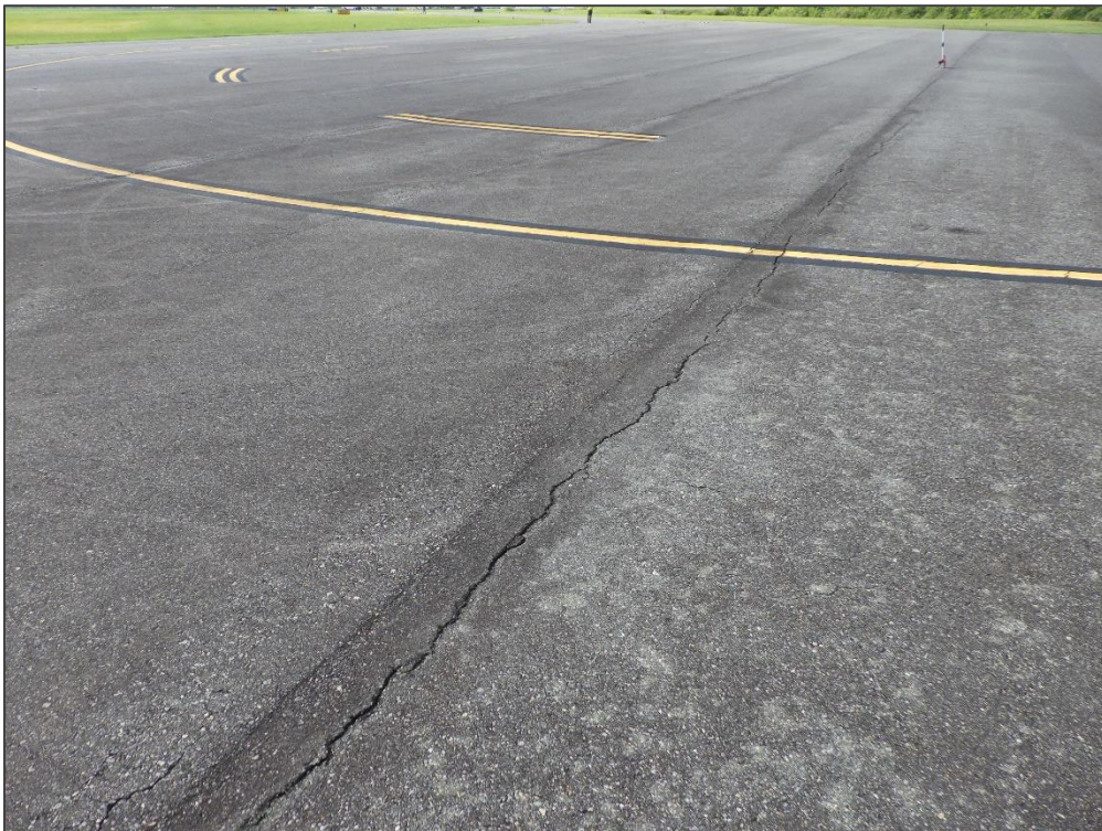
AP RU 14, Section 5310, Sample Unit 102 – Longitudinal & Transverse Cracking and Swelling
