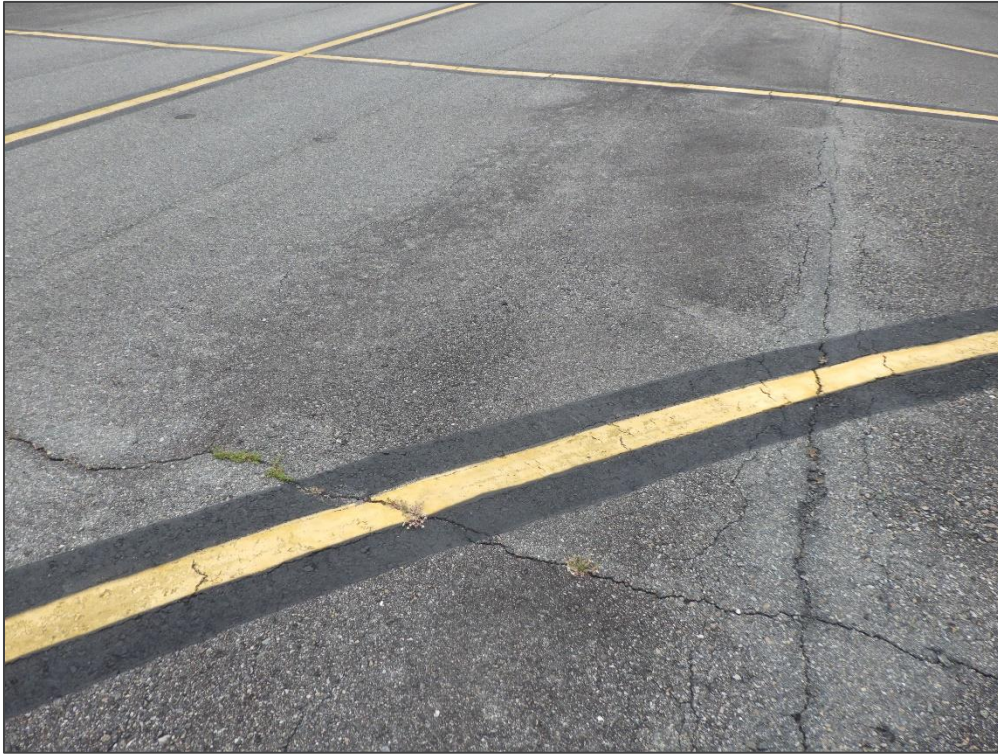
TW B, Section 225, Sample Unit 120 – Longitudinal & Transverse Cracking and Swelling
