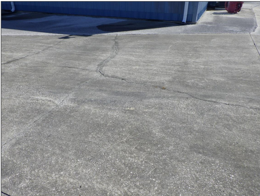
AP SW, Section 4405, Sample Unit 101 – Shattered Slab
