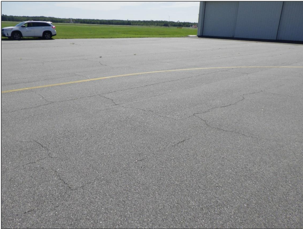
AP MID, Section 4210, Sample Unit 209 – Block Cracking
