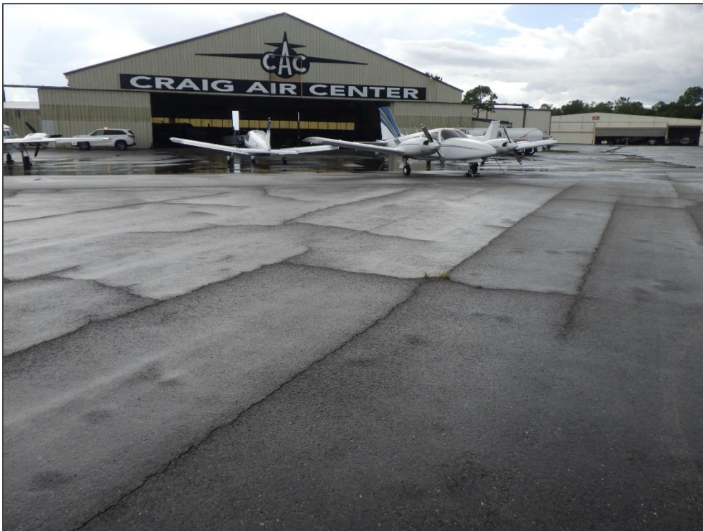
AP NW, Section 4305, Sample Unit 551 – Longitudinal & Transverse Cracking
