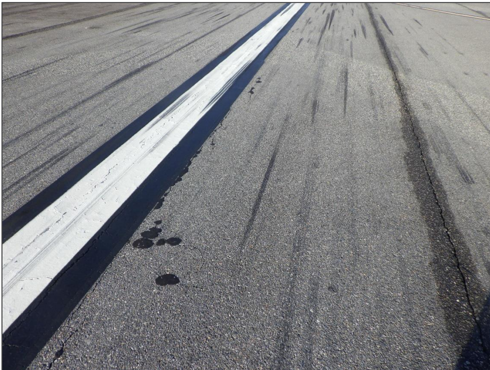
RW 5-23, Section 6105, Sample Unit 168 – Bleeding and Longitudinal & Transverse Cracking
