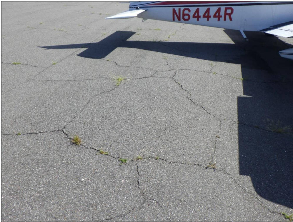
AP S, Section 4105, Sample Unit 203 – Block Cracking
