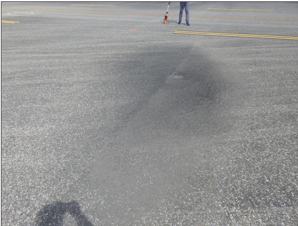
AP FAA, Section 4505, Sample Unit 603 – Depression
