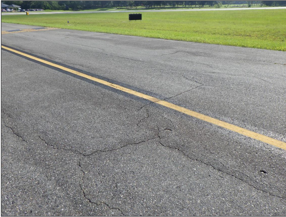
TW A, Section 105, Sample Unit 158 – Longitudinal & Transverse Cracking and Swelling
