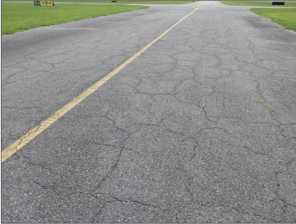
TW B4, Section 245, Sample Unit 407 – Block Cracking
