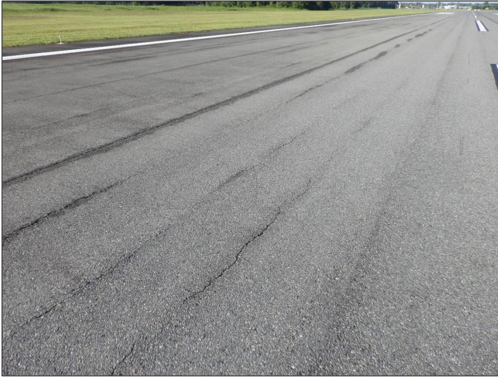
RW 5-23, Section 6105, Sample Unit 135 – Longitudinal & Transverse Cracking
