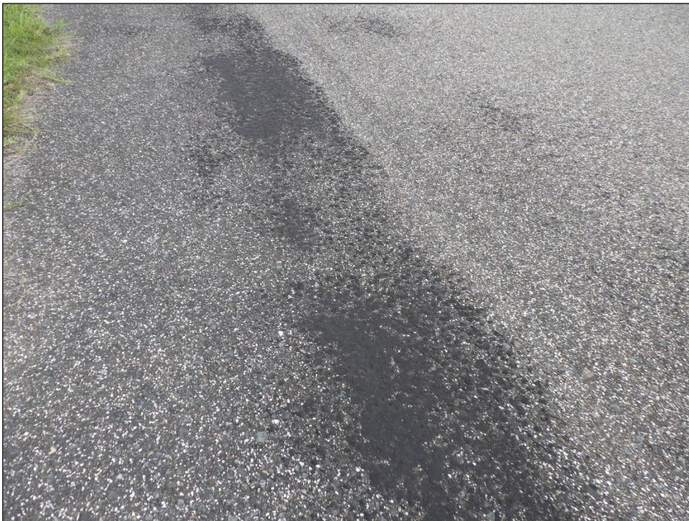
TW A, Section 120, Sample Unit 216 – Bleeding
