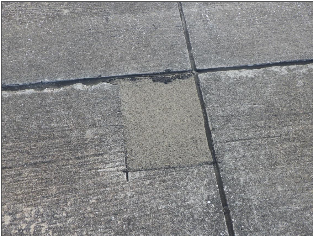
AP TERM, Section 4105, Sample Unit 707 – Small Patch
