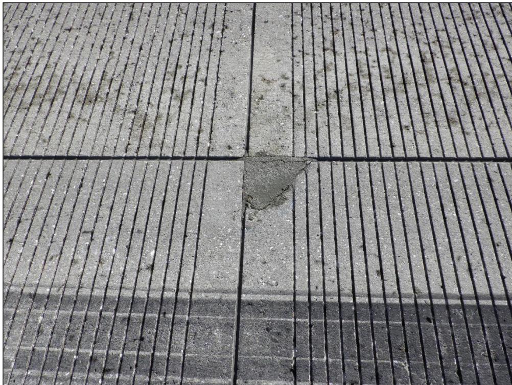
RW 16-34, Section 6105, Sample Unit 433 – Small Patch
