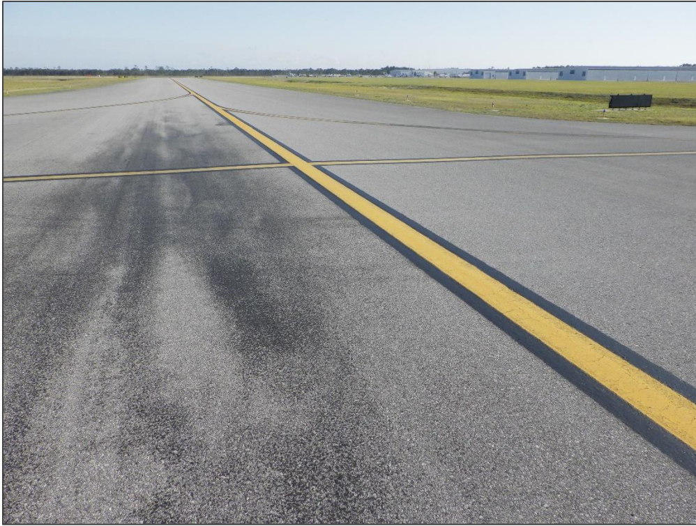
TW D, Section 405, Sample Unit 266 – Bleeding
