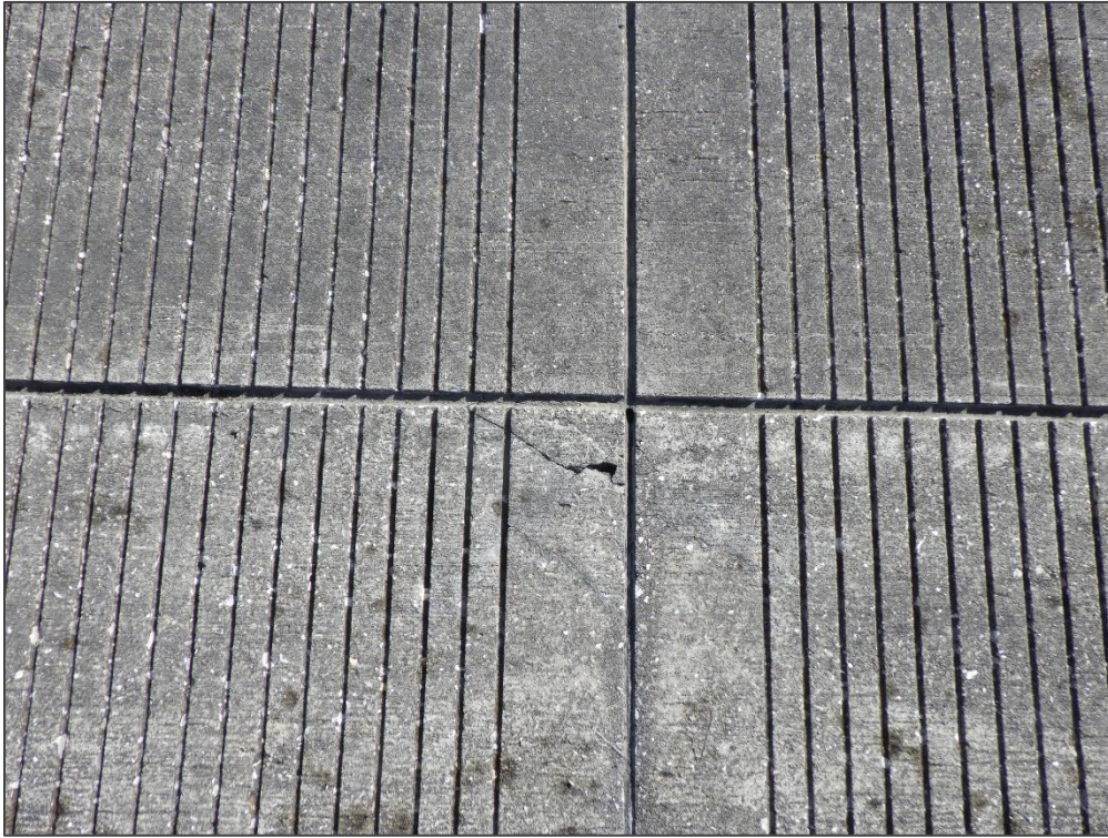
RW 16-34, Section 6110, Sample Unit 632 – Corner Spall
