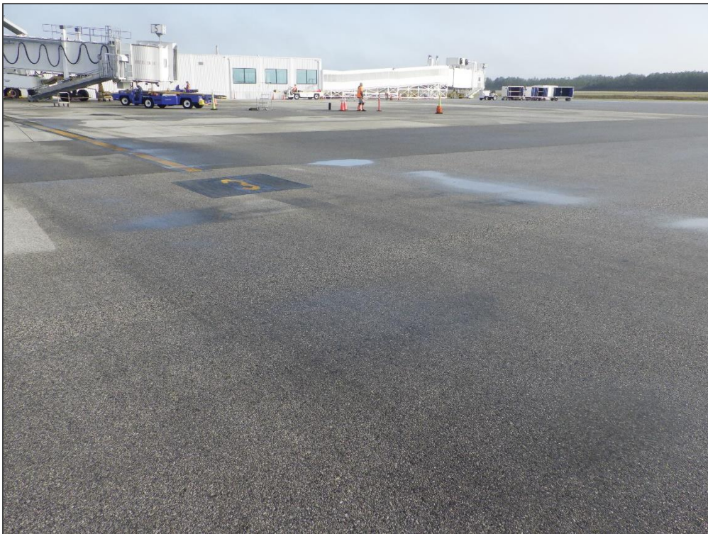
AP TERM, Section 4110, Sample Unit 357 – Rutting
