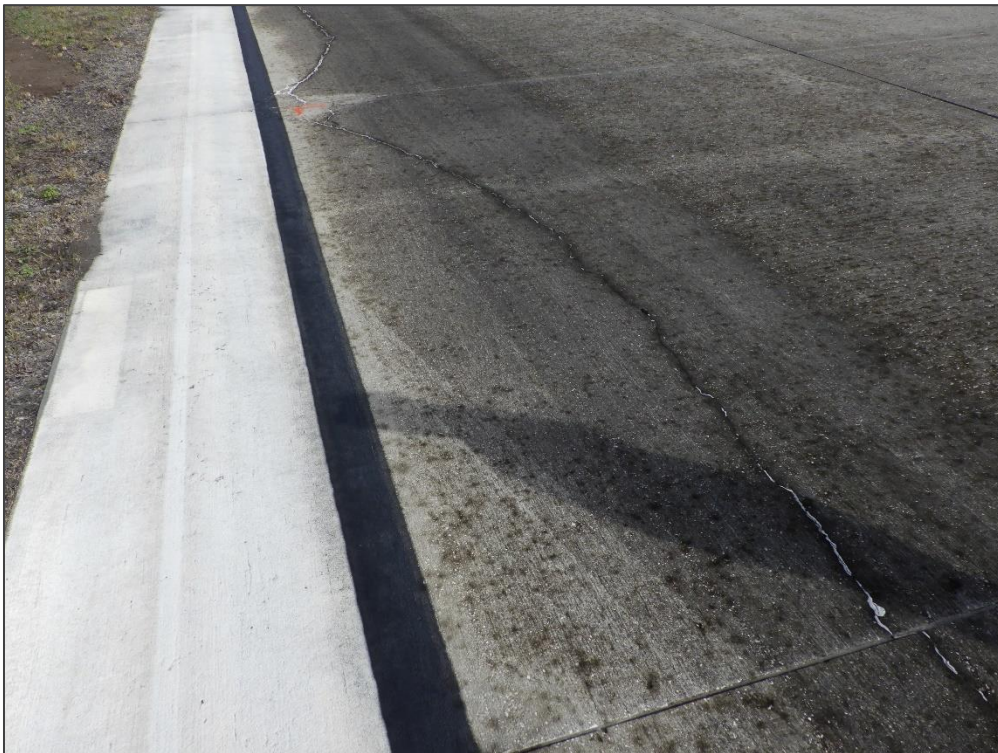
RW 16-34, Section 6110, Sample Unit 248 – Linear Cracking
