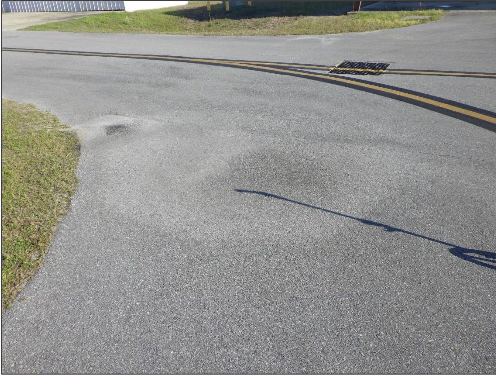
AP T-HANG, Section 4310, Section 450 – Depression
