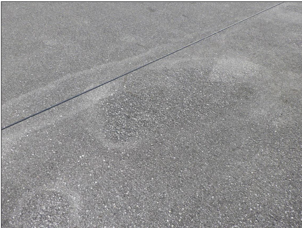
AP GA, Section 4405, Sample Unit 153 – Oil Spillage
