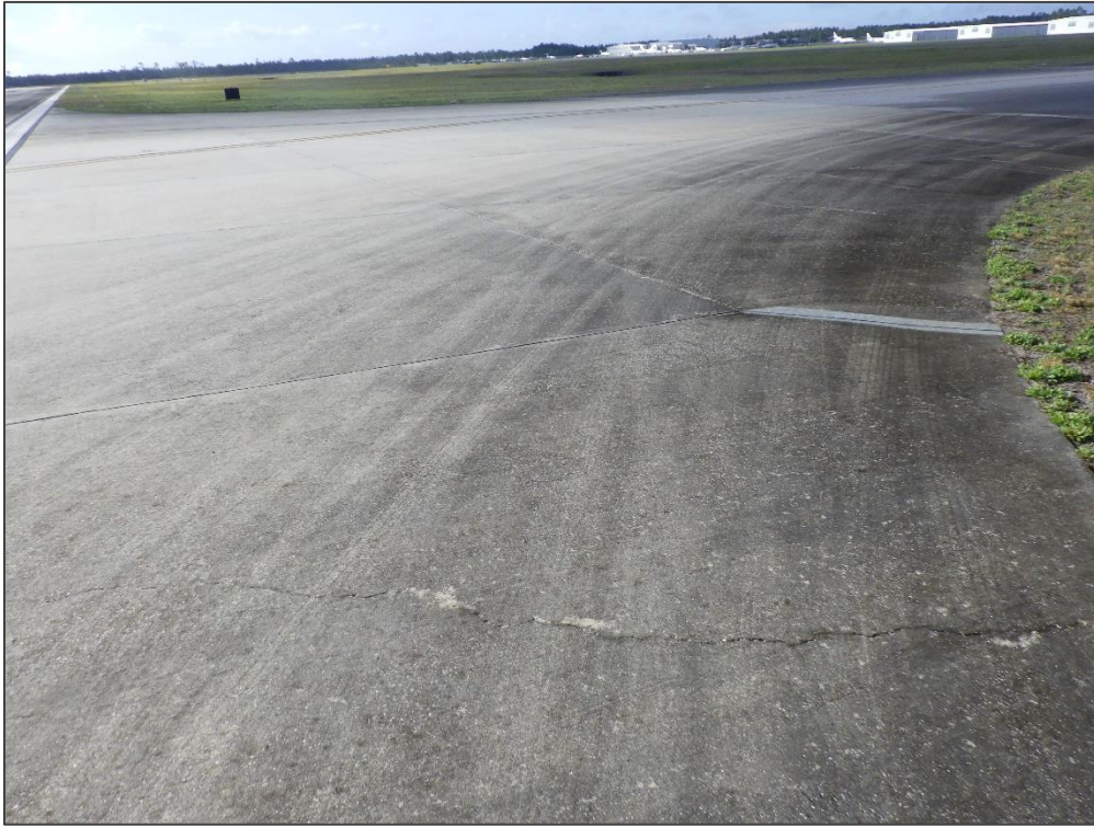
TW M, Section 1305, Sample Unit 500 – Linear Cracking and Small Patch
