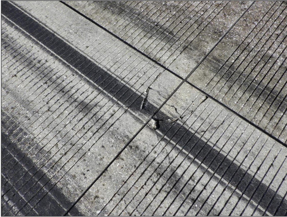
RW 16-34, Section 6105, Sample Unit 450 – Corner Spall
