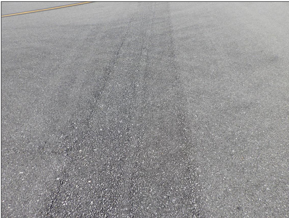
TW F, Section 605, Sample Unit 384 – Raveling
