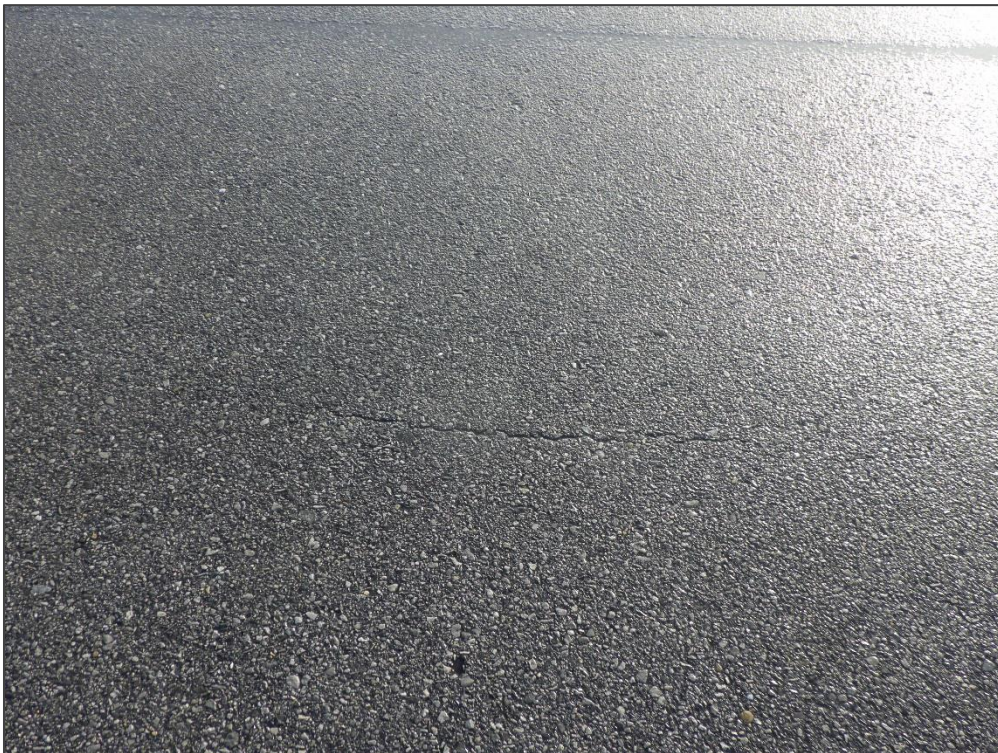
AP TERM, Section 4110, Sample Unit 156 – Longitudinal & Transverse Cracking and Weathering
