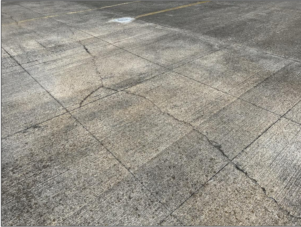
AP, Section 4121, Sample Unit 100 (Whitetopping) – Slab Cracking
