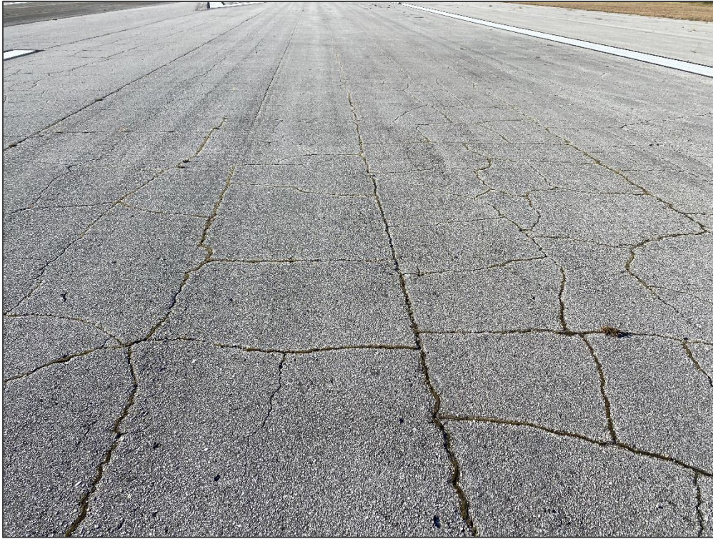
RW 2-20, Section 6405, Sample Unit 107 - Block Cracking
