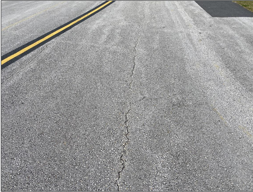
TW C, Section 310, Sample Unit 135 - Longitudinal & Transverse Cracking
