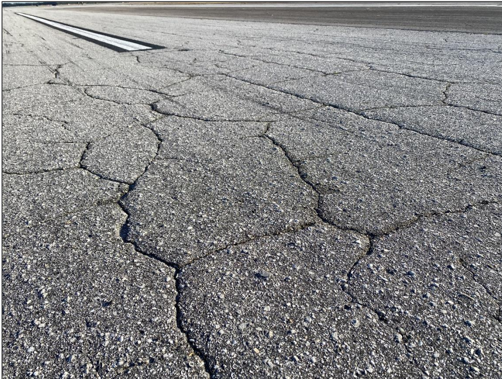
RW 2-20, Section 6425, Sample Unit 128 - Block Cracking
