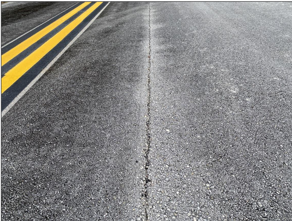
TW B, Section 215, Sample Unit 123 - Longitudinal & Transverse Cracking
