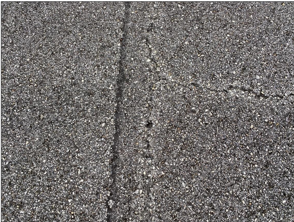
RW 11-29, Section 6105, Sample Unit 170 - Longitudinal & Transverse Cracking
