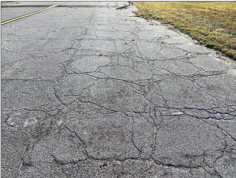
TW D, Section 415, Sample Unit 98 - Block Cracking
