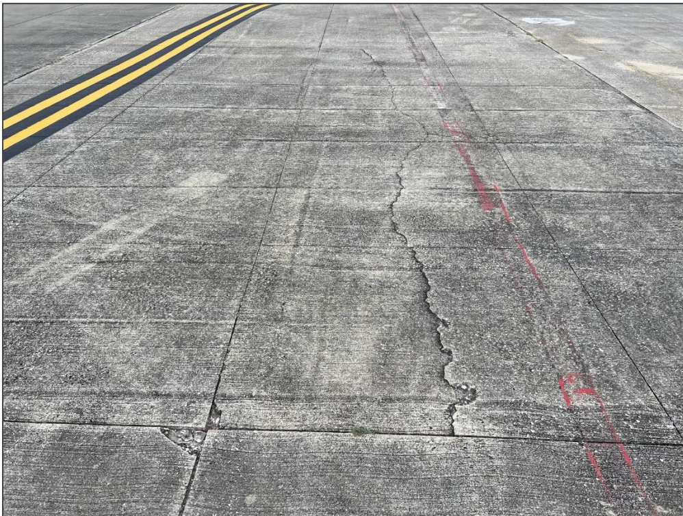
AP, Section 4155, Sample Unit 102 (Whitetopping) – Slab Cracking
