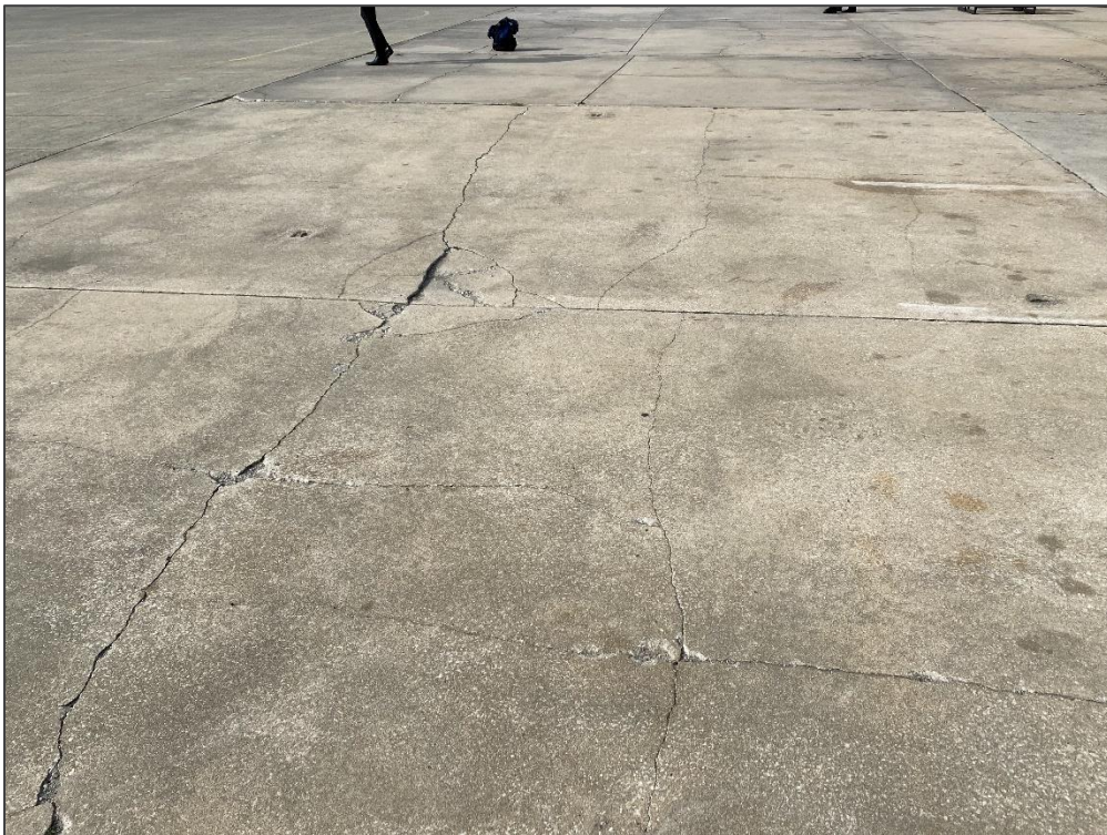
AP, Section 4115, Sample Unit 101 - Shattered Slab
