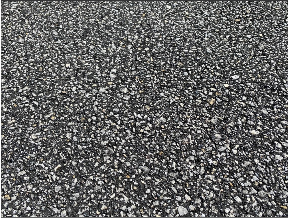
RW 7-25, Section 6202, Sample Unit 103 - Weathering
