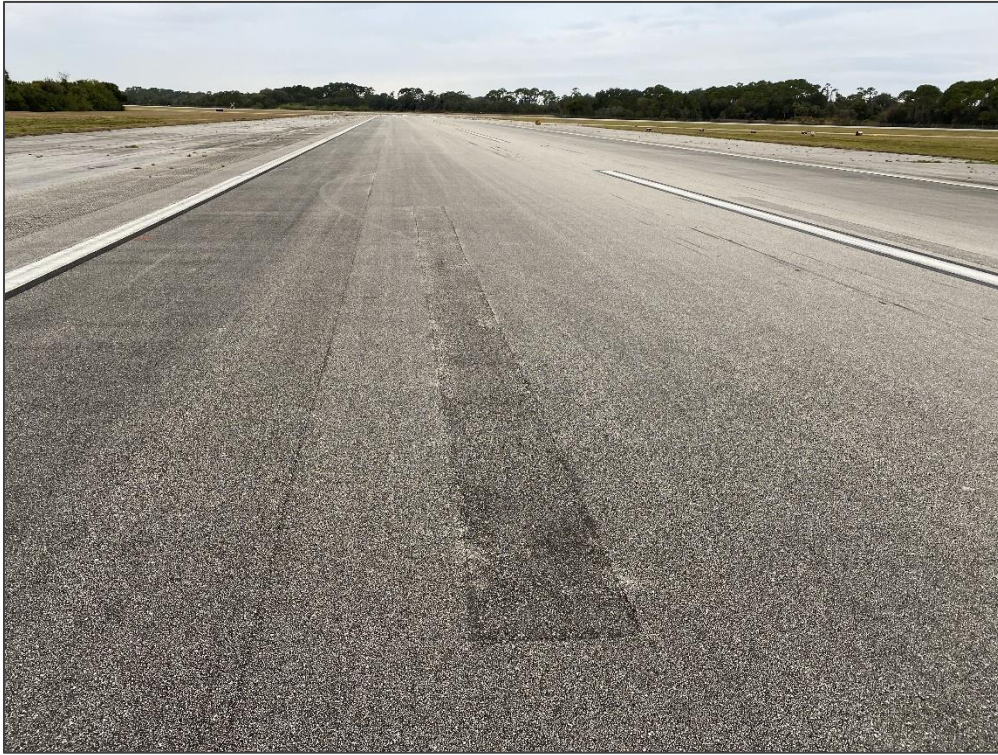
RW 11-29, Section 6105, Sample Unit 119 - Patching
