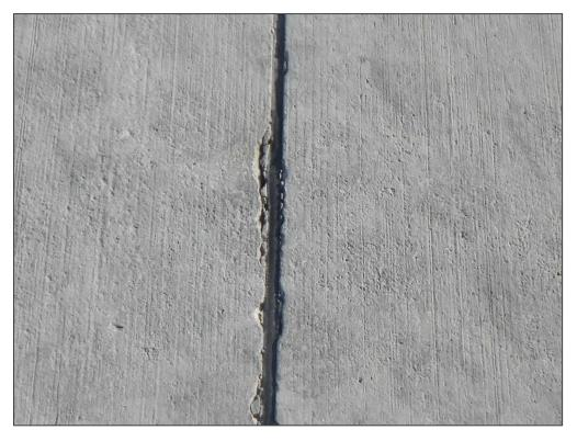
AP TERM, Section 4106, Sample Unit 109 - Joint Seal Damage
