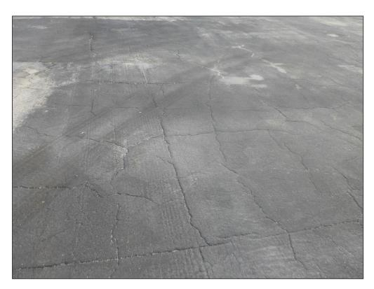
AP TERM, Section 4105, Sample Unit 500 - Block Cracking
