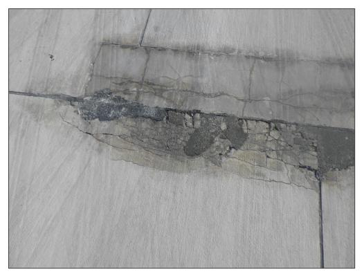
TW B9, Section 257, Sample Unit 201 - Joint Spall
