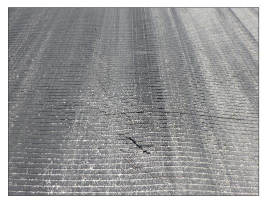
RW 9-27, Section 6105, Sample Unit 127 - Slippage Cracking
