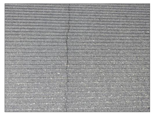
RW 9-27, Section 6105, Sample Unit 172 - Longitudinal & Transverse Cracking
