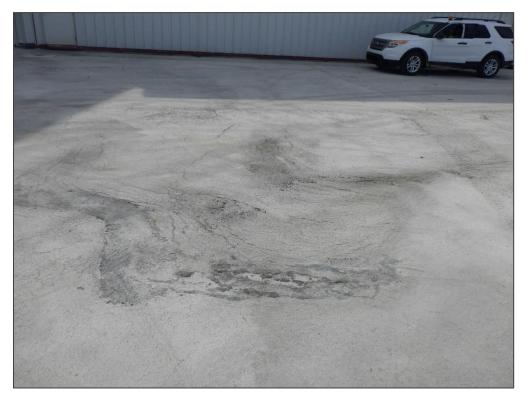
AP GA, Section 4155, Sample Unit 816 - Slippage Cracking
