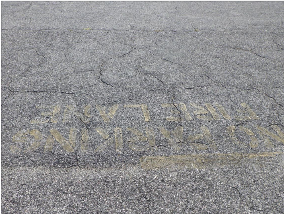
AP NW, Section 4105, Sample Unit 100 – Block Cracking and Swelling
