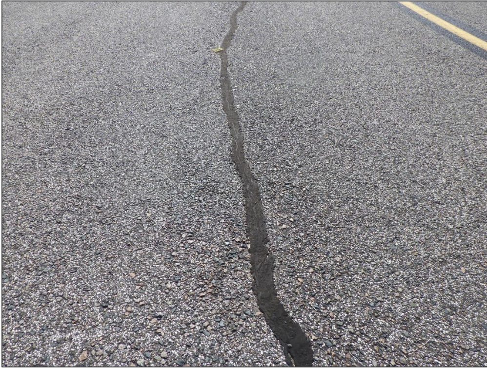
TW D, Section 410, Sample Unit 103 – Longitudinal & Transverse Cracking
