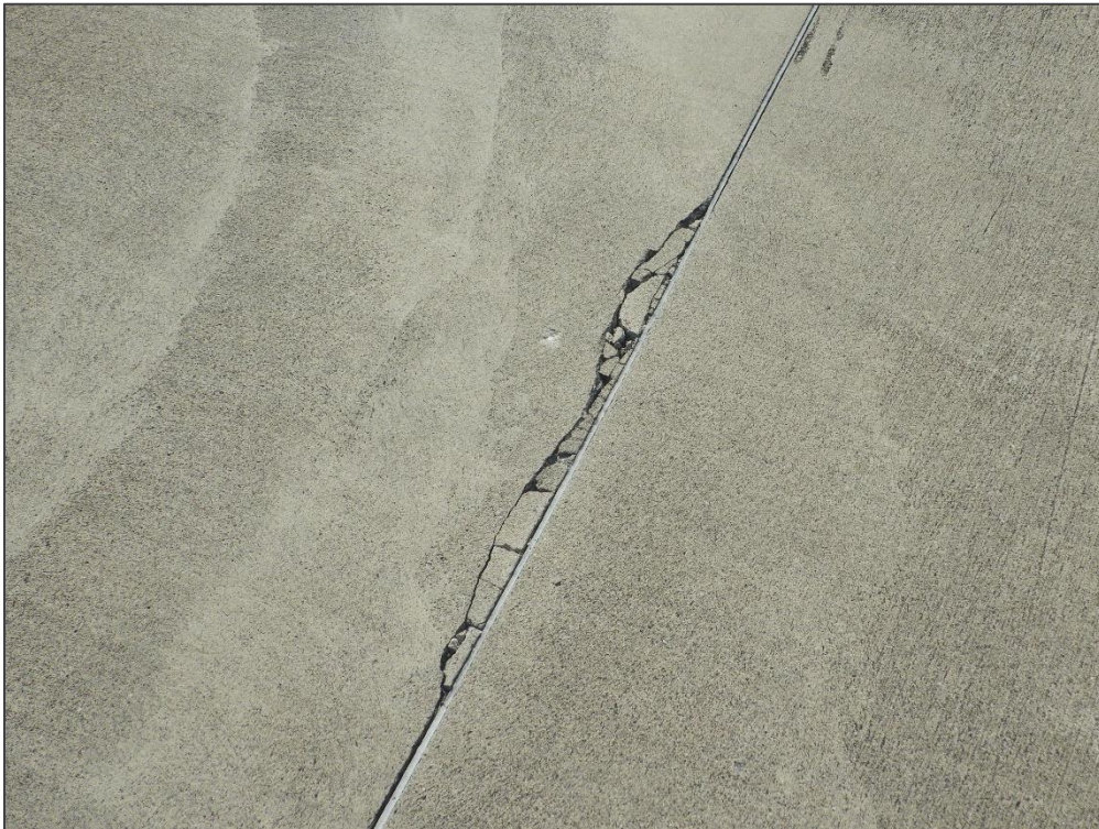
TW C, Section 125, Sample Unit 99 – Joint Spall
