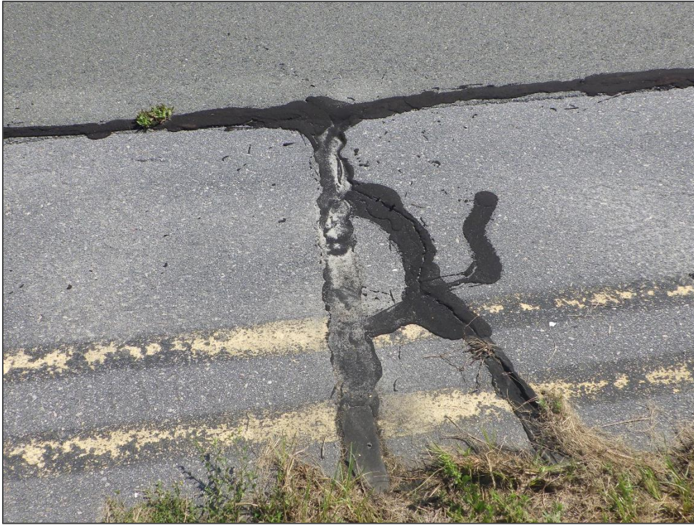
TW B, Section 230, Sample Unit 141 – Longitudinal & Transverse Cracking
