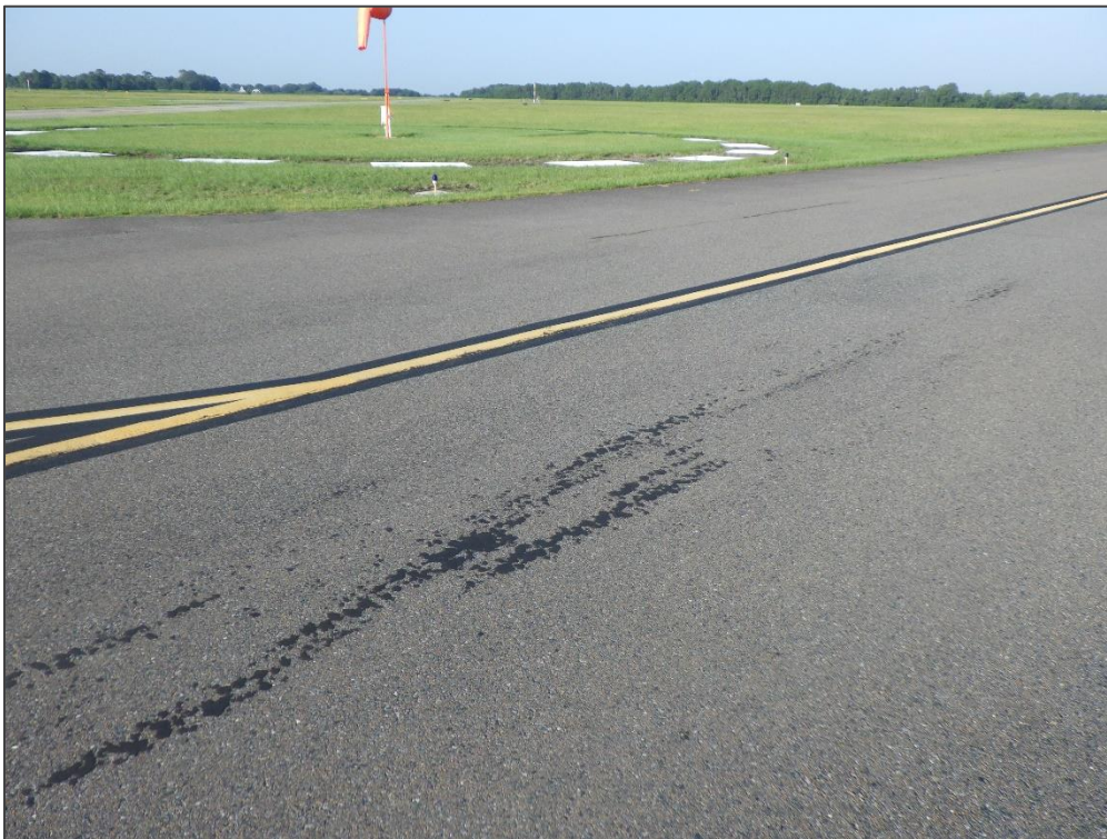
TW A, Section 325, Sample Unit 125 – Bleeding
