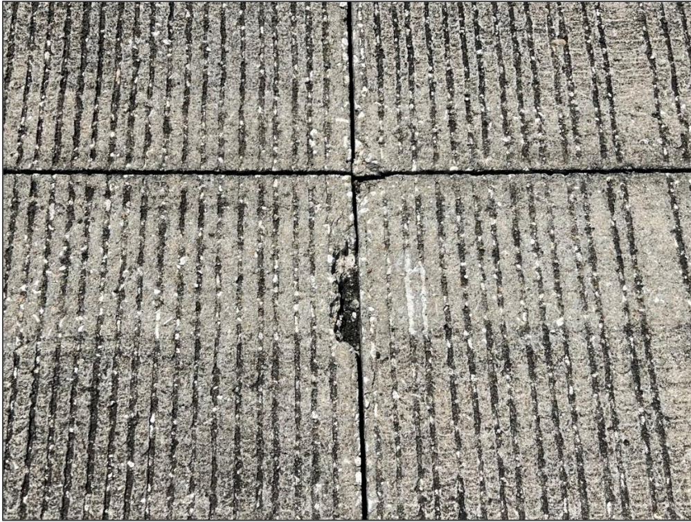
RW 9-27, Section 6315, Sample Unit 324 (Whitetopping) – Spalling
