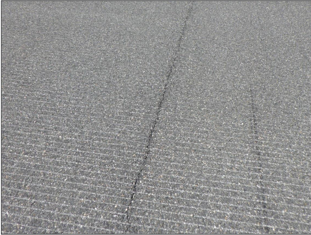
RW 4-22, Section 6110, Sample Unit 185 – Longitudinal & Transverse Cracking
