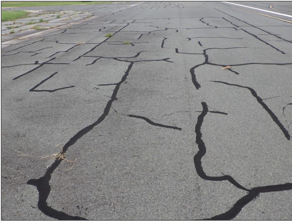
RW 13-31, Section 6215, Sample Unit 365 – Longitudinal & Transverse Cracking
