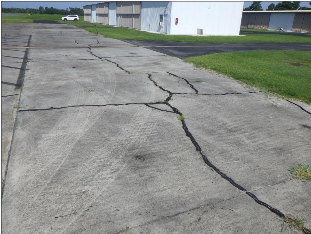
AP N, Section 4220, Sample Unit 365 – Shattered Slab
