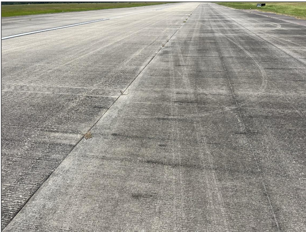
RW 9-27, Section 6330, Sample Unit 364 (Whitetopping) – Joint Seal Damage
