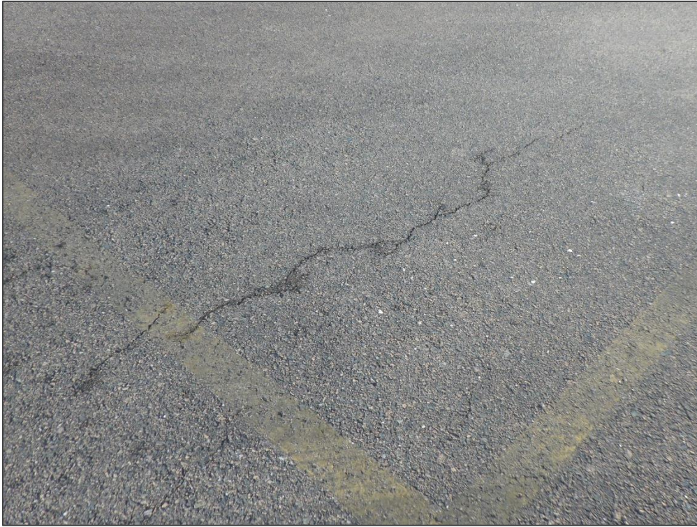
AP N, Section 4240, Sample Unit 252 – Longitudinal & Transverse Cracking
