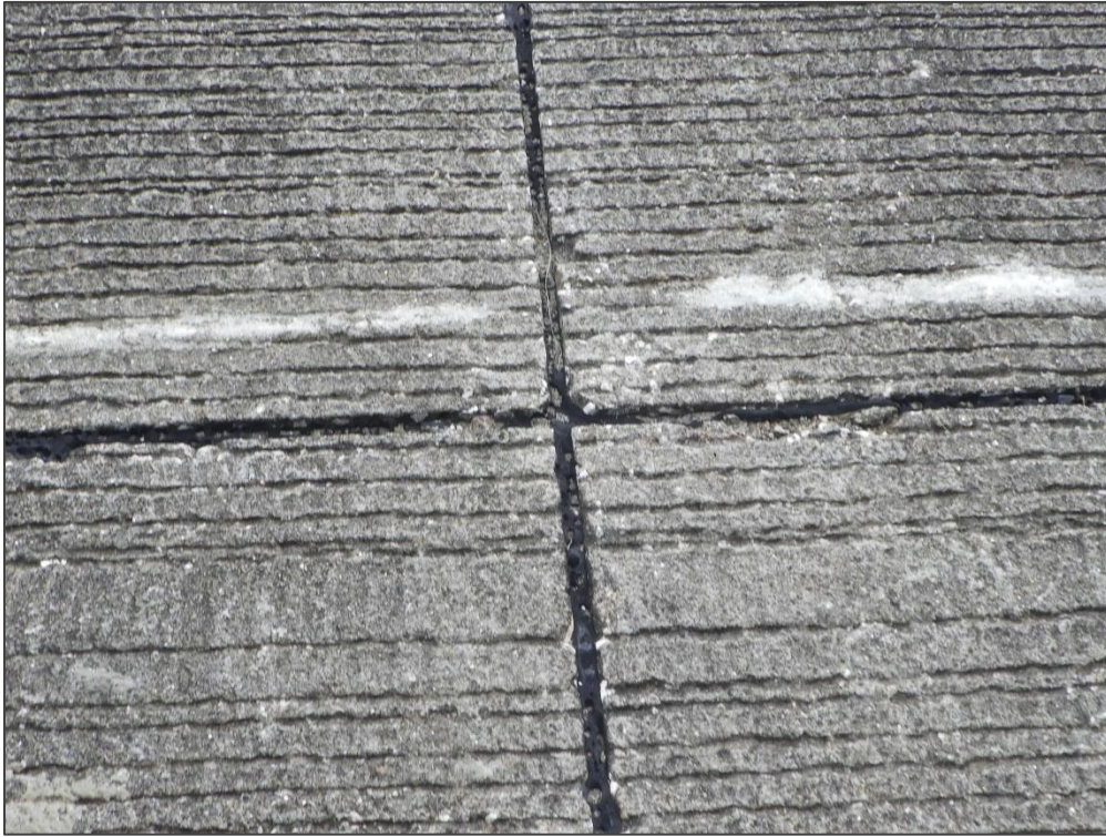
RW 9-27, Section 6335, Sample Unit 406 – Joint Seal Damage
