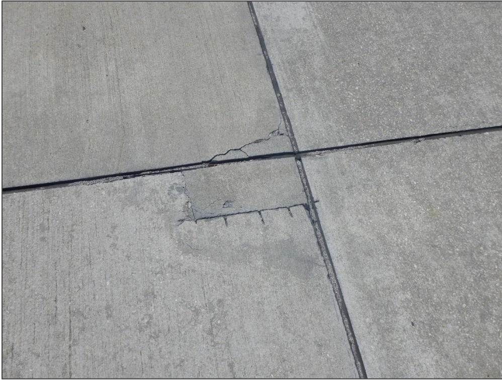
AP TERM 1, Section 4110, Sample Unit 356 – Small Patch and Corner Spall
