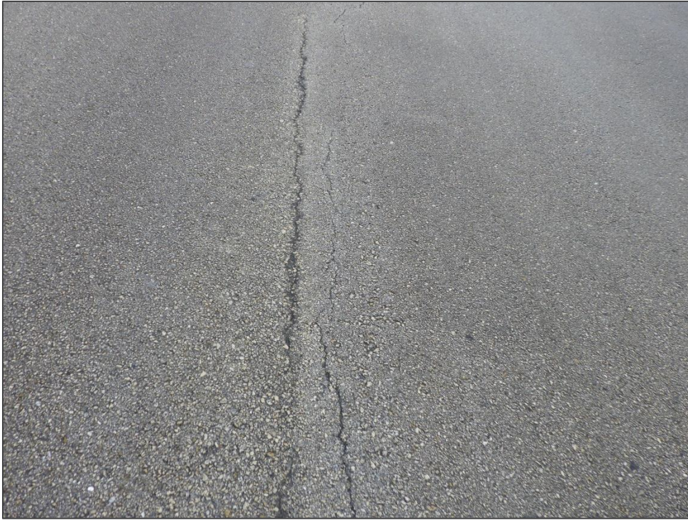
TW A, Section 157, Sample Unit 466 – Longitudinal & Transverse
