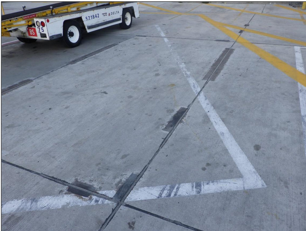
AP TERM 2, Section 4220, Sample Unit 341 – Small Patch
