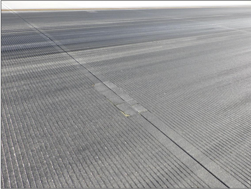
RW 10R-28L, Section 6205, Sample Unit 332 – Small Patch
