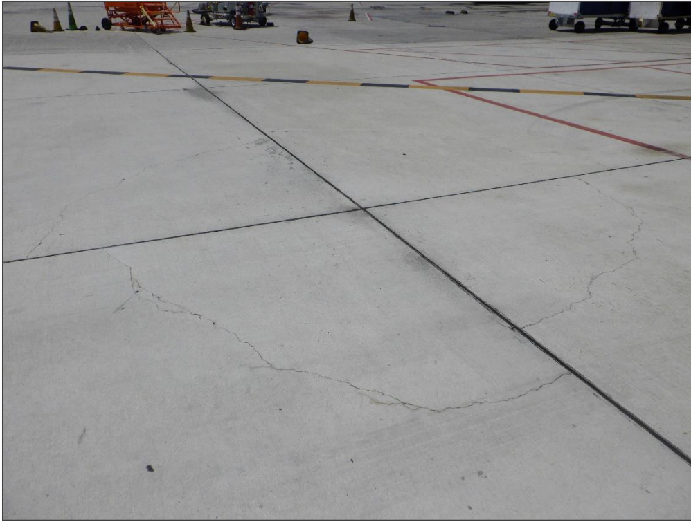
AP TERM 4, Section 4410, Sample Unit 298 – Corner Break
