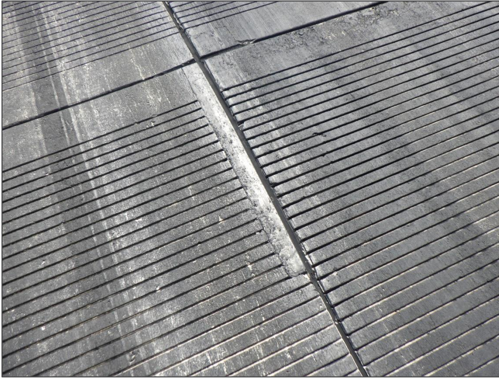
RW 10L-28R, Section 6115, Sample 319 – Small Patch
