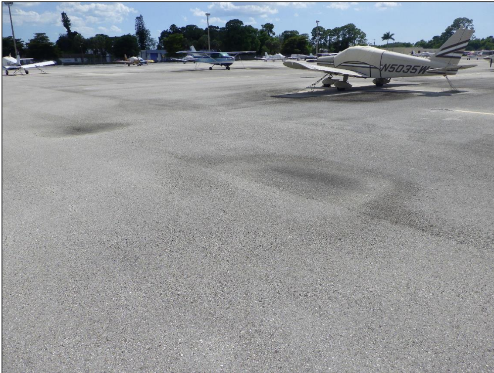
AP SE, Section 4420, Sample Unit 707 – Depression
