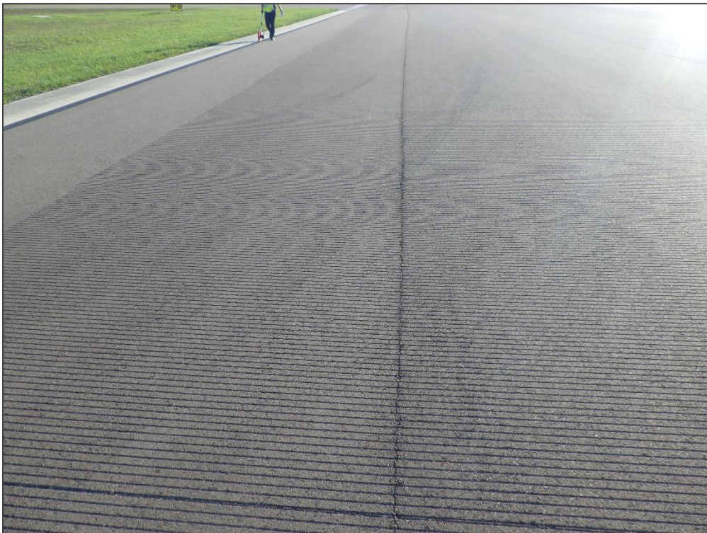
RW 5-23, Section 6140, Sample Unit 180 – Longitudinal & Transverse Cracking
