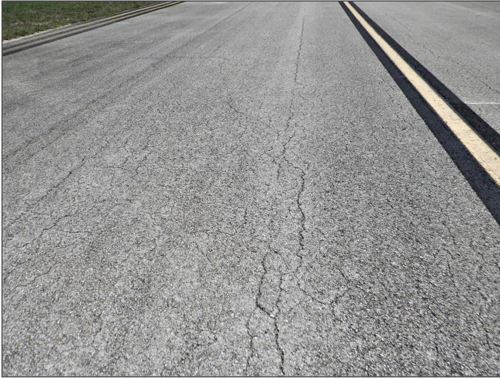
TW D2, Section 160, Sample 101 – Alligator Cracking
