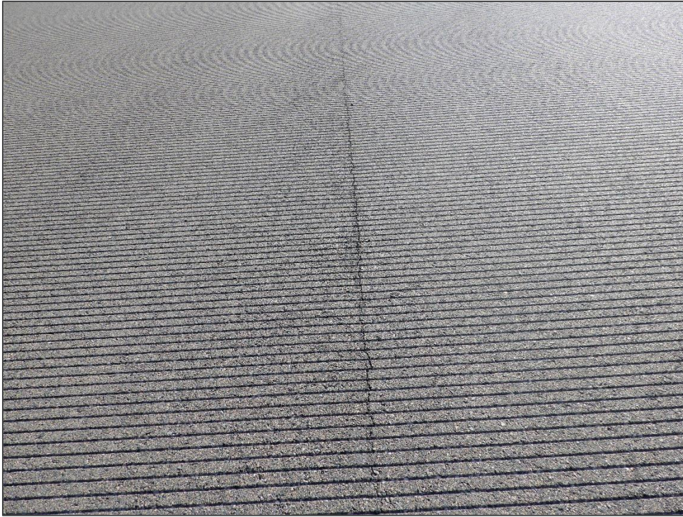
RW 5-23, Section 6115, Sample Unit 346 – Longitudinal & Transverse Cracking
