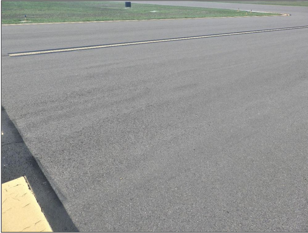
TW A, Section 110, Sample Unit 141 – Swelling
