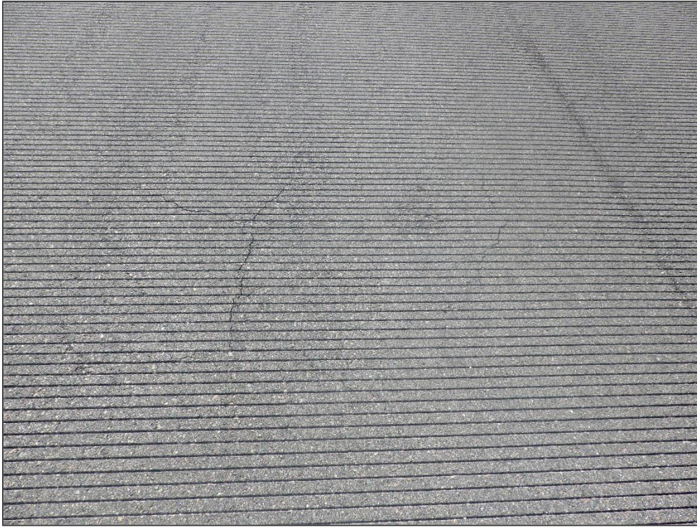
RW 13-31, Section 6205, Sample Unit 381 – Longitudinal & Transverse Cracking
