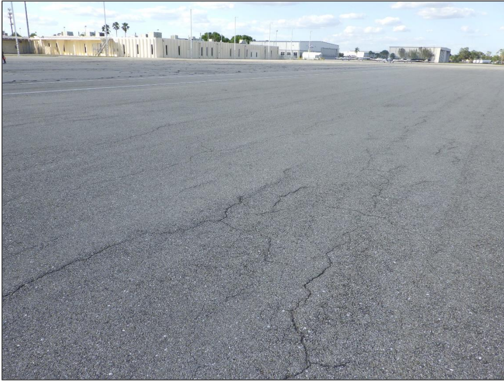
AP N, Section 4305, Sample Unit 502 – Longitudinal & Transverse Cracking and Swelling
