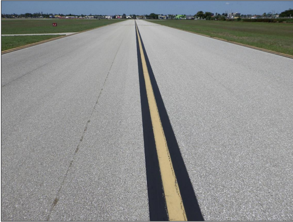
TW C, Section 305, Sample Unit 213 – Longitudinal & Transverse Cracking
