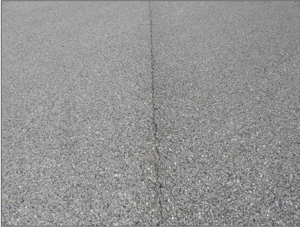
AP W, Section 4805, Sample Unit 451 – Longitudinal & Transverse Cracking
