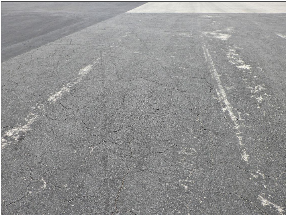
AP S, Section 4120, Sample Unit 103 – Block Cracking and Raveling
