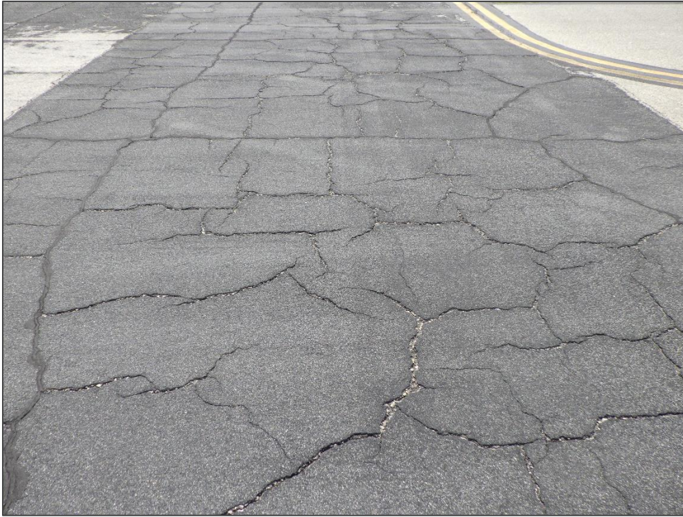
AP SE, Section 4415, Sample Unit 102 – Block Cracking
