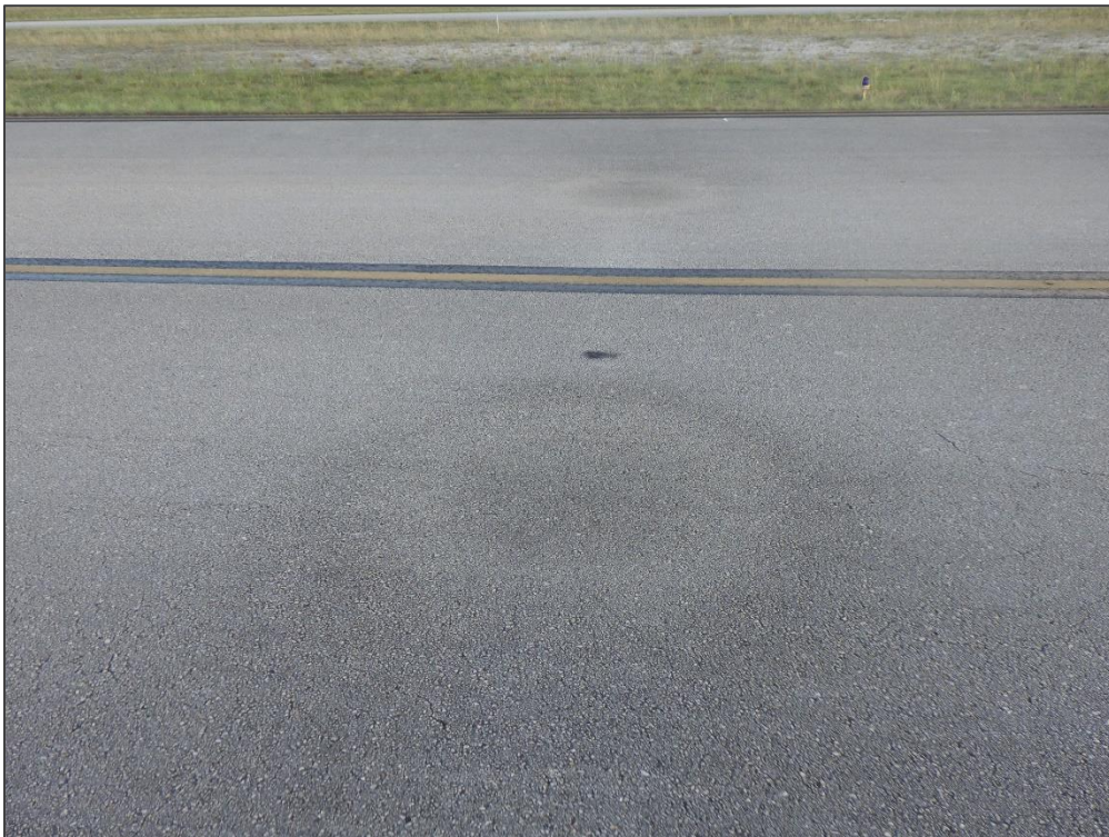
TW E, Section 530, Sample Unit 148 – Depression
