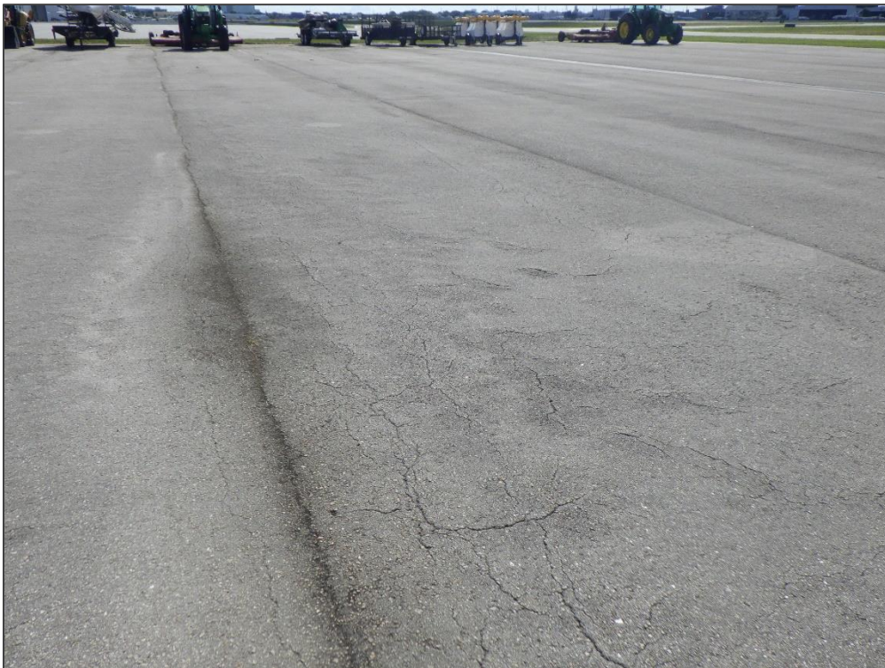
AP MAINT, Section 5405, Sample Unit 104 – Longitudinal & Transverse Cracking and Swelling
