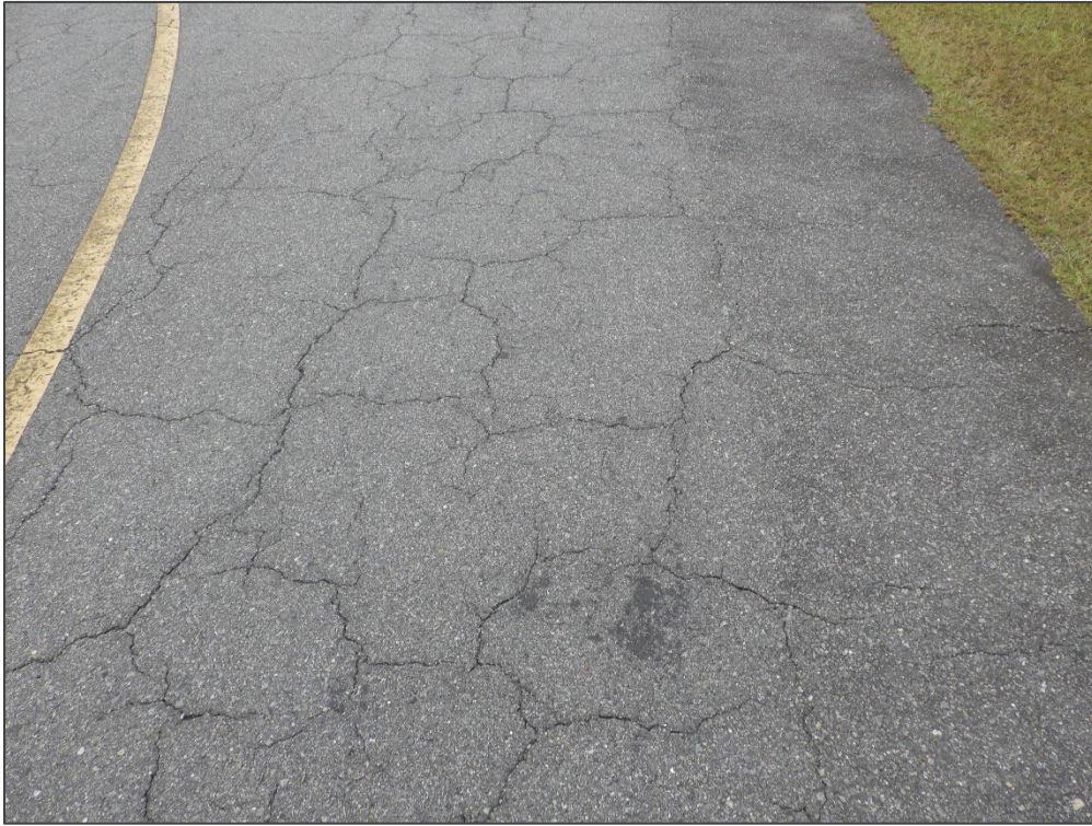
TL T-HANG, Section 915, Sample Unit 300 – Block Cracking
