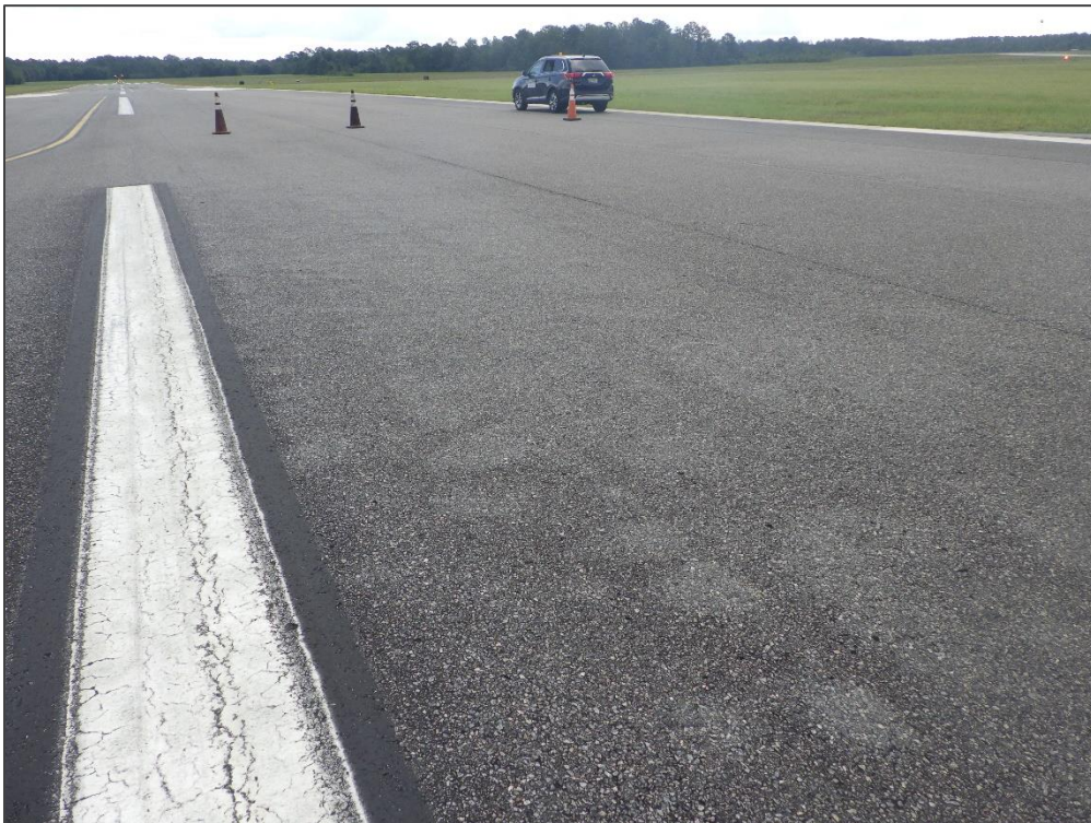
RW 7-25, Section 6110, Sample Unit 149 – Swelling
