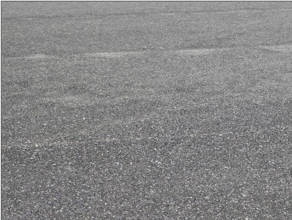
AP NW, Section 4115, Sample Unit 502 – Swelling and Weathering
