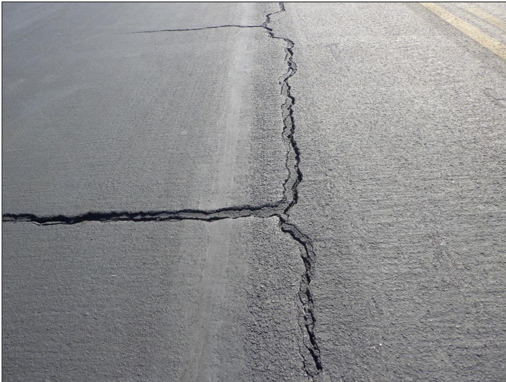
AP FBO, Section 4220, Sample Unit 250 – Longitudinal & Transverse Cracking
