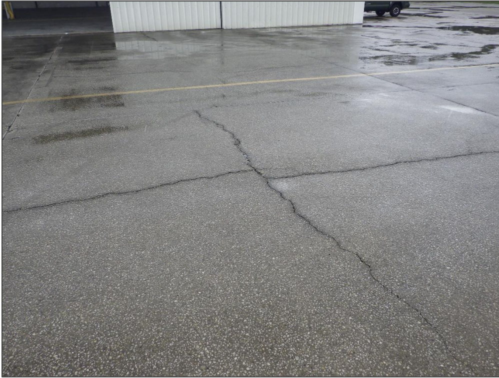
AP NE, Section 4410, Sample Unit 101 – Shattered Slab
