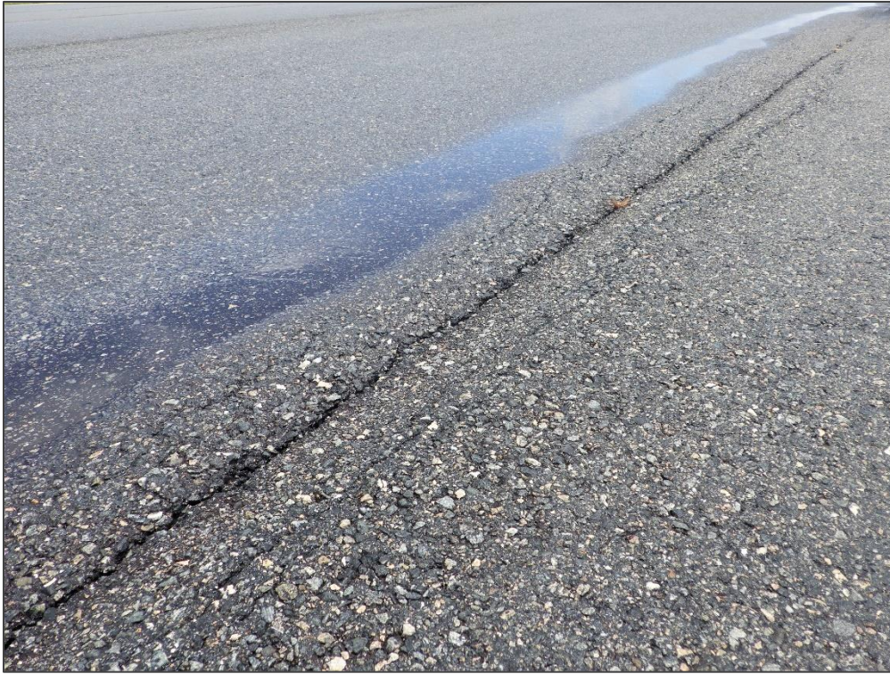
RW 7-25, Section 6105, Sample Unit 161 – Longitudinal & Transverse Cracking and Swelling
