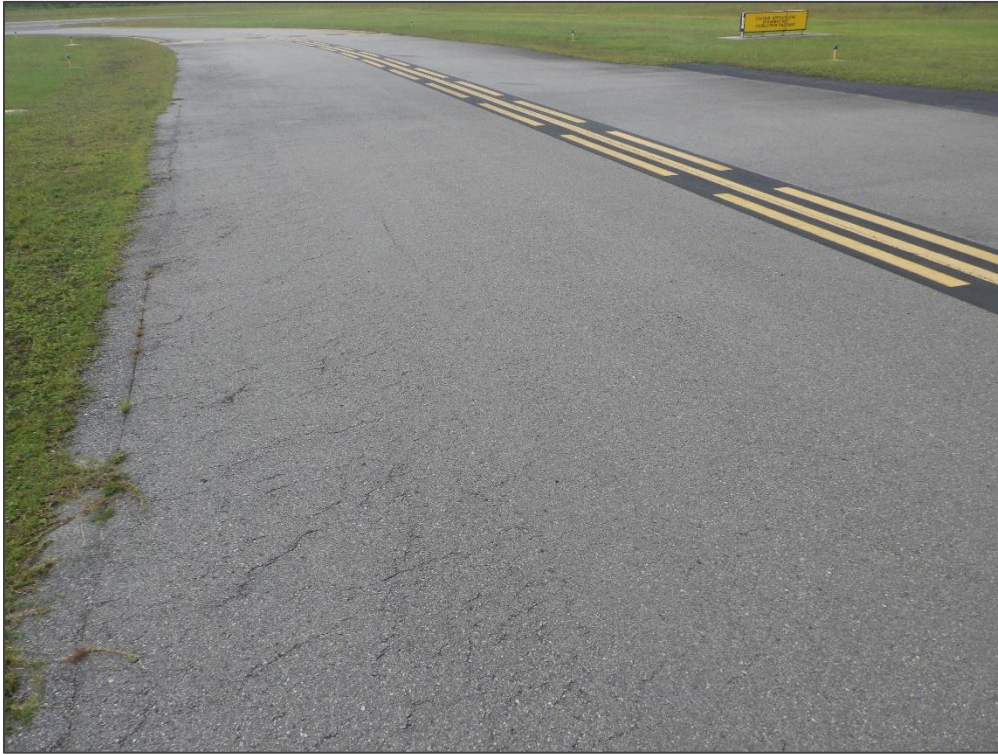
TW A, Section 105, Sample Unit 102 – Longitudinal & Transverse Cracking and Patching
