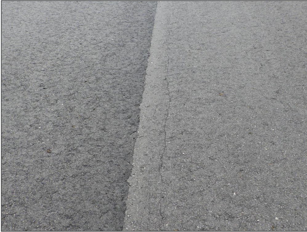
RW 11-29, Section 6205, Sample Unit 143 – Longitudinal & Transverse Cracking
