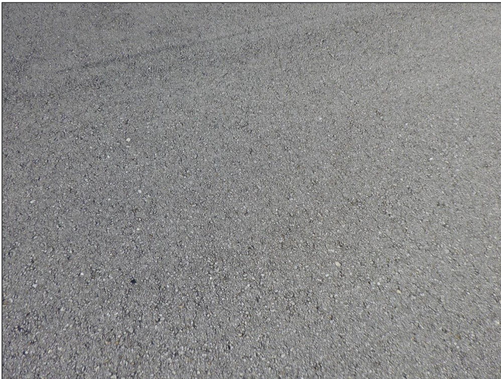
RW 10L-28R, Section 6205, Sample Unit 120 - Weathering
