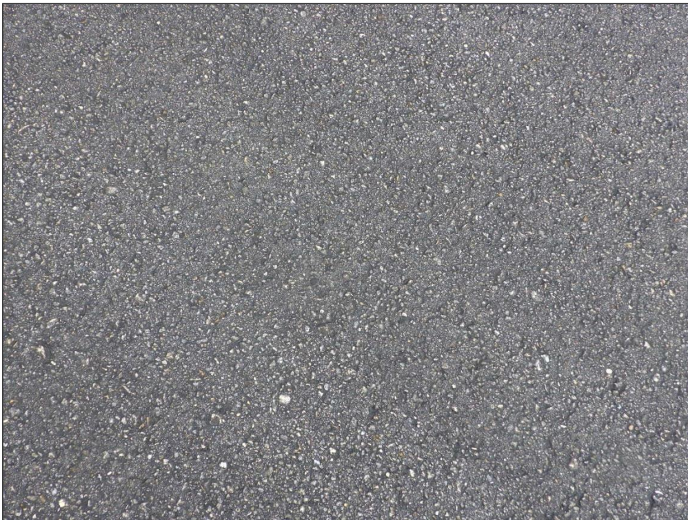
RW 01R-19L, Section 6305, Sample Unit 149 - Weathering
