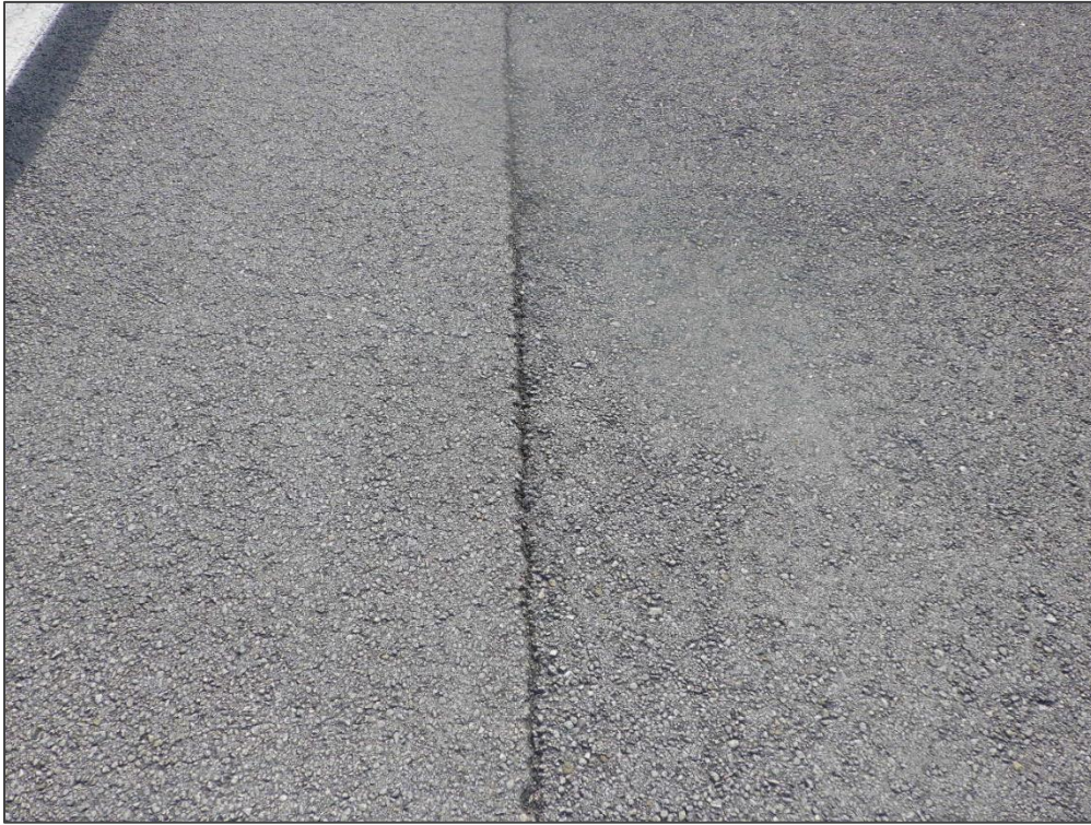
RW 10R-28L, Section 6405, Sample Unit 101 - Longitudinal & Transverse Cracking
