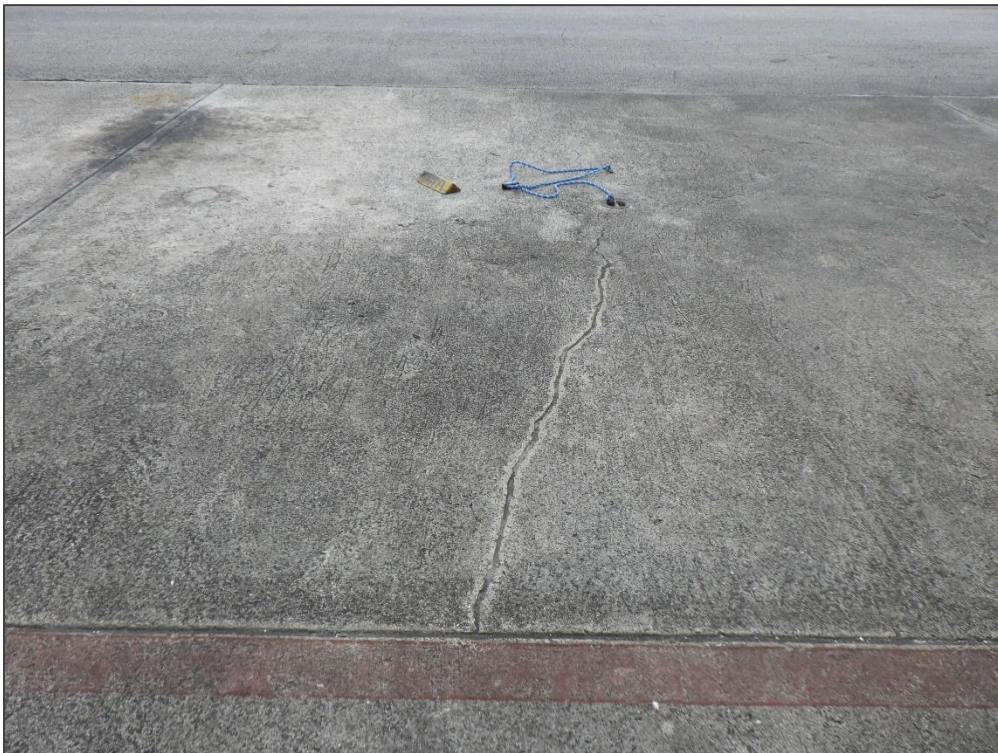
AP SOUTH, Section 4110, Sample Unit 303 - Linear Cracking
