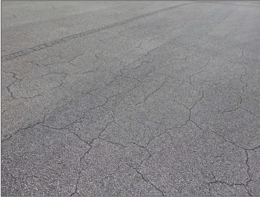
AP SOUTH, Section 4105, Sample Unit 309 - Block Cracking
