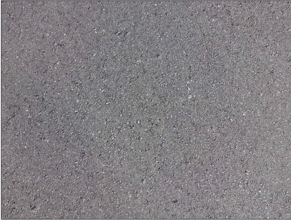
RW 10L-28R, Section 6205, Sample Unit 103 - Weathering
