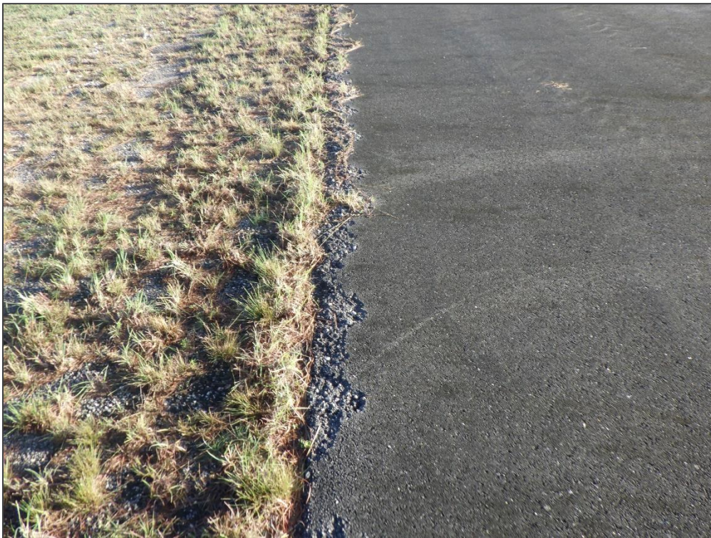
RW 01L-19R, Section 6105, Sample Unit 126 -Raveling
