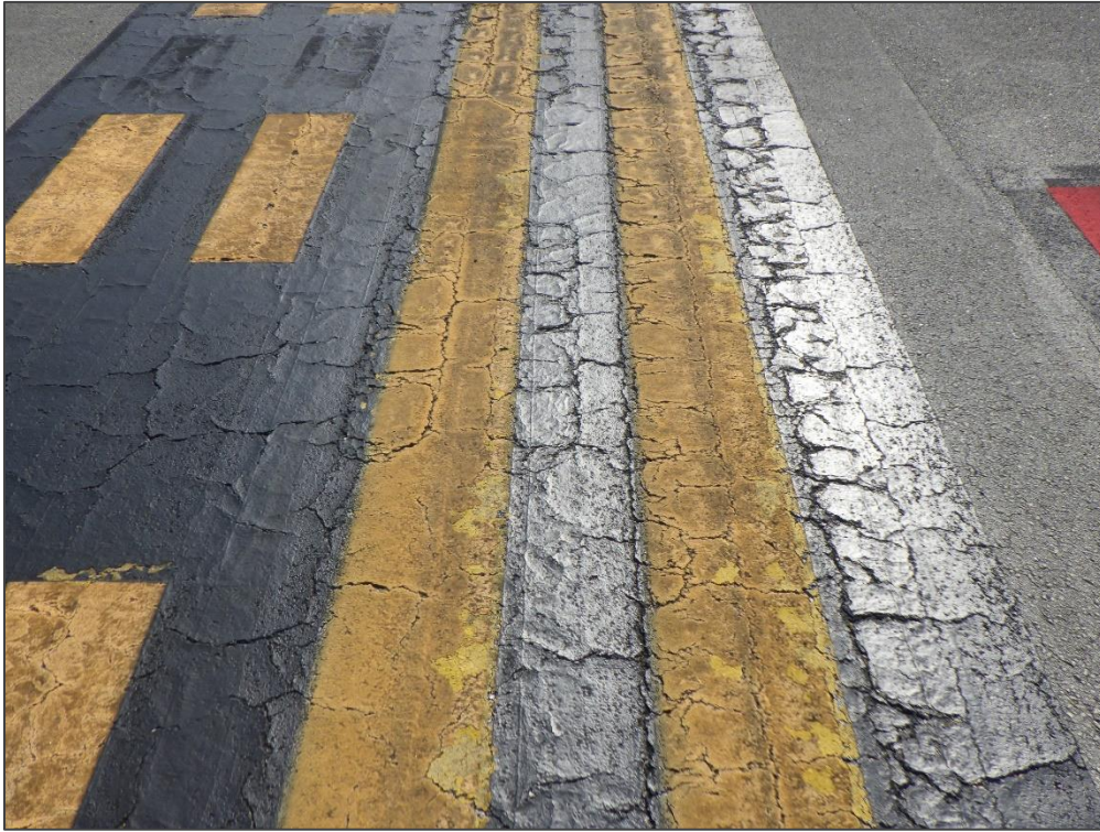
TW D, Section 403, Sample Unit 100 - Raveling
