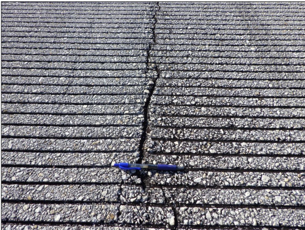
RW 15-33, Section 6150, Sample Unit 369 - Longitudinal & Transverse Cracking
