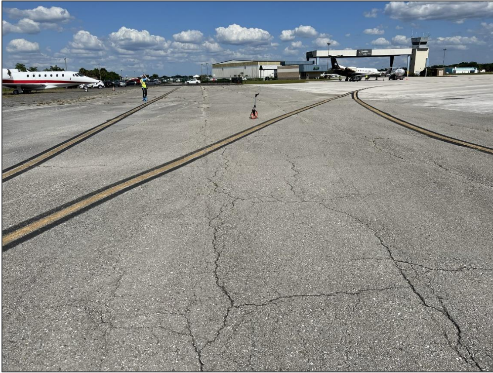
AP N, Section 4115, Sample Unit 119 - Block Cracking
