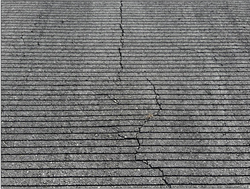
RW 6-24, Section 6226, Sample Unit 354 - Longitudinal & Transverse Cracking
