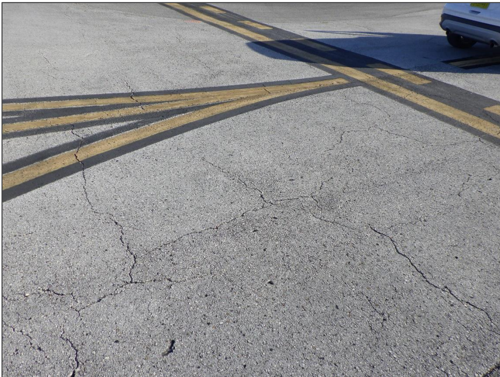
AP NW, Section 4305, Sample Unit 100 - Block Cracking
