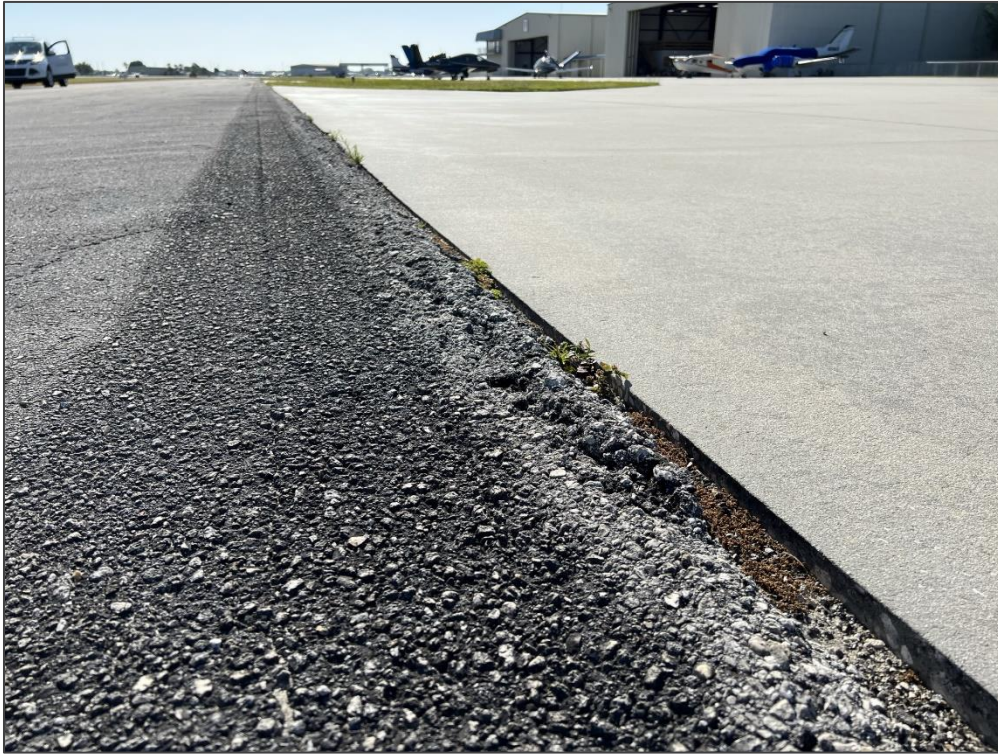
TW C, Section 320, Sample Unit 112 - Shoving
