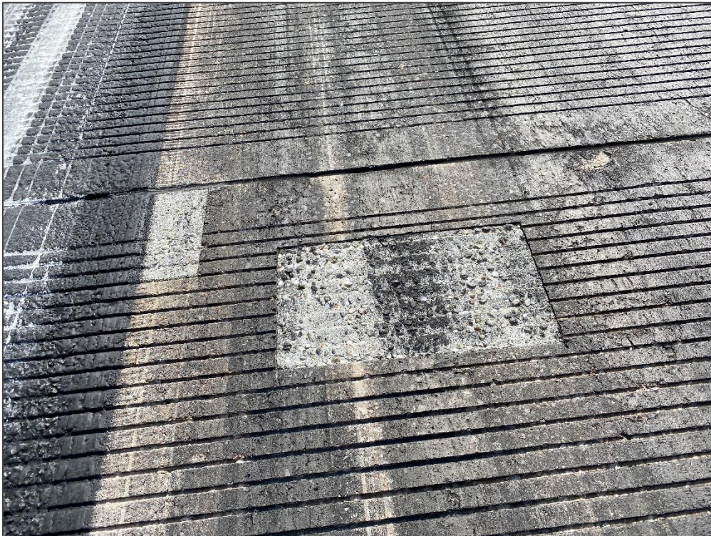
RW 8-26, Section 6105, Sample Unit 369 – Small Patch
