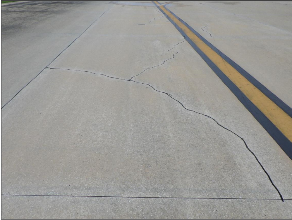
TW H, Section 555, Sample Unit 101 – Corner Break and Linear Cracking
