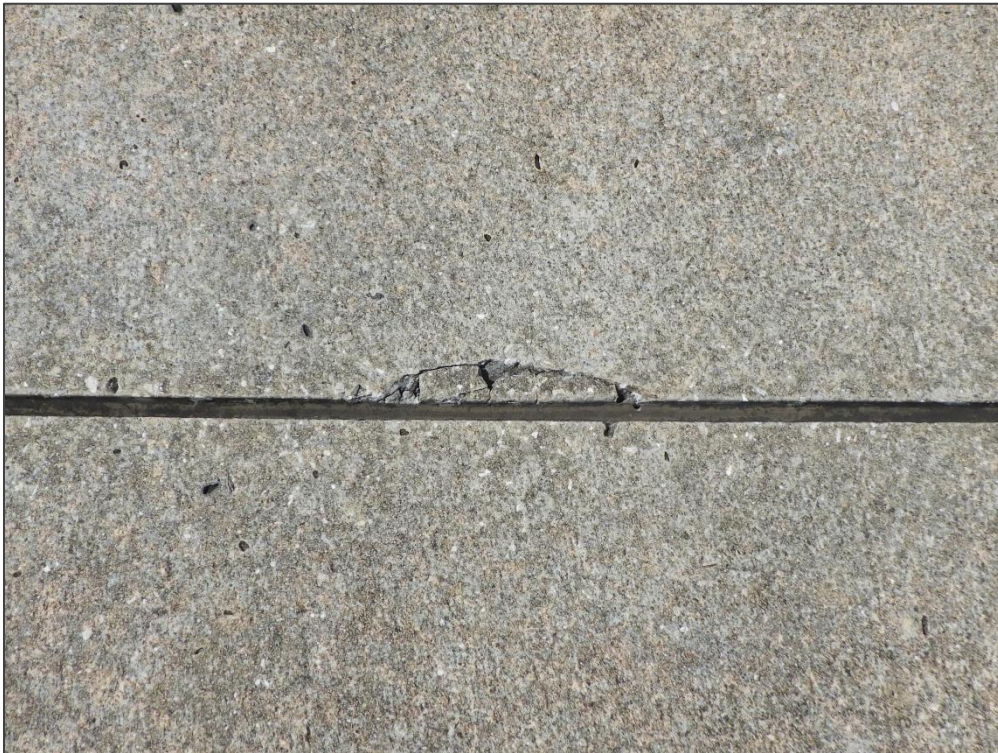
TW R, Section 575, Sample Unit 104 – Joint Spall
