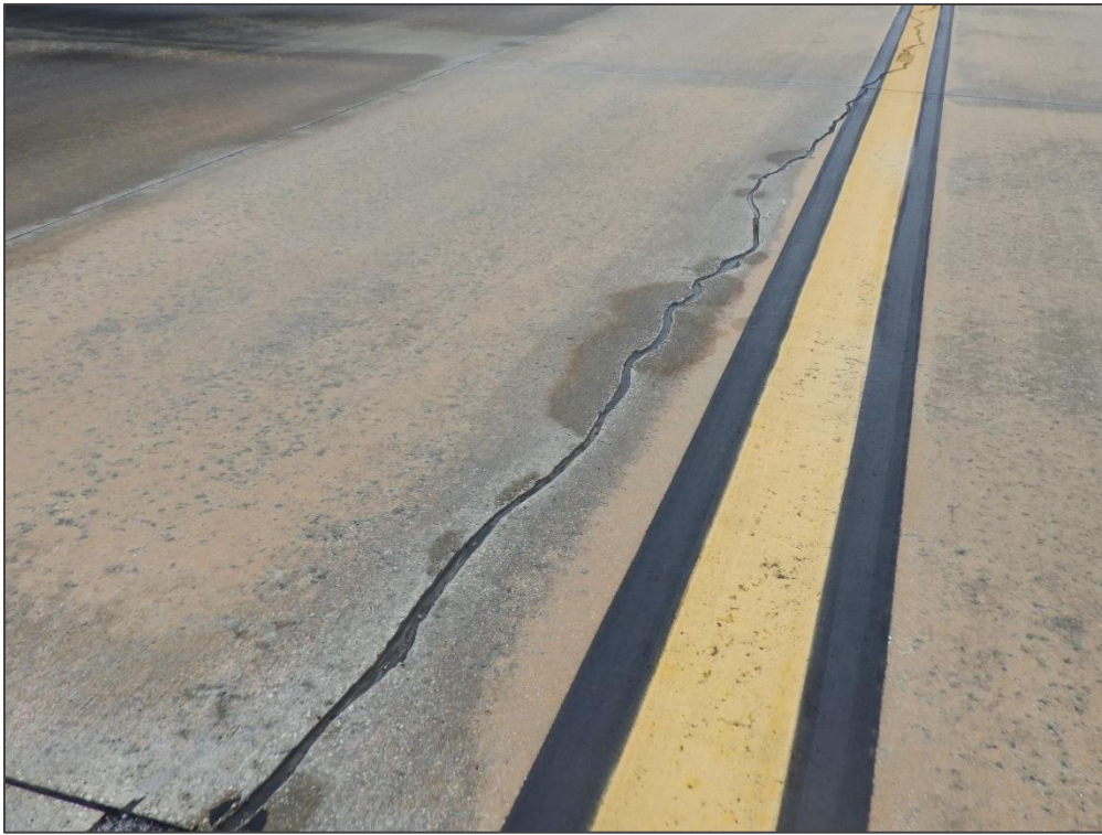
TW A, Section 125, Sample Unit 149 – Linear Cracking
