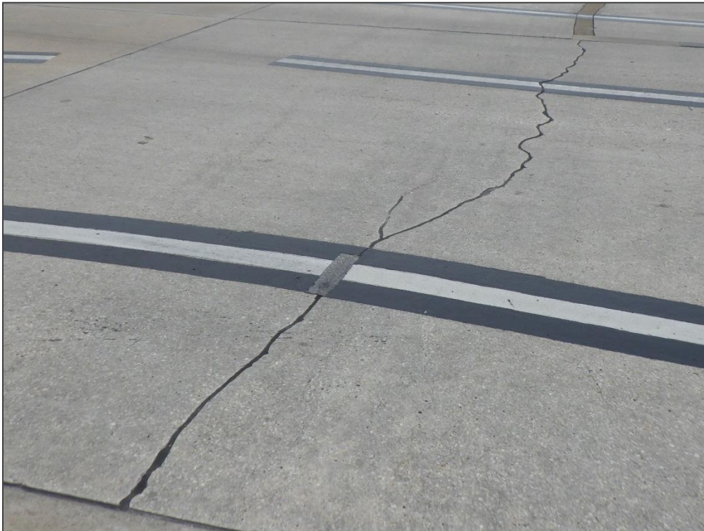
AP TERM, Section 4430, Sample Unit 604 – Linear Cracking and Small Patch
