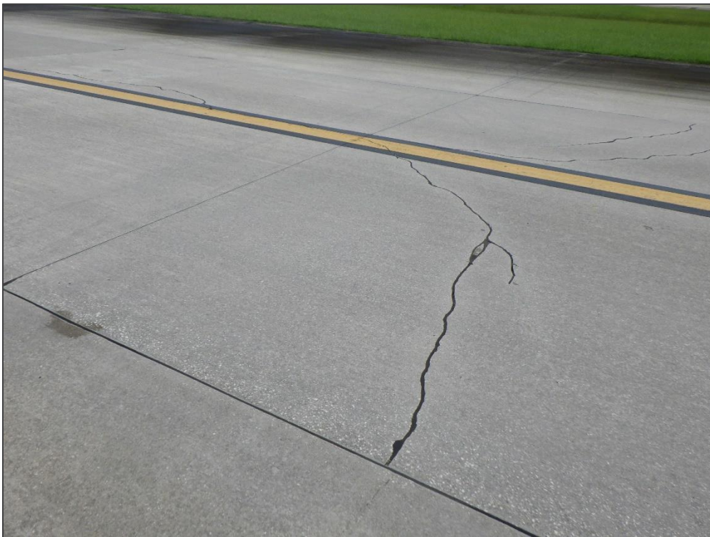
TW A, Section 120, Sample Unit 135 – Corner Break
