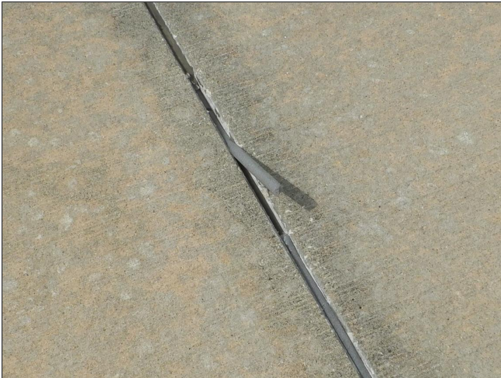
TW J, Section 765, Sample Unit 114 – Joint Seal Damage
