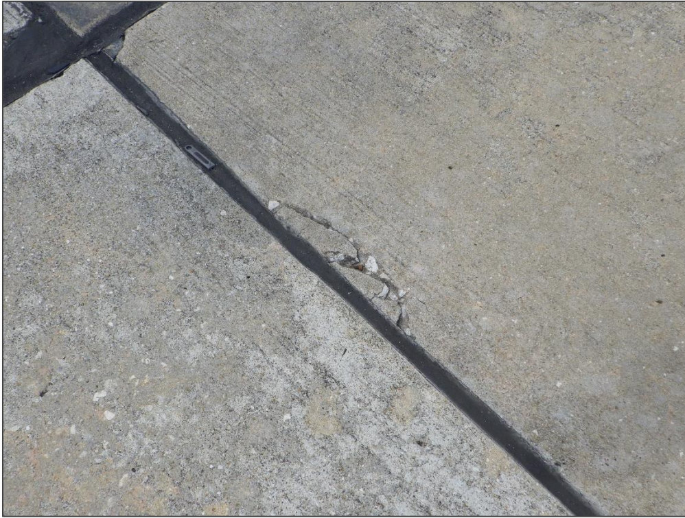
AP TERM, Section 4435, Sample Unit 609 – Joint Spall
