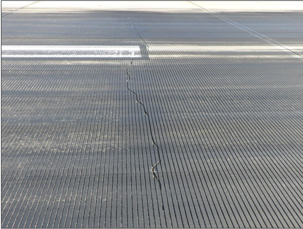
RW 8-26, Section 6105, Sample Unit 309 – Linear Cracking
