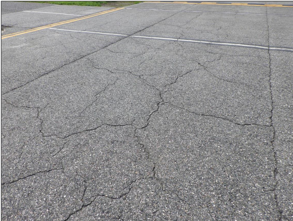
TW F, Section 1155, Sample Unit 102 – Block Cracking
