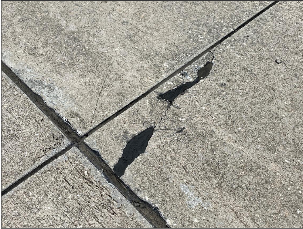
TW B, Section 805, Sample Unit 114 – Corner Spall
