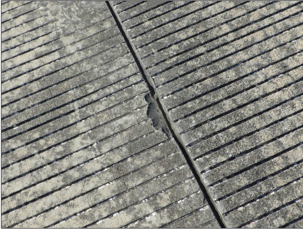
RW 14-32, Section 6215, Sample Unit 521 – Joint Spall
