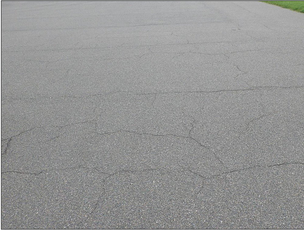
AP GA, Section 5105, Sample Unit 89 – Block Cracking
