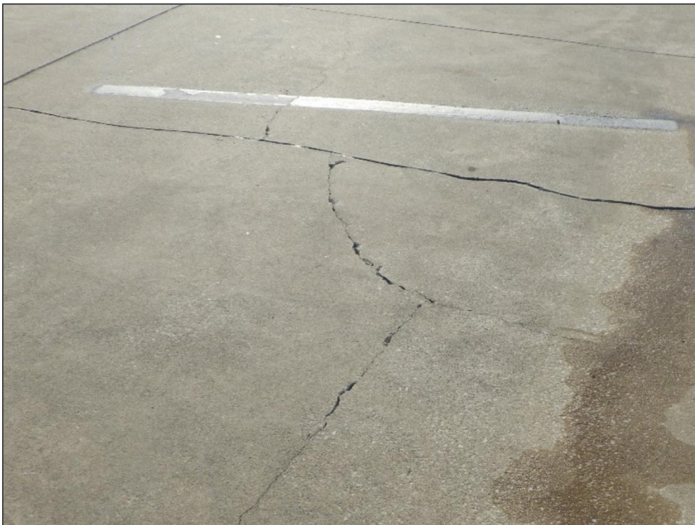
AP CARGO, Section 4135, Sample Unit 451 – Shattered Slab
