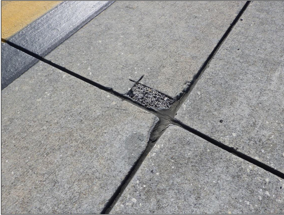
TW N, Section 305, Sample Unit 134 – Small Patch
