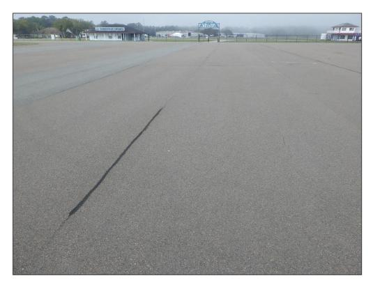
AP CENTER, Section 4510, Sample Unit 94 – Longitudinal & Transverse Cracking and Patching
