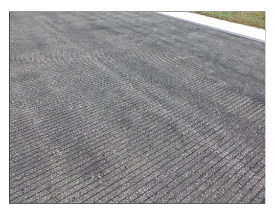
RW 5-23, Section 6250, Sample Unit 592 - Longitudinal & Transverse Cracking
