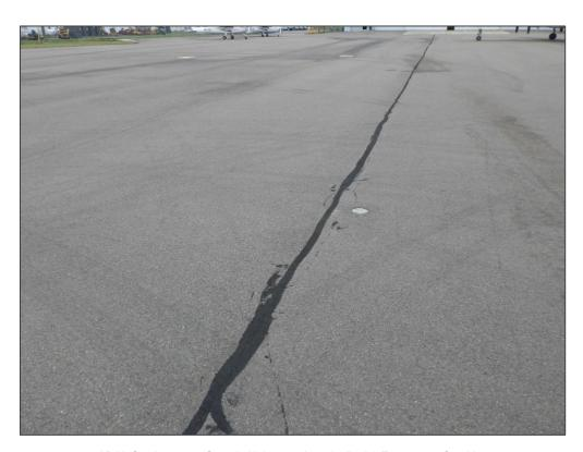
AP N, Section 4155, Sample Unit 107 - Longitudinal & Transverse Cracking
