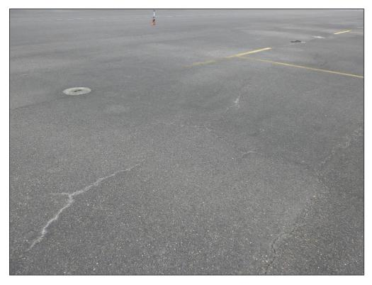
AP SE, Section 4310, Sample Unit 601 - Longitudinal & Transverse Cracking
