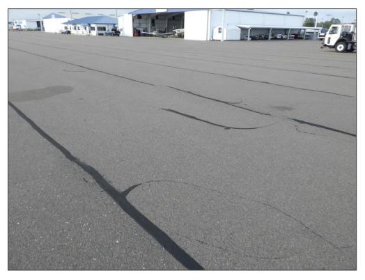
AP N, Section 4115, Sample Unit 307 - Longitudinal & Transverse Cracking
