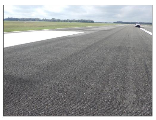
RW 5-23, Section 6215, Sample Unit 322 – Longitudinal & Transverse Cracking
