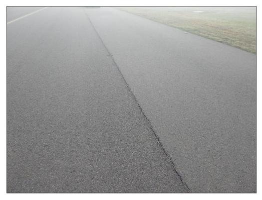
TW D, Section 405, Sample Unit 110 - Longitudinal & Transverse Cracking
