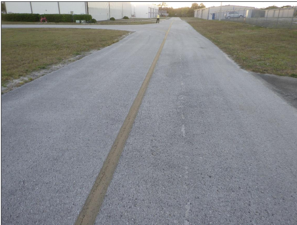
TL T-HANG, Section 4205, Sample Unit 105 – Vicinity
