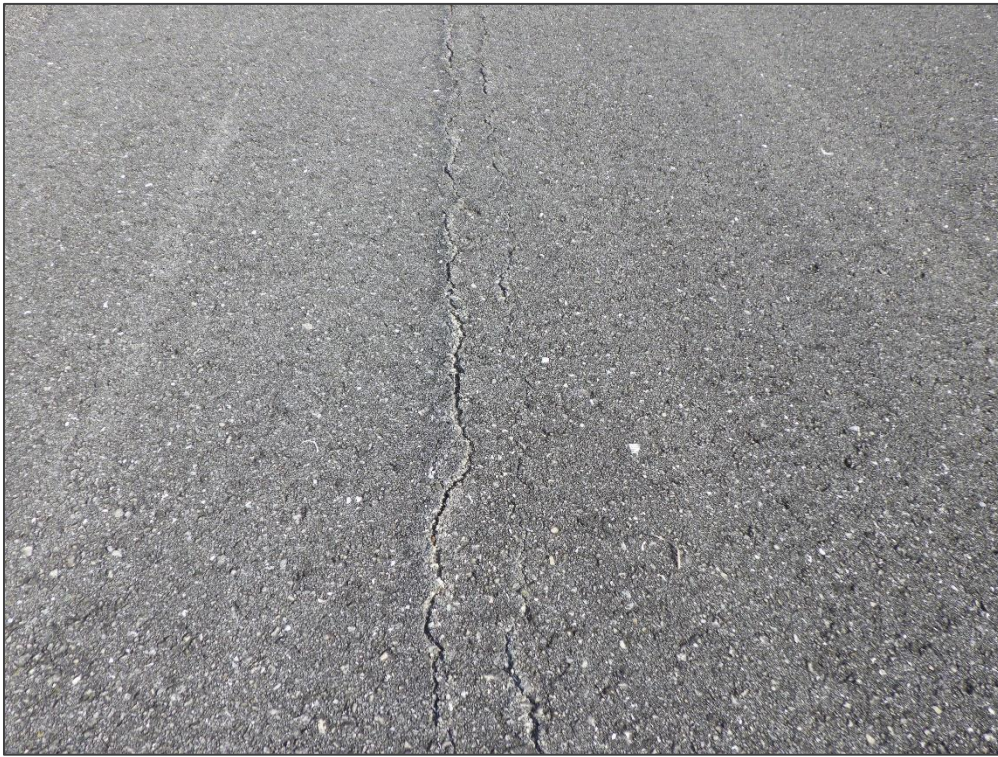
RW 16-34, Section 6215, Sample Unit 152 – Longitudinal and Transverse Cracking
