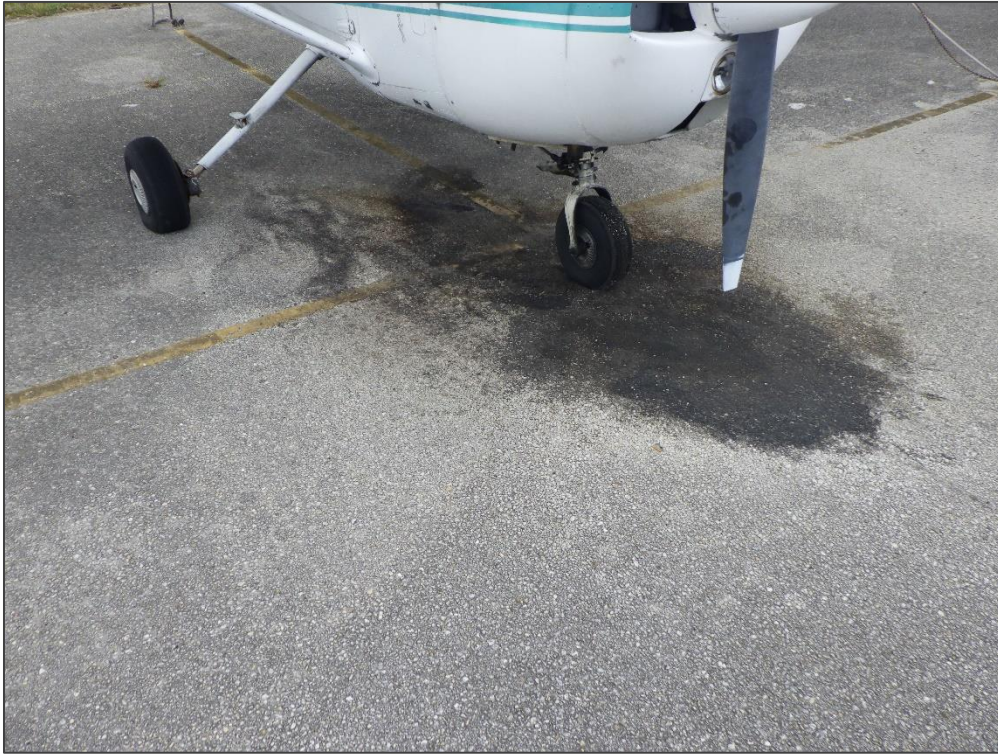
AP GA, Section 4110, Sample Unit 553 – Oil Spillage
