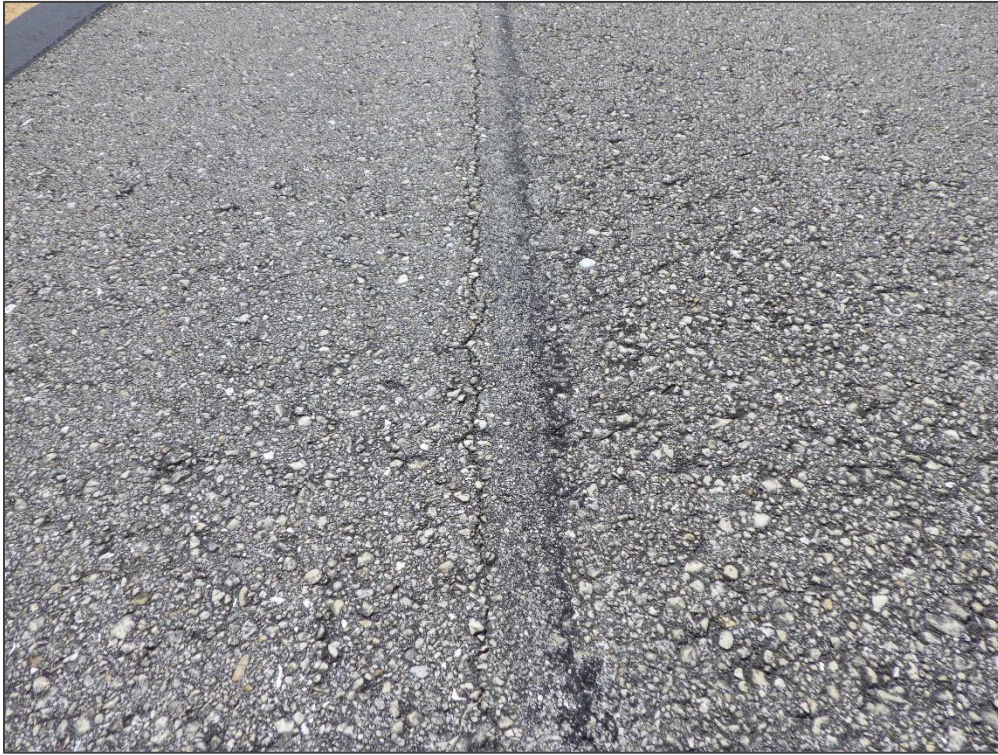
TW C, Section 105, Sample Unit 115 – Longitudinal and Transverse Cracking
