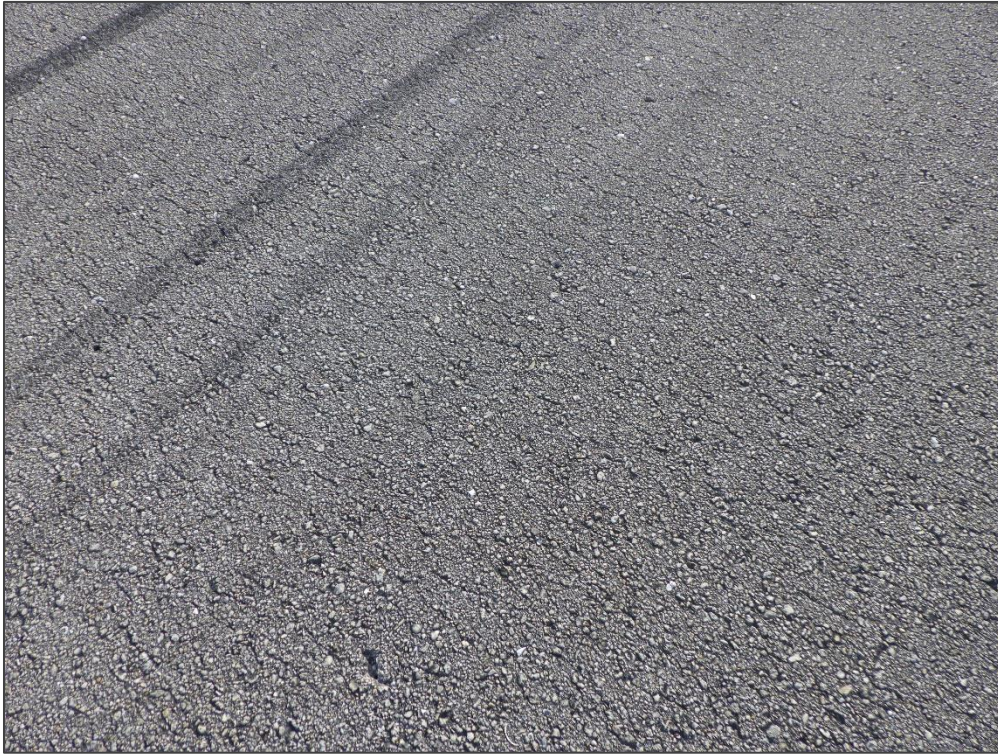
RW 10-28, Section 6105, Sample Unit 331 – Weathering
