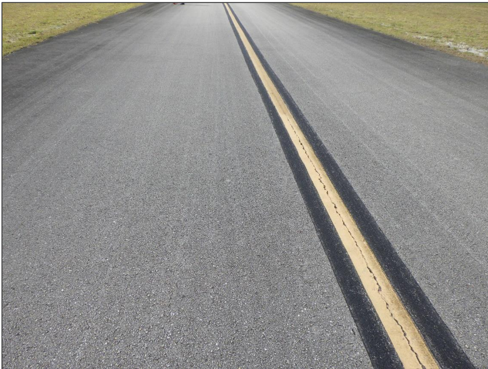
TW B, Section 205, Sample Unit 109 – Longitudinal and Transverse Cracking
