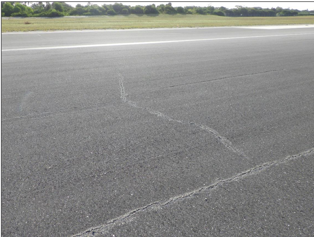
RW 16-34, Section 6215, Sample Unit 124 – Longitudinal and Transverse Cracking
