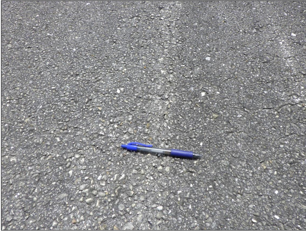
RW 4-22, Section 6305, Sample Unit 124 – Longitudinal and Transverse Cracking
