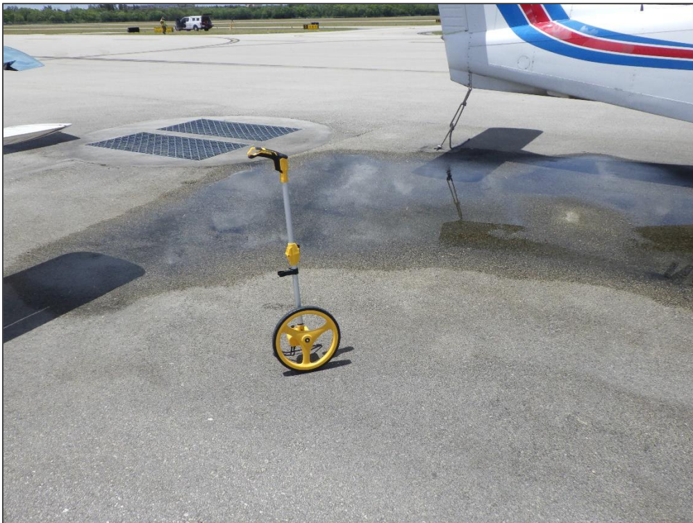
AP GA, Section 4120, Sample Unit 667 – Depression
