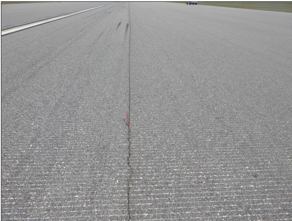
RW 9L-27R, Section 6210, Sample Unit 381 – Longitudinal and Transverse Cracking
