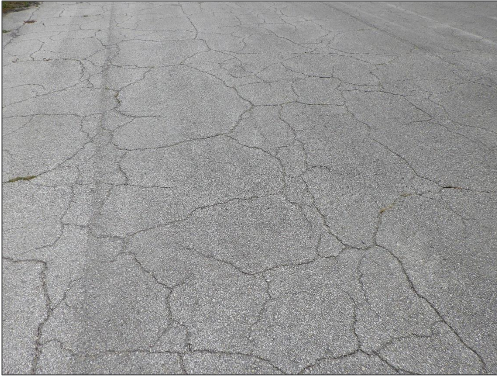
AP E, Section 4406, Sample Unit 810 – Block Cracking
