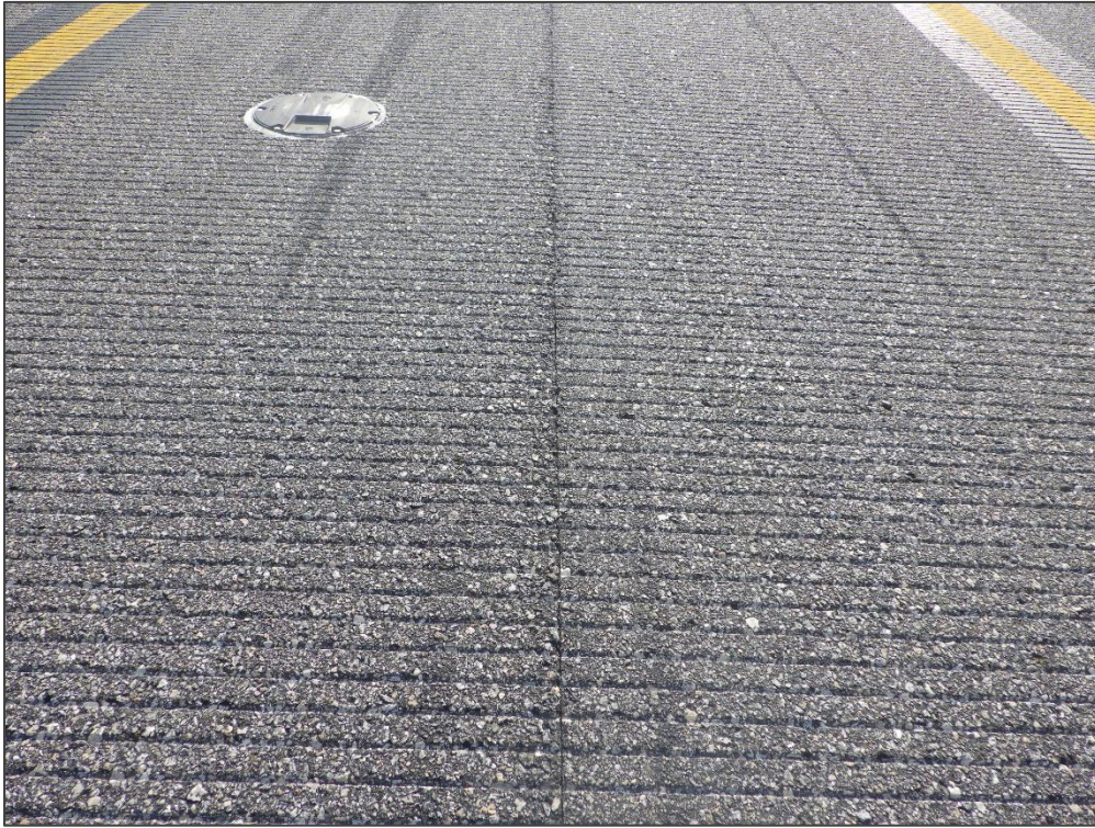
RW 9R-27L, Section 6105, Sample Unit 382 – Longitudinal & Transverse Cracking and Weathering
