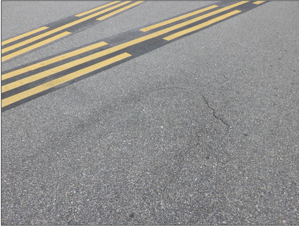
TW A, Section 105, Sample Unit 106 – Slippage Cracking
