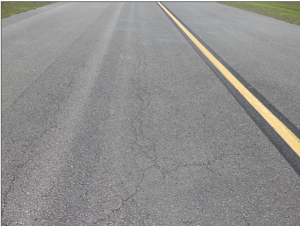
TW D, Section 410, Sample Unit 123 – Alligator Cracking and Longitudinal & Transverse Cracking
