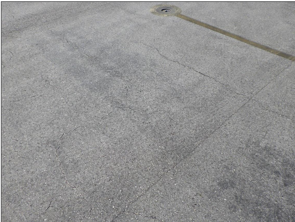
AP SW, Section 4710, Sample Unit 301 – Longitudinal & Transverse Cracking
