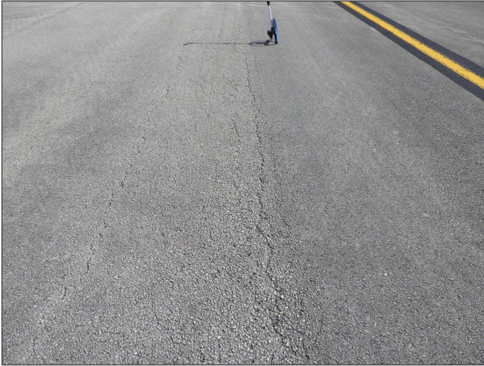
TW C, Section 330, Sample Unit 113 – Alligator Cracking and Longitudinal & Transverse Cracking
