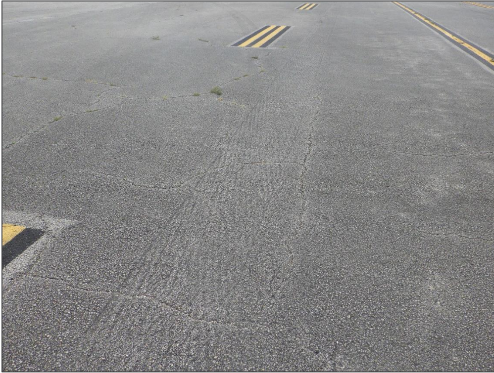
TW S, Section 510, Sample Unit 106 – Block Cracking and Swelling
