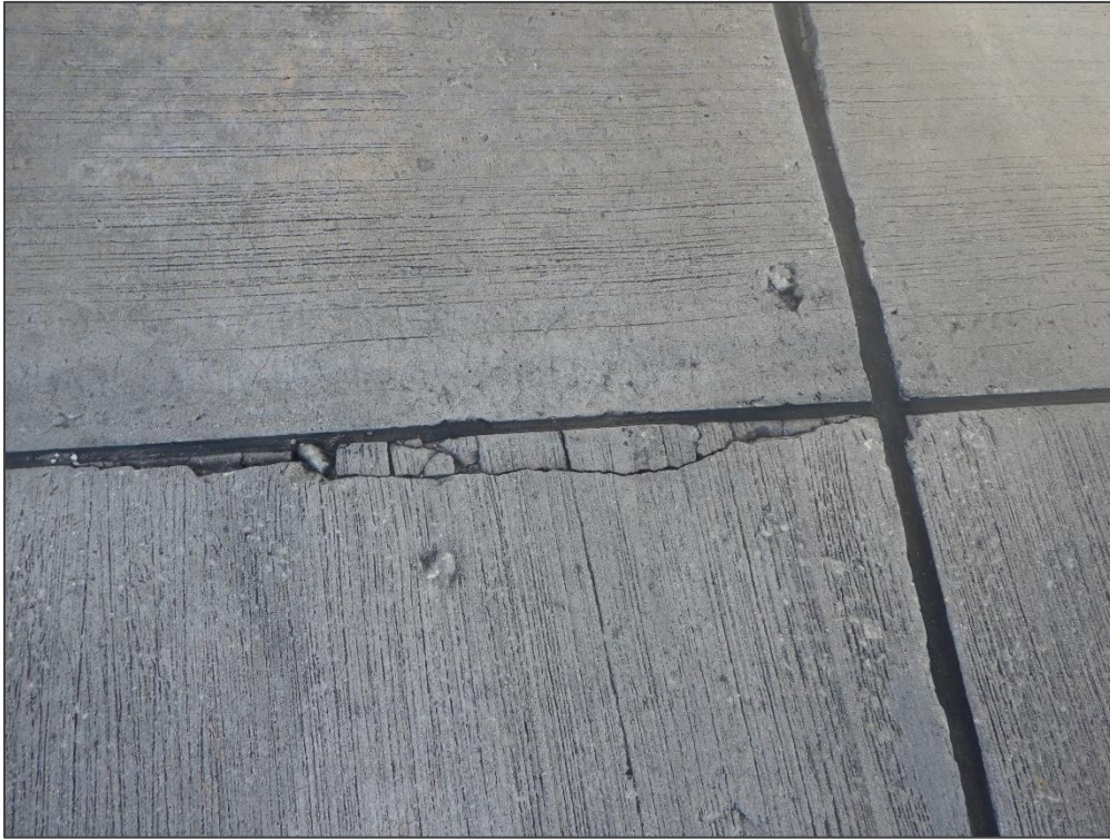
AP TERM, Section 4205, Sample Unit 202 – Joint Spall
