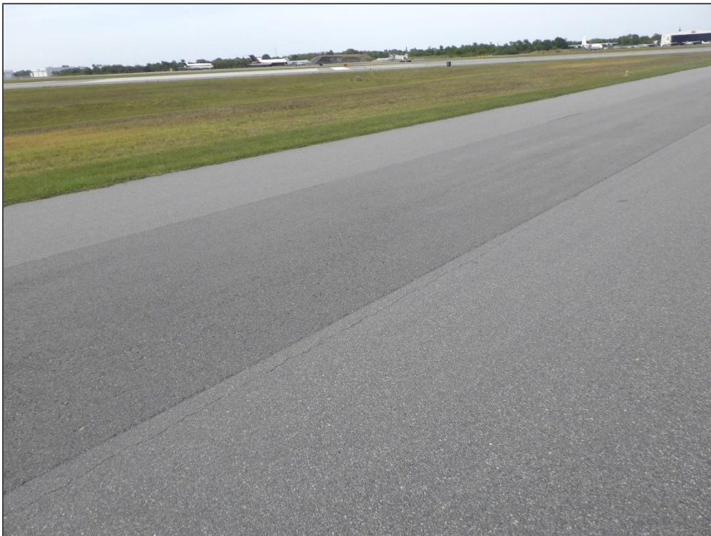
RW 5-23, Section 6305, Sample Unit 154 – Patching
