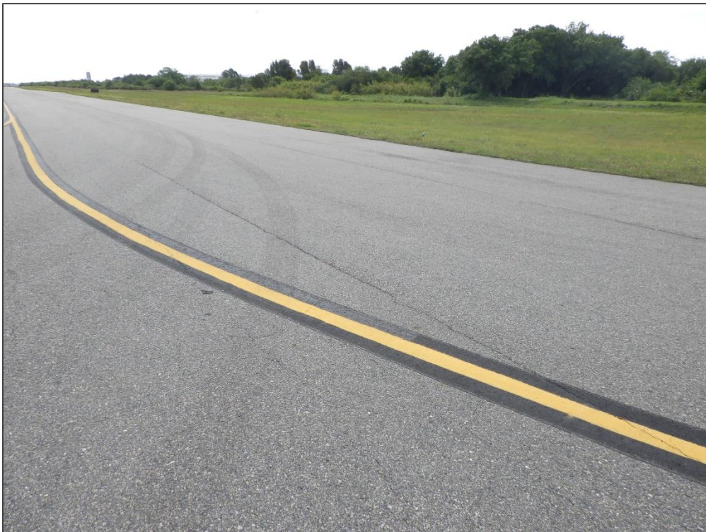
TW A, Section 120, Sample Unit 101 – Longitudinal & Transverse Cracking
