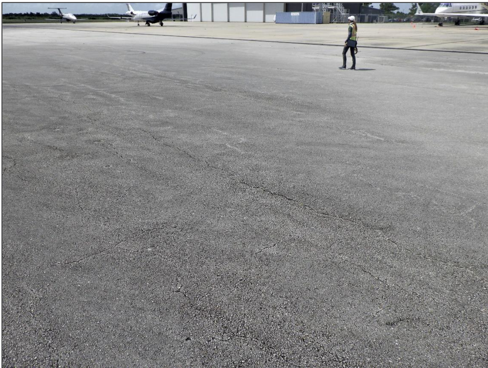
AP N, Section 4120, Sample Unit 402 – Longitudinal & Transverse Cracking and Swelling
