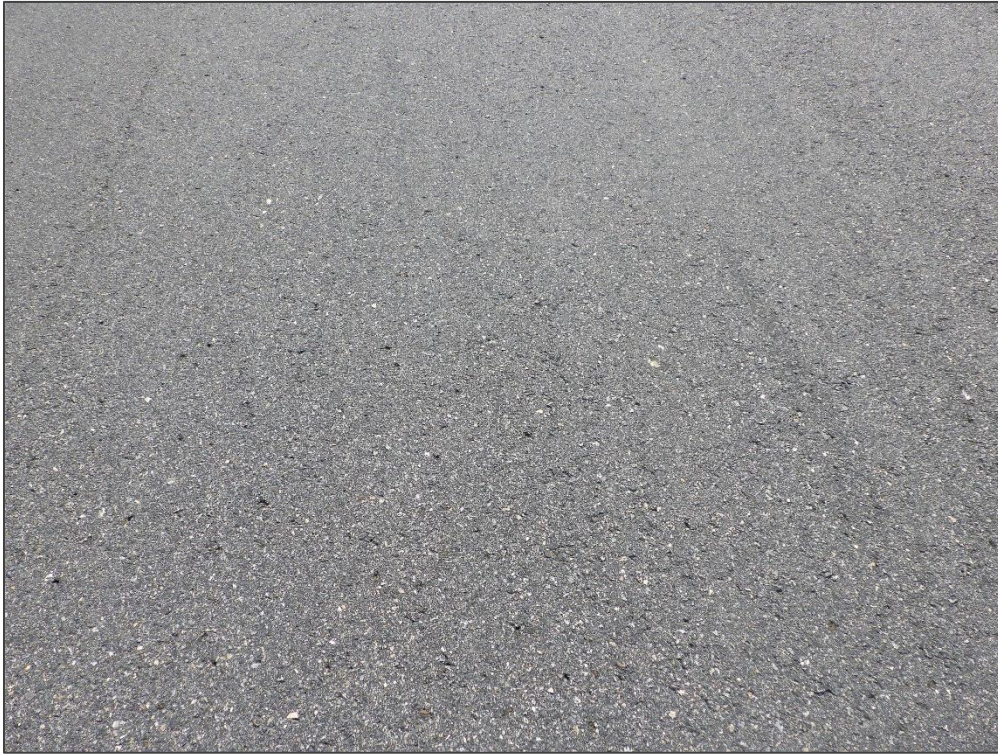
RW 5-23, Section 6305, Sample Unit 108 – Raveling
