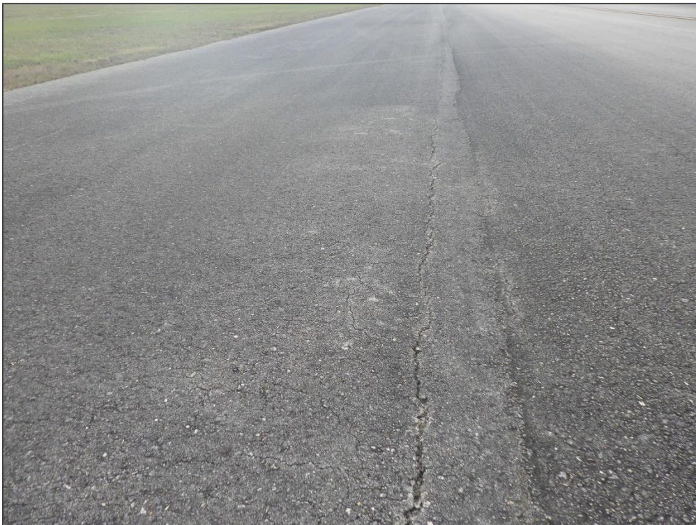
TW K, Section 1135, Sample Unit 187 – Longitudinal & Transverse Cracking, Swelling, and Weathering
