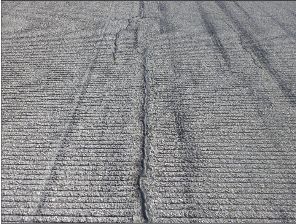
RW 7-25, Section 6105, Sample Unit 127 - Longitudinal & Transverse Cracking
