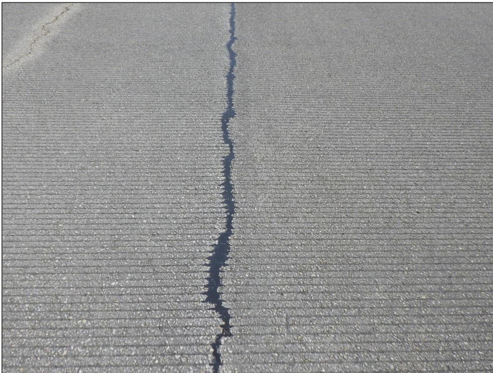
RW 7-25, Section 6105, Sample Unit 174 - Longitudinal & Transverse Cracking
