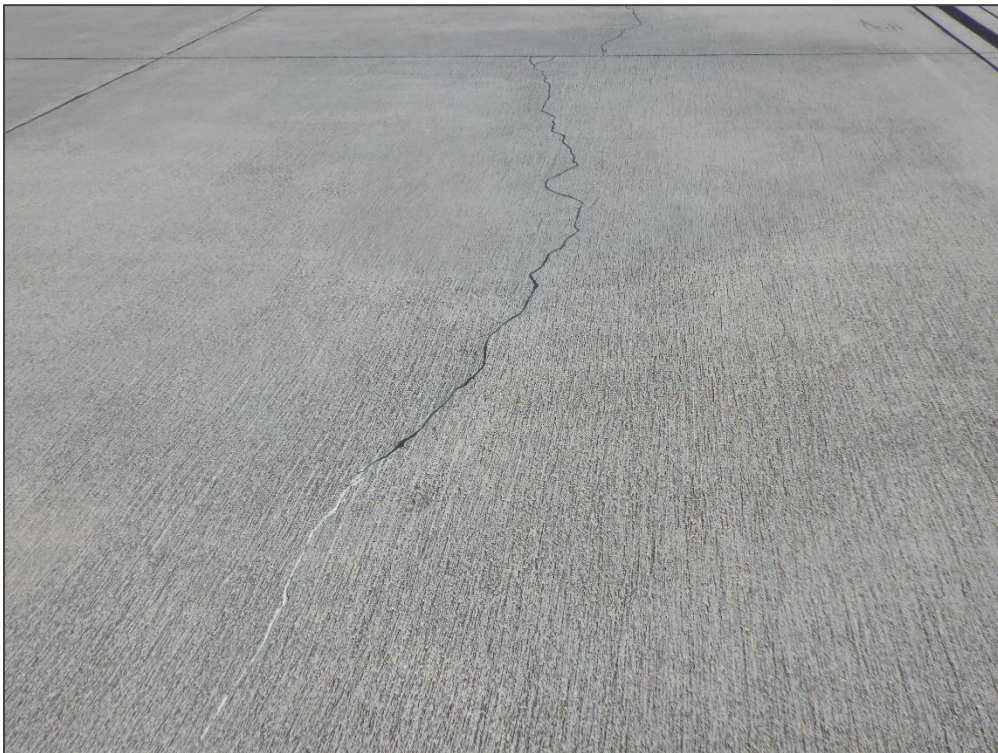
AP TERM, Section 4220, Sample Unit 307 - Linear Cracking
