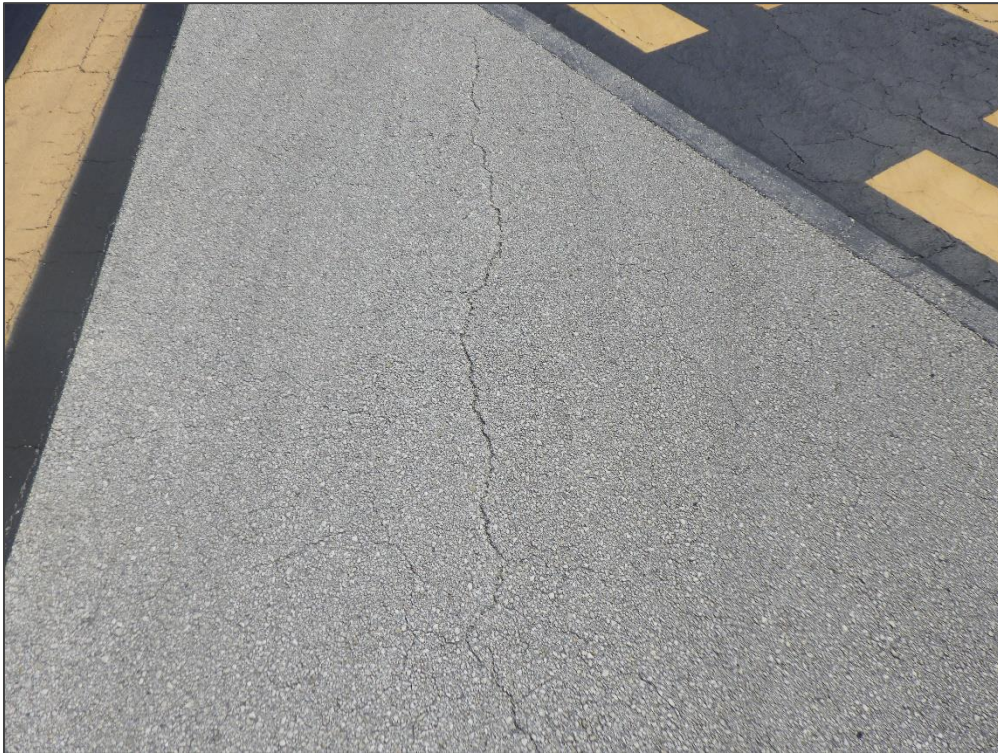
TW D, Section 305, Sample Unit 302 - Longitudinal & Transverse Cracking
