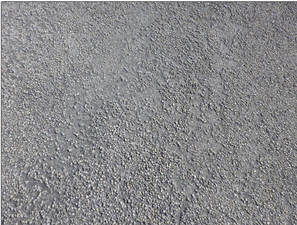
AP JET CTR, Section 4305, Sample Unit 151 - Raveling
