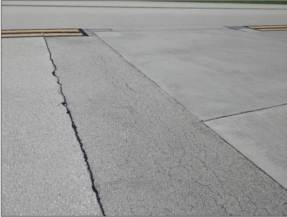
AP TERM, Section 4210, Sample Unit 304 - Patching
