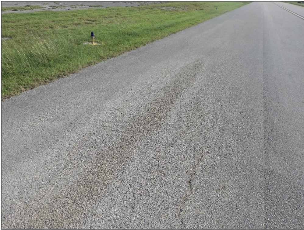
TW A, Section 105, Sample Unit 111 - Longitudinal & Transverse Cracking and Raveling
