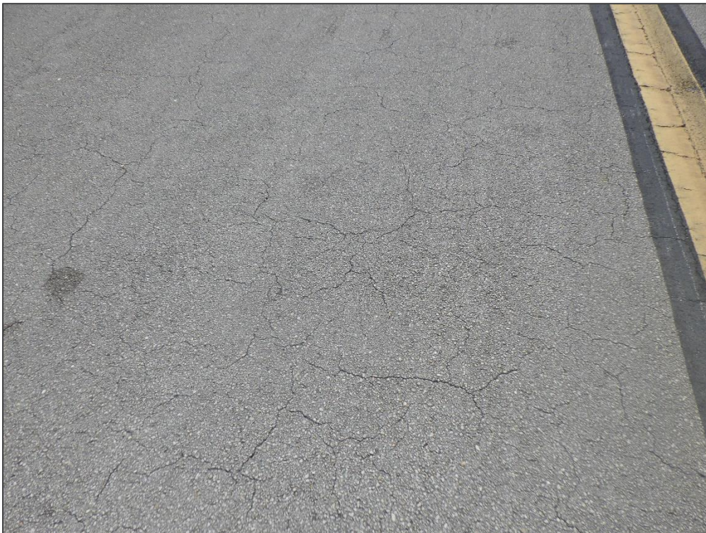
TW A, Section 115, Sample Unit 402 - Block Cracking
