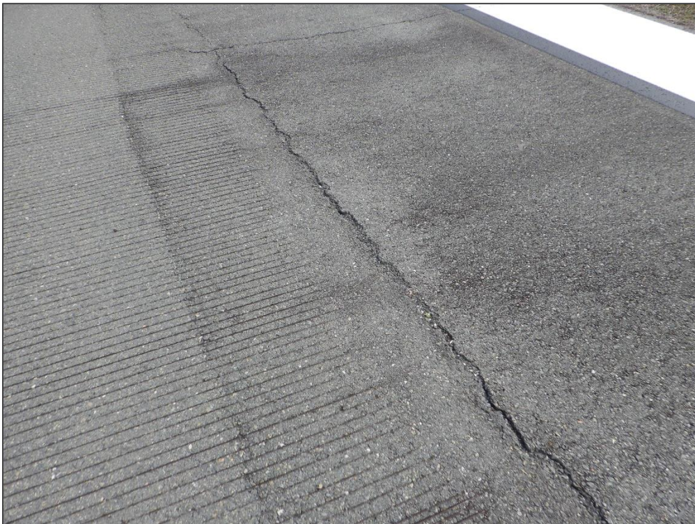
RW 18-36, Section 6110, Sample Unit 564 – Longitudinal & Transverse Cracking
