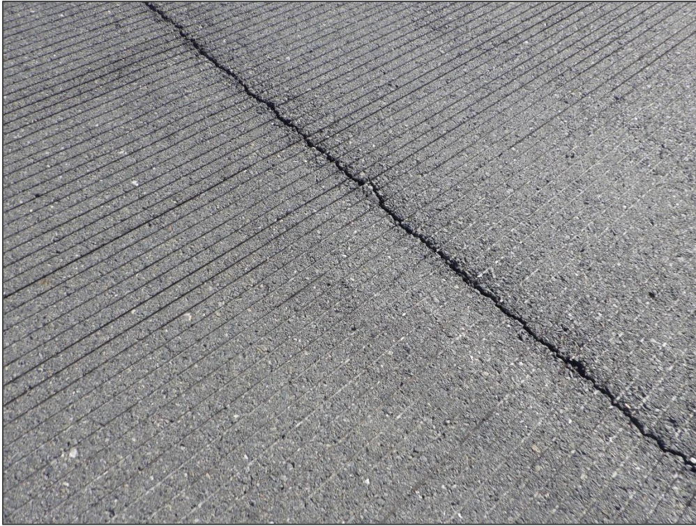
RW 18-36, Section 6105, Sample Unit 333 – Longitudinal & Transverse Cracking
