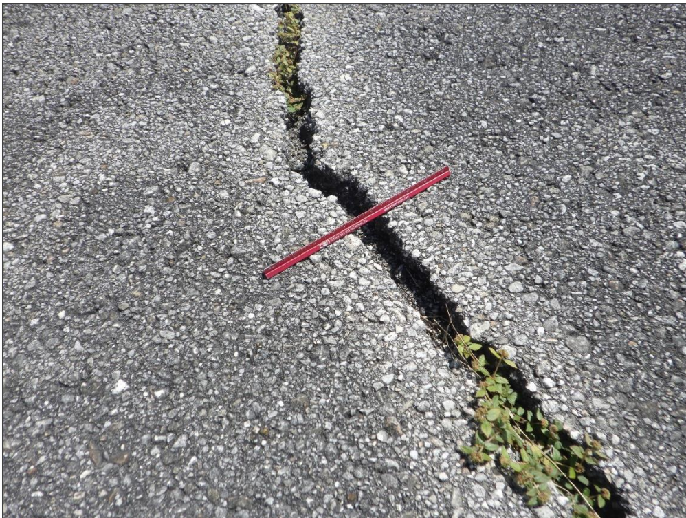
TW B, Section 105, Sample Unit 102 – Longitudinal & Transverse Cracking
