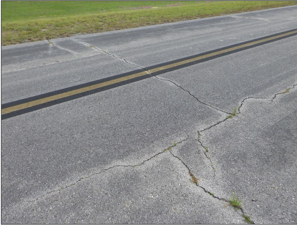
TW B, Section 105, Sample Unit 107 – Longitudinal & Transverse Cracking
