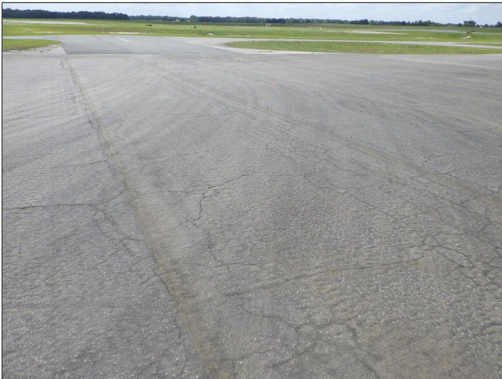
AP N, Section 4210, Sample Unit 700 – Block Cracking
