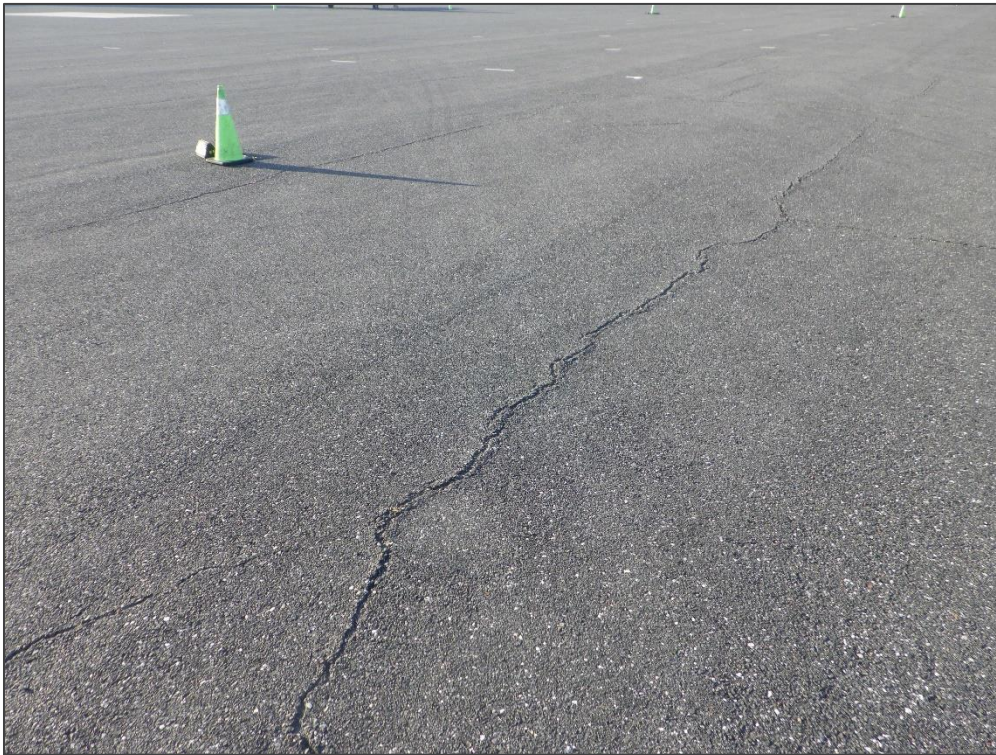
AP CENTER, Section 4105, Sample Unit 104 – Longitudinal & Transverse Cracking and Swelling
