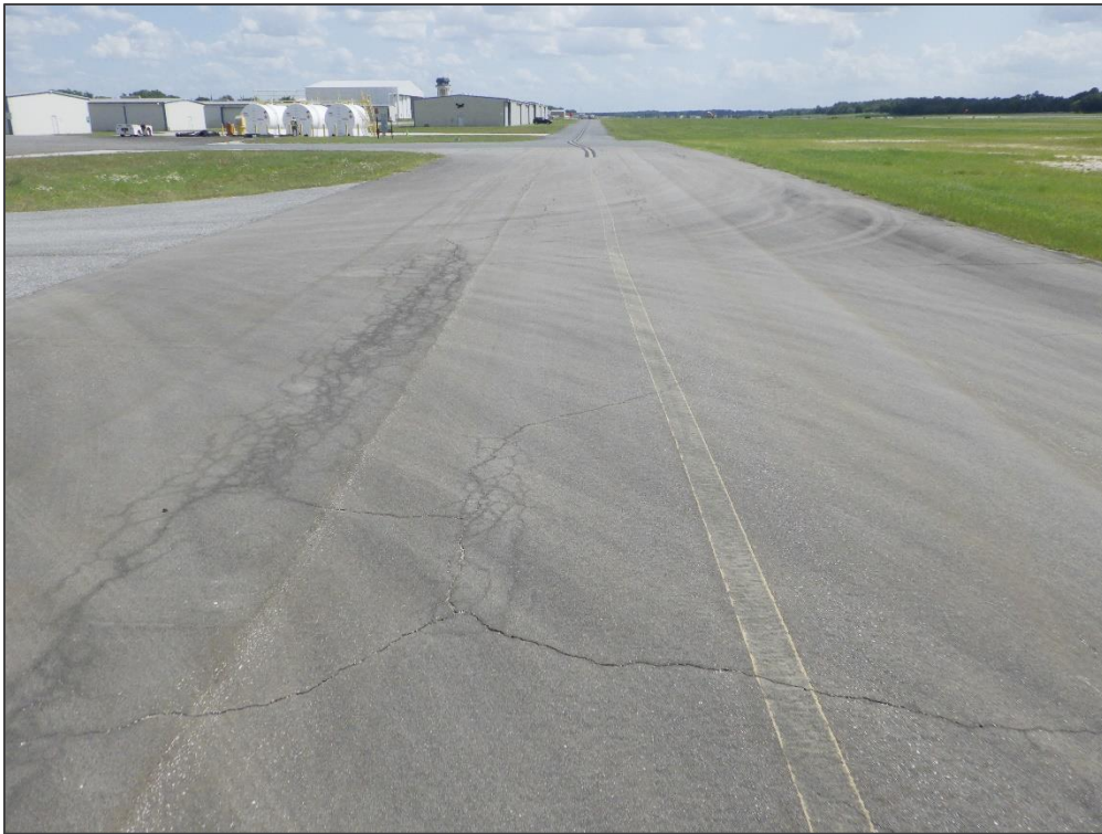
TW AP N, Section 595, Sample Unit 301 – Alligator Cracking and Longitudinal & Transverse Cracking
