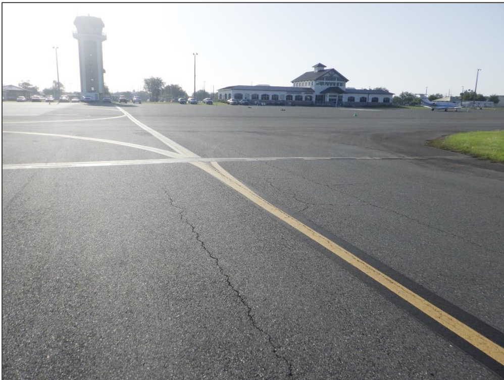
TW A5, Section 520, Sample Unit 401 – Longitudinal & Transverse Cracking
