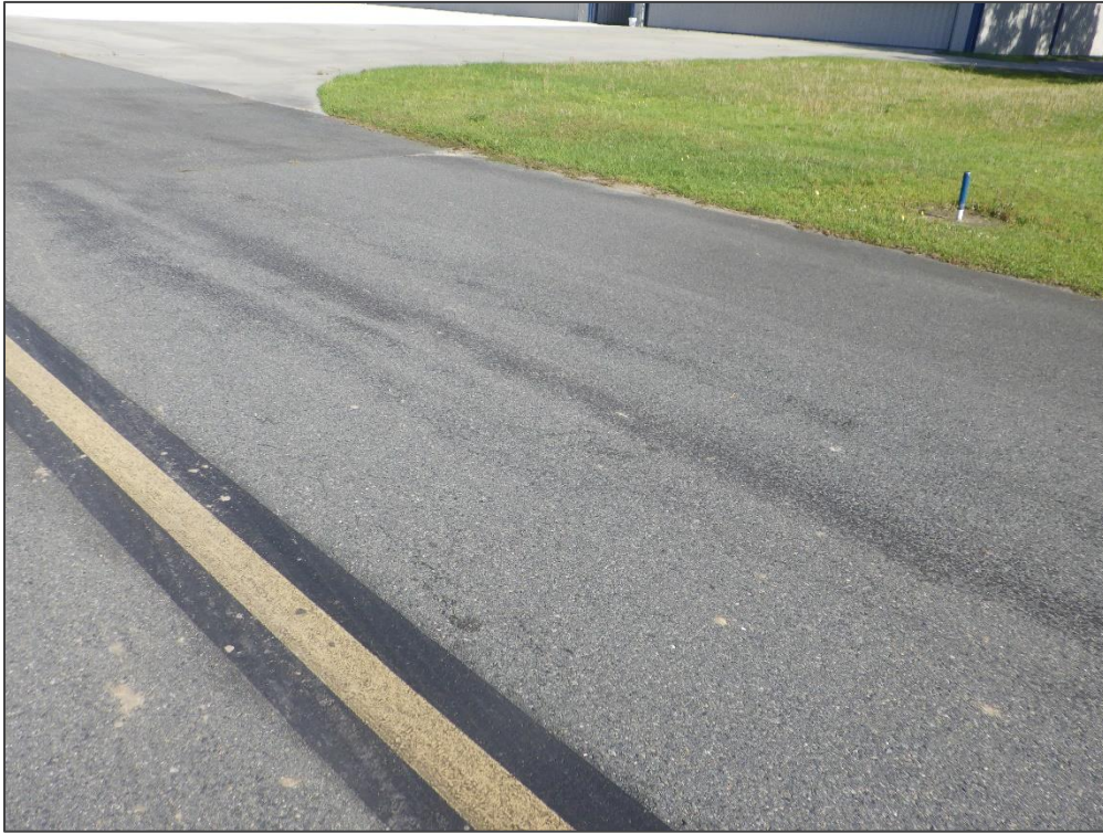
TW A9, Section 550, Sample Unit 105 – Bleeding
