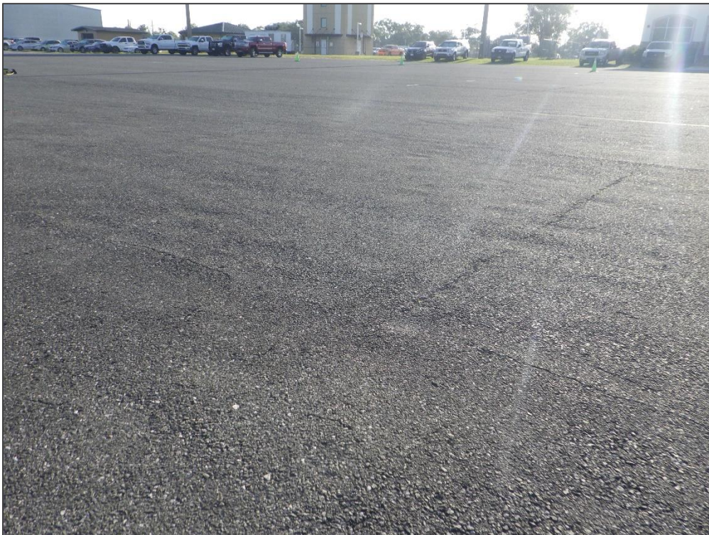
AP CENTER, Section 4105, Sample Unit 303 – Longitudinal & Transverse Cracking and Swelling
