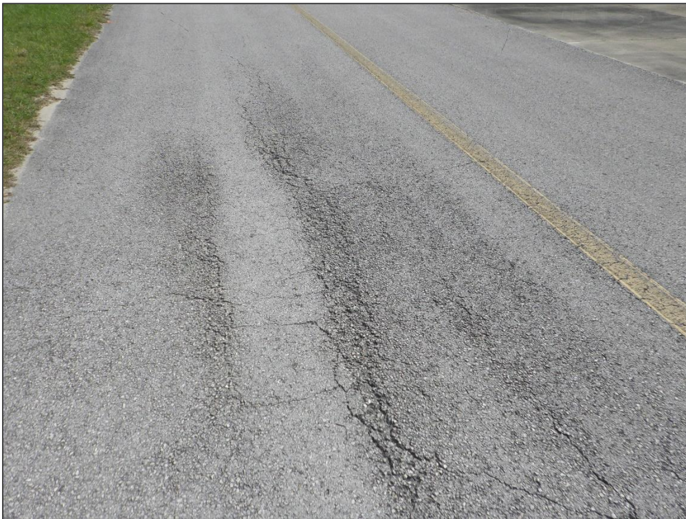
TL T-HANG, Section 3580, Sample Unit 902 – Alligator Cracking and Raveling
