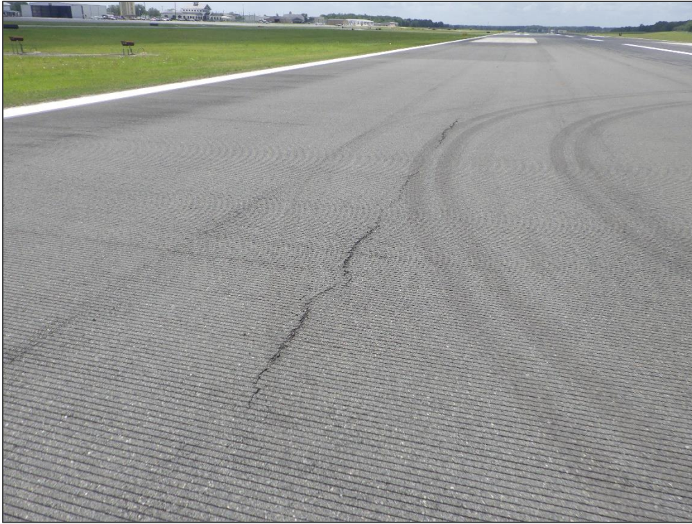
RW 18-36, Section 6110, Sample Unit 606 – Longitudinal & Transverse Cracking
