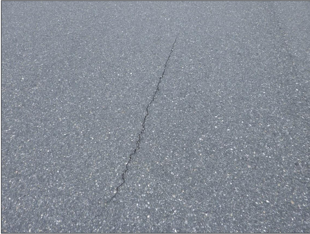
RW 8-26, Section 6205, Sample Unit 104 – Longitudinal & Transverse Cracking
