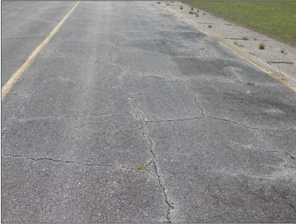
TW E, Section 505, Sample Unit 107 – Block Cracking
