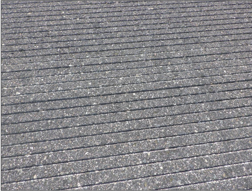
RW 9-27, Section 6105, Sample Unit 118 – Weathering
