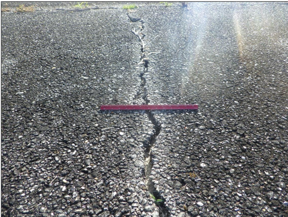
TW F, Section 605, Sample Unit 108 – Longitudinal & Transverse Cracking and Raveling
