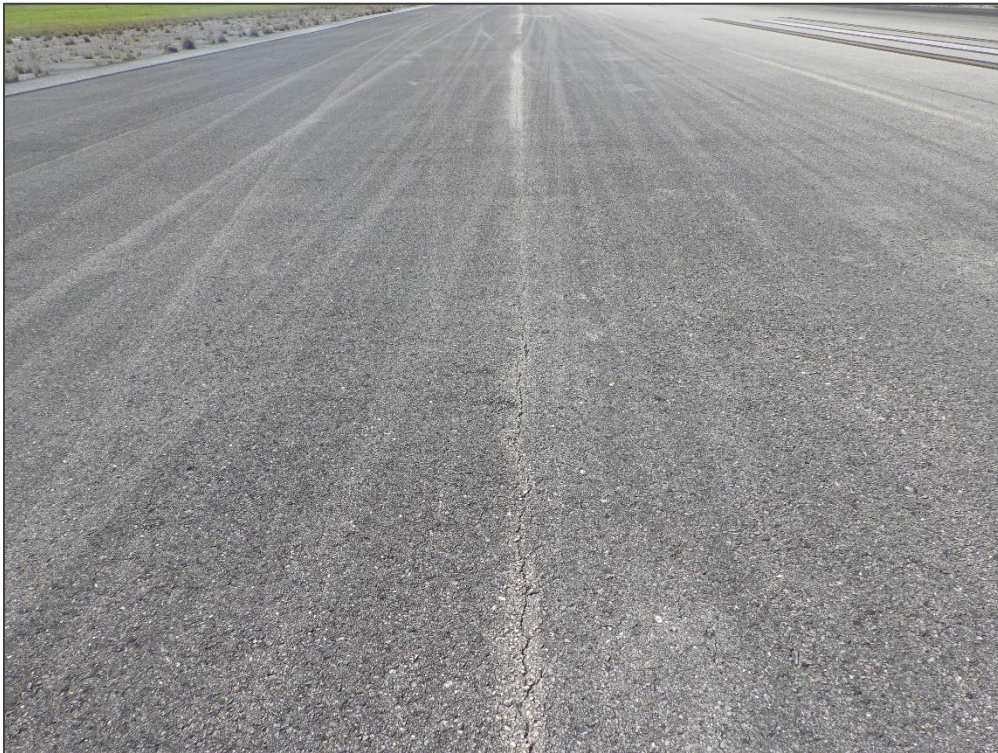
RW 17-35, Section 6205, Sample Unit 139 – Longitudinal & Transverse Cracking
