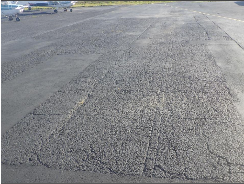
AP FBO, Section 4110, Sample Unit 111 – Alligator Cracking, Block Cracking, Patching, and Raveling
