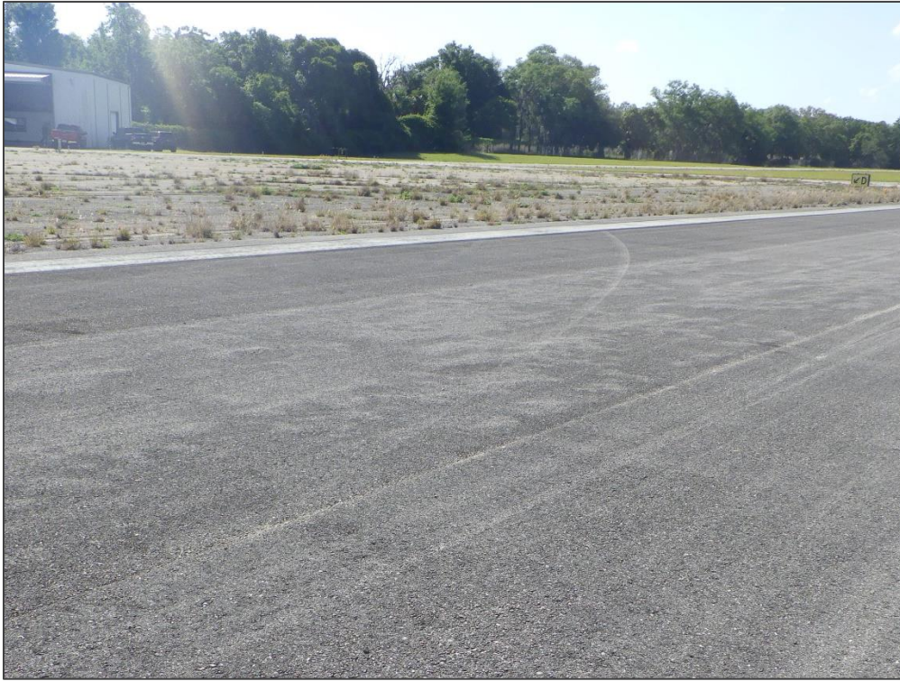
RW 17-35, Section 6205, Sample Unit 126 – Swelling
