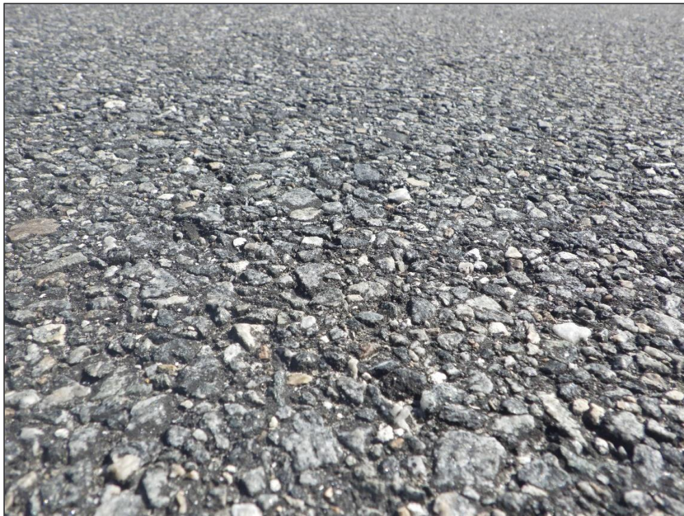
TW C, Section 305, Sample Unit 106 – Weathering
