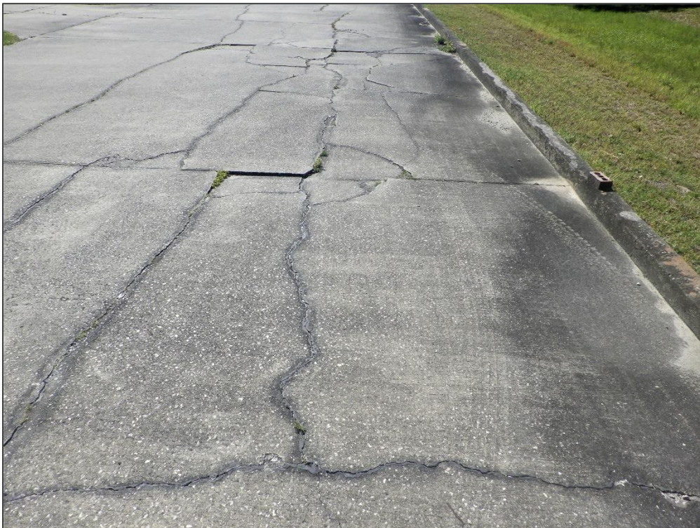
TL SW, Section 2004, Sample Unit 602 – Shattered Slab
