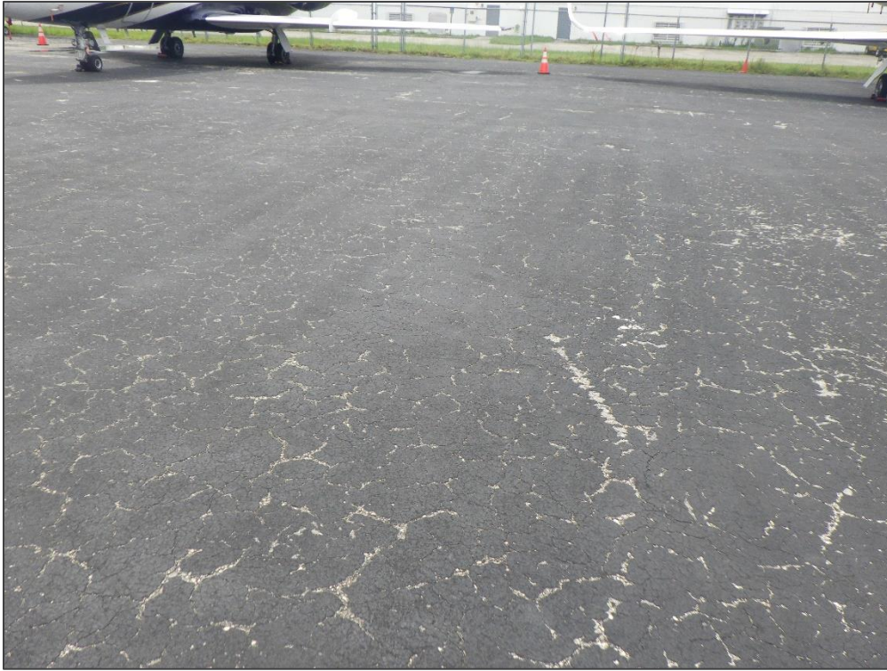
AP E, Section 4210, Sample Unit 457 – Raveling
