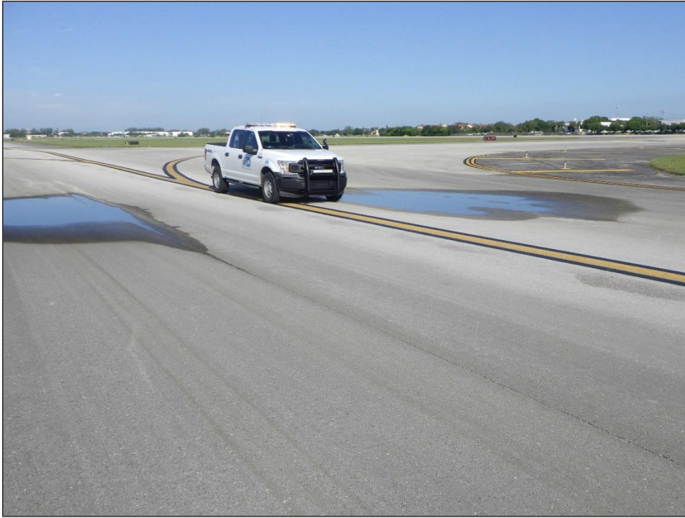
TW N, Section 1422, Sample Unit 168 – Vicinity
