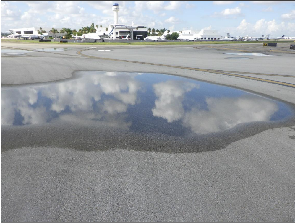
TW C, Section 315, Sample Unit 102 – Depression
