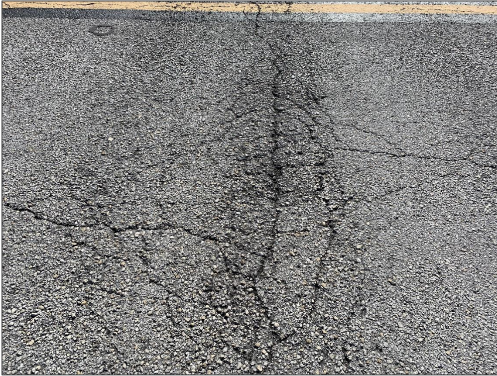
TW A1, Section 112, Sample Unit 109 – Alligator Cracking
