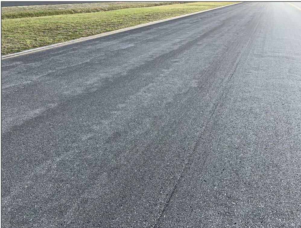
TW A, Section 125, Sample Unit 166 – Swelling
