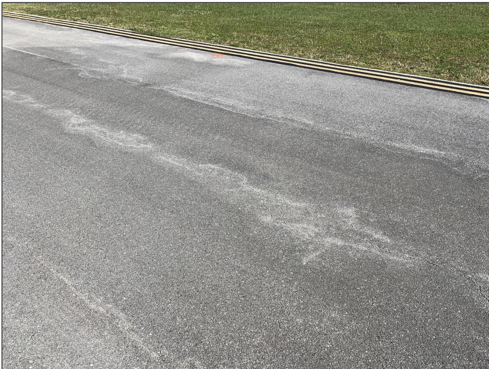
TW B, Section 103, Sample Unit 190 – Swelling
