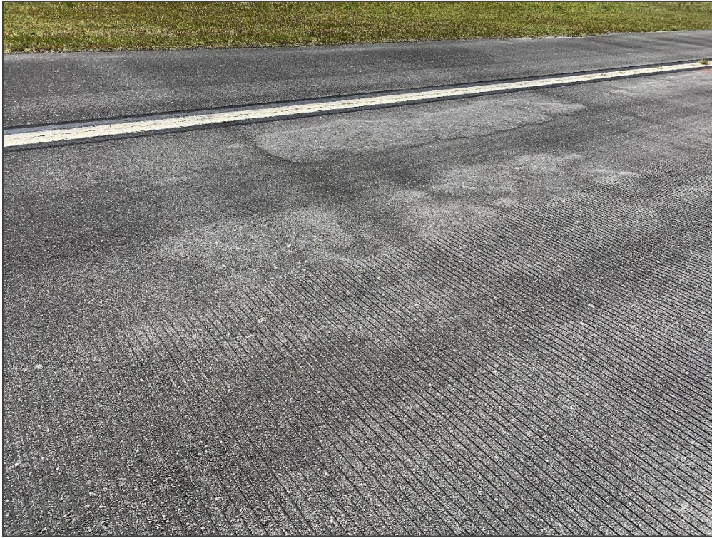
RW 13-31, Section 6205, Sample Unit 185 – Swelling
