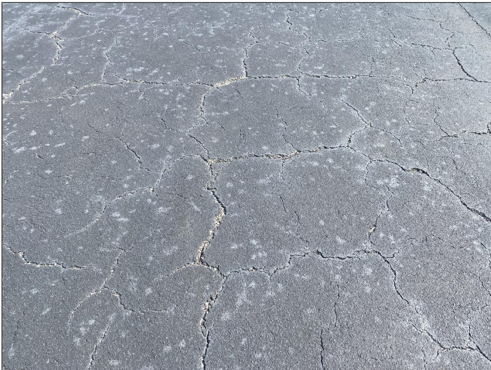
AP W, Section 4610, Sample Unit 424 – Block Cracking
