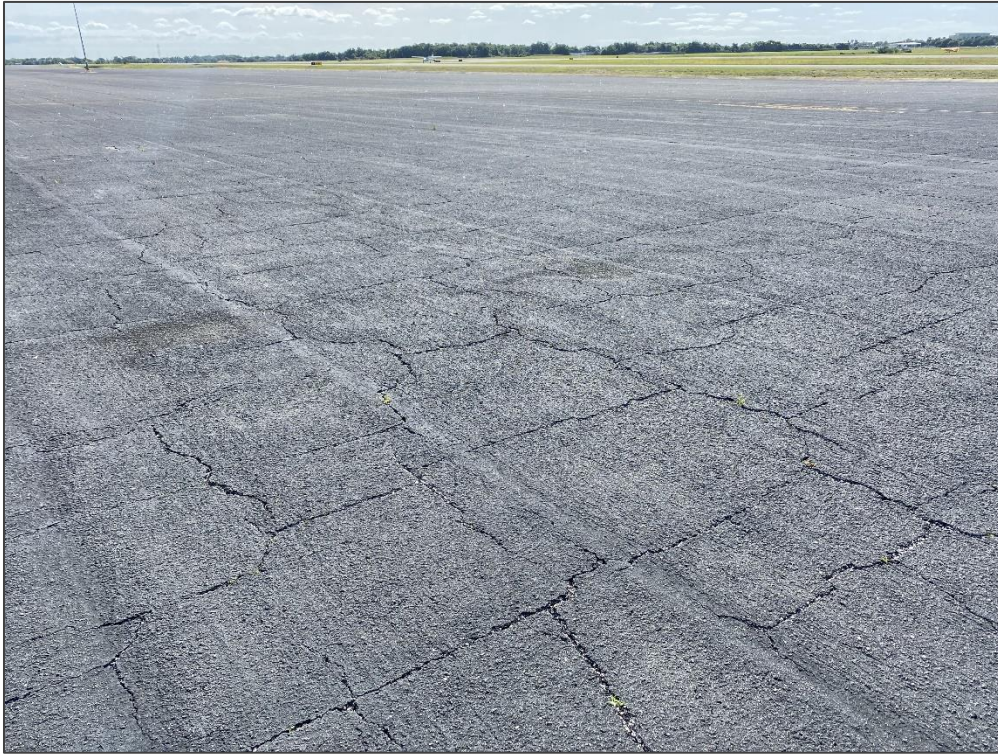
AP E, Section 4205, Sample Unit 251– Block Cracking
