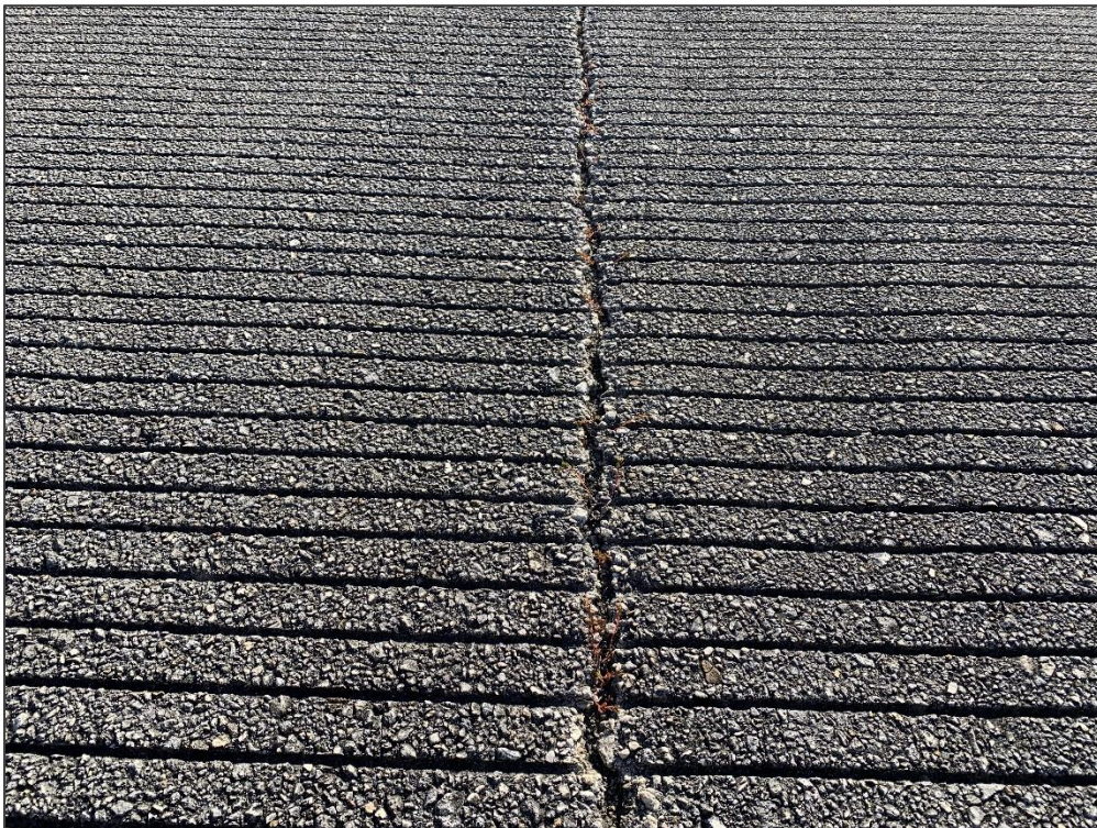
RW 7-25, Section 6105, Sample Unit 412 – Longitudinal & Transverse Cracking
