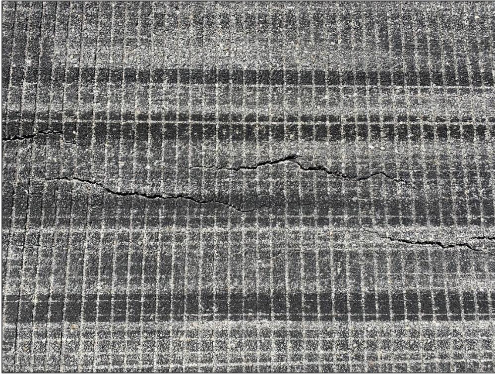
RW 7-25, Section 6105, Sample Unit 328 – Alligator Cracking
