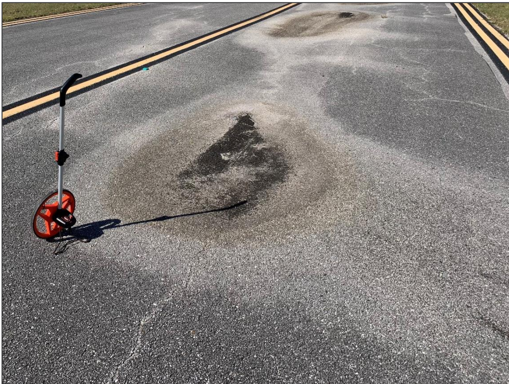
TW E3, Section 420, Sample Unit 405 – Depression
