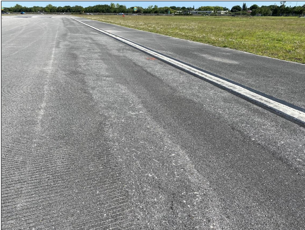
RW 13-31, Section 6205, Sample Unit 115 – Swelling
