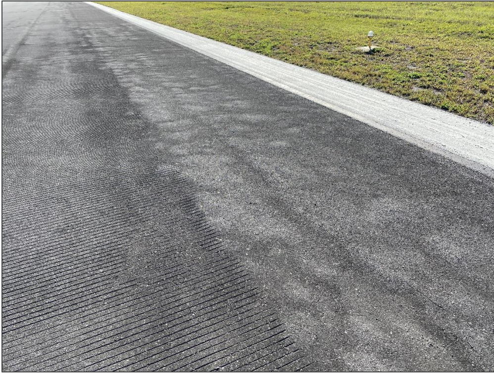
RW 7-25, Section 6110, Sample Unit 568 – Swelling
