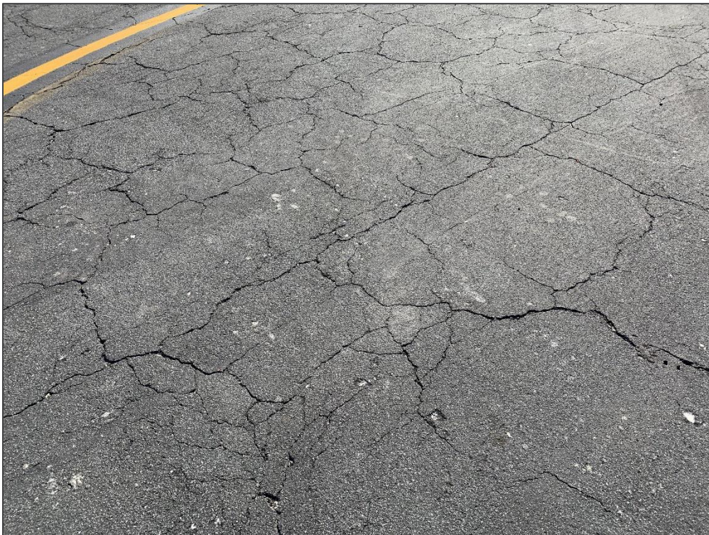
AP N, Section 4125, Sample Unit 106 – Block Cracking
