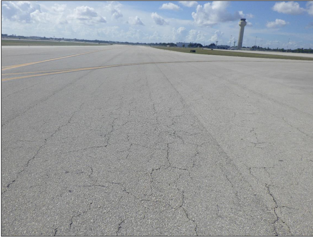
TW B, Section 220, Sample Unit 164 – Vicinity
