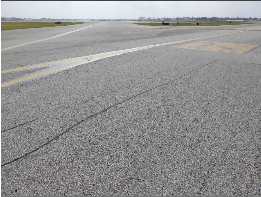
TW F, Section 605, Sample Unit 110 – Vicinity
