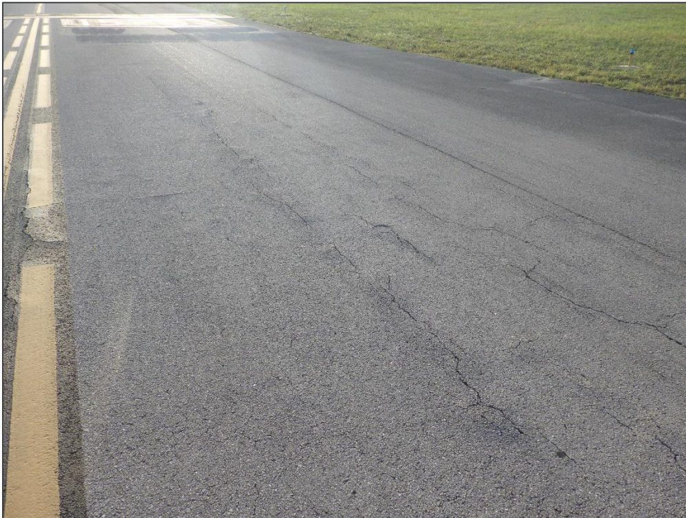
TW D, Section 120, Sample Unit 152 – Longitudinal & Transverse Cracking and Swelling
