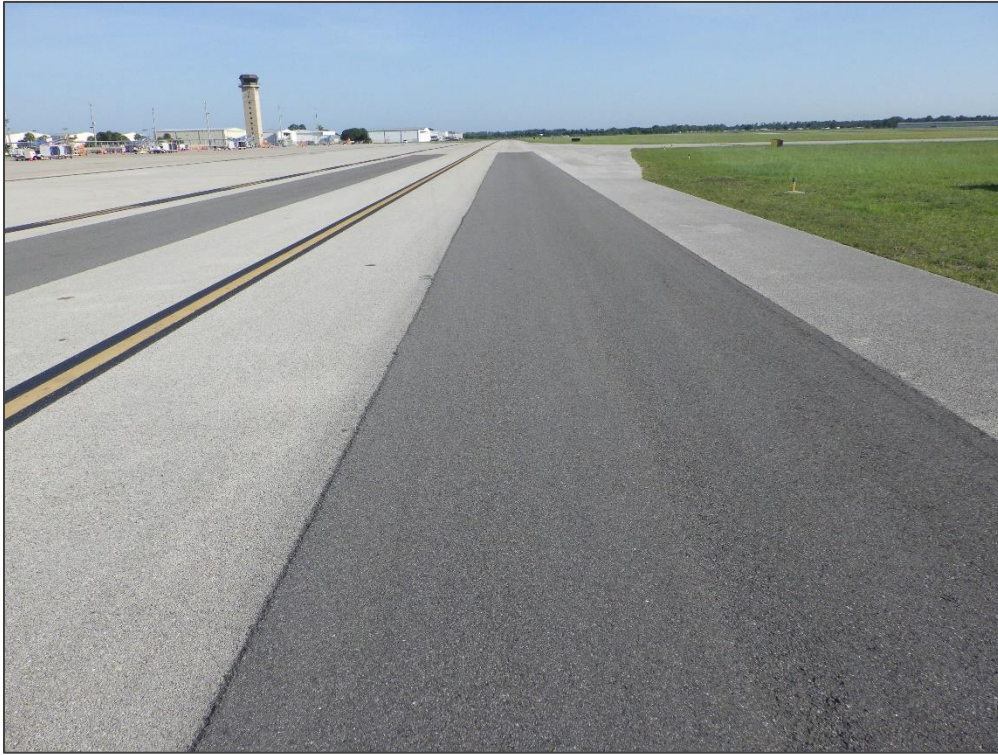
TW D, Section 115, Sample Unit 122 – Patching
