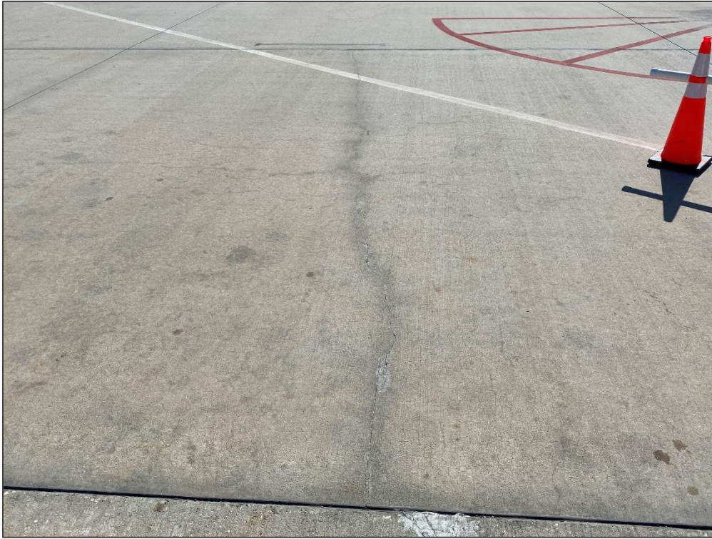
AP TERM, Section 4205, Sample Unit 200 – Linear Cracking
