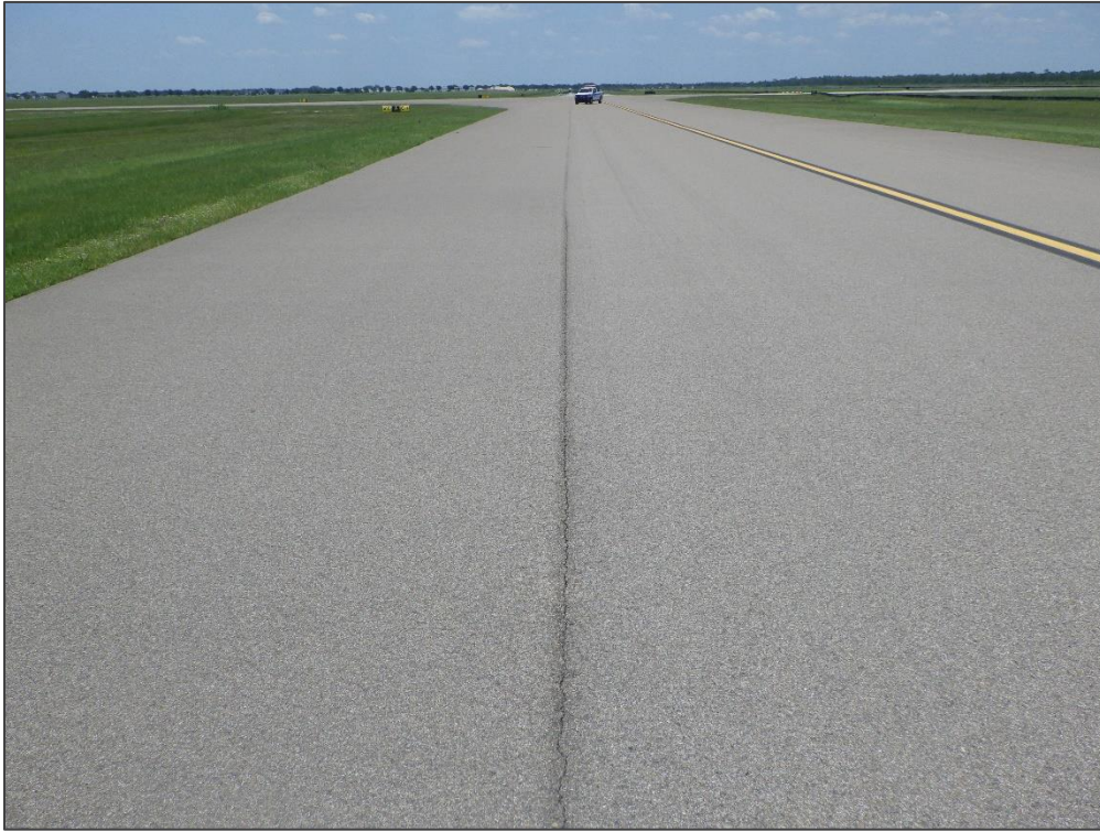
TW A, Section 320, Sample Unit 257 - Longitudinal & Transverse Cracking
