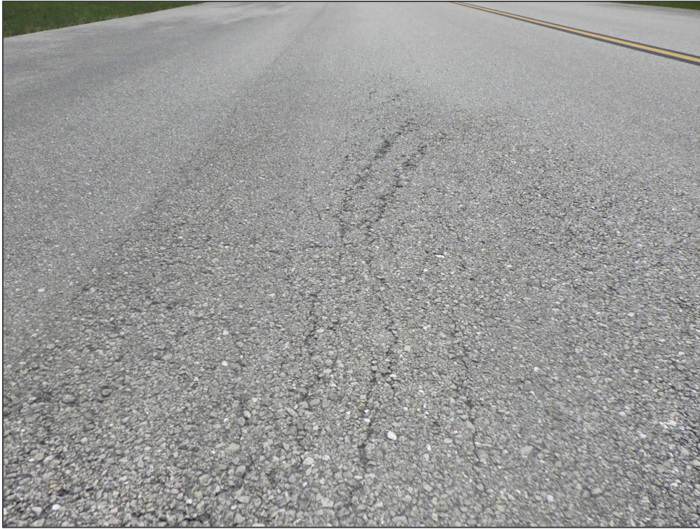
TW A, Section 330, Sample Unit 211 – Alligator Cracking
