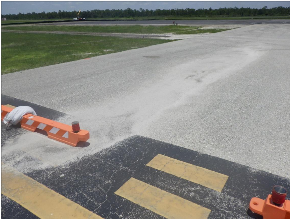
TW A, Section 330, Sample Unit 203 - Rutting
