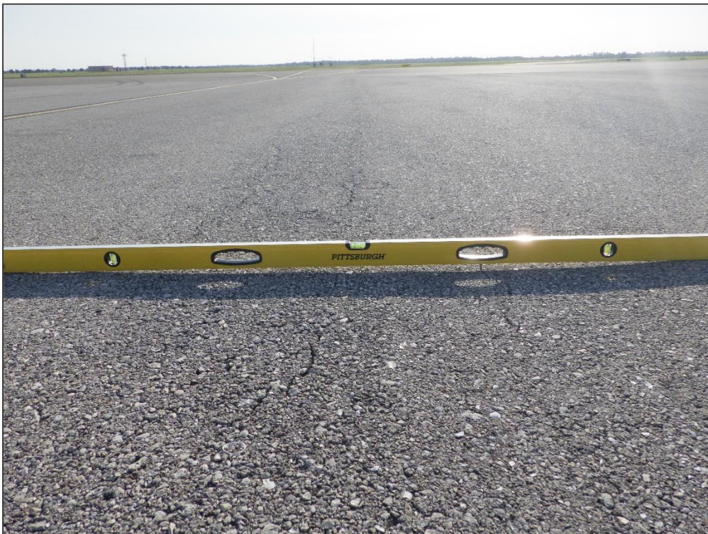
TW C, Section 305, Sample Unit 303 – Rutting
