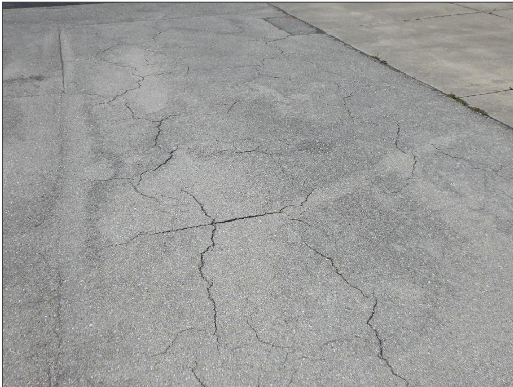
AP S, Section 4105, Sample Unit 405 – Block Cracking
