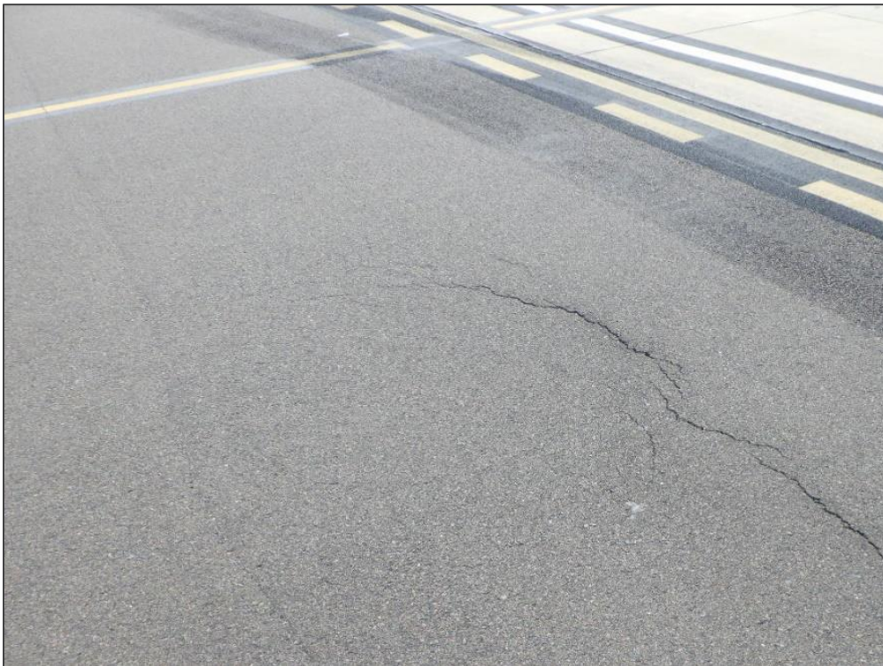
AP MAIN, Section 4110, Sample Unit 603 – Slippage Cracking
