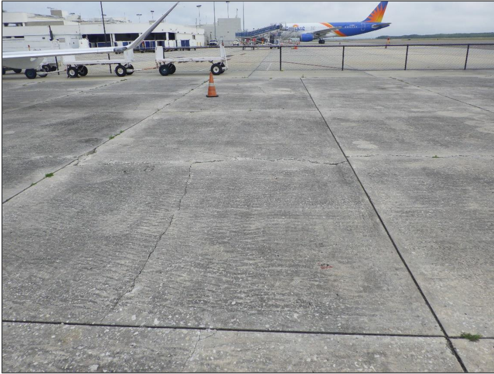
AP MAIN, Section 4175, Sample Unit 603 – Shattered Slab
