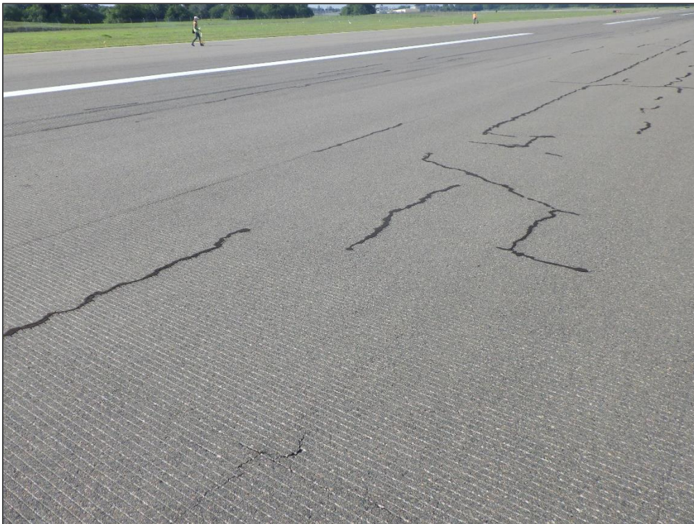
RW 4-22, Section 6205, Sample Unit 373 – Longitudinal & Transverse Cracking
