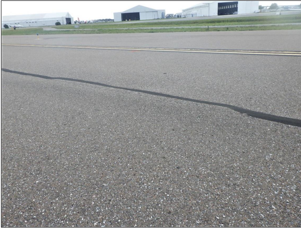
TW A, Section 130, Sample Unit 343 – Longitudinal & Transverse Cracking and Swelling
