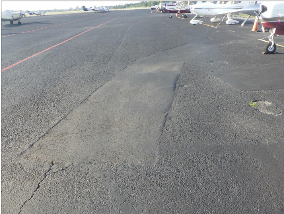
AP MAIN, Section 4180, Sample Unit 404 – Patching
