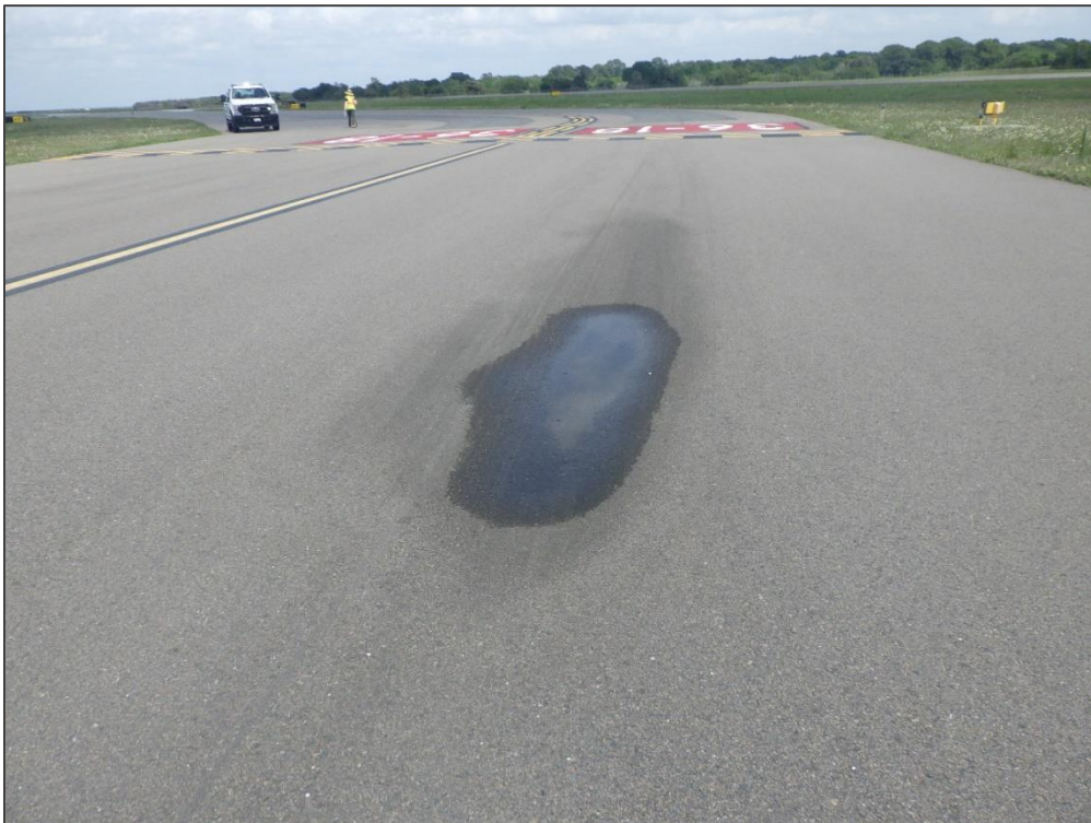
TW G, Section 1315, Sample Unit 101 – Rutting
