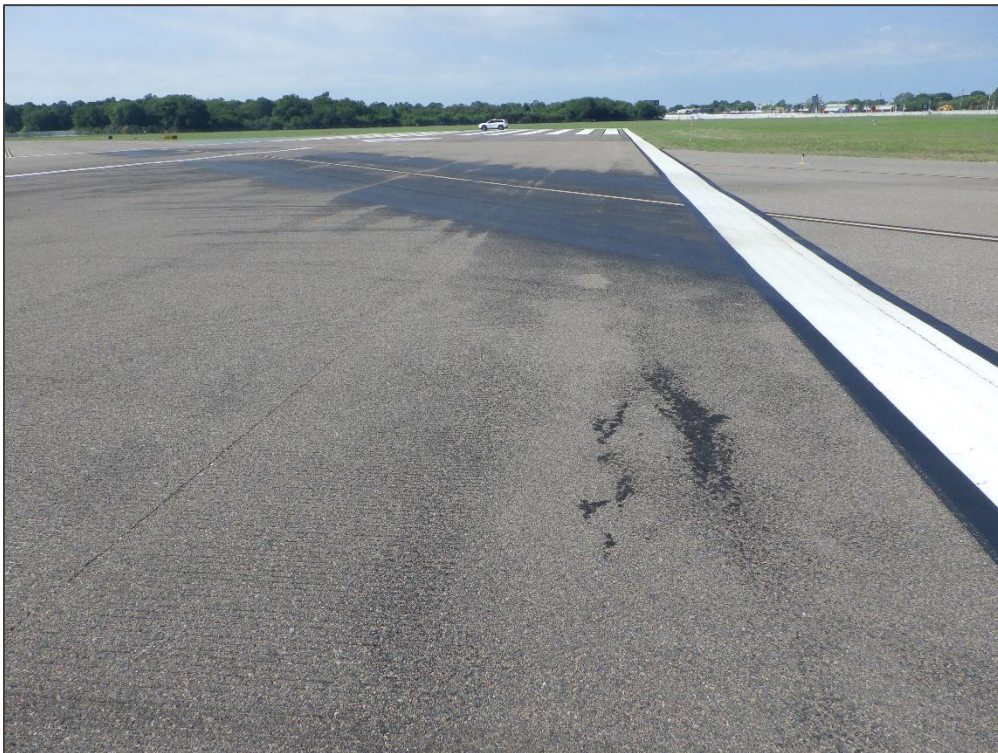
RW 4-22, Section 6230, Sample Unit 210 – Bleeding
