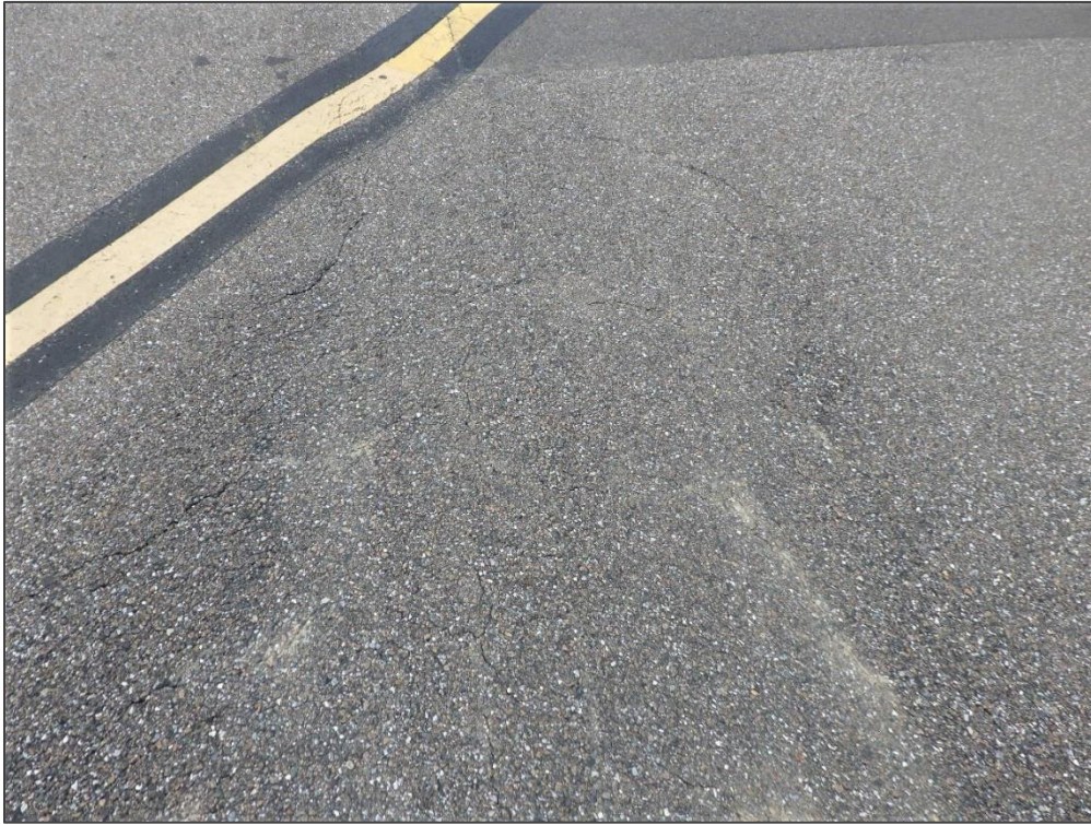
TW A, Section 115, Sample Unit 114 – Slippage Cracking
