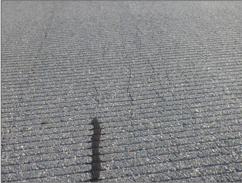
RW 4-22, Section 6205, Sample Unit 308 – Alligator Cracking
