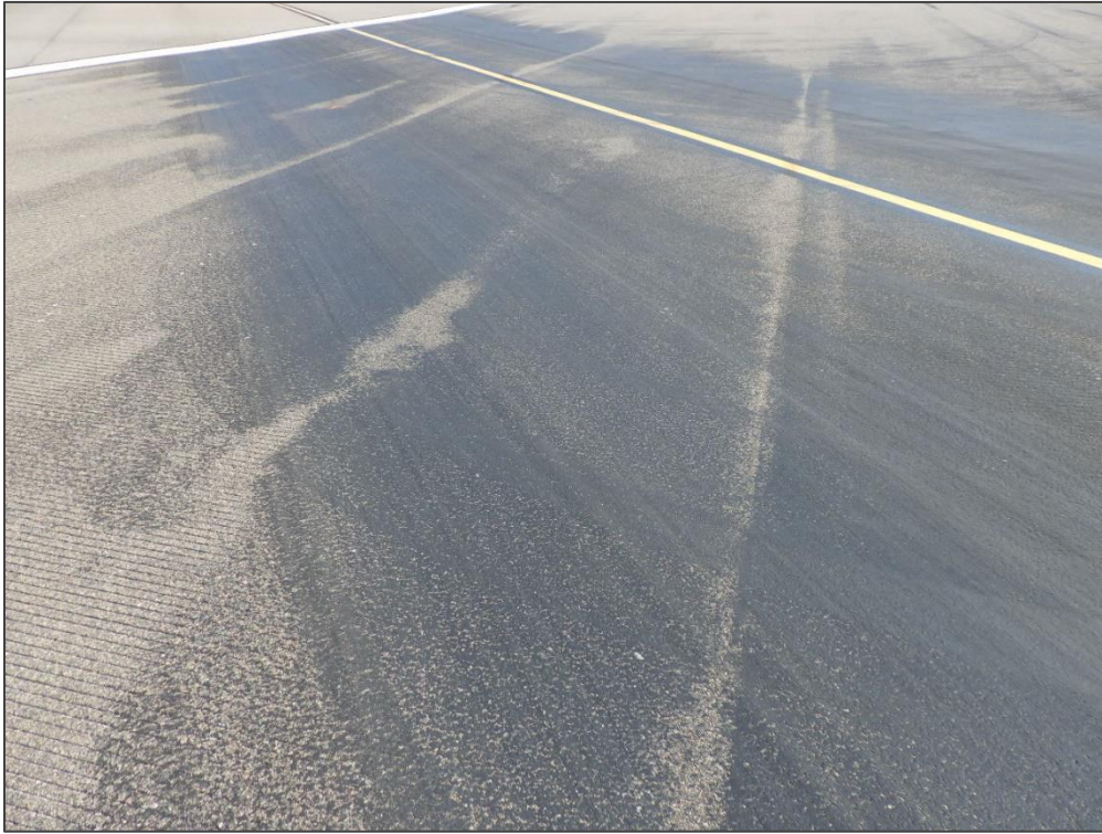
RW 4-22, Section 6225, Sample Unit 412 – Bleeding and Rutting
