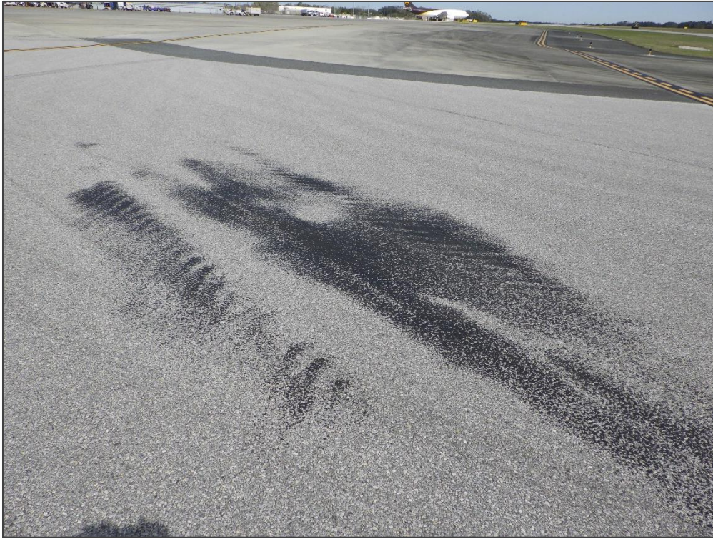
TW A7, Section 215, Sample Unit 601 – Bleeding
