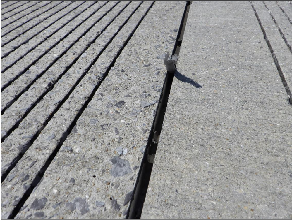
RW 17-35, Section 6105, Sample Unit 301 – Joint Seal Damage
