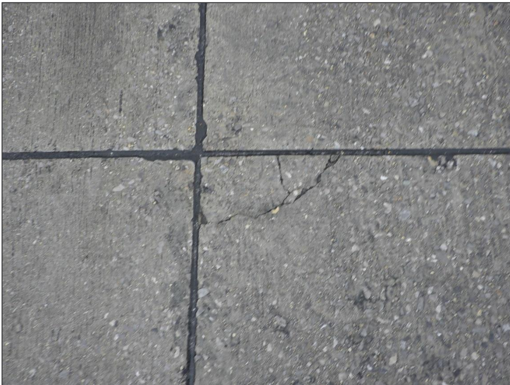
AP TERM, Section 4205, Sample Unit 211 – Corner Spall
