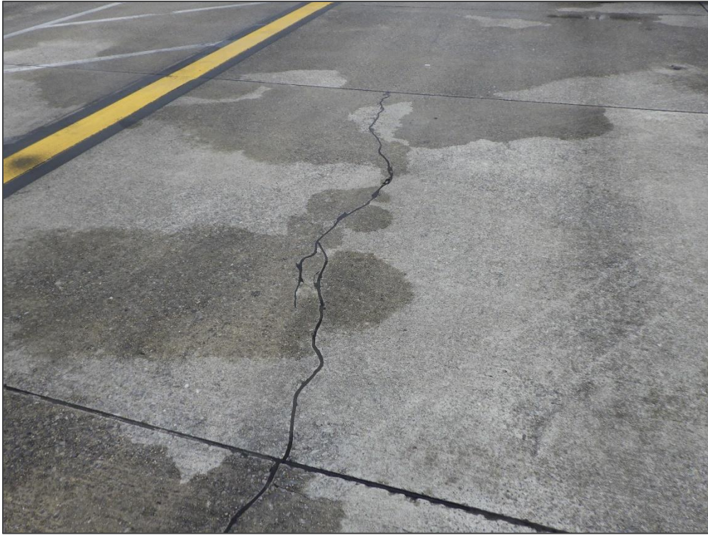
AP TERM, Section 4210, Sample Unit 803 – Linear Cracking
