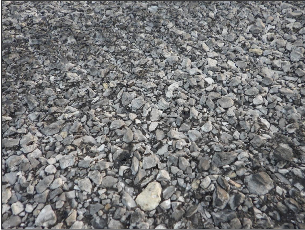
RW 8-26, Section 6215, Sample Unit 327 – Raveling
