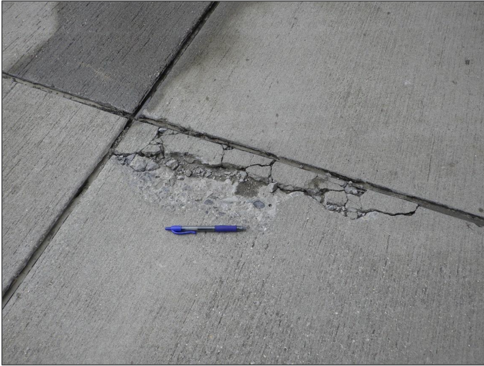
AP CARGO, Section 4330, Sample Unit 157 – Joint Spall
