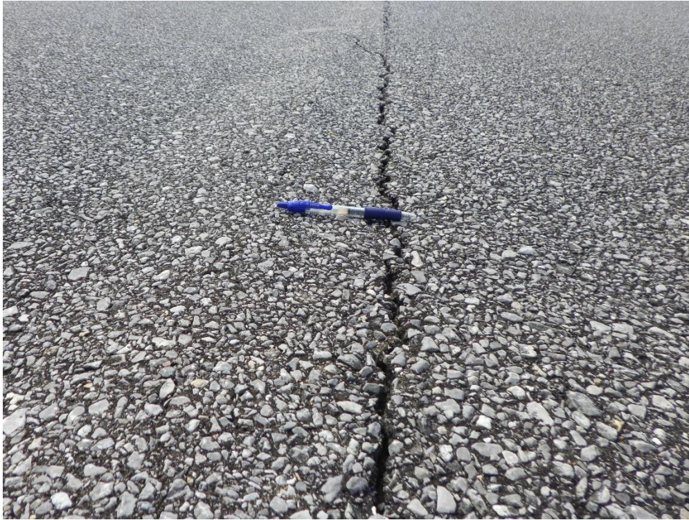
TW A, Section 115, Sample Unit 123 – Longitudinal & Transverse Cracking
