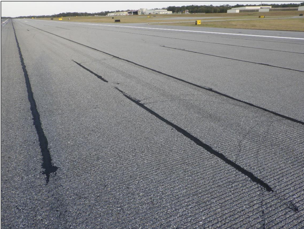
RW 8-26, Section 6235, Sample Unit 366 – Longitudinal & Transverse Cracking
