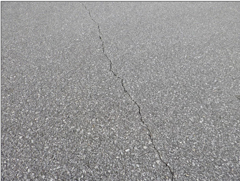
TW D, Section 405, Sample Unit 413 – Longitudinal & Transverse Cracking
