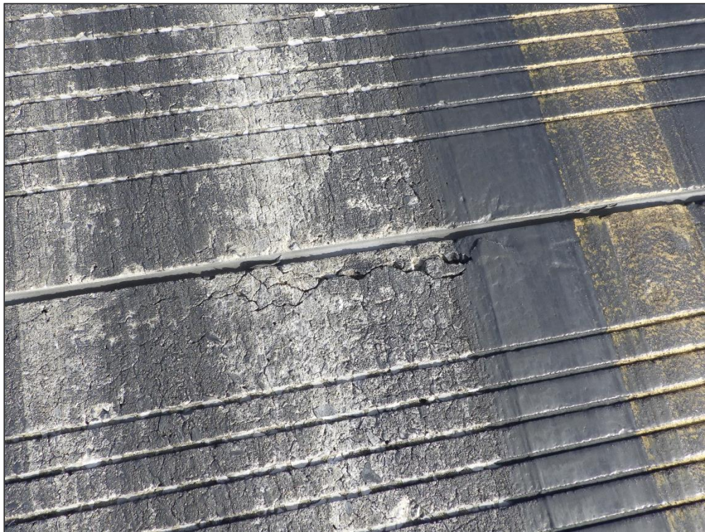
RW 17-35, Section 6125, Sample Unit 388 – Joint Spall
