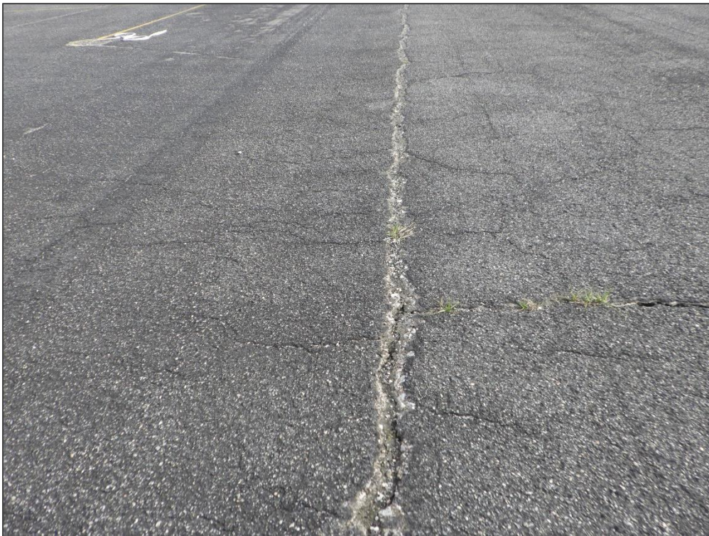
AP GA, Section 4510, Sample Unit 311 – Longitudinal & Transverse Cracking and Raveling
