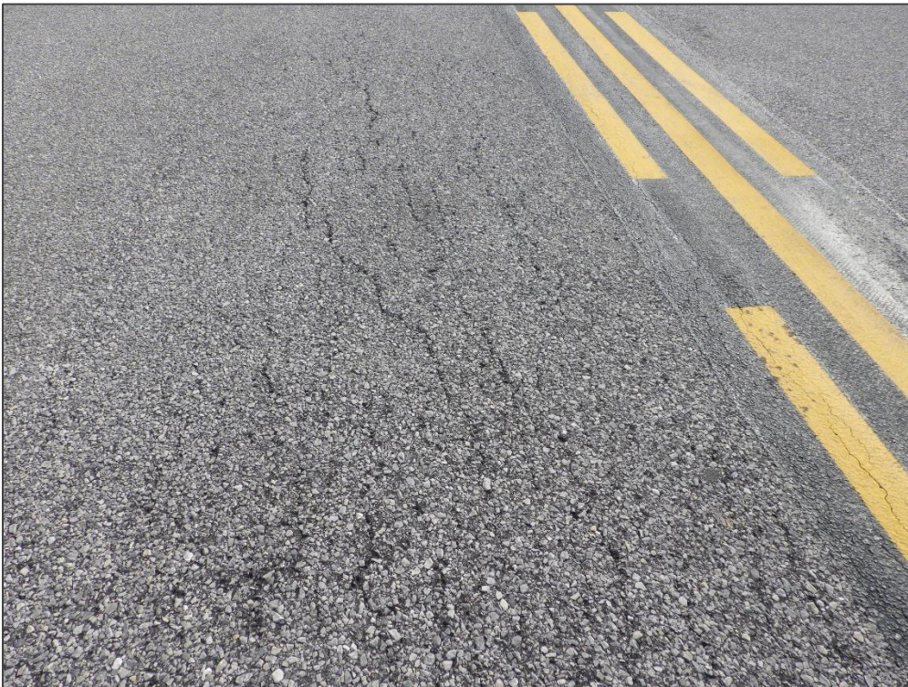
TW A1, Section 120, Sample Unit 102 – Alligator Cracking
