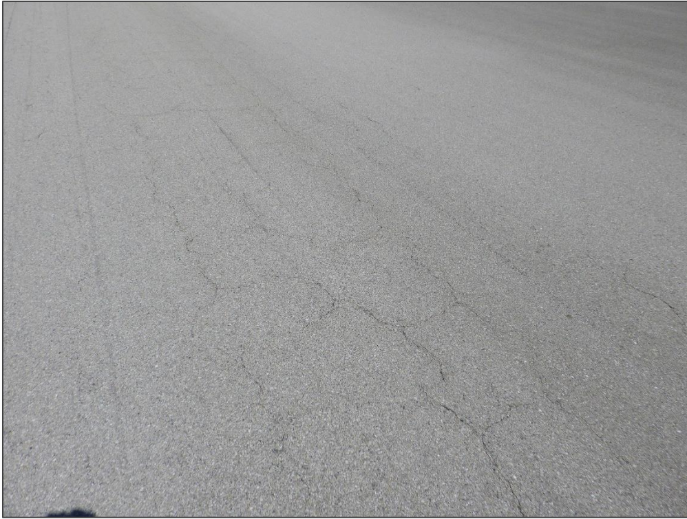
TW G, Section 1210, Sample Unit 432 – Alligator Cracking
