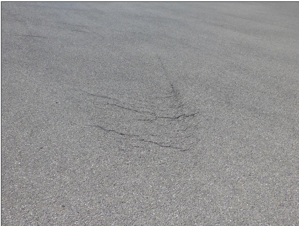
TW F4, Section 525, Sample Unit 200 – Slippage Cracking
