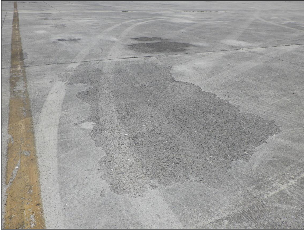
AP N, Section 4315, Sample Unit 310 – Scaling
