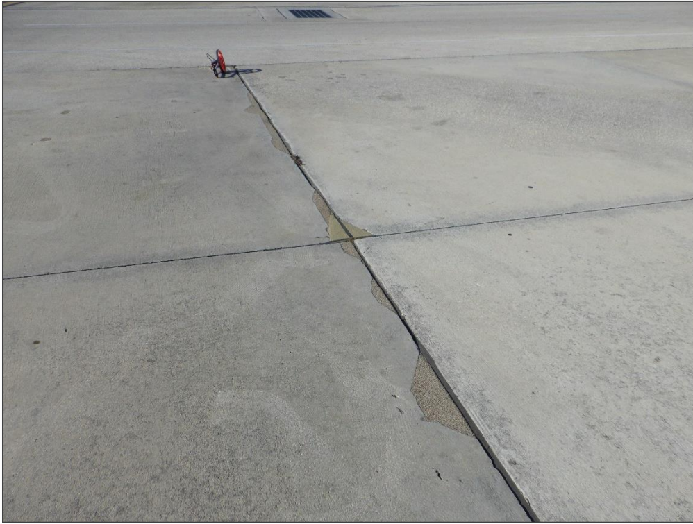
AP TERM, Section 4420, Sample Unit 507 – Small Patch
