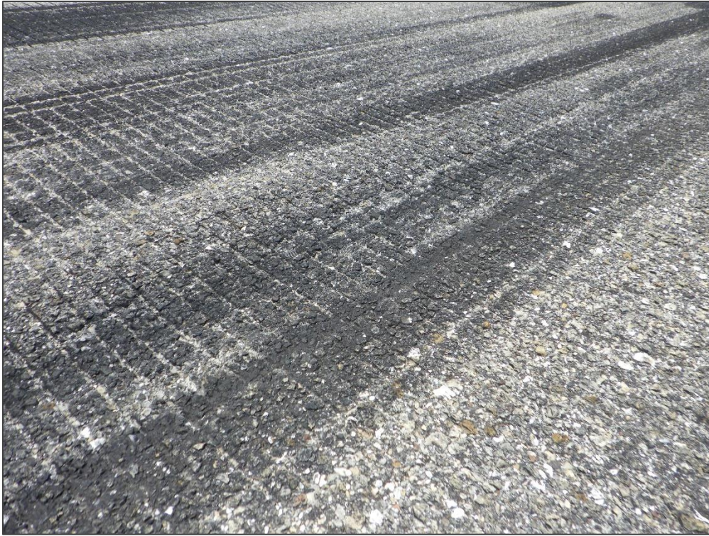
RW 6-24, Section 6115, Sample Unit 480 – Raveling
