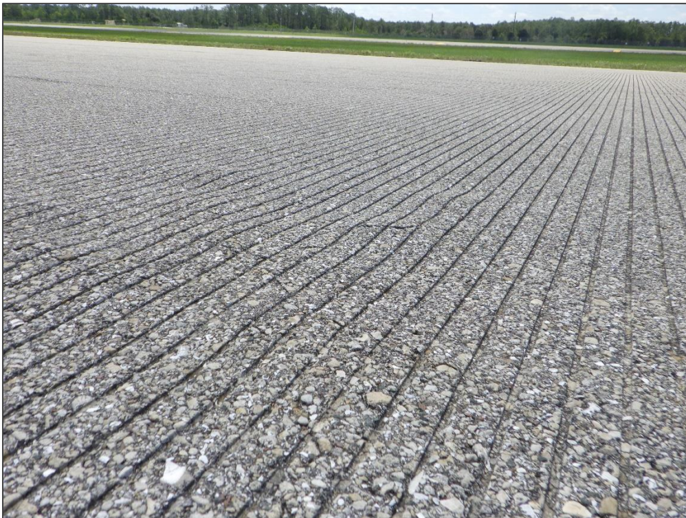
RW 6-24, Section 6105, Sample Unit 641 – Swelling
