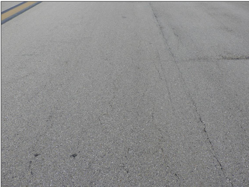
TW J, Section 535, Sample Unit 549 – Alligator Cracking and Longitudinal & Transverse Cracking
