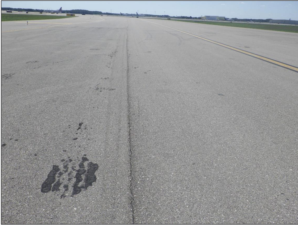
TW H, Section 1005, Sample Unit 624 – Longitudinal & Transverse Cracking
