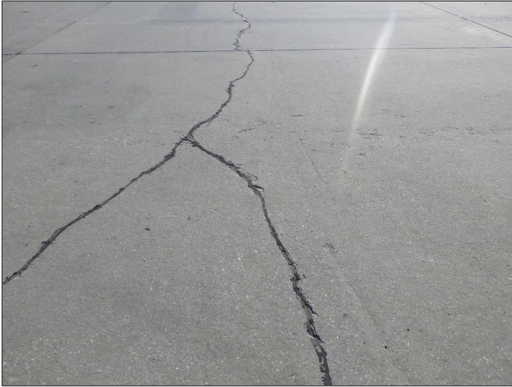
AP CARGO, Section 4110, Sample Unit 104 – Linear Cracking
