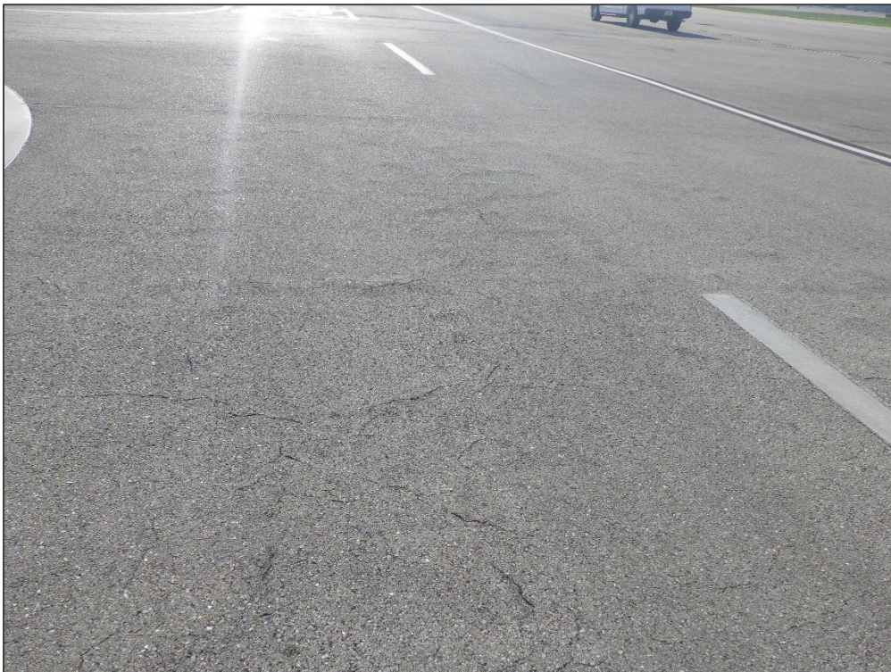
AP TERM, Section 4415, Sample Unit 214 – Longitudinal & Transverse Cracking and Swelling
