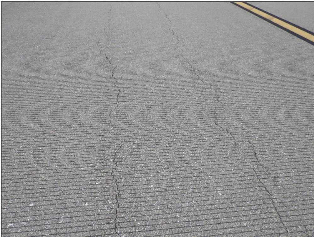
TW A, Section 105, Sample Unit 279 – Longitudinal & Transverse Cracking
