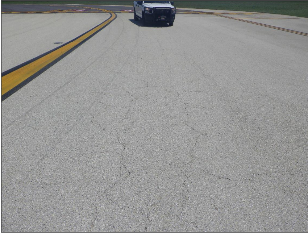
TW F1, Section 240, Sample Unit 102 – Alligator Cracking
