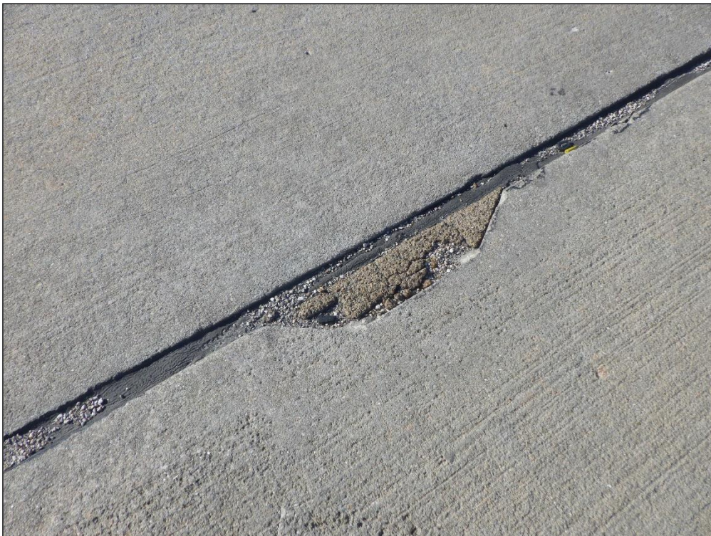
AP TERM, Section 4430, Sample Unit 102 – Small Patch
