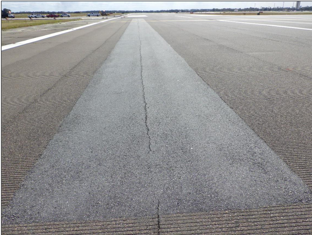
RW 18-36, Section 6233, Sample Unit 636 – Patching
