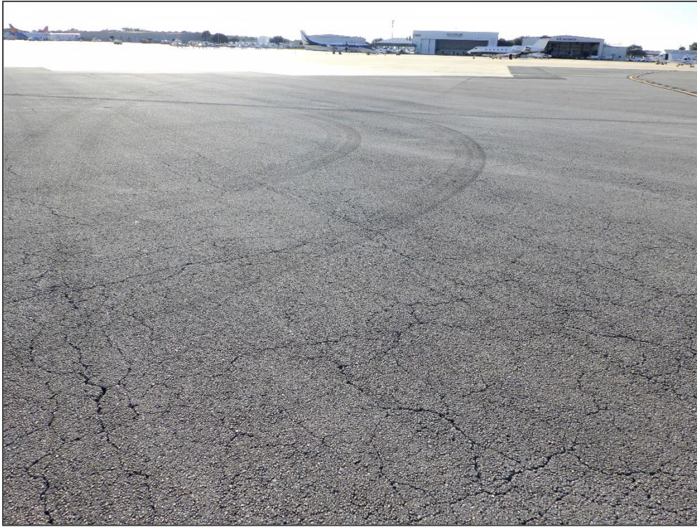
AP SW, Section 4205, Sample Unit 505 – Vicinity
