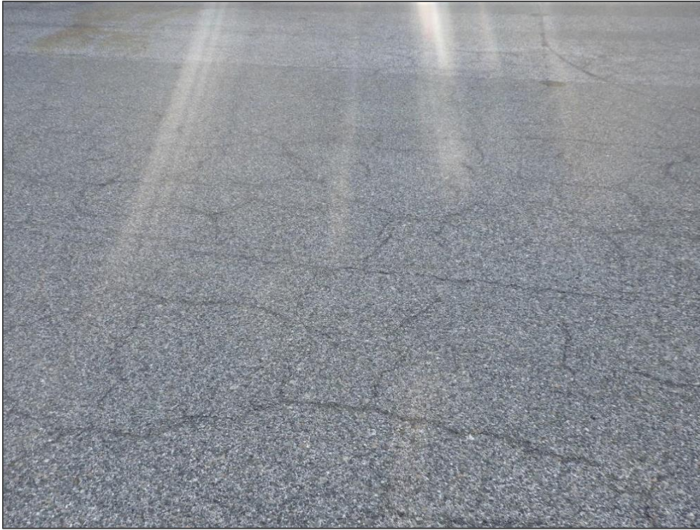
AP, Section 4110, Sample Unit 207 – Block Cracking
