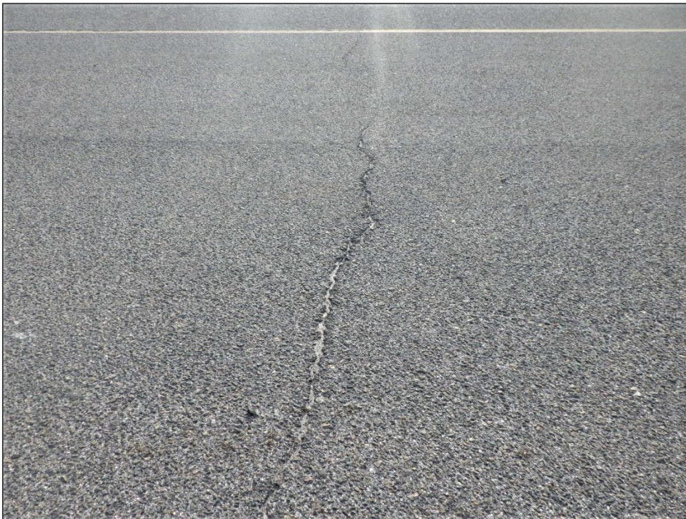
TW B, Section 205, Sample Unit 108– Longitudinal & Transverse Cracking
