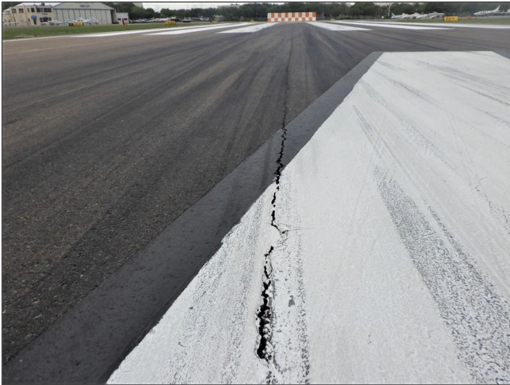
RW 7-25, Section 6208, Sample Unit 158 – Longitudinal & Transverse Cracking
