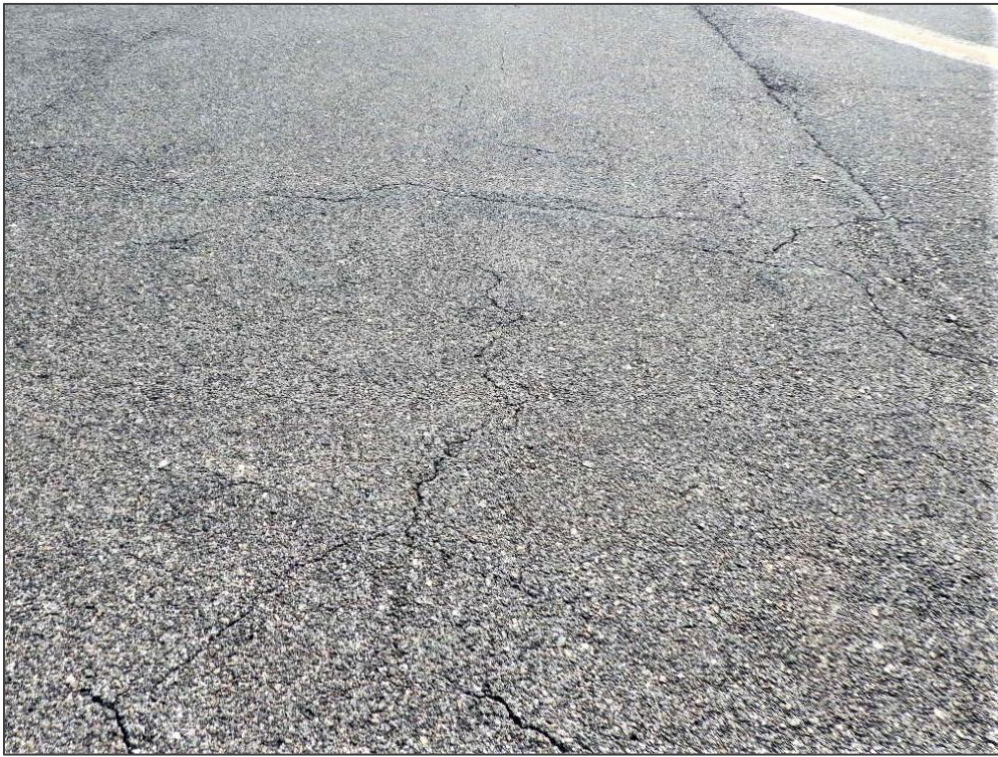
TW A, Section 105, Sample Unit 103 – Longitudinal & Transverse Cracking, Swelling, and Raveling
