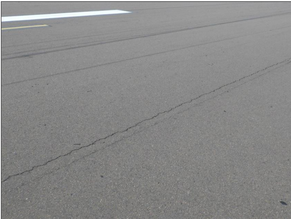
RW 7-25, Section 6210, Sample Unit 136 – Longitudinal & Transverse Cracking
