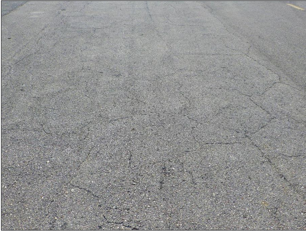
TW C, Section 307, Sample Unit 209 – Block Cracking and Swelling
