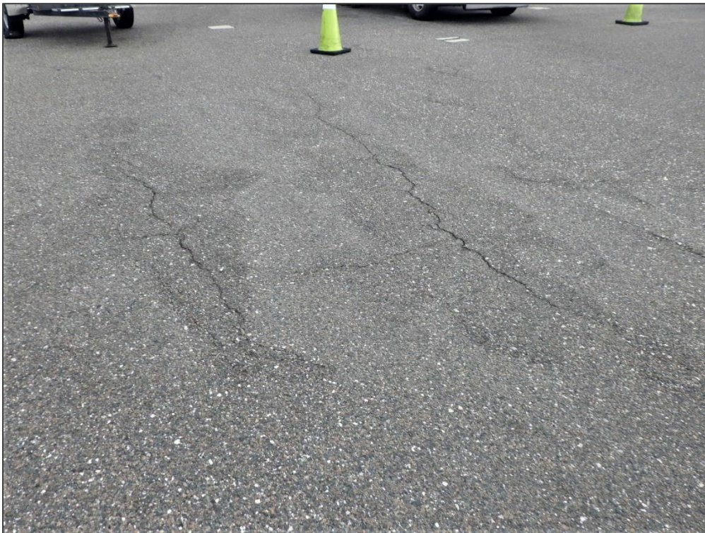
AP NW, Section 4310, Sample Unit 200 – Longitudinal & Transverse Cracking and Swelling
