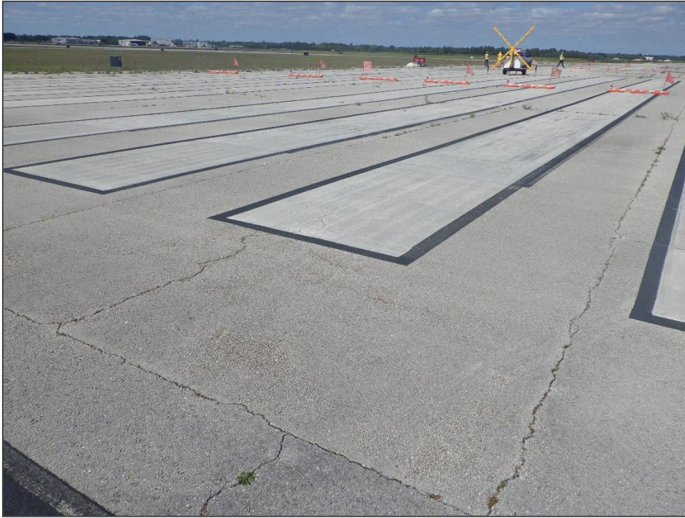
RW 9-27, Section 6205, Sample Unit 100 – Longitudinal & Transverse Cracking and Weathering
