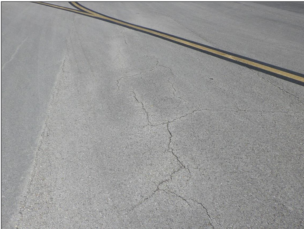
TW C, Section 305, Sample Unit 704– Longitudinal & Transverse Cracking
