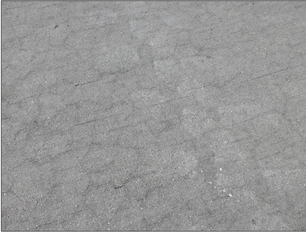
AP HELI, Section 4260, Sample Unit 646 – Shrinkage Cracking
