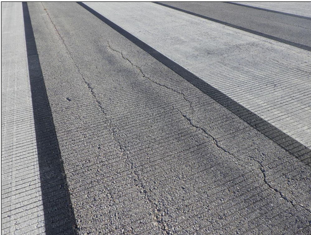
RW 18-36, Section 6105, Sample Unit 302 – Longitudinal & Transverse Cracking and Swelling
