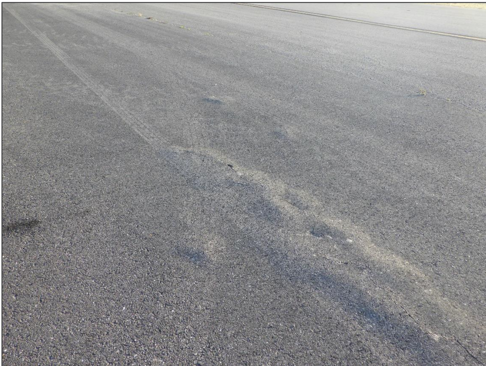
TW A, Section 120, Sample Unit 151 – Swelling
