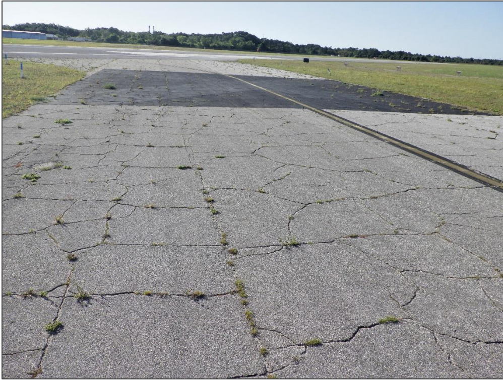
TW F, Section 605, Sample Unit 301 – Block Cracking
