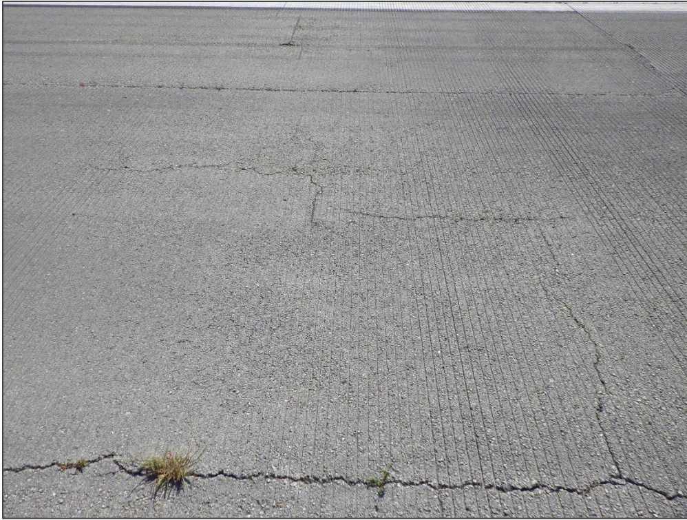
RW 18-36, Section 6105, Sample Unit 376 – Longitudinal & Transverse Cracking
