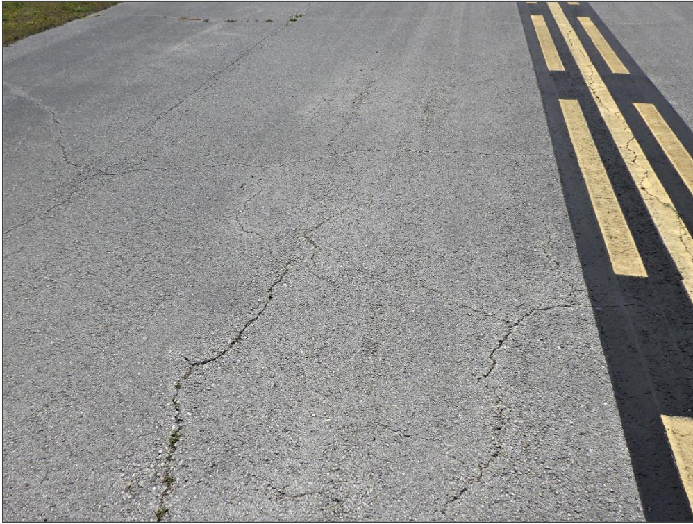
TW B, Section 205, Sample Unit 502 – Longitudinal & Transverse Cracking
