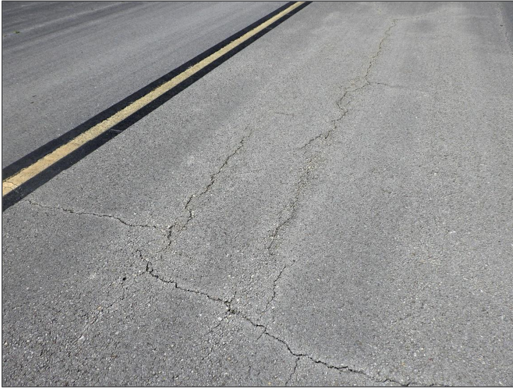
TW A, Section 105, Sample Unit 108 – Longitudinal & Transverse Cracking and Weathering
