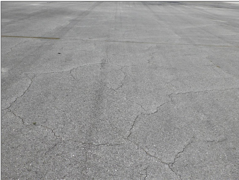
AP E, Section 4205, Sample Unit 250 – Block Cracking
