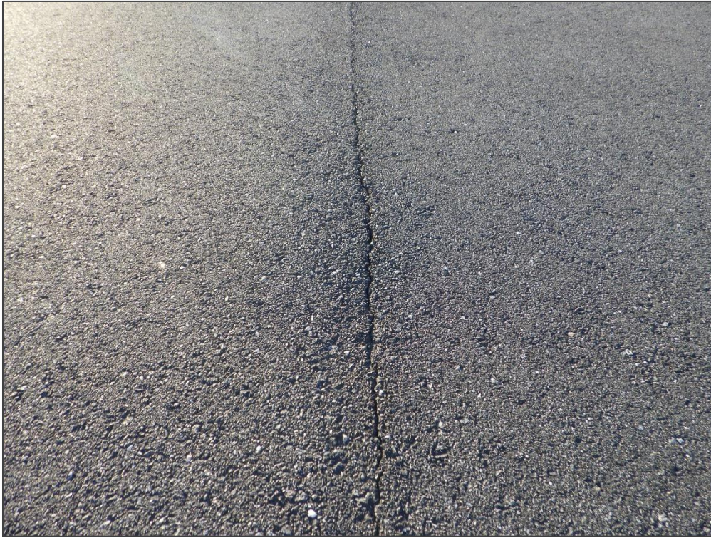
AP S, Section 4310, Sample Unit 450 - Longitudinal & Transverse Cracking
