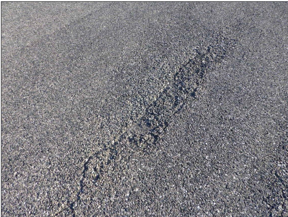
TW A, Section 106, Sample Unit 216 - Raveling
