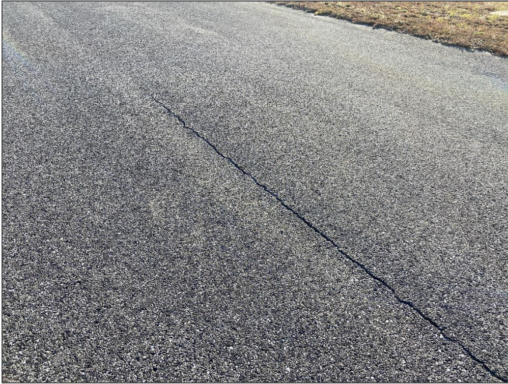
TW A, Section 106, Sample Unit 169 – Longitudinal & Transverse Cracking
