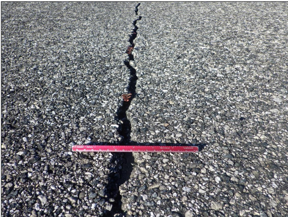
AP TERM, Section 4110, Sample Unit 97 - Joint Reflection Cracking
