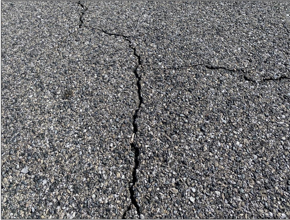
TW B, Section 205, Sample Unit 228 – Longitudinal and Transverse Cracking
