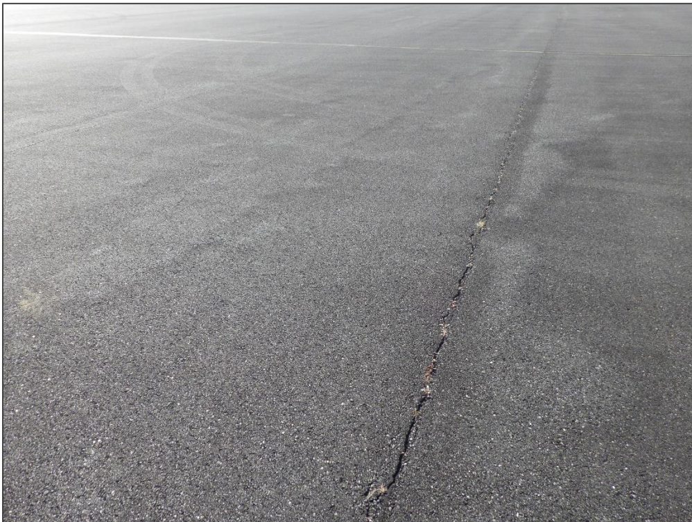
AP N, Section 4410, Sample Unit 554 - Longitudinal & Transverse Cracking and Swelling
