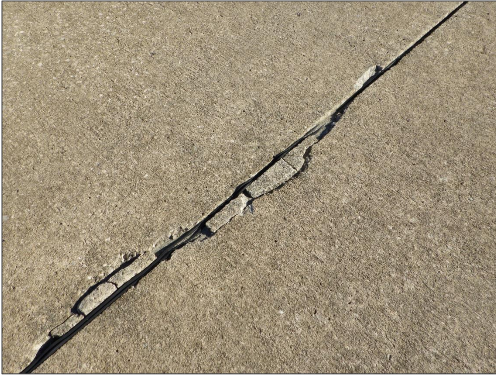
AP TERM, Section 4105, Sample Unit 456 - Joint Spall
