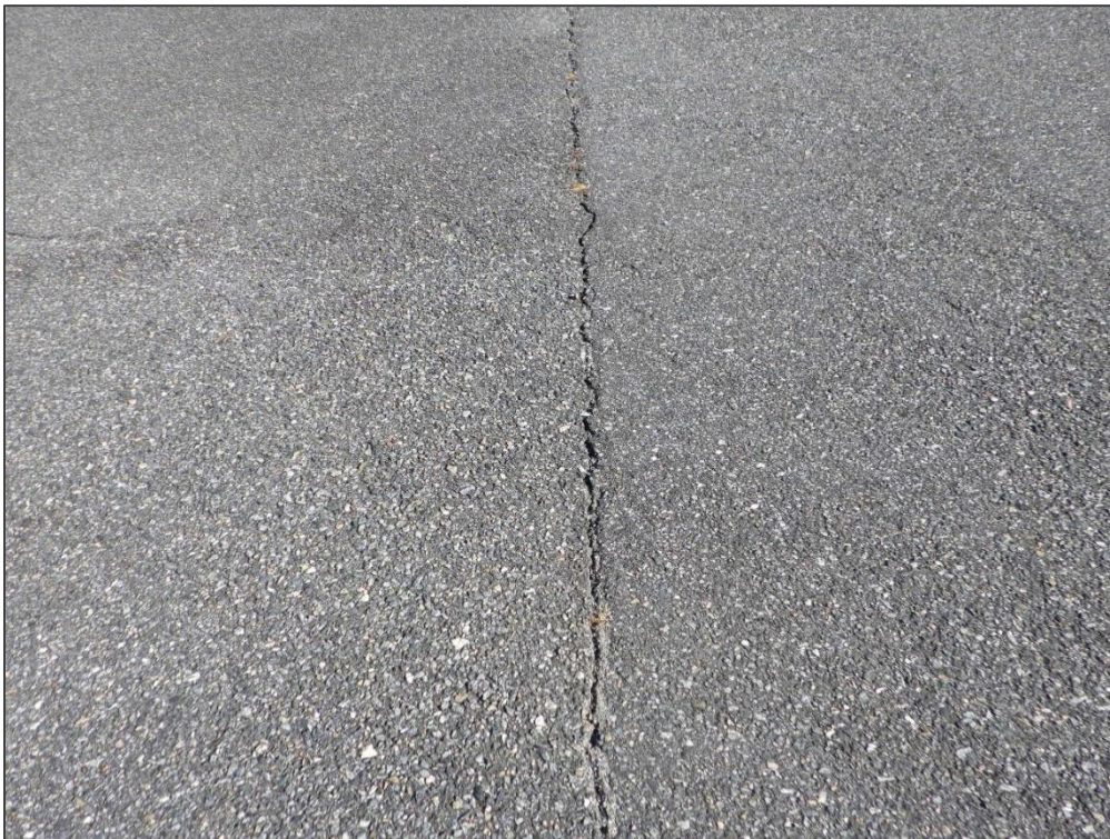
AP C, Section 4505, Sample Unit 101 - Longitudinal and Transverse Cracking
