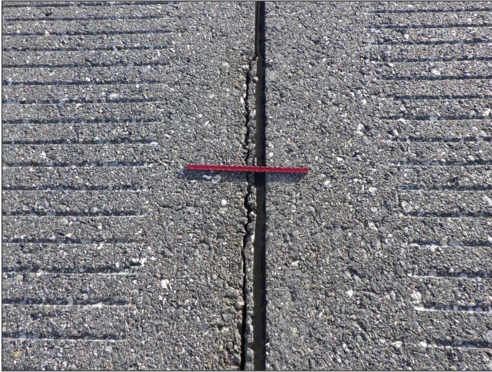
RW 9-27, Section 6210, Sample Unit 128 - Longitudinal & Transverse Cracking
