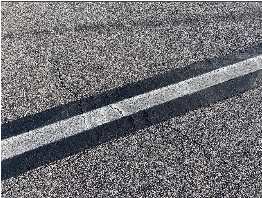
AP RU 18, Section 5505, Sample Unit 101 - Longitudinal & Transverse Cracking
