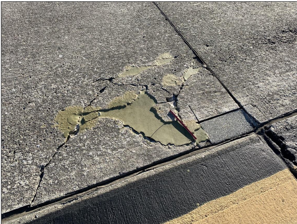
AP TERM, Section 4105, Sample Unit 110 - Corner Break
