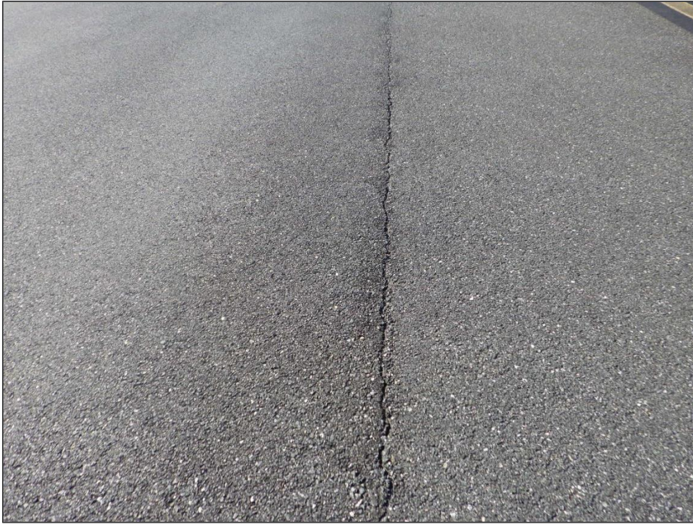
AP N, Section 4415, Sample Unit 362 - Longitudinal & Transverse Cracking
