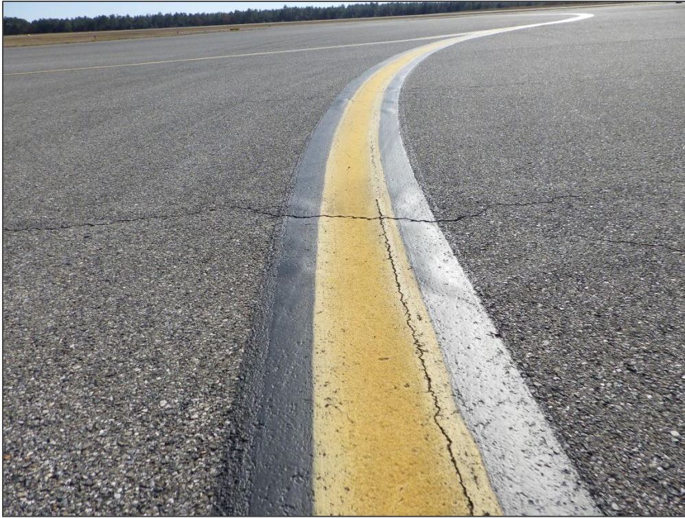
AP CARGO, Section 4210, Sample Unit 213 - Longitudinal & Transverse Cracking
