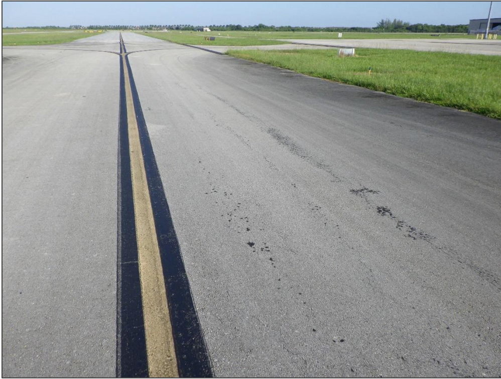
TW C, Section 910, Sample Unit 115 – Bleeding
