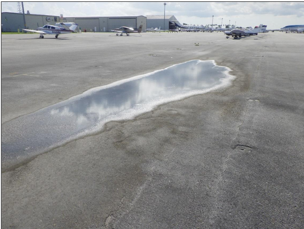
AP N, Section 4205, Sample Unit 312 – Depression and Longitudinal & Transverse Cracking
