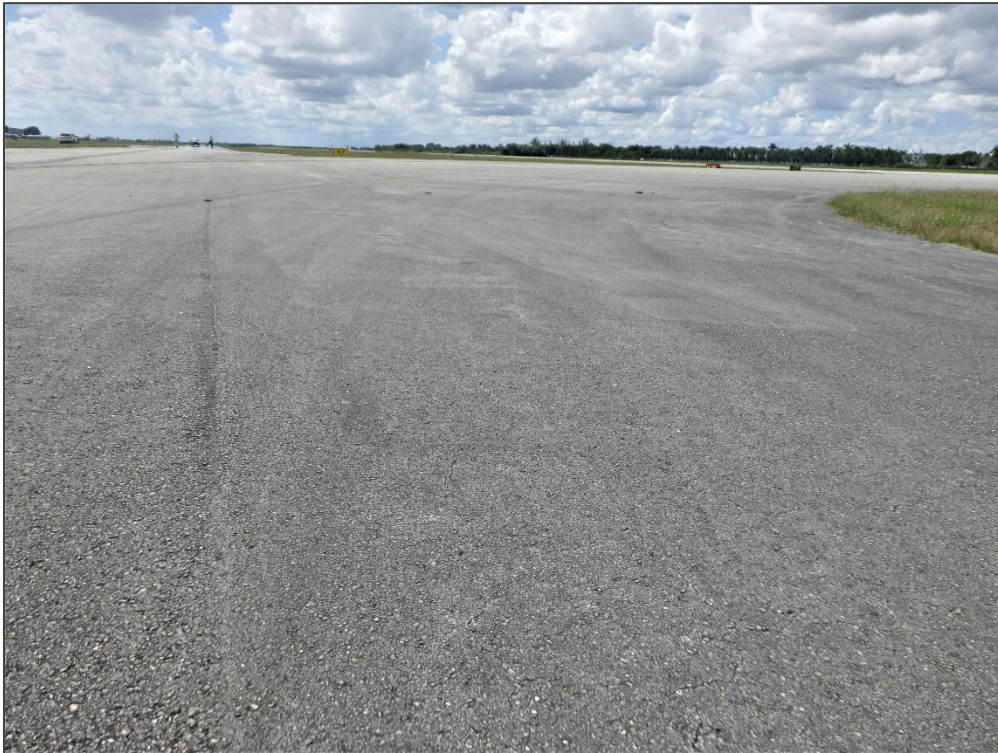
TW A, Section 108, Sample Unit 148 – Swelling
