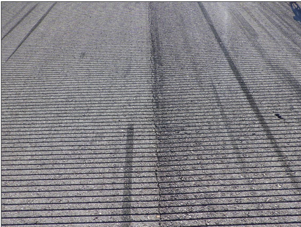
RW 9R-27L, Section 6305, Sample Unit 336 – Longitudinal & Transverse Cracking
