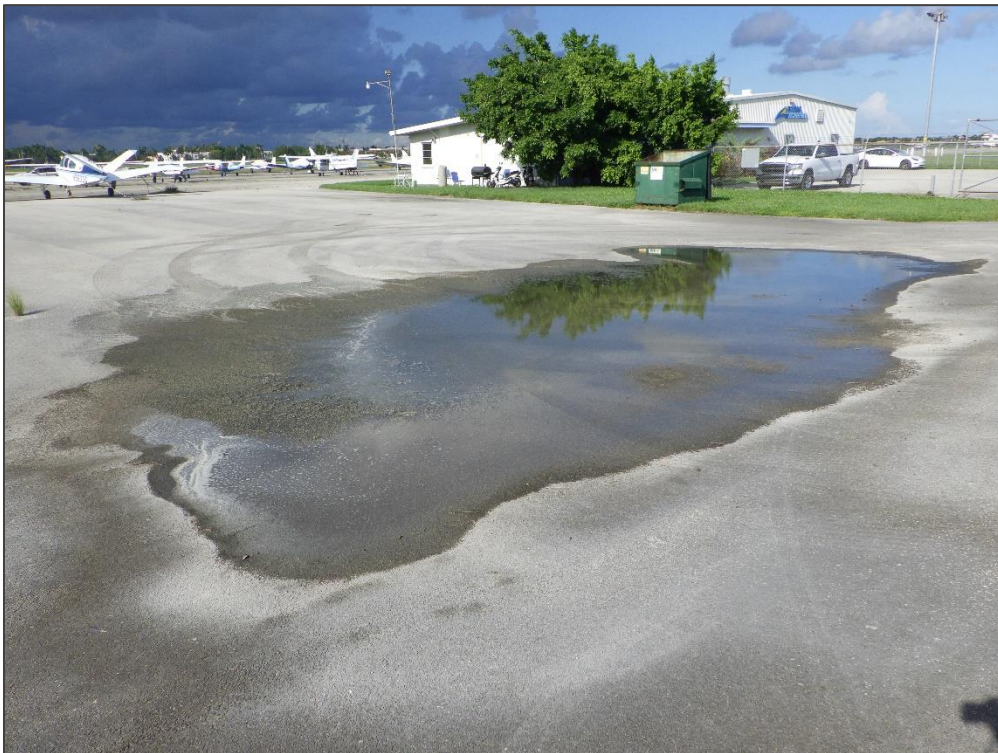
AP N, Section 4230, Sample Unit 102 – Depression
