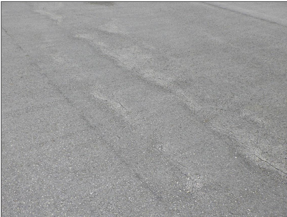
AP S, Section 4115, Sample Unit 534 – Longitudinal & Transverse Cracking and Swelling
