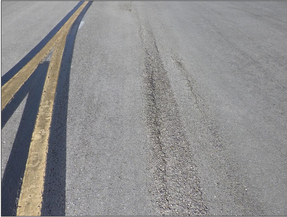
TW E, Section 535, Sample Unit 158 – Longitudinal & Transverse Cracking and Raveling
