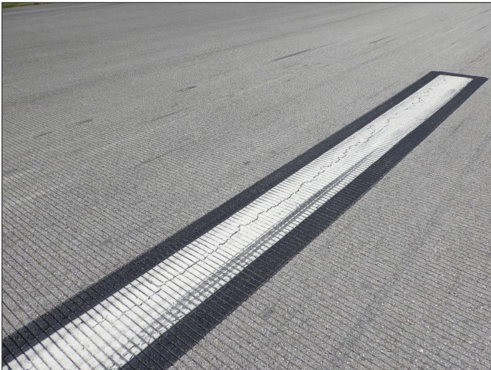
RW 9L-27R, Section 6105, Sample Unit 312 – Longitudinal & Transverse Cracking
