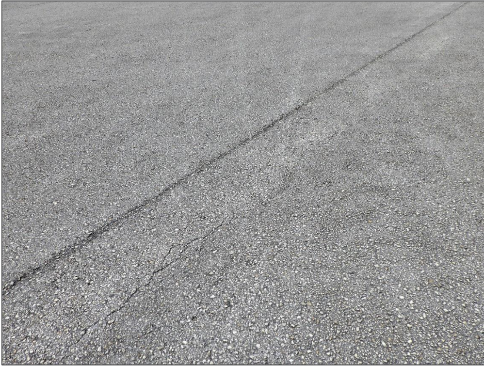
AP S, Section 4115, Sample Unit 235 – Longitudinal & Transverse Cracking and Swelling
