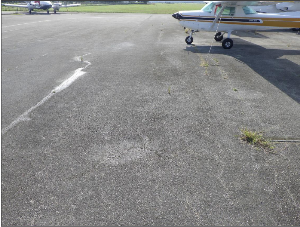
AP N, Section 4220, Sample Unit 532 – Block Cracking and Swelling
