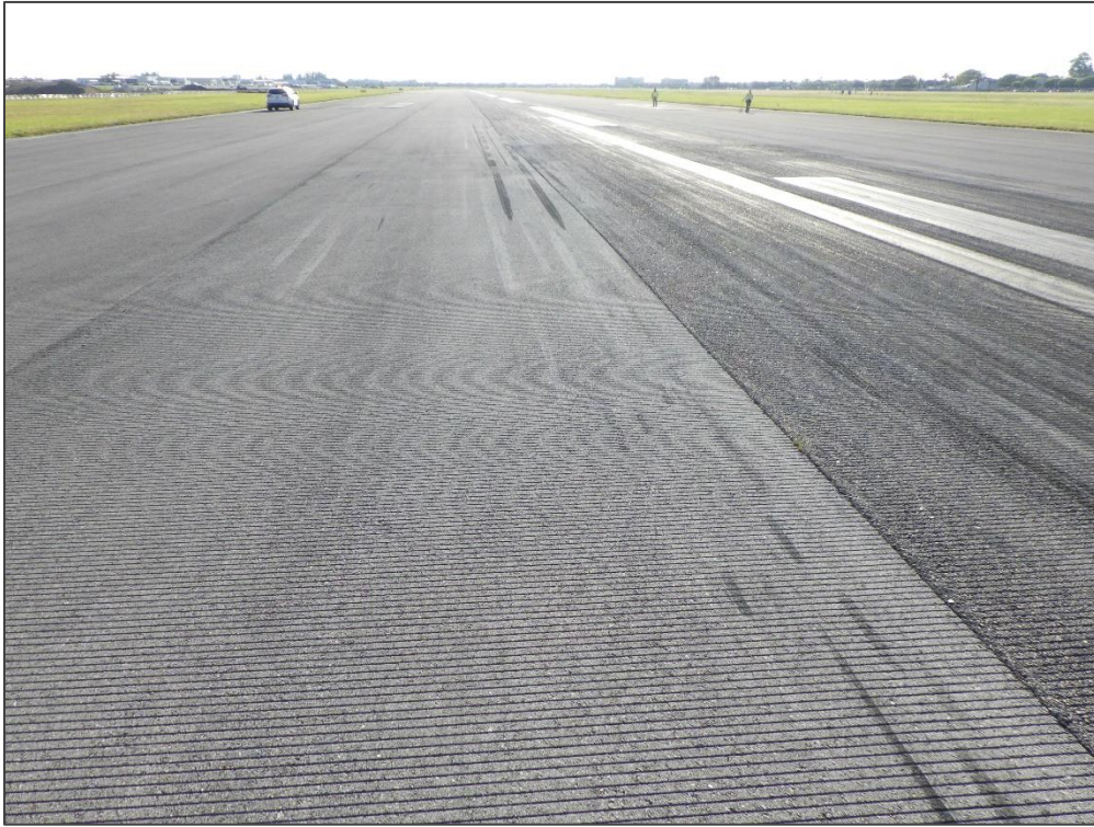
RW 9R-27L, Section 6305, Sample Unit 325 – Longitudinal & Transverse Cracking
