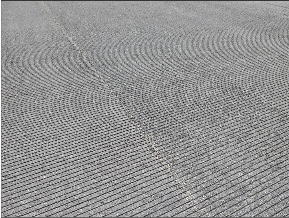
RW 9L-27R, Section 6105, Sample Unit 309 – Longitudinal & Transverse Cracking
