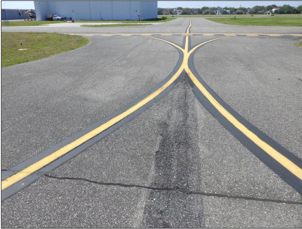
TW E, Section 650, Sample Unit 300– Longitudinal & Transverse Cracking and Raveling
