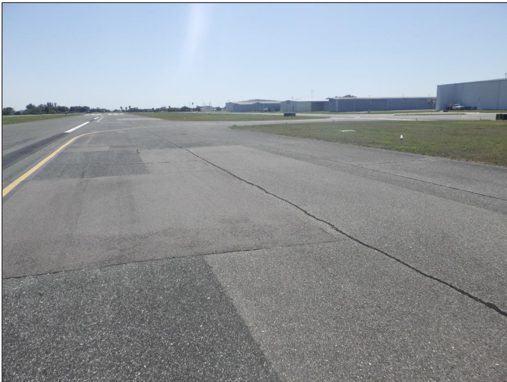
RW 18-36, Section 6205, Sample Unit 122 – Longitudinal & Transverse Cracking and Patching
