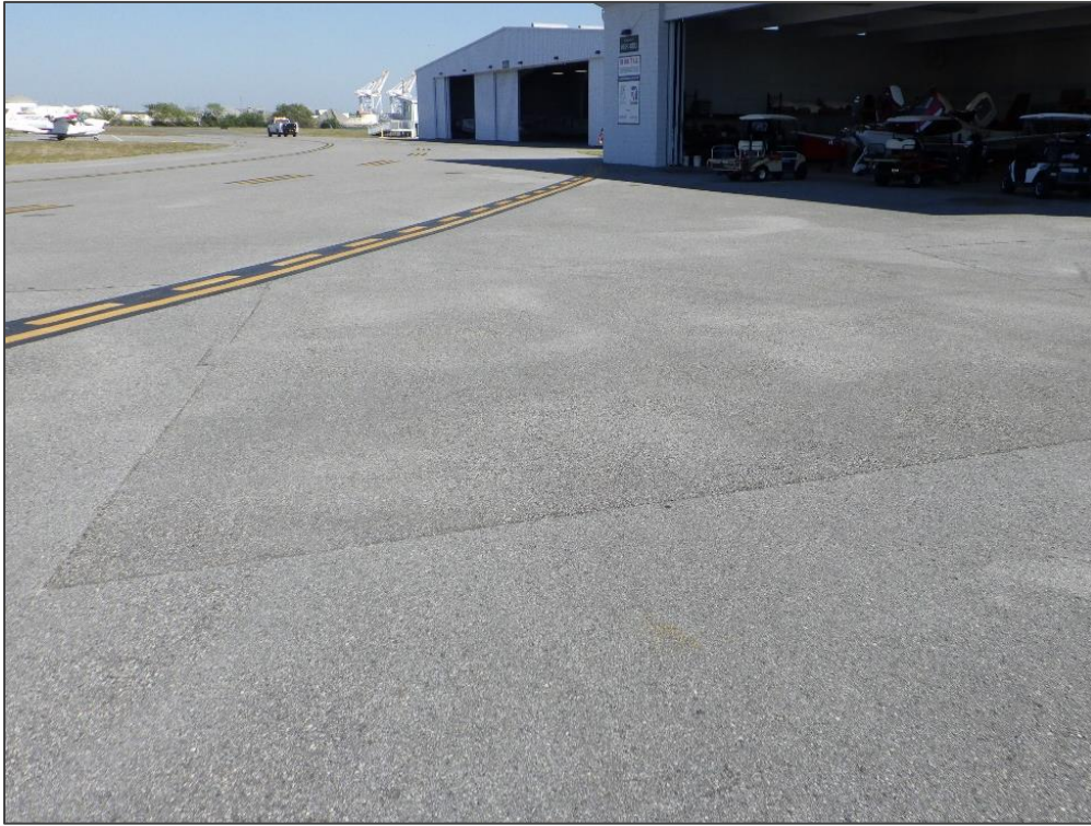
AP MID, Section 4110, Sample Unit 603 – Patching
