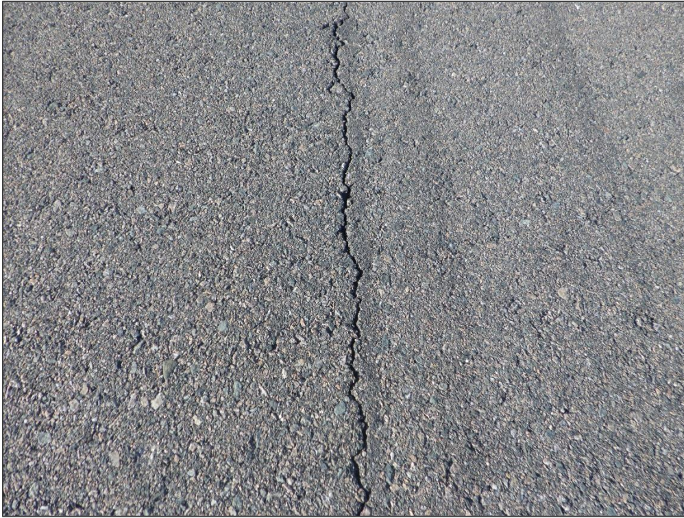
RW 4-22, Section 6105, Sample Unit 121 – Longitudinal & Transverse Cracking
