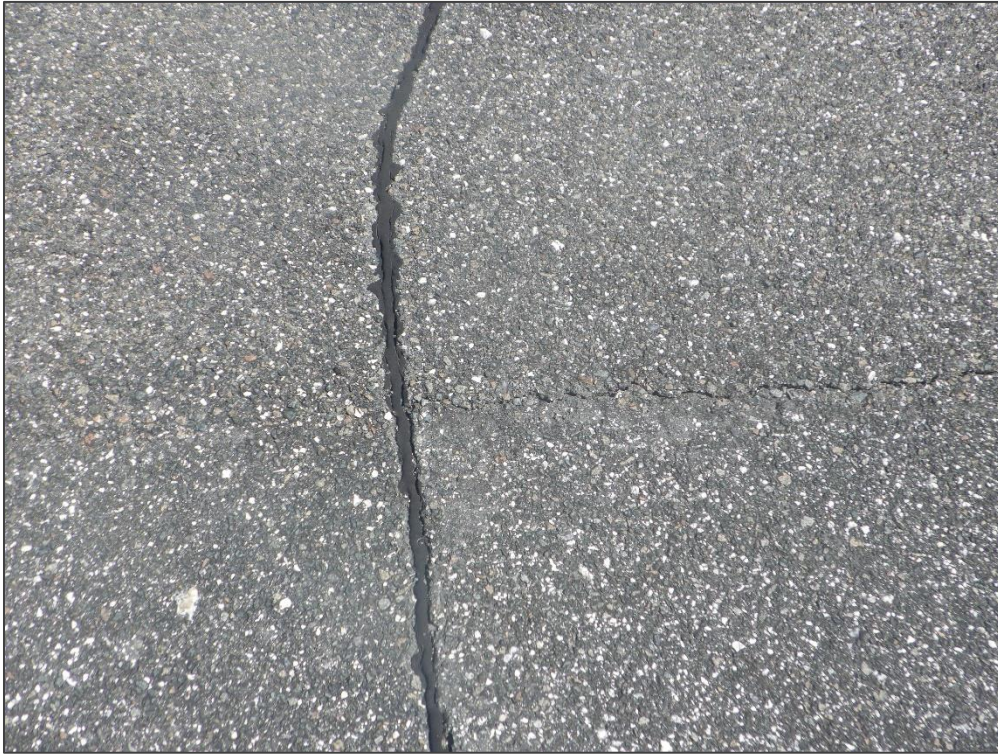
RW 18-36, Section 6205, Sample Unit 102 – Longitudinal & Transverse Cracking
