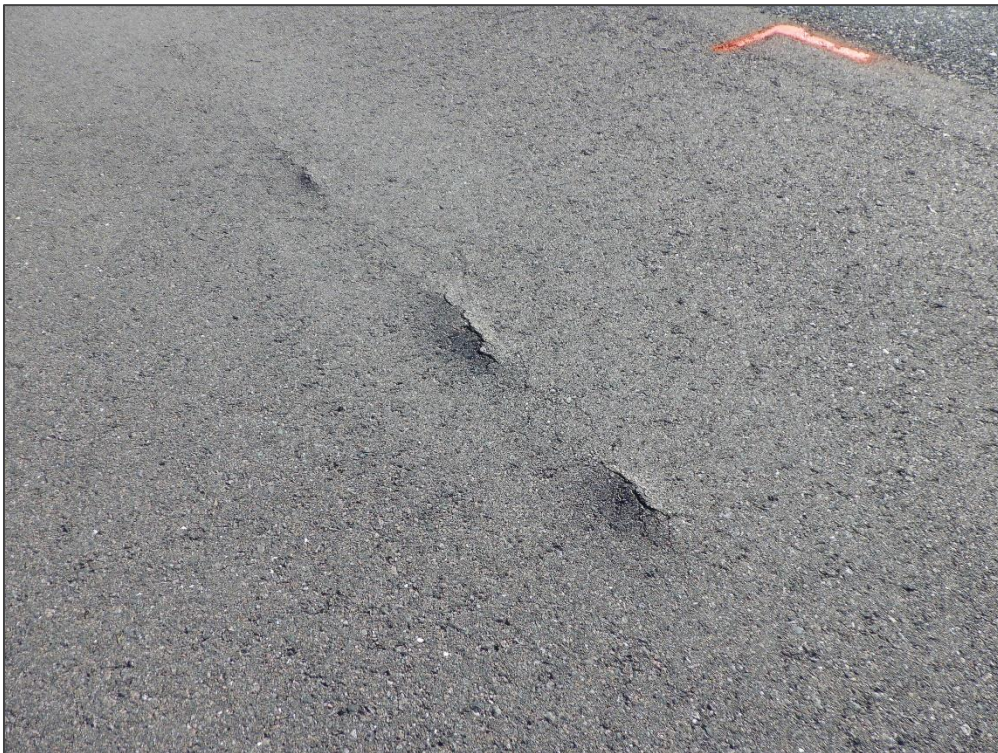
RW 4-22, Section 6105, Sample Unit 161 – Longitudinal & Transverse Cracking and Swelling
