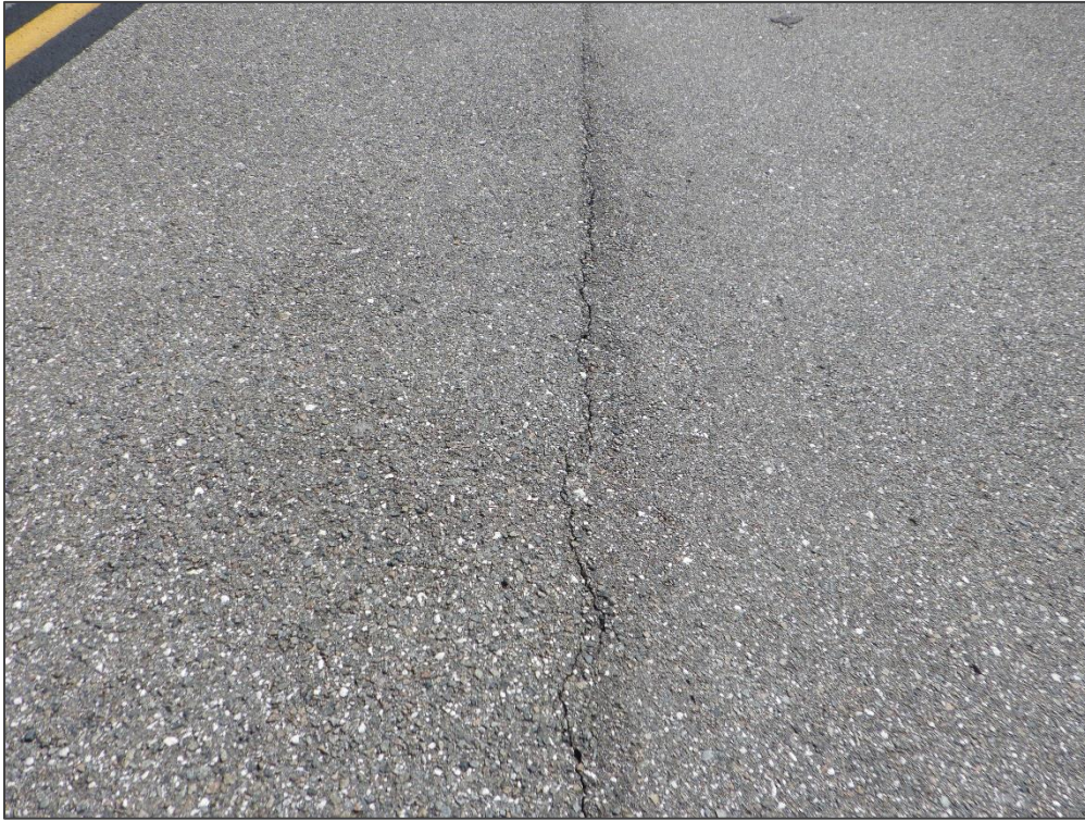
TW G, Section 750, Sample Unit 401 – Longitudinal & Transverse Cracking and Weathering
