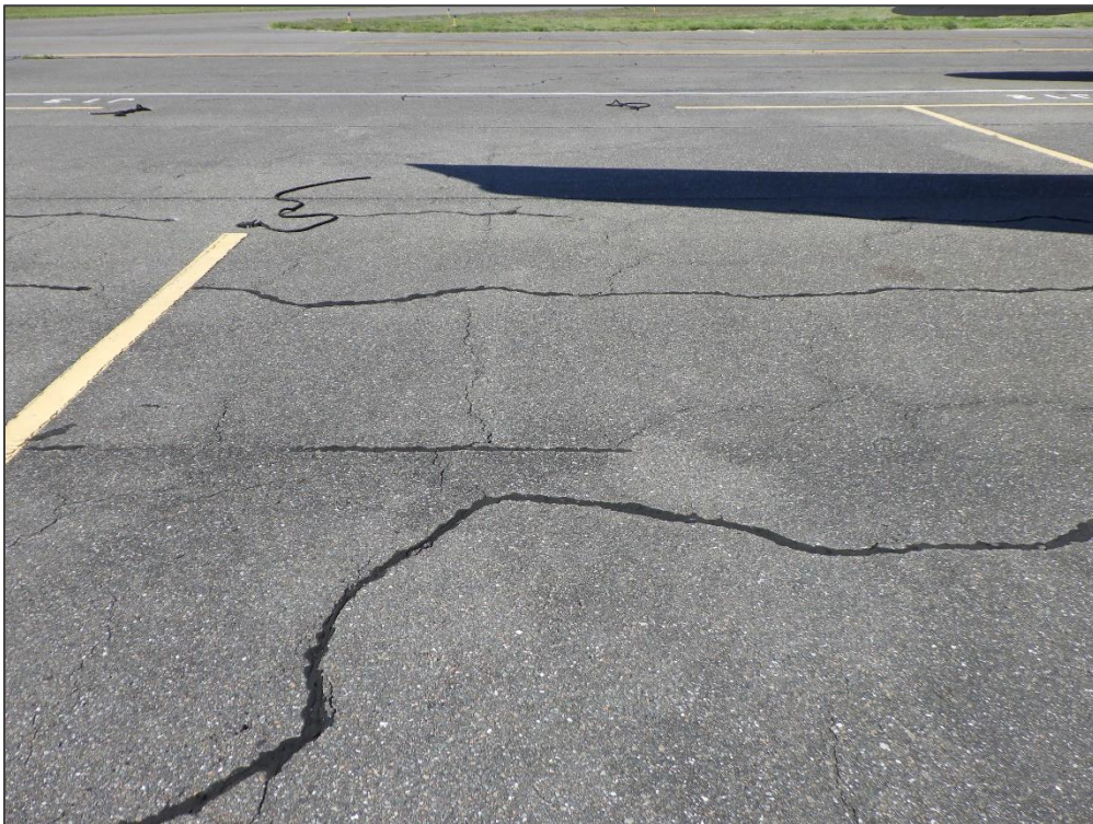
AP MID, Section 4125, Sample Unit 401 – Longitudinal & Transverse Cracking
