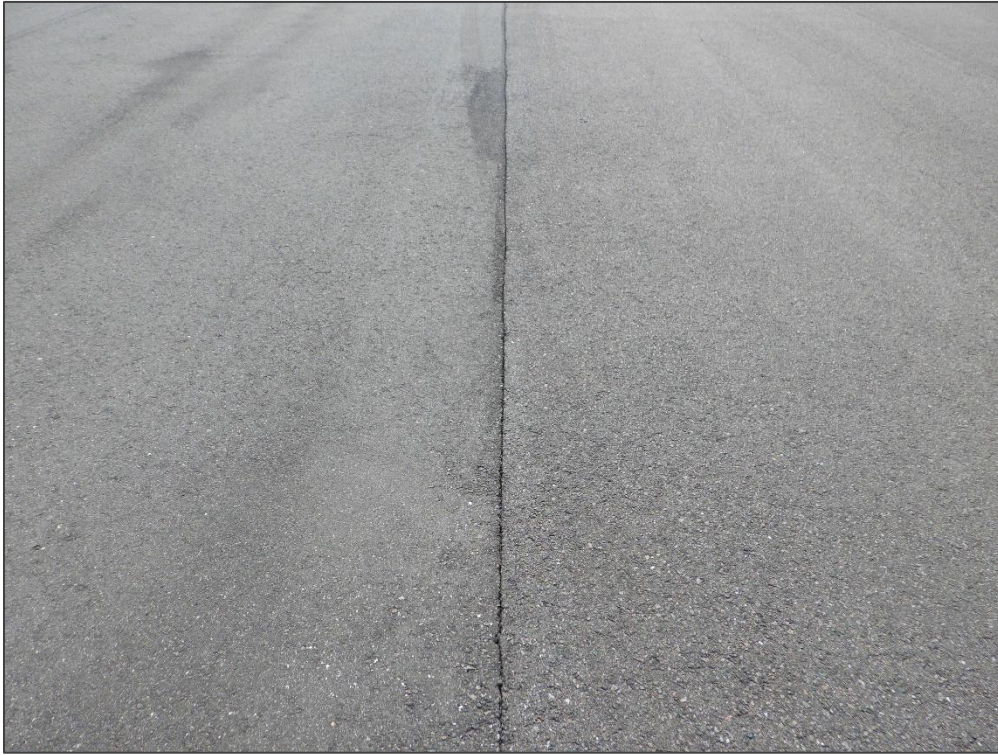
TW A, Section 105, Sample Unit 122 – Longitudinal & Transverse Cracking
