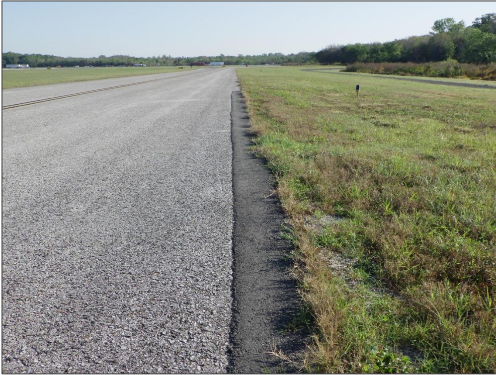
TW E, Section 505, Sample Unit 134 – Patching
