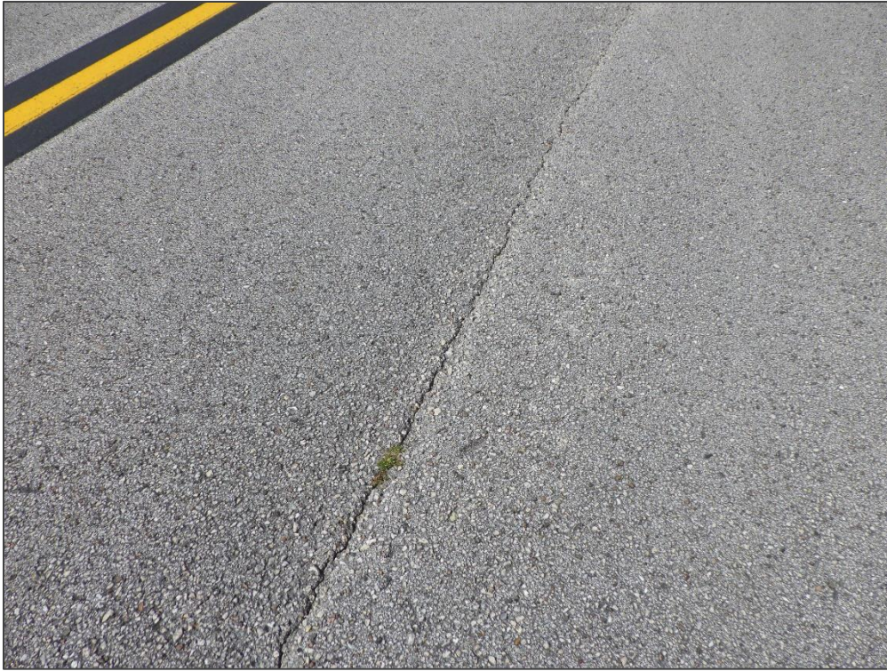
TW A, Section 105, Sample Unit 109 – Longitudinal & Transverse Cracking
