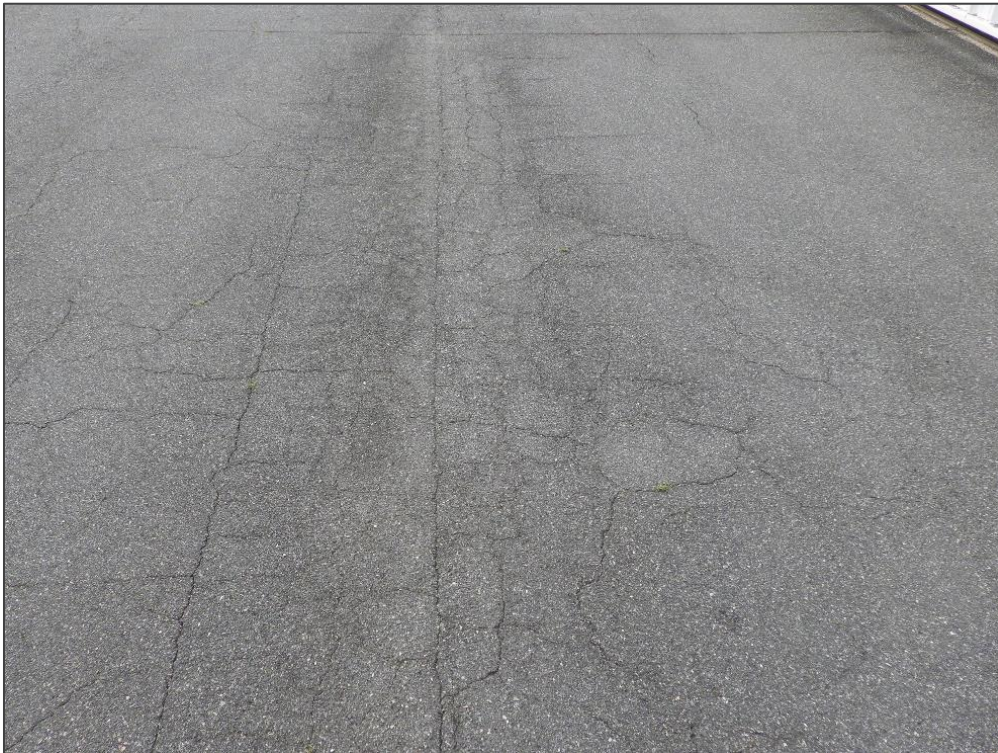
AP T-HANG, Section 4310, Sample Unit 105 – Alligator Cracking
