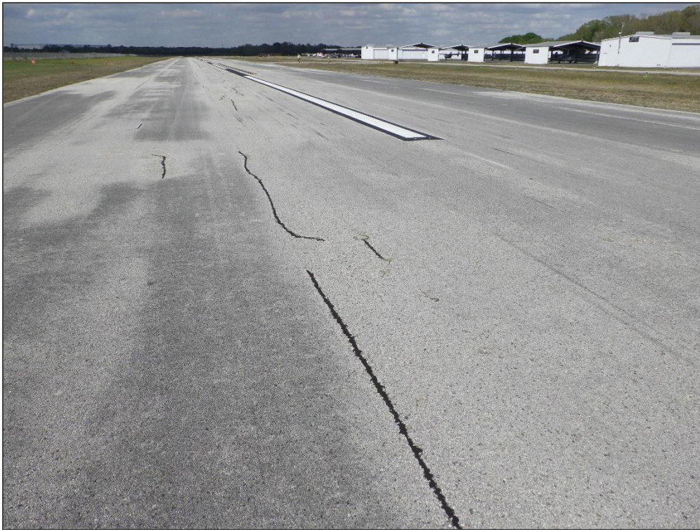
RW 18-38, Section 6105, Sample Unit 105 – Longitudinal & Transverse Cracking
