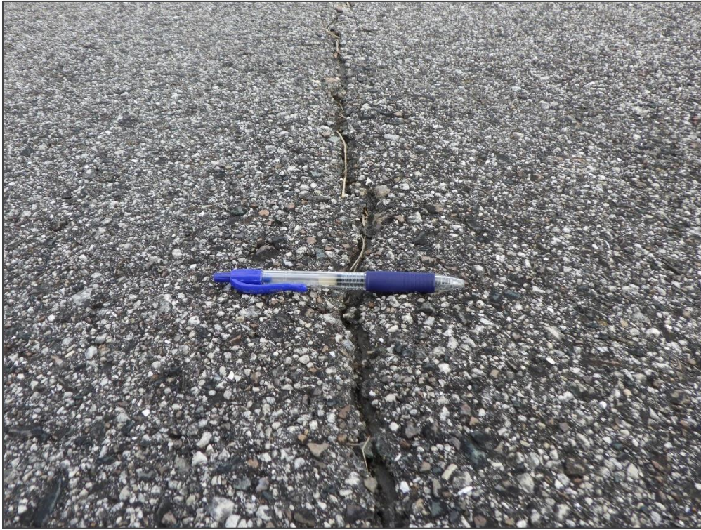
AP S, Section 4110, Sample Unit 252 – Longitudinal & Transverse Cracking
