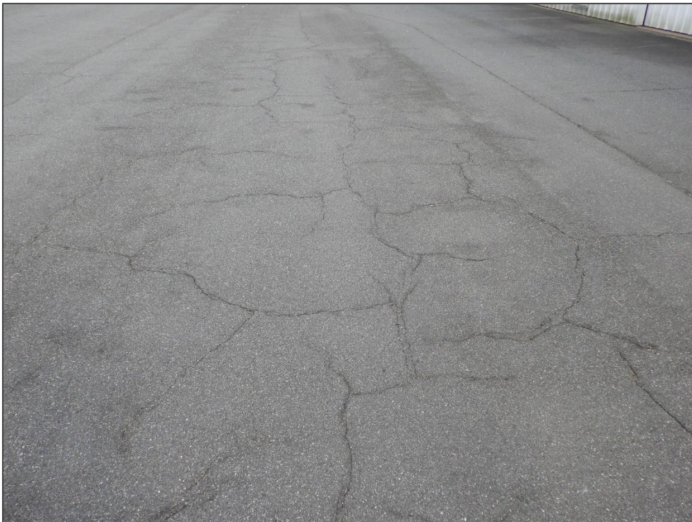
AP N, Section 4210, Sample Unit 306 – Block Cracking
