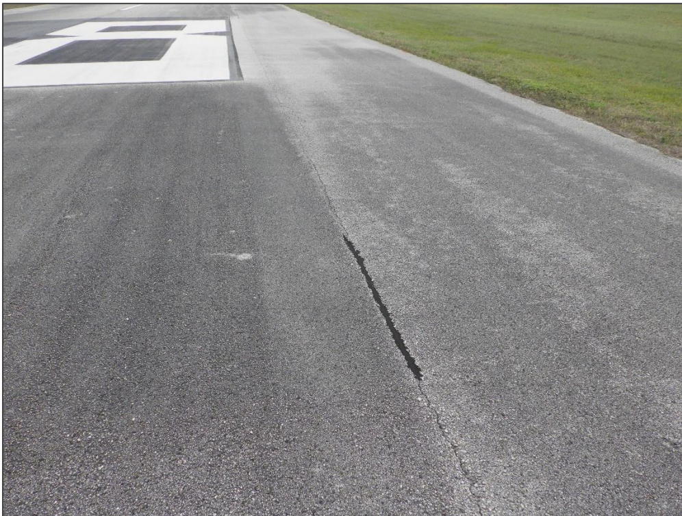
RW 18-36, Section 6105, Sample Unit 160 – Longitudinal & Transverse Cracking
