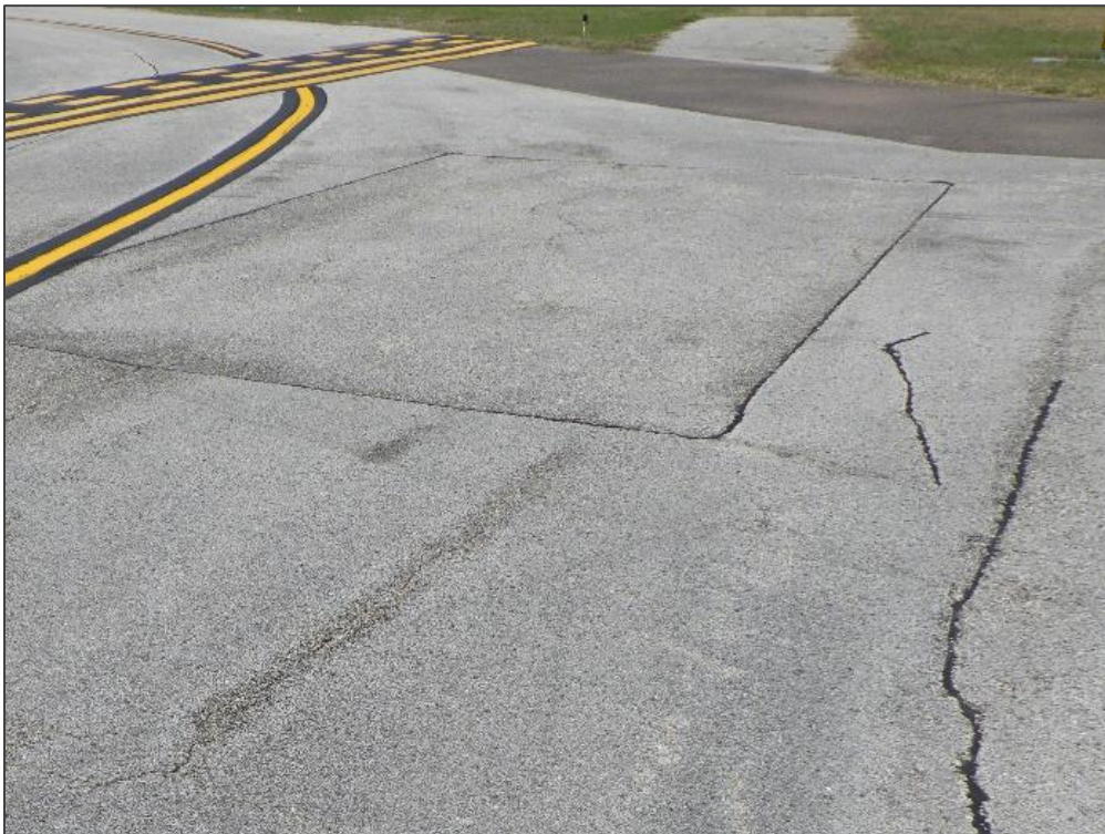
TW A6, Section 190, Sample Unit 130 – Patching and Longitudinal & Transverse Cracking
