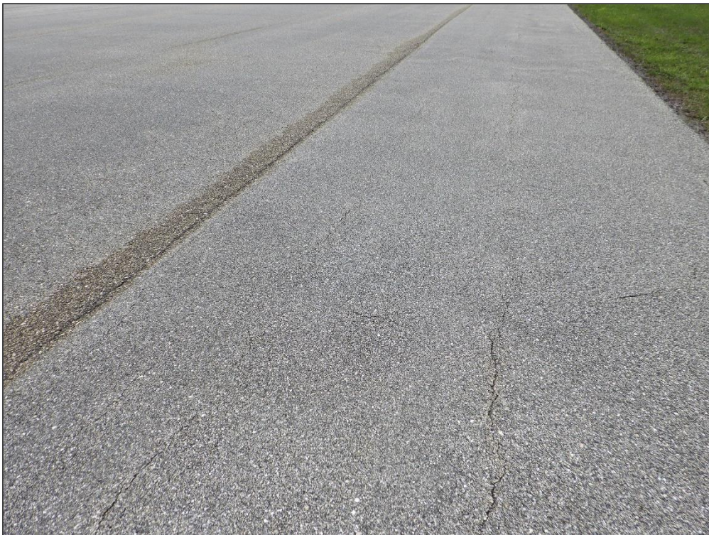
RW 13-31, Section 6110, Sample Unit 128 – Longitudinal & Transverse Cracking and Swelling
