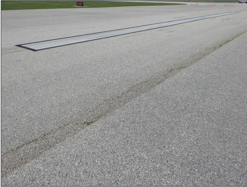
RW 13-31, Section 6105, Sample Unit 336 – Longitudinal & Transverse Cracking
