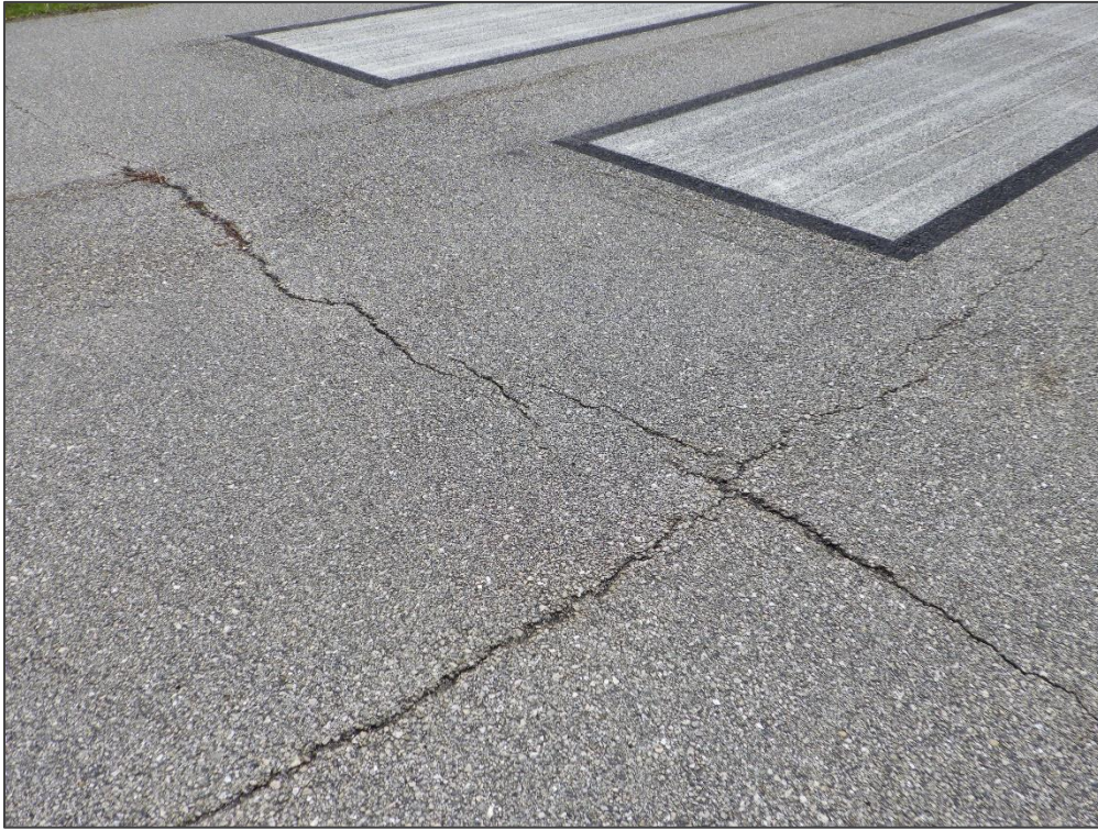
RW 13-31, Section 6125, Sample Unit 395 – Joint Reflection Cracking
