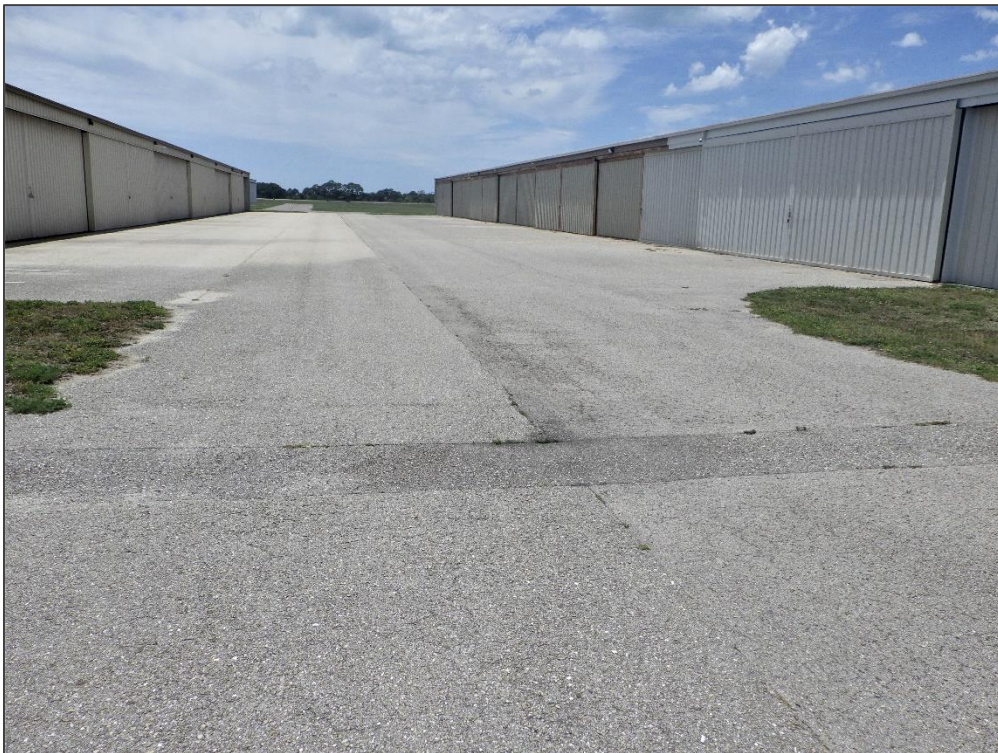
TL T-HANG, Section 710, Sample Unit 150 – Patching
