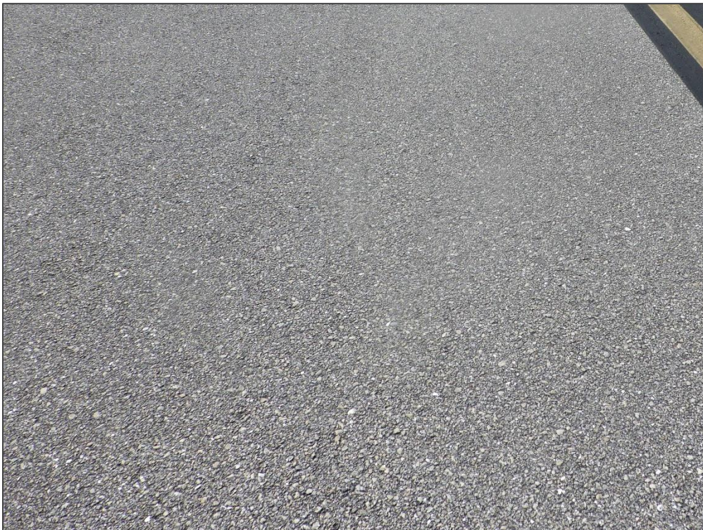
TW D, Section 410, Sample Unit 420 – Weathering
