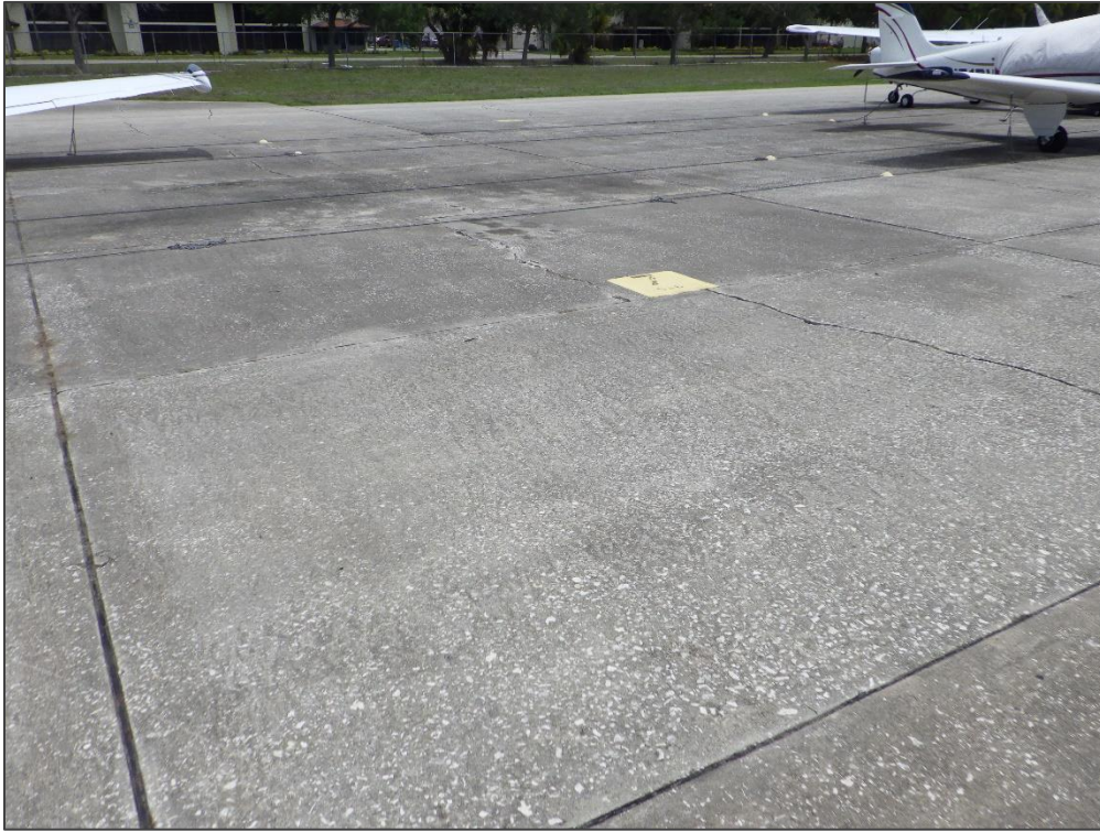
AP, Section 4105, Sample Unit 513 – Linear Cracking
