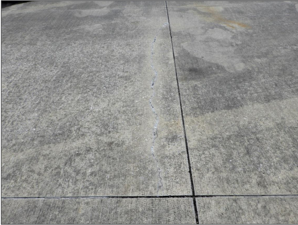
AP TERM, Section 4120, Sample Unit 304 – Linear Cracking
