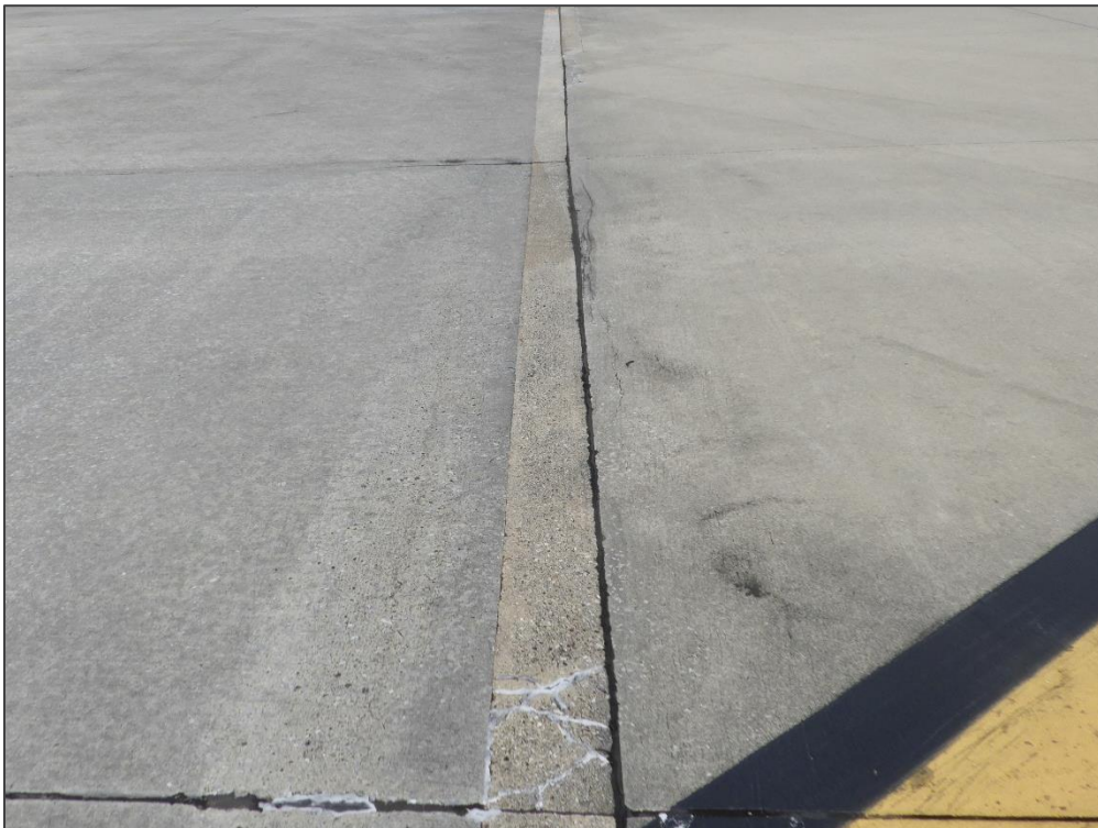
AP TERM, Section 4120, Sample Unit 450 – Large Patch
