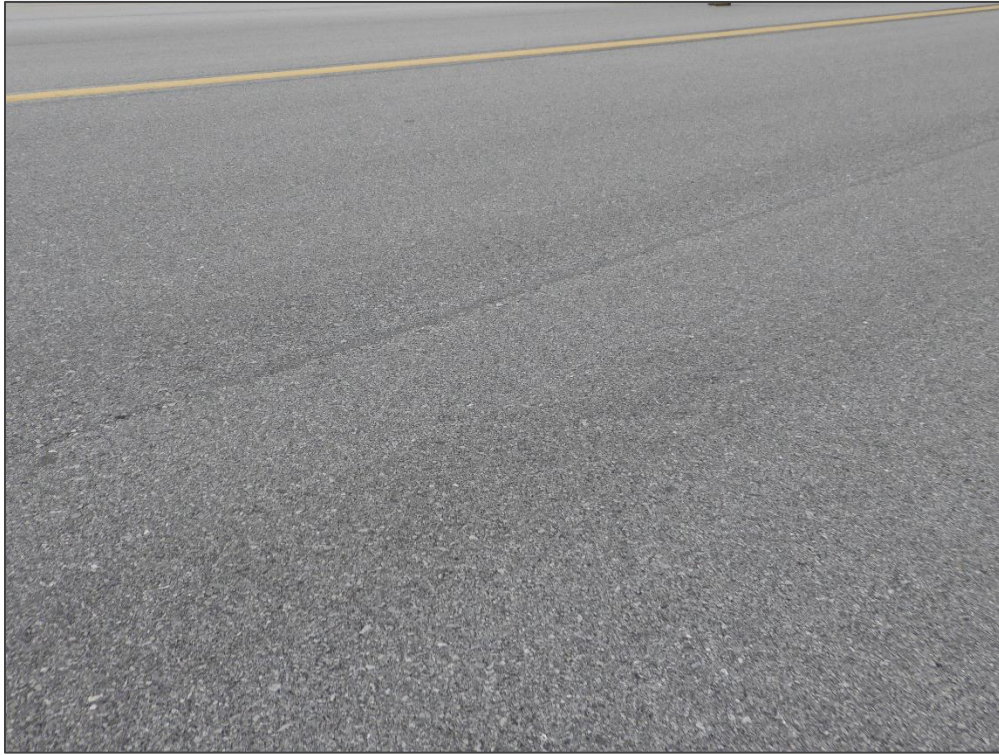
TW D1, Section 105, Sample Unit 114 – Rutting
