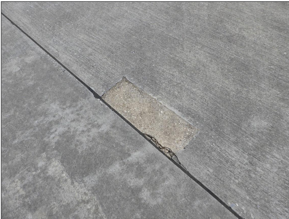
AP TERM, Section 4115, Sample Unit 512 – Small Patch
