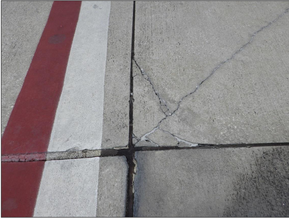
AP TERM, Section 4110, Sample Unit 153 – Linear Cracking and Corner Spall
